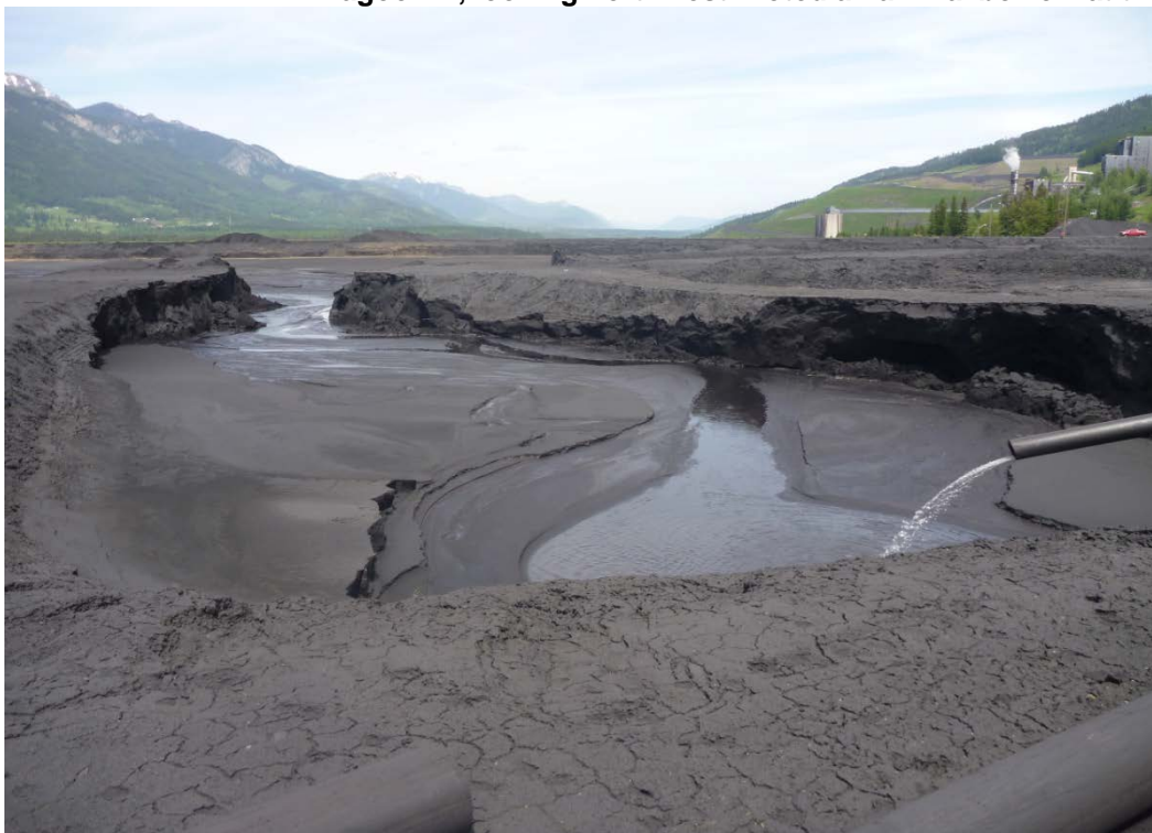
Photograph J - 34: Showing a tailings cell at southeast section of Lagoon D, looking northeast. (Photo P1100742, 2017/06/07)
