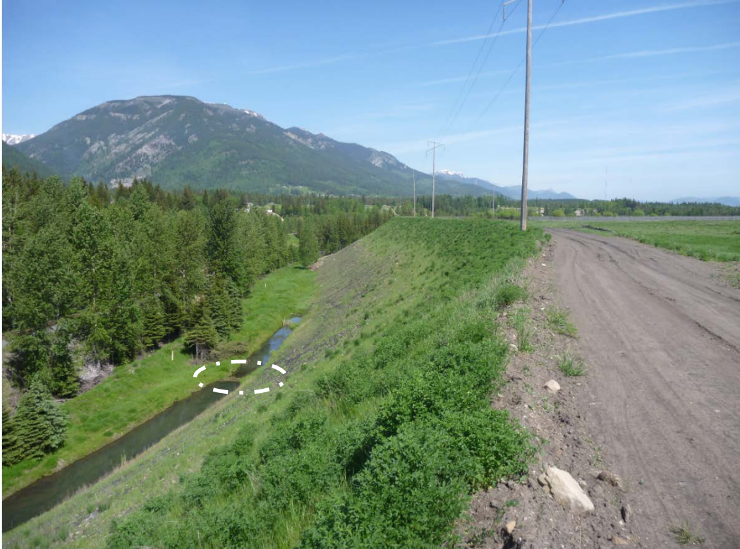
Photograph I - 15: Showing west crest and slope of Lagoon C at southwest corner, looking northwest. Noted beaver activities at the pond (Photo No. P1100644, 2017/06/07).
