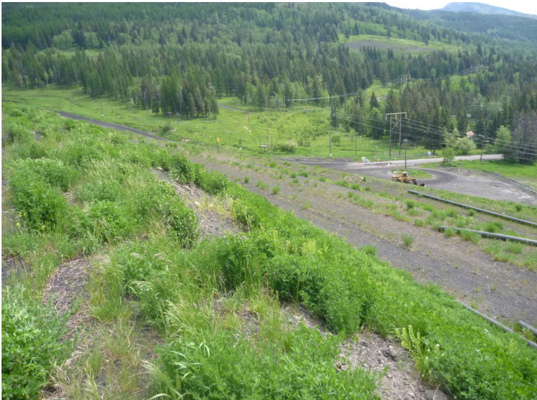
Photograph J - 28: Showing the crest shoulder at the south corner of Lagoon D, looking southeast. (Photo P1100733, 2017/06/07).
