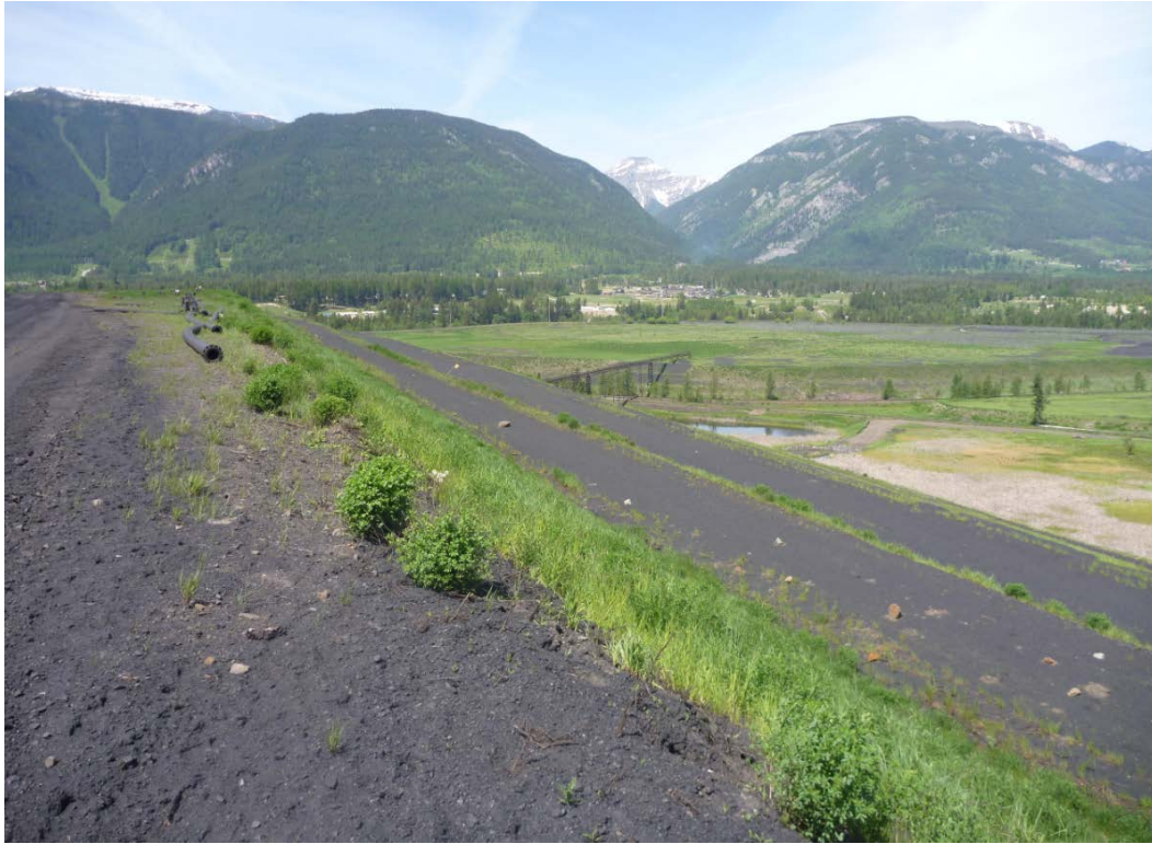
Photograph J - 9: Showing the north crest at east end of Lagoon D, looking west. (Photo P1100689, 2017/06/06)
