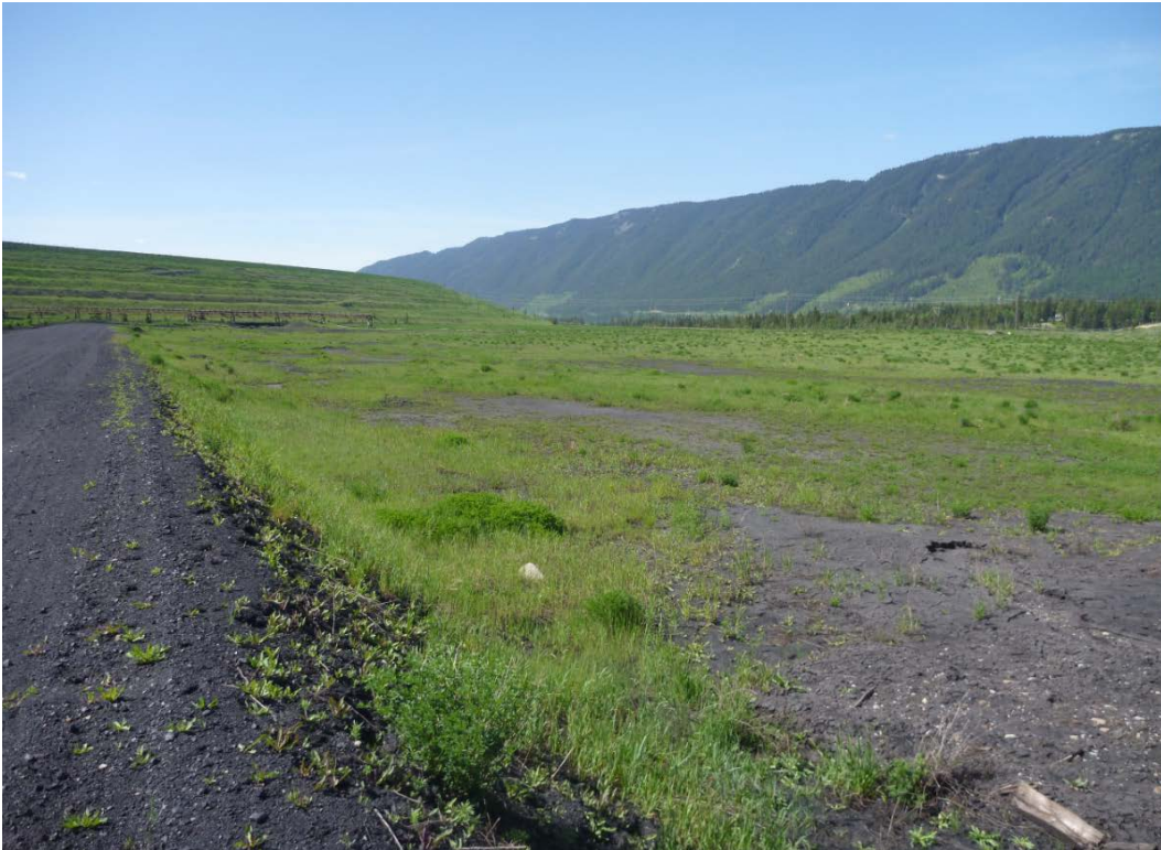
Photograph I - 7: Showing the crest and upstream from the north end of Lagoon C, looking south. (Photo No. P1100611, 2017/06/07)
