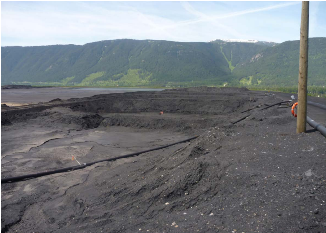
Photograph J - 7: Showing an upstream tailings cells at the northeast corner of Lagoon D, looking west. (Photo P1100684, 2017/06/06)
