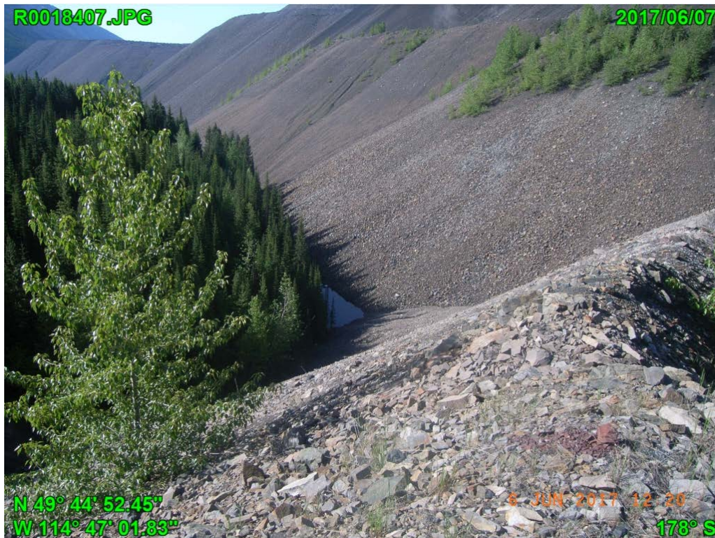
Photograph F - 20: Showing toe of Cowboy dump looking south. Note toe is located approximately 450 m downstream of crest centerline.
