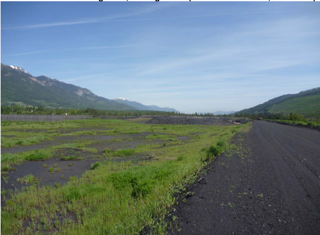
Photograph I - 8: Showing the crest and upstream at the north end of Lagoon C, looking north. (Photo No. P1100615, 2017/06/07)
