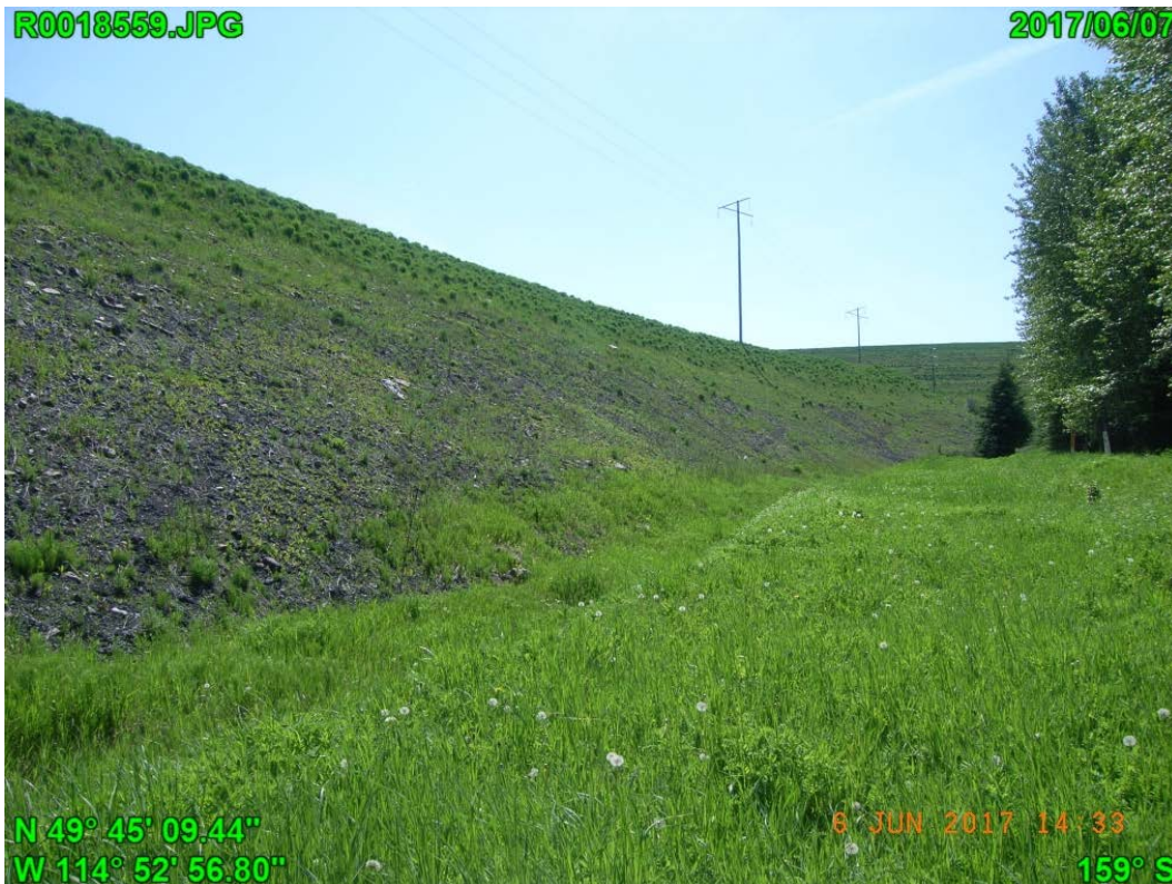
Photograph I - 16: Showing west slope and toe of Lagoon C, looking southeast.
