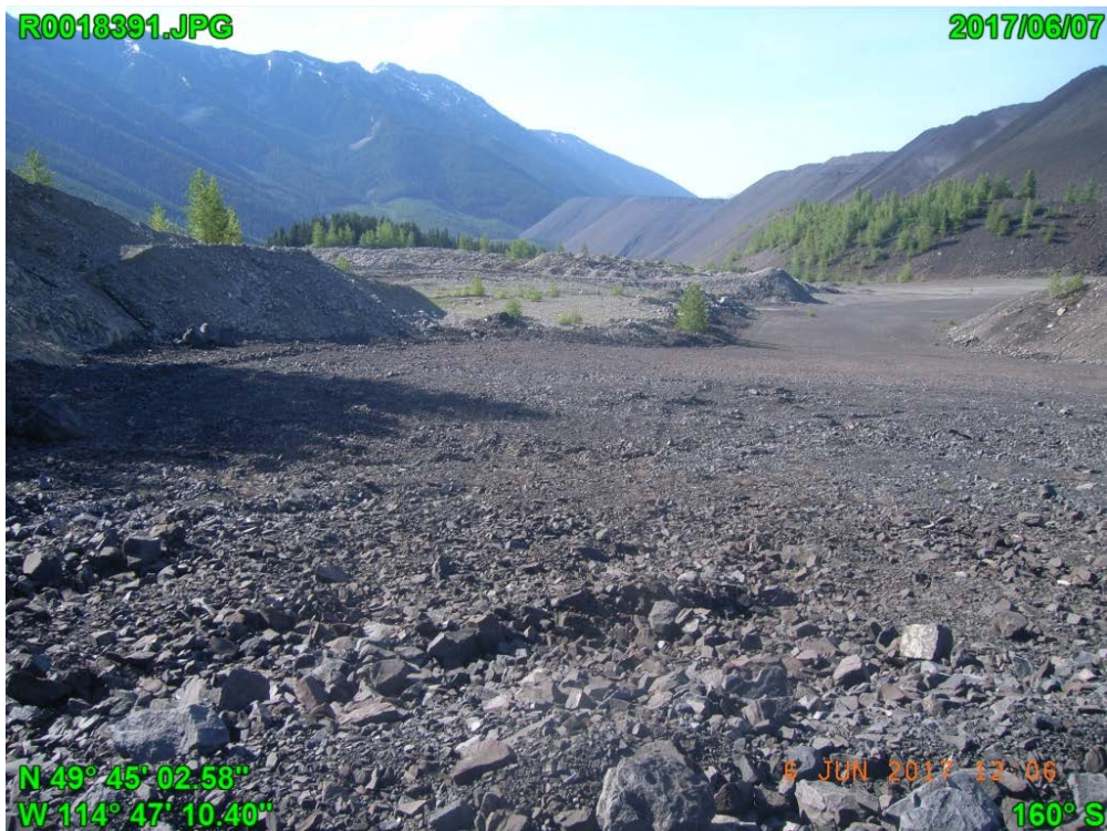
Photograph F - 18: Showing downstream slope, east abutment and toe looking south.
