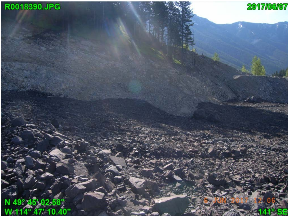
Photograph F - 17: Showing east abutment at WTFF downstream slope, looking southeast.
