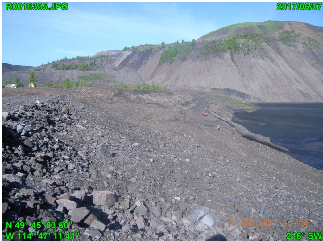
Photograph F - 6: Showing the south abutment, looking southwest from east abutment.
