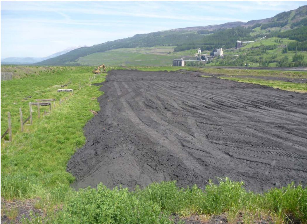
Photograph J - 24: Showing tailings placement on the surface at the west corner of Lagoon D, looking north. (Photo P1100717, 2017/06/06)
