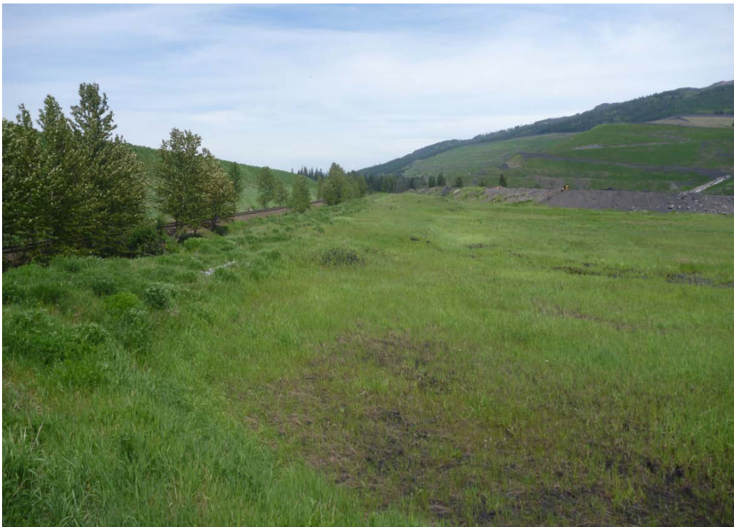
Photograph H - 10: Showing west surface of Lagoon B, view from southwest corner, looking north. (Photo No. P1100769, 2017/06/07)
