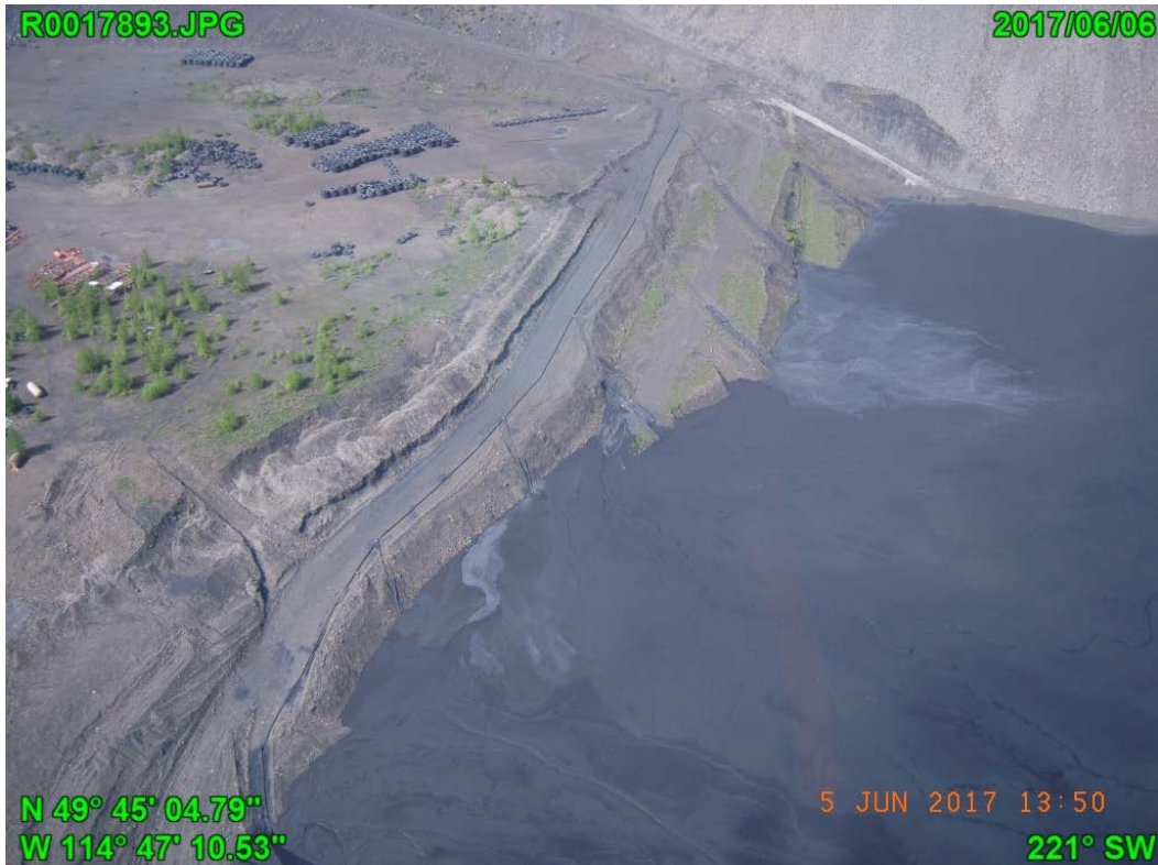
Photograph F - 3: Showing an aerial view of tailings pipelines and tailings beaching at the WTF, looking west.
