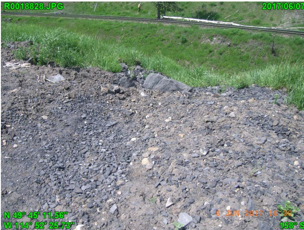
Photograph G - 17: Showing a closer view of the amoured outlet at the west end of the north slope, looking northeast.
