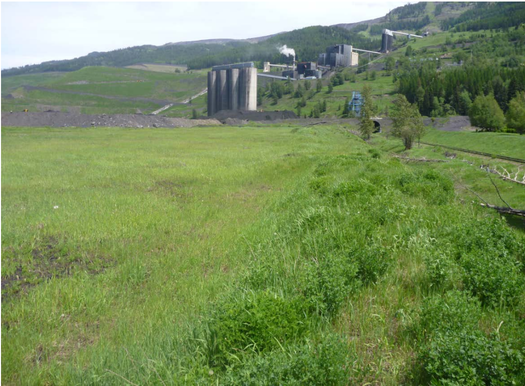
Photograph H - 11: Showing south surface of Lagoon B, view from southwest corner, looking northeast. (Photo No. P1100767, 2017/06/07)
