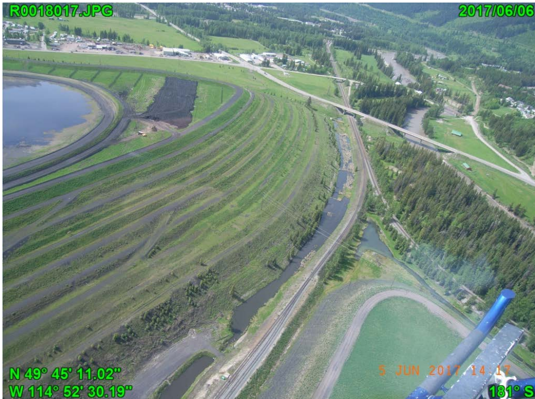
Photograph J - 4: Showing surface of the east corner and west end of the north slope of Lagoon D, looking southwest.
