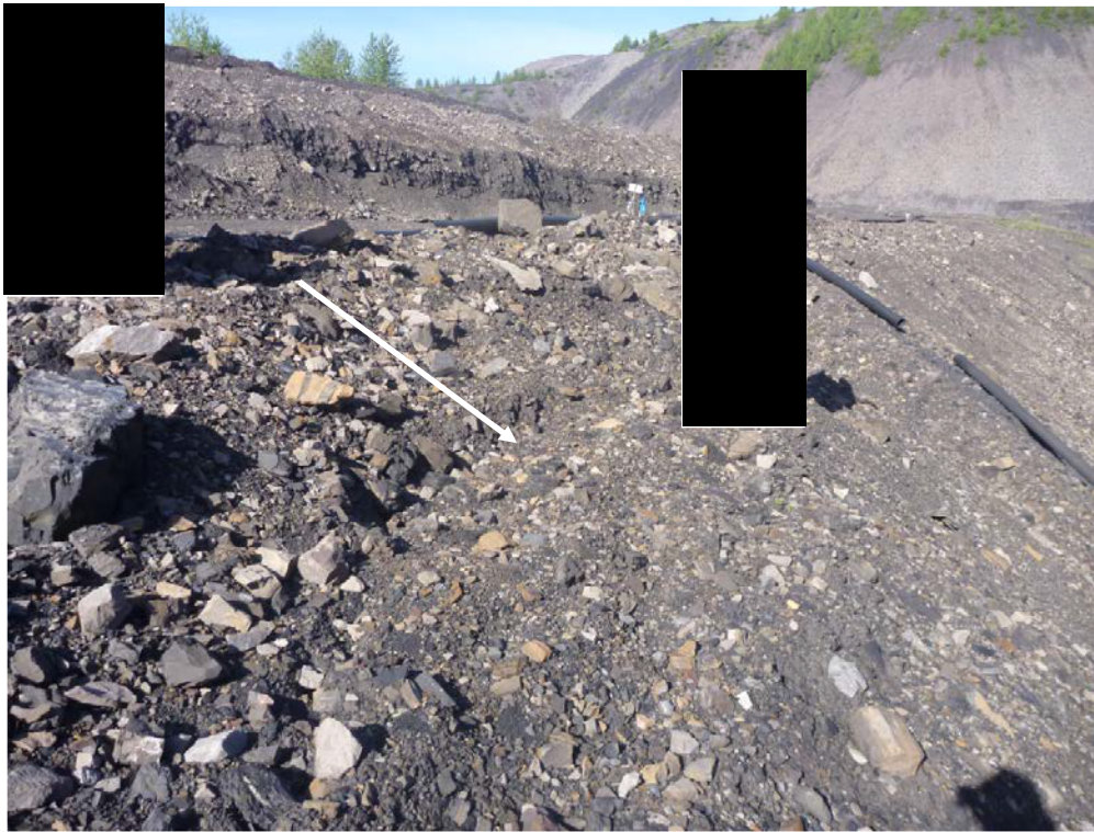
Photograph F - 19: Showing a longitudinal cracking around spigot 5 (Photo P1100577, 06/06/2017).
