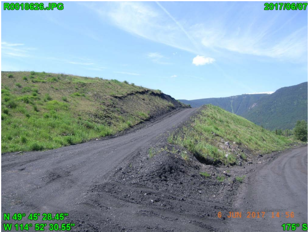
Photograph I - 29: Showing the toe of northeast corner of Lagoon C, looking west.
