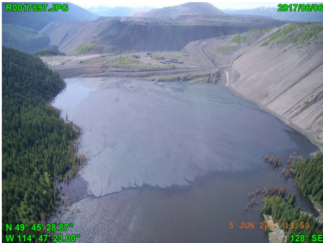
Photograph F - 2: Showing aerial overview of upstream of WFTF, looking south.
