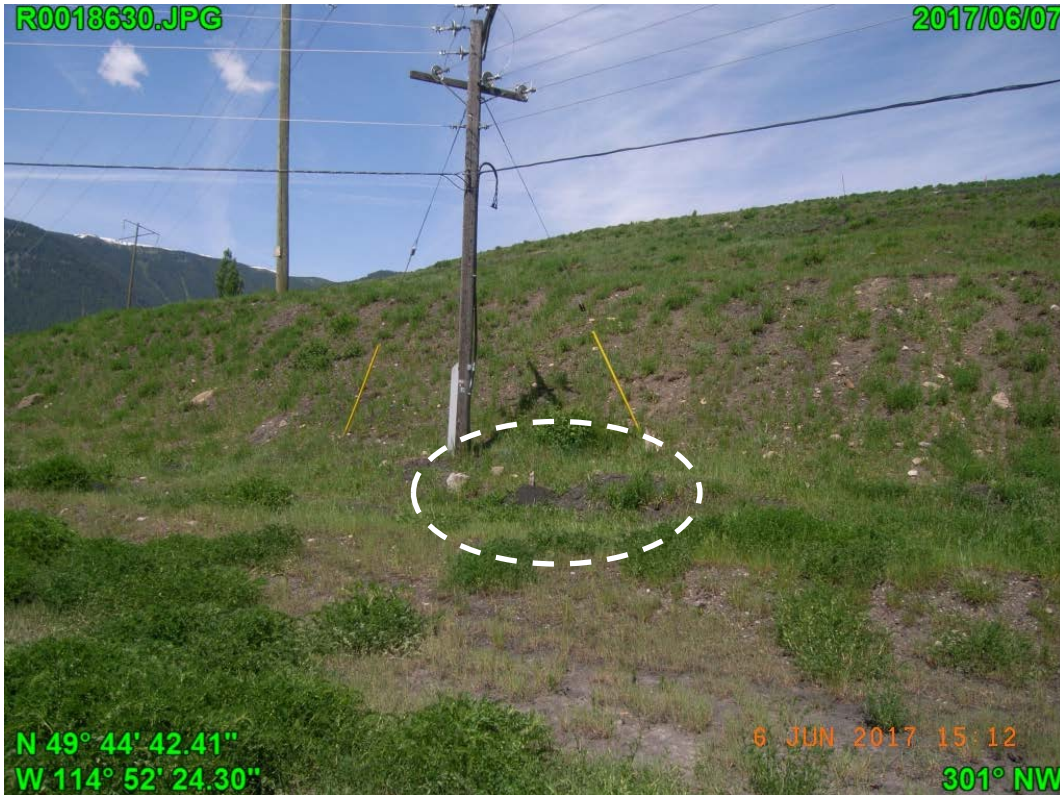
Photograph J - 33: Showing the toe and lower south slope at south corner of Lagoon D, looking northwest. Noted an animal burrow at the toe.
