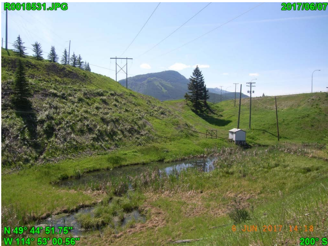
Photograph J - 25: Showing the toe at the west corner of Lagoon D, looking southwest.
