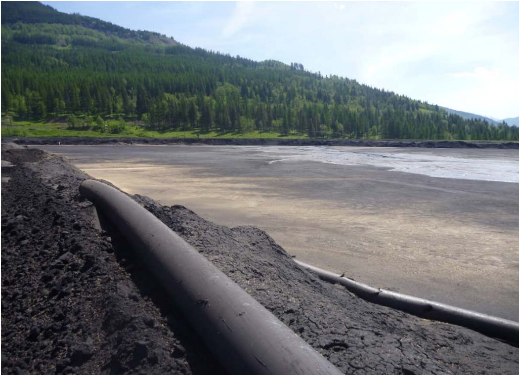
Photograph J - 21: Showing upstream tailings beach at the north section of Lagoon D, looking east. (Photo P1100702, 2017/06/06)
