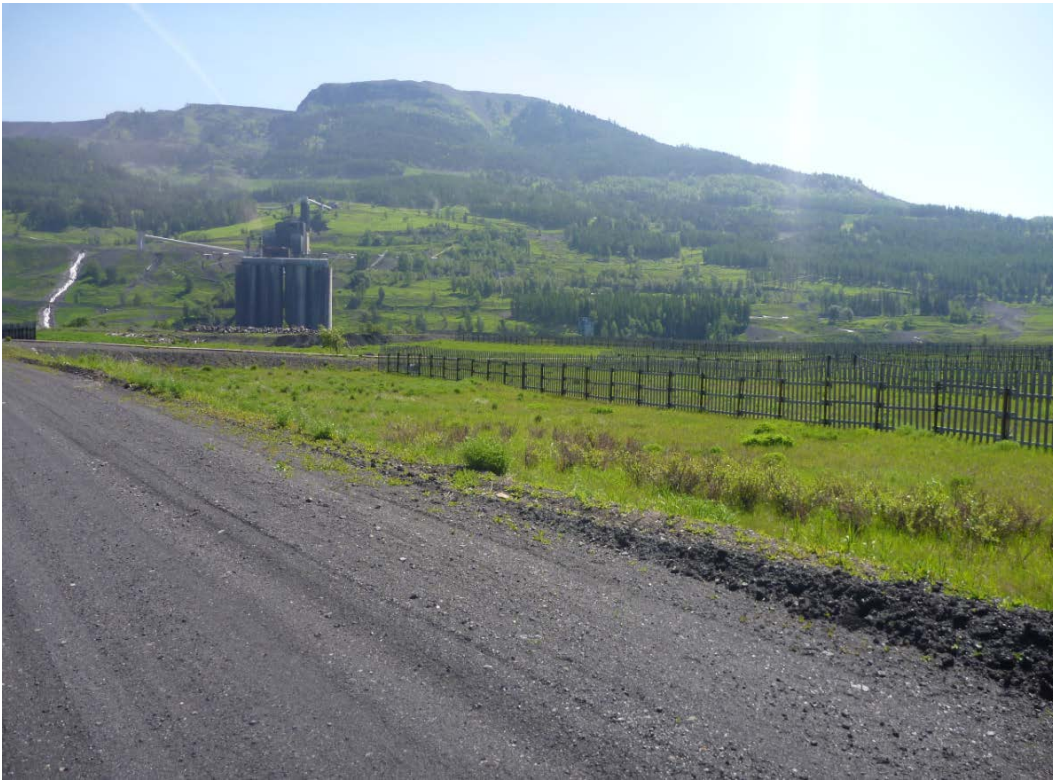
Photograph I - 25: Showing crest and upstream at the northwest corner of Lagoon C, looking northeast. (Photo No. P1100670, 2017/06/07)
