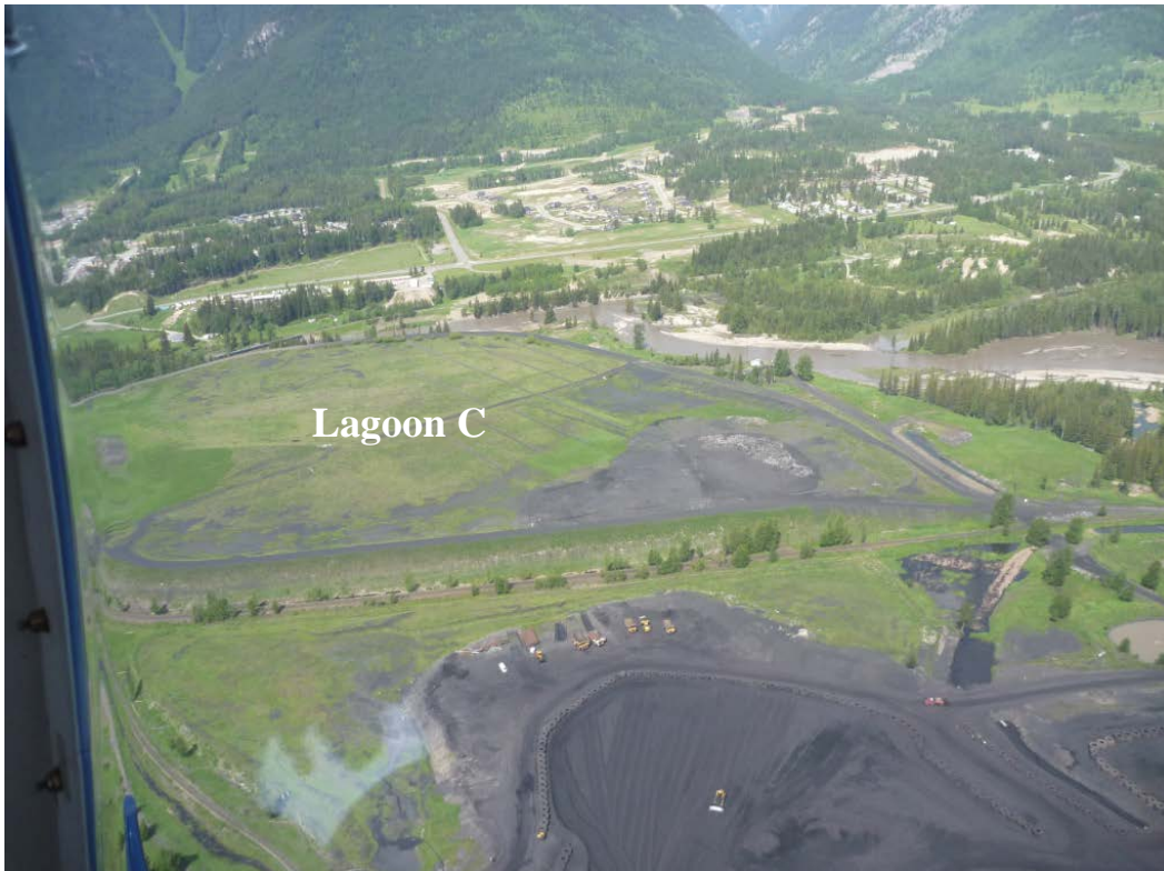
Photograph I - 4: Showing aerial overview of Lagoon C, looking west. (Photo No. P1100452, 2017/06/06)
