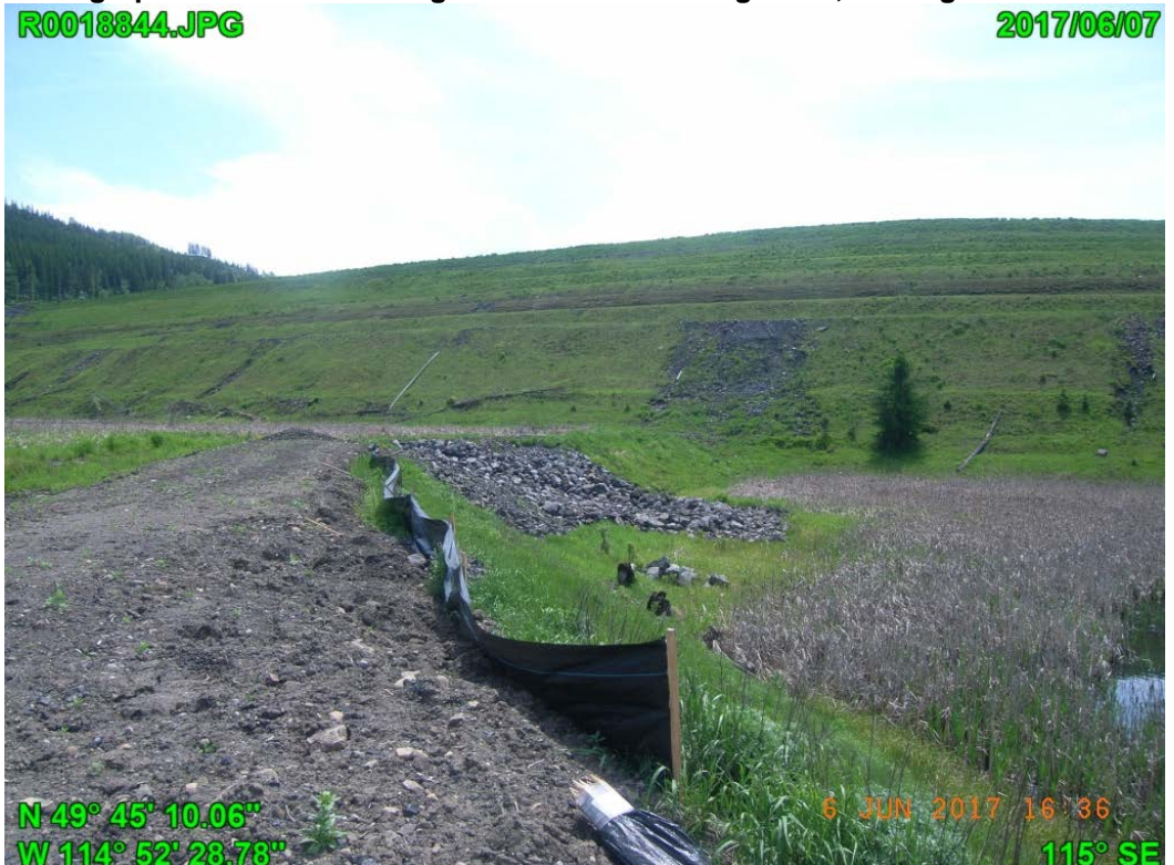
Photograph G - 4: Showing west berm and the spillway, looking southeast.
