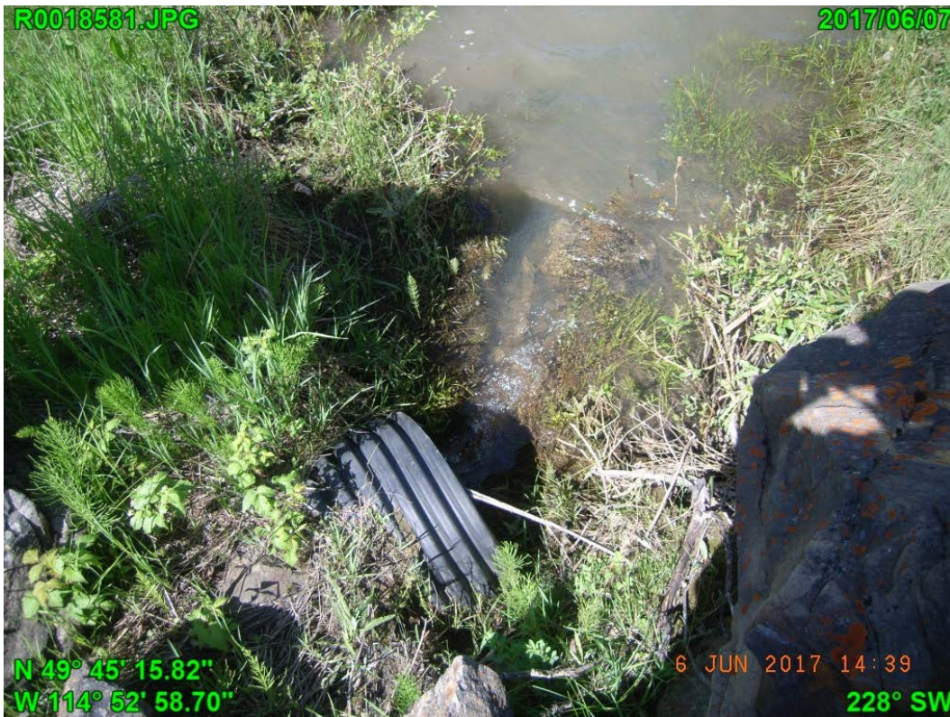
Photograph I - 20: Showing discharge outlet at the west slope toe of Lagoon C.
