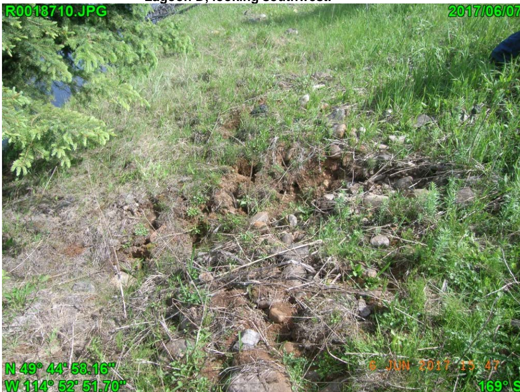
Photograph J - 20: Showing an animal activity at the toe of the north slope of Lagoon D, looking northwest.
