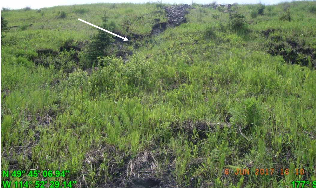
Photograph J - 13: Showing erosion gully at lower north slope, looking south up from the toe.
