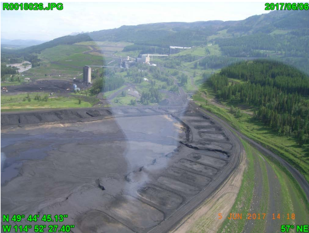
Photograph J - 6: Showing surface of the east corner and east end of the south slope of Lagoon D, looking northeast.
