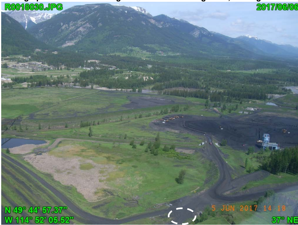
Photograph G - 2: Showing an overview of the Lagoon A. Noted the Cossarini Creek inflow to east side of Lagoon A through 2 culverts, looking northwest.
