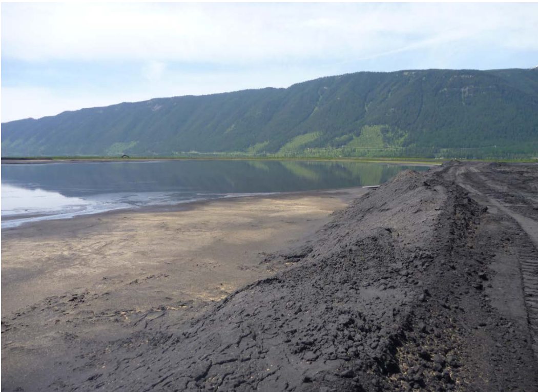
Photograph J - 22: Showing upstream tailings beach at the north section of Lagoon D, looking west. (Photo P1100703, 2017/06/06)
