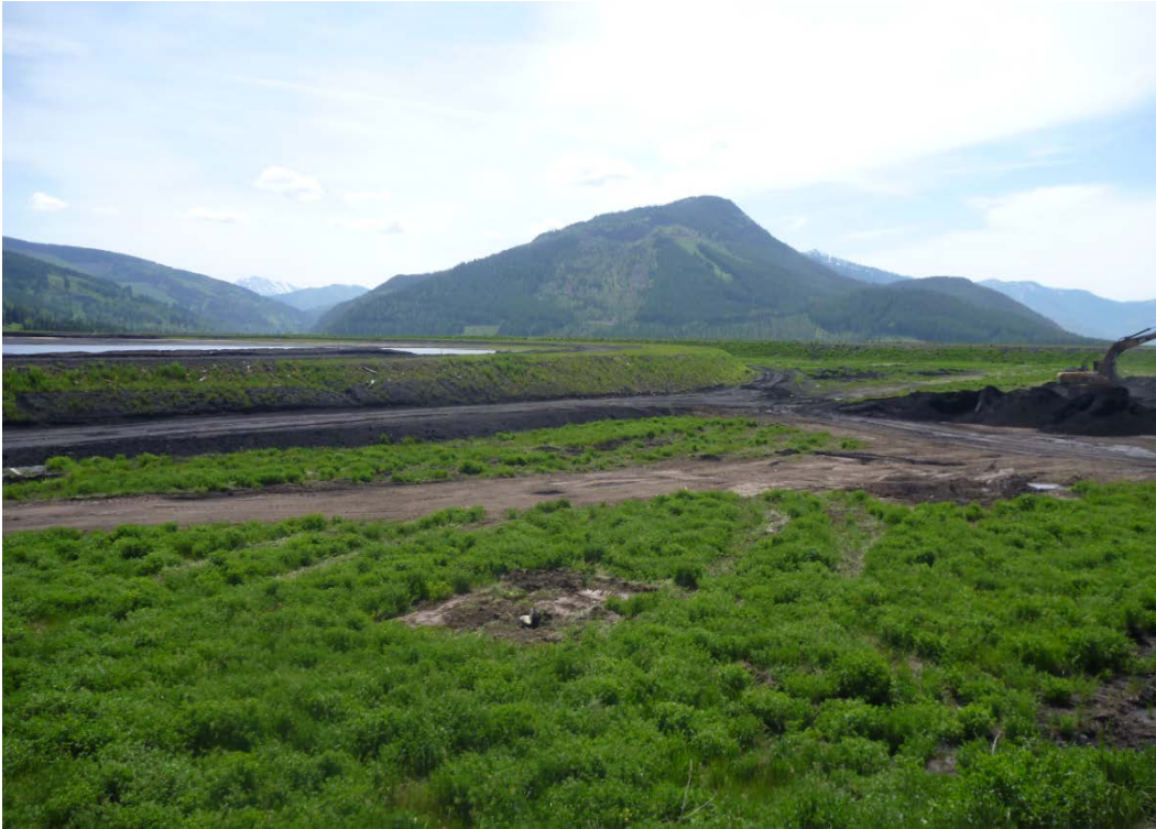
Photograph J - 23: Showing surface of the west corner of Lagoon D, looking south. Noted active tailings deposition on the surface (Photo P1100719, 2017/06/06)
