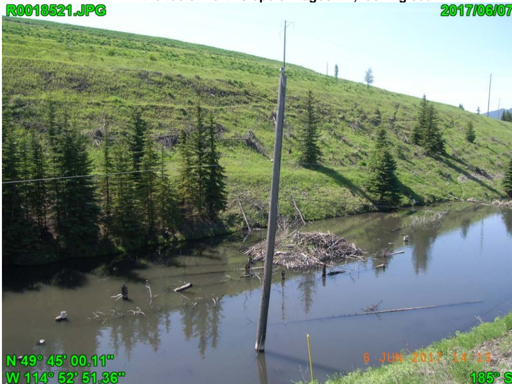
Photograph J - 18: Showing the toe at west end of the north slope of Lagoon D, looking southwest. Noted beaver activities within this area.
