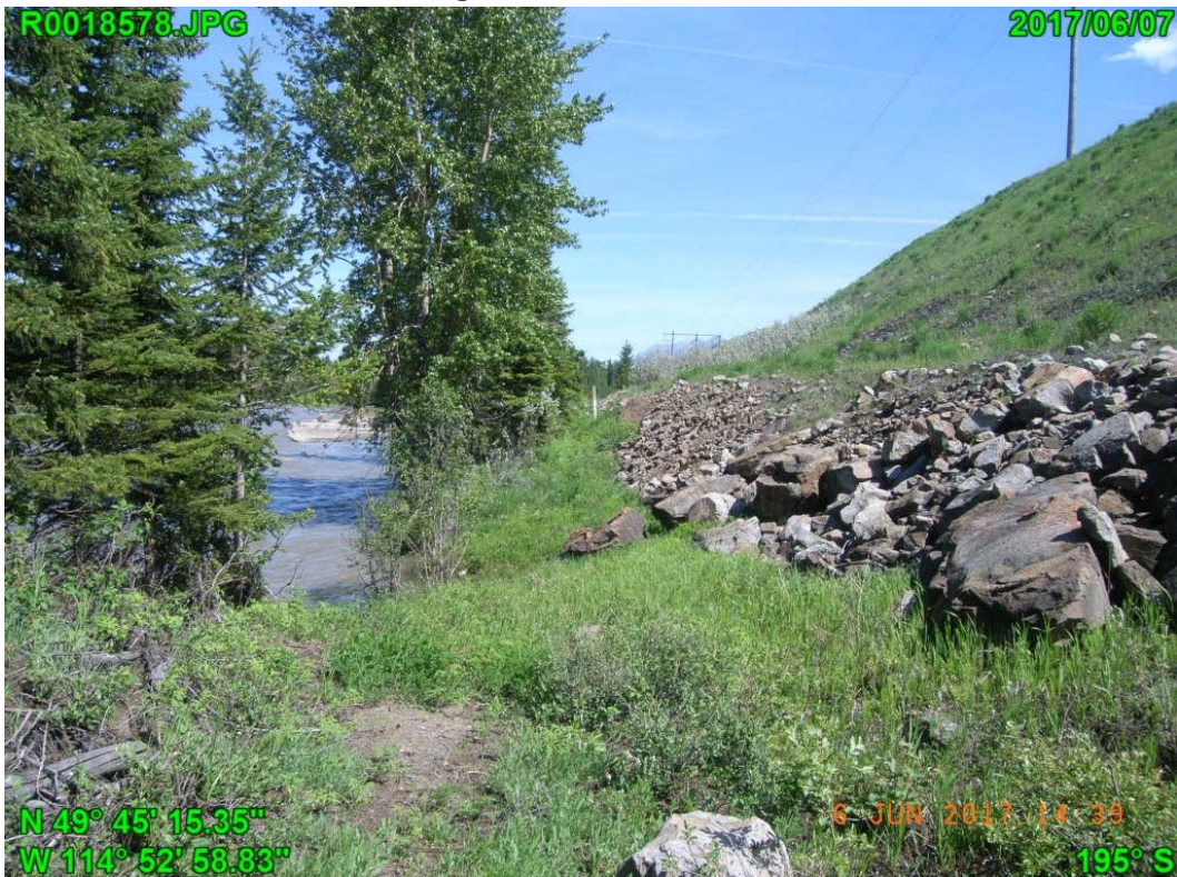
Photograph I - 18: Showing west slope and toe of Lagoon C, showing erosion protection, looking north.
