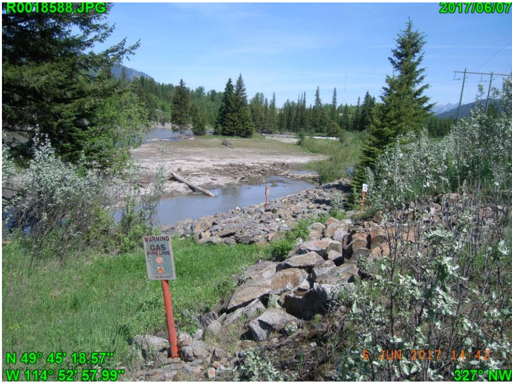
Photograph I - 21: Showing the sign of natural gas line at west slope toe of Lagoon C, looking north.
