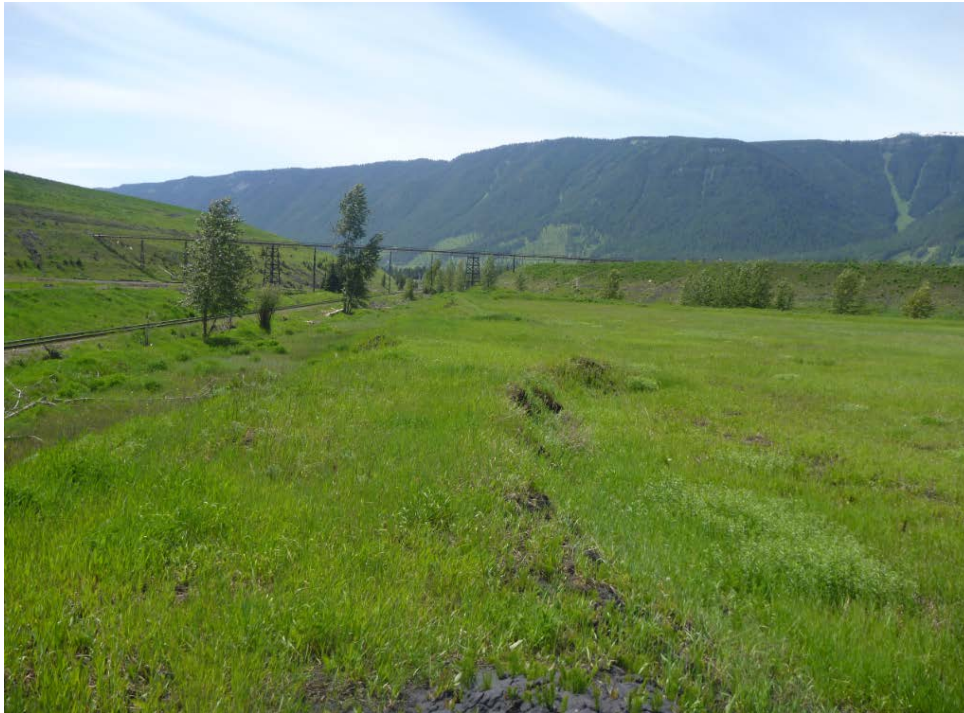
Photograph H - 15: Showing crest and slope on south side of Lagoon B, Looking southwest (Photo No. P1100758, 2017/06/07).
