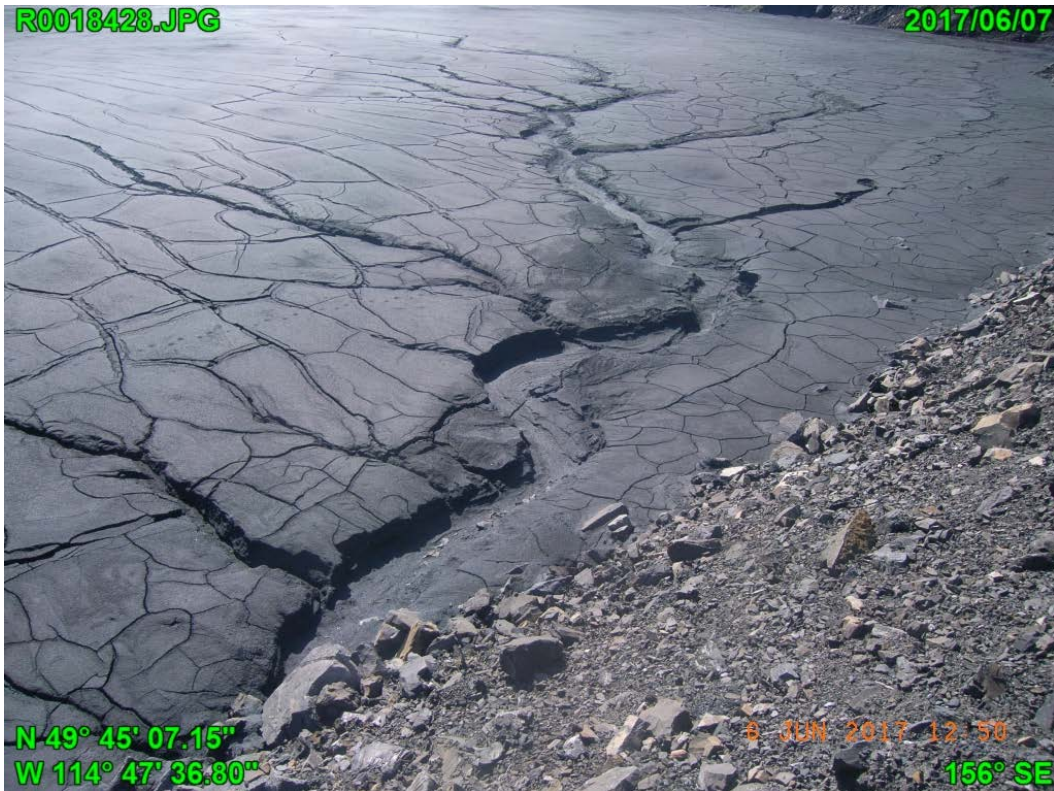
Photograph F - 9: Showing evidence of infiltration on the west side of the WTFF near the Adit dump, looking south.
