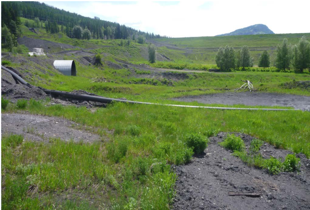
Photograph H - 18: Showing tailings discharge area located at the southeast corner of Lagoon B, looking southeast (Photo No. P1100748, 2017/06/07).
