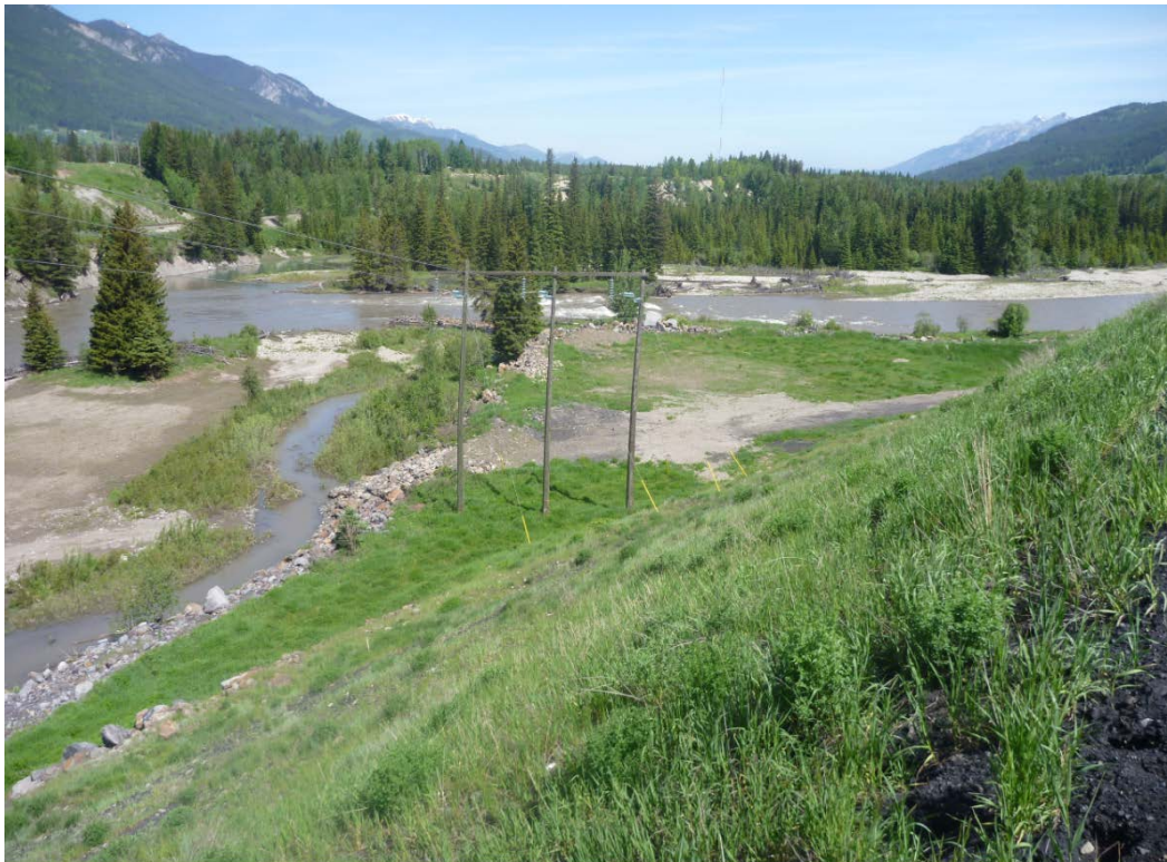
Photograph I - 22: Showing west slope and toe of Lagoon C at northwest corner, looking north. (Photo No.P1100665, 2017/06/07)
