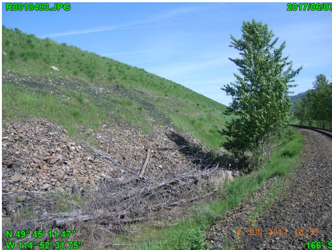
Photograph I - 10: Showing erosion at the south end of the east slope toe of Lagoon C, looking north.
