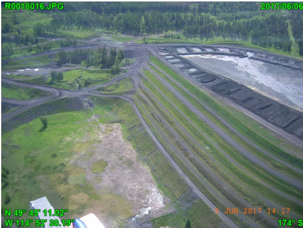
Photograph J - 3: Showing surface of the west corner and east end of the north slope of Lagoon D, looking east.
