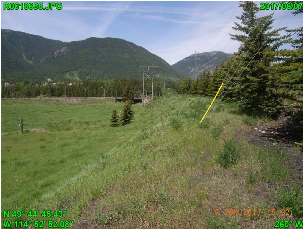
Photograph J - 26: Showing the toe of the dam at west end of Lagoon D, looking northwest.
