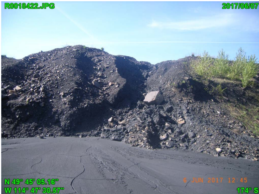
Photograph F - 11: Showing an erosion gully on upstream slope due to tailings discharged from spigot 1 pipe located close to the Adit dump, looking south.
