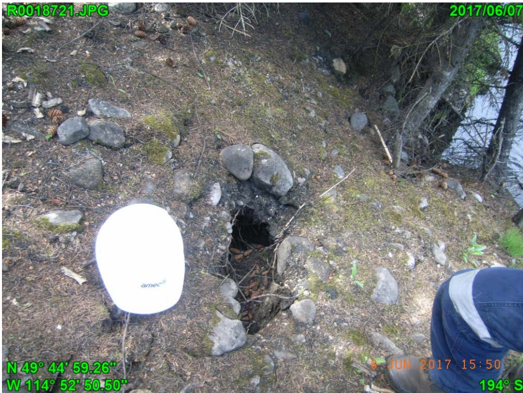
Photograph J - 19: Showing an animal burrow on the toe of north slope of Lagoon D, looking southwest.
