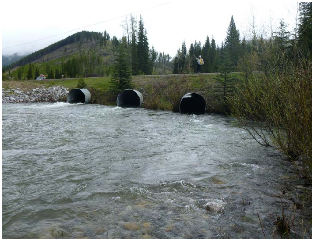
Figure 3.3.24. Ewin Creek Fording Road culvert illustrating fish passage characteristics.
