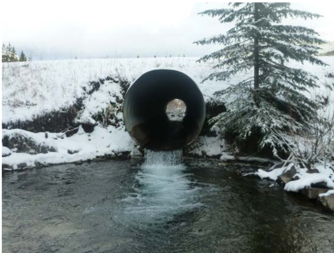
Figure 3.2.13. Chauncey Creek Fording Road culvert illustrating potential upstream passage barrier approximately 900 m upstream from the Chauncey Creek confluence with the upper Fording River.
