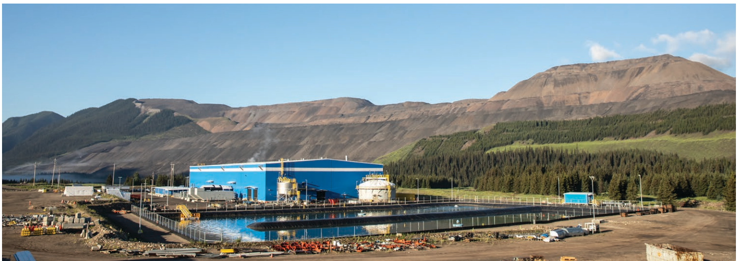
Image: View of the Fording River Operations South Active Water Treatment Facility
