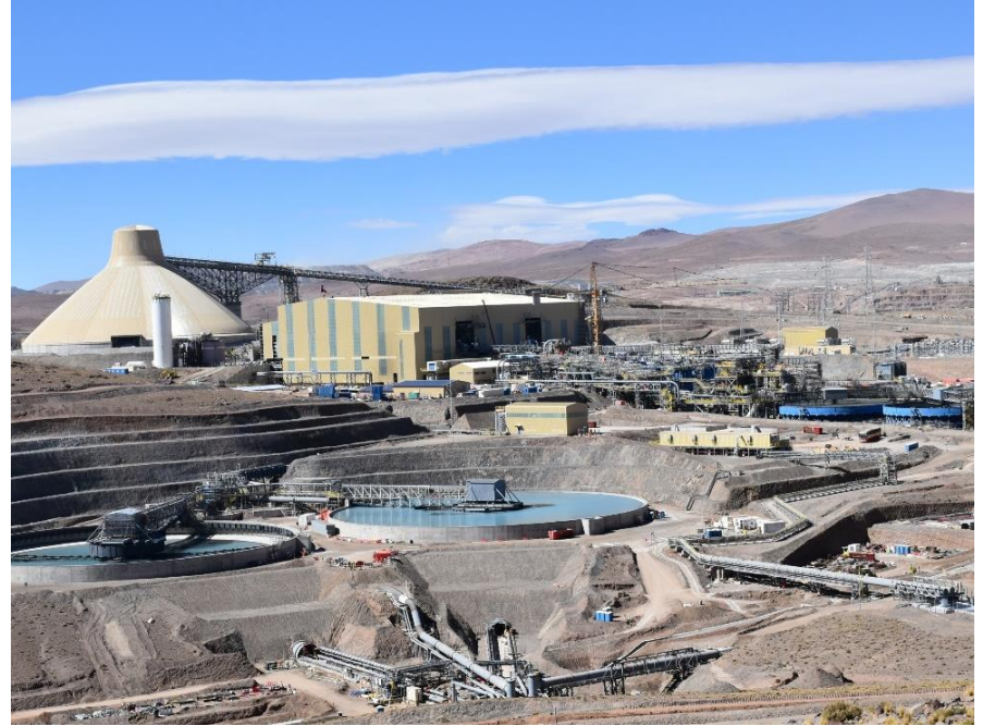
QB Operations site overview, October 2023.
