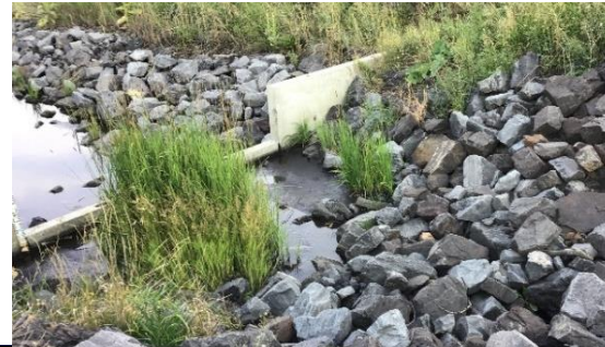
Upstream Aqueduct Pond
