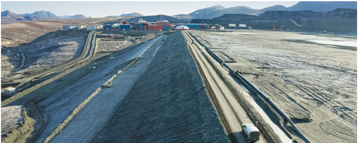
The tailings impoundment dam construction occurs during the summer months.
