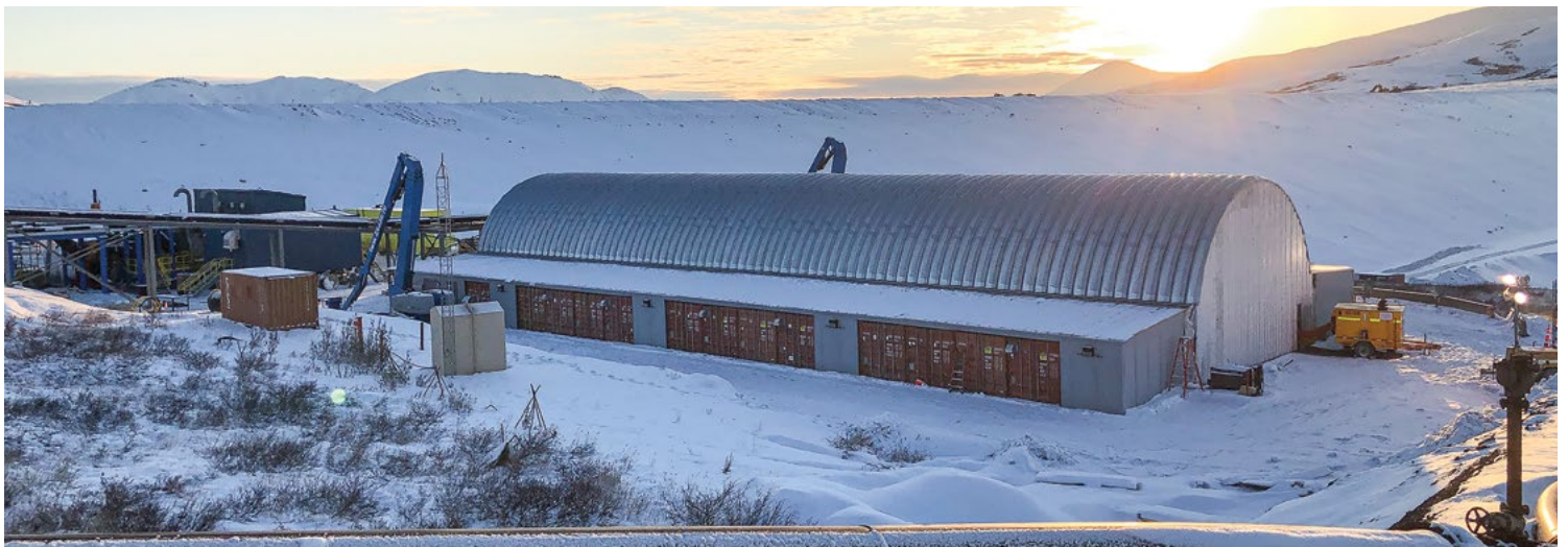
The reverse osmosis plant was built in 2019 and can filter up to 2.8 million gallons of water a day.
