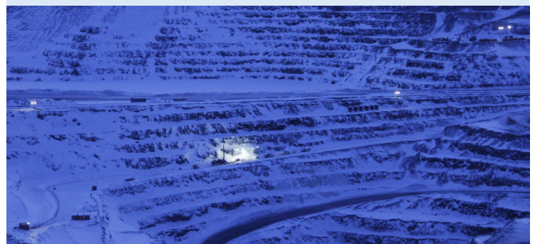
Drilling on the Aqqaluk Pit 775 Ramp
