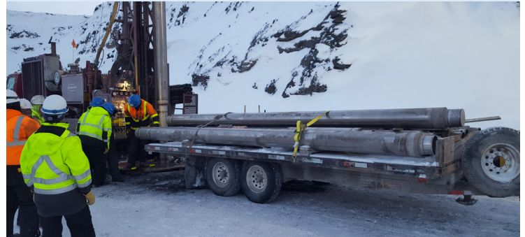
Tuuq Drilling installing the Well Screens
