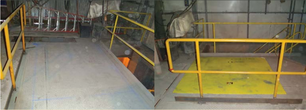
Before: Deck plate above conveyor prior to access door.
