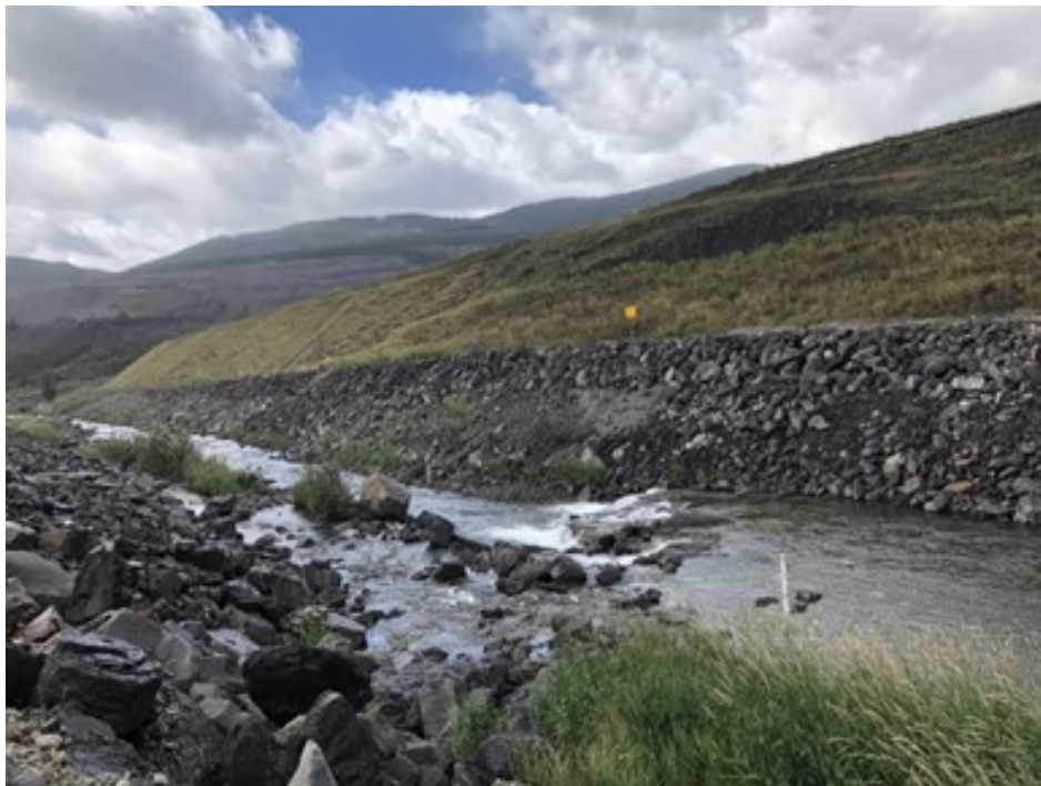
Figure 4. Looking downstream at FR_FRNTP n August 5, 2020.
