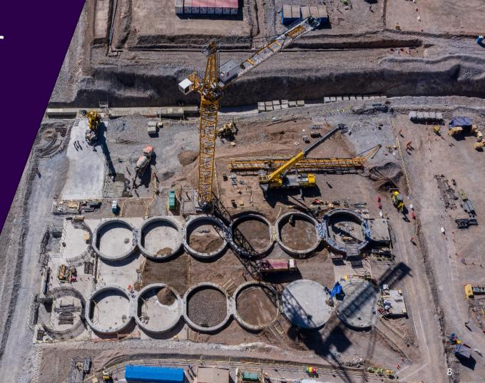
Grinding Area – Foundations for SAG mills (left) and ball mills (right)
