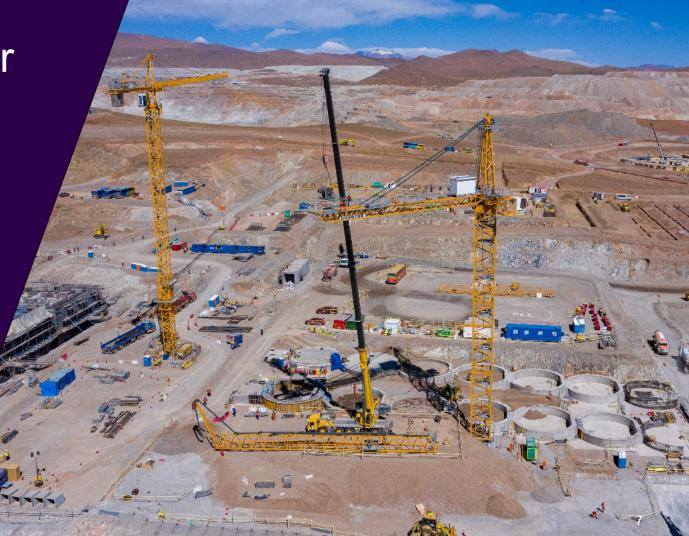
Flotation Area – Foundations for 650m<sup>3</sup> rougher cells
