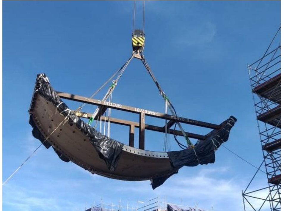
SAG Mill #1 Shell Lift, January 2020
