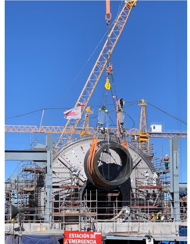
SAG #1 trunnion installation, August 2020
