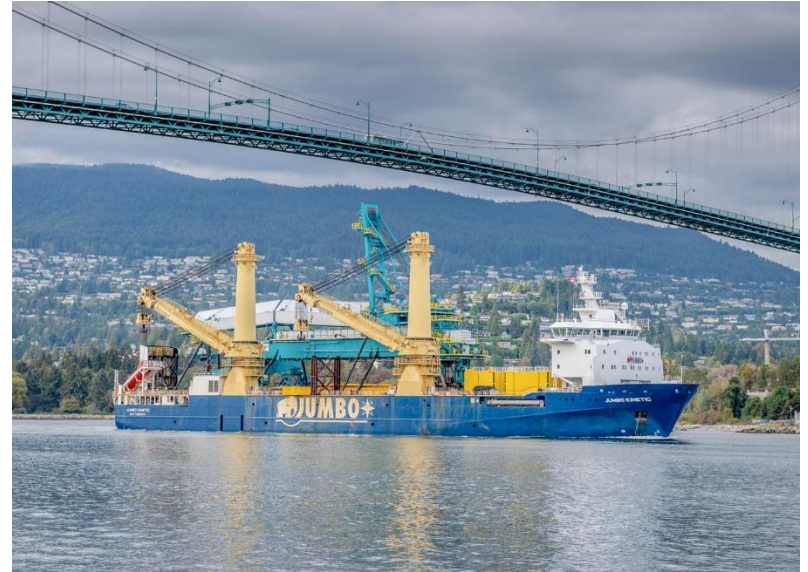
Neptune Terminals' new shiploader crossing under Vancouver's Lions' Gate Bridge, October 8, 2020.
