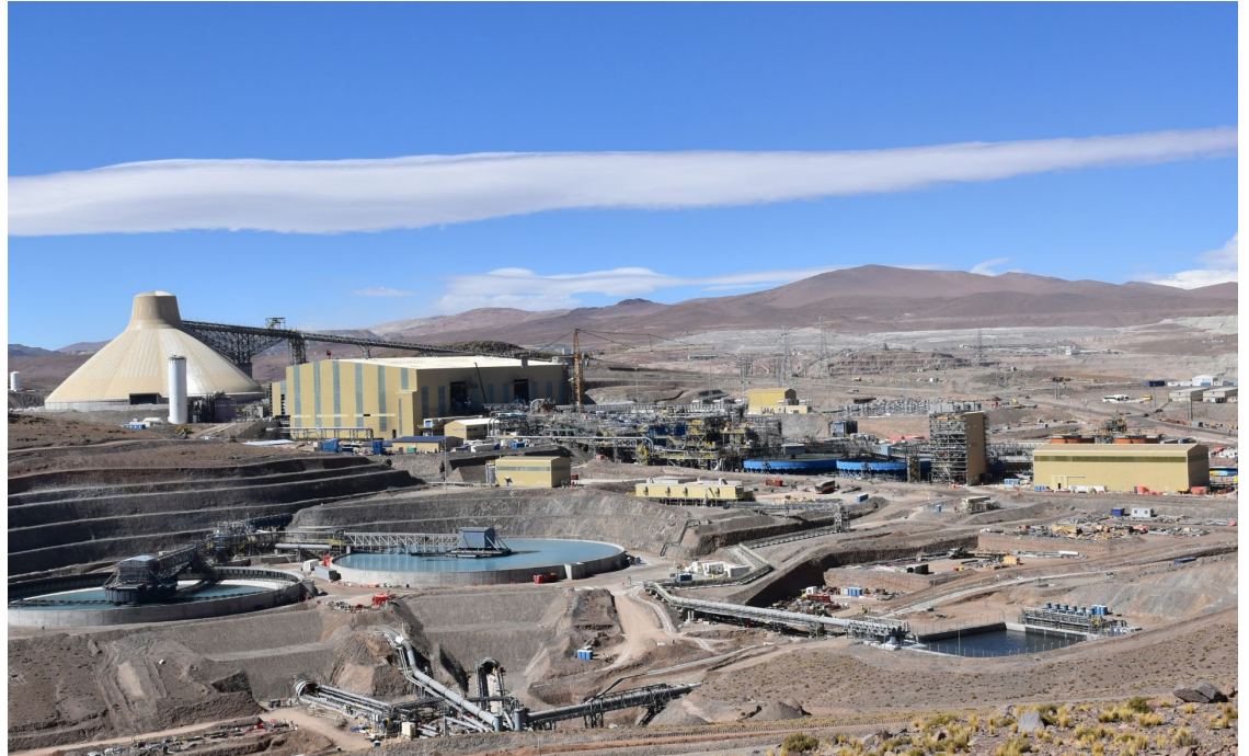
Ore stockpile, grinding building, flotation area, and tailings thickeners.
