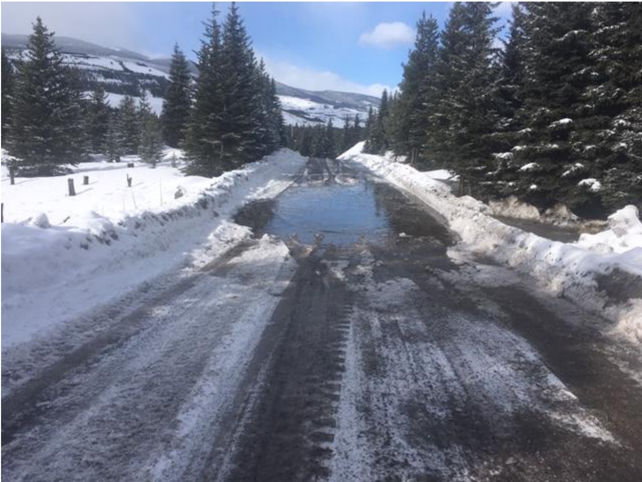
Photograph 1- Unauthorized Discharge located in the low lying depression on the Swift Creek access road.
