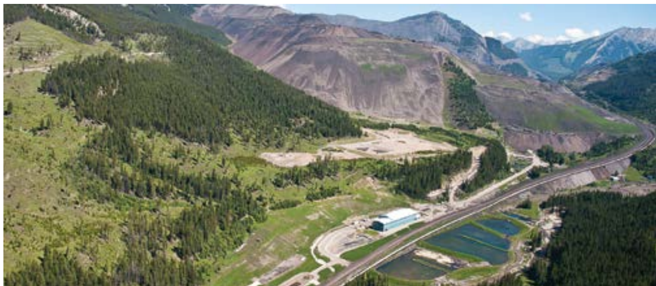
Figure 9-3. The active water treatment facility at Teck's Line Creek Operations.
