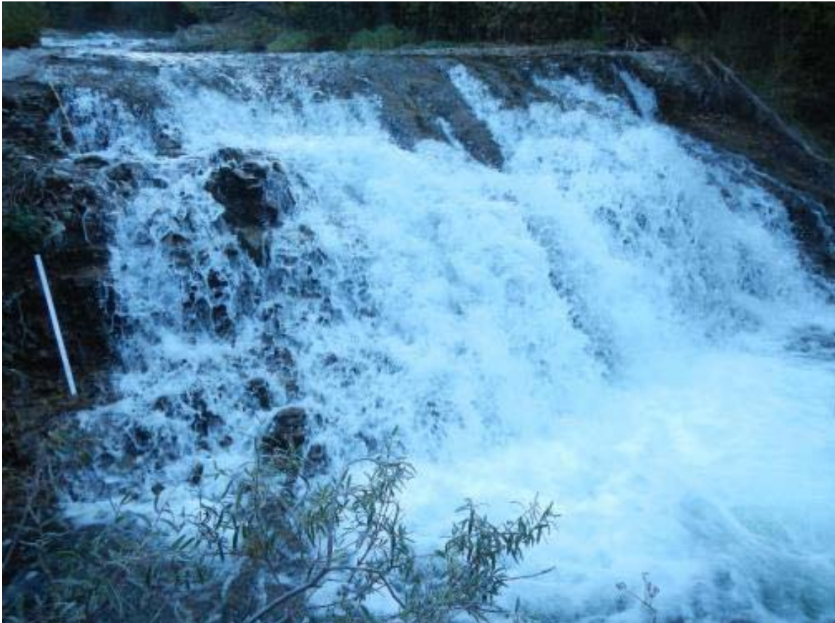
Photo 7.1: Upstream view of the 3 m high waterfall below the Grave Lake confluence in Grave Creek (Lotic 2015a).
