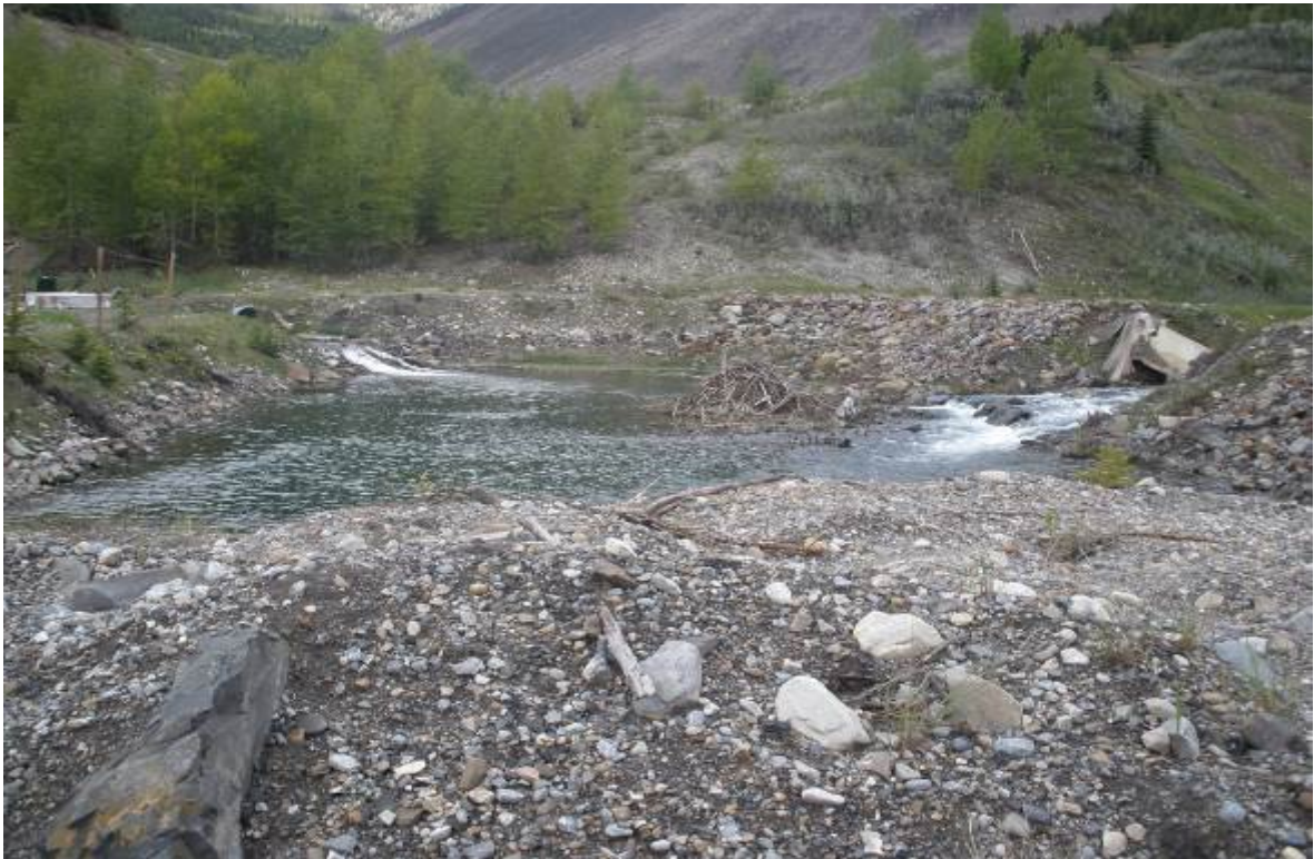
Photo 4.2: Downstream end of the rock drain in Line Creek (Minnow unpublished).
