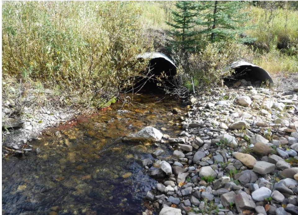
Figure 41. The section of Dry Creek downstream of the two culverts that are considered a fish barrier on June 7, 2016.
