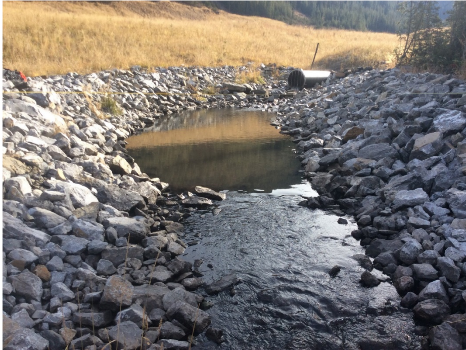
Figure 39. Dry Creek settling pond outlet channel on October 28, 2017.
