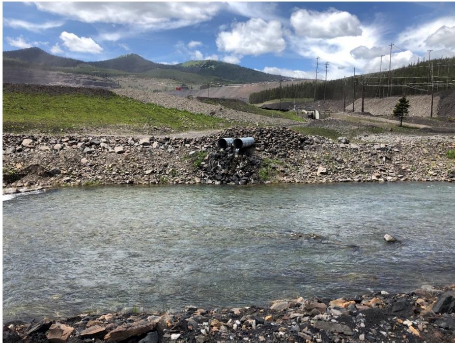
Figure 17. Discharge culverts in Liverpool Sediment Ponds Channel on June 22, 2020.
