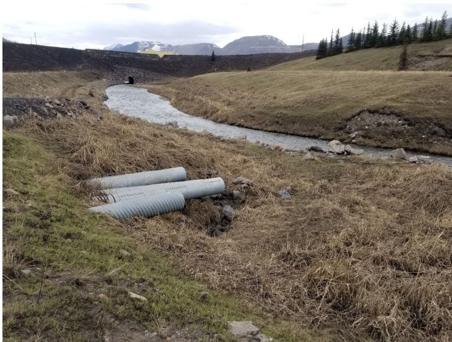
Figure 16 Discharge culverts in Eagle Settling Ponds Channel on May 12, 2020.
