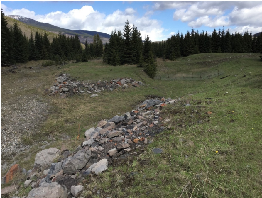
Figure 26. Kilmarnock Phase 1 Discharge Channel and Fording River Side Channel confluence on June 14, 2020.
