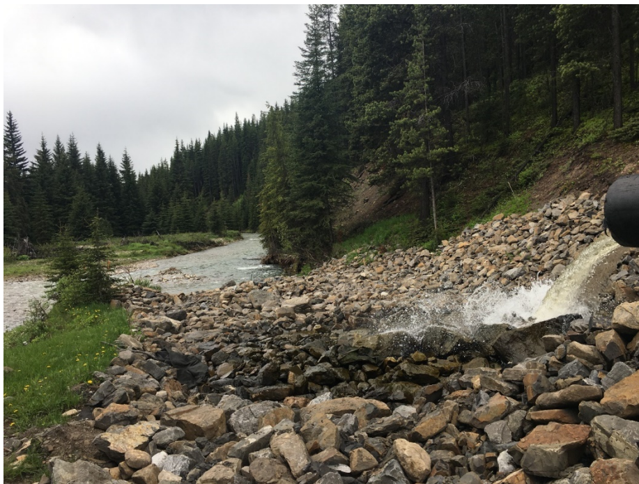
Figure 3 Discharge from Post Ponds Channel on June 17, 2020.
