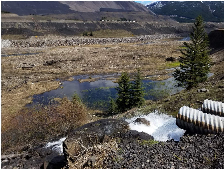
Figure 20. Discharge culvert on Smith Ponds Channel on May 13, 2020.
