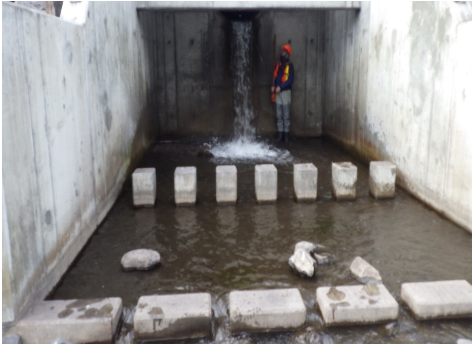
Figure 13. Plunge pool at base of fish exclusion structure at Lake Mountain Creek on October 9, 2018.
