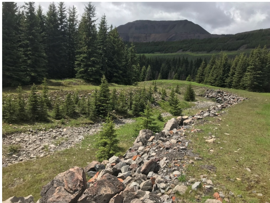
Figure 25. Kilmarnock Phase 1 Discharge Channel on June 14, 2020.
