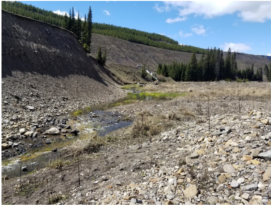
Figure 21. Smith Ponds Channel downstream of culverts on May 13, 2020.
