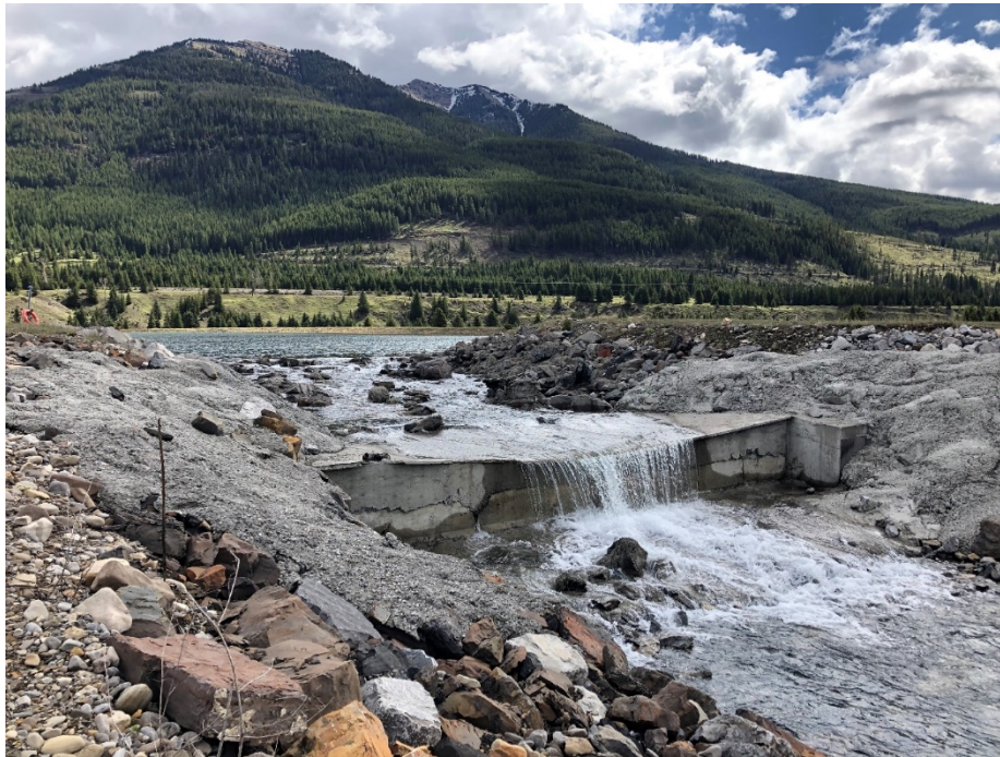
Figure 29. Kilmarnock Creek Phase 2 fish exclusion structure on May 26, 2020.
