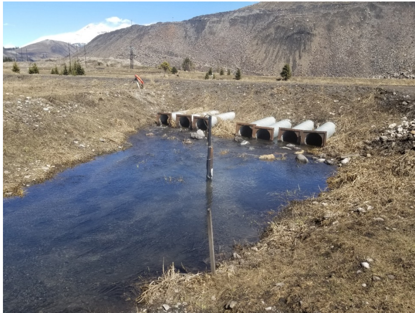
Figure 7. Discharge culverts on Clode Creek on April 28, 2020.
