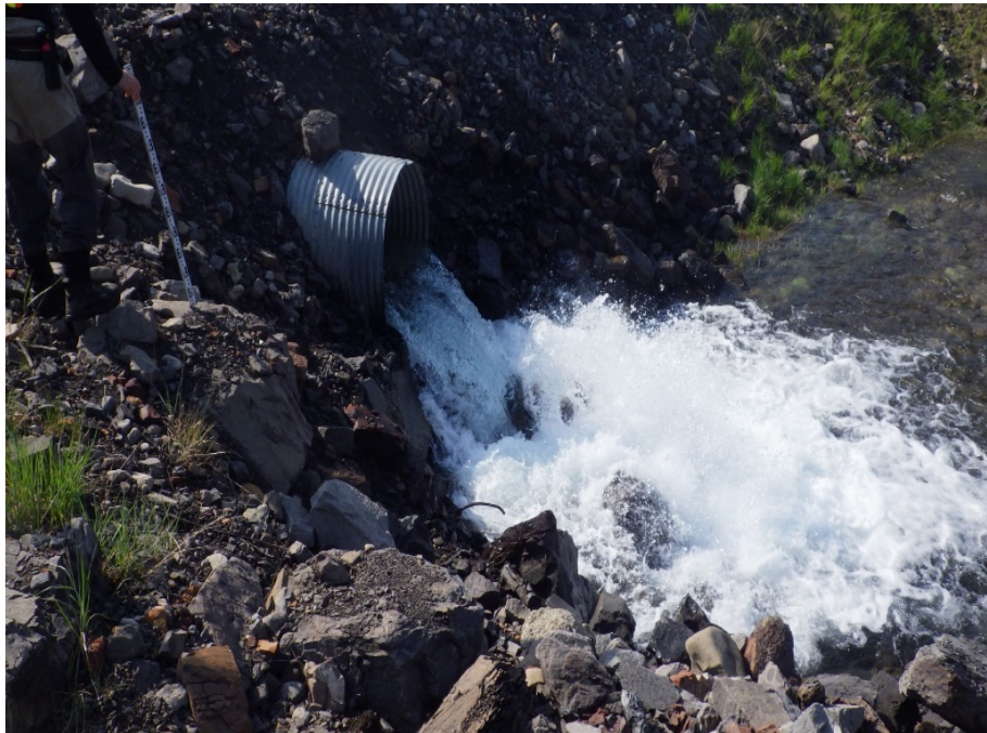
Figure 24. Discharge culvert on Kilmarnock Phase 1 Discharge Channel, June 6, 2018.
