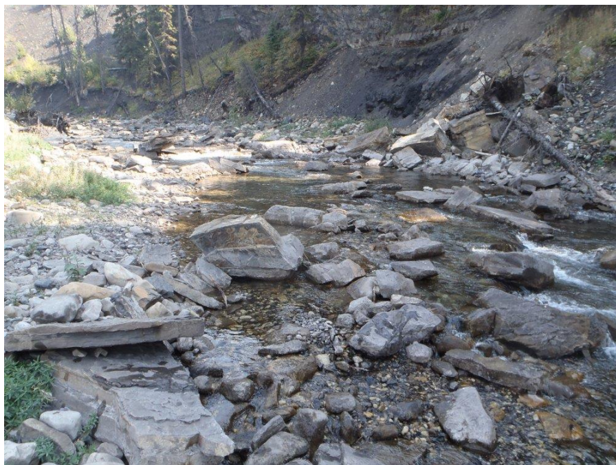
Figure 51. Looking upstream at HEN-CA02 Unit 2 on September 1, 2017.
