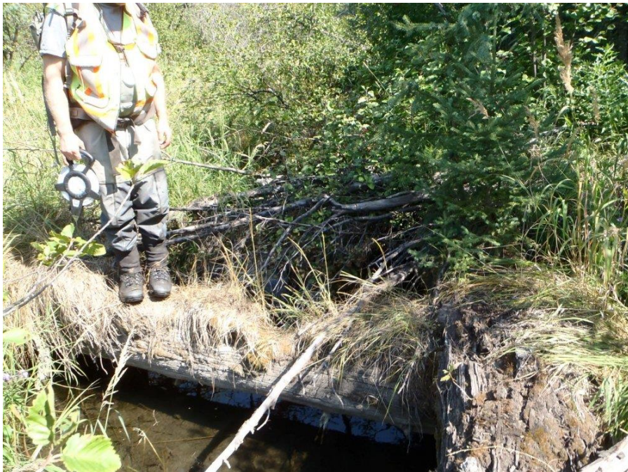
Figure 22. Looking upstream at GRE FHAP Unit 19 on August 26, 2017.
