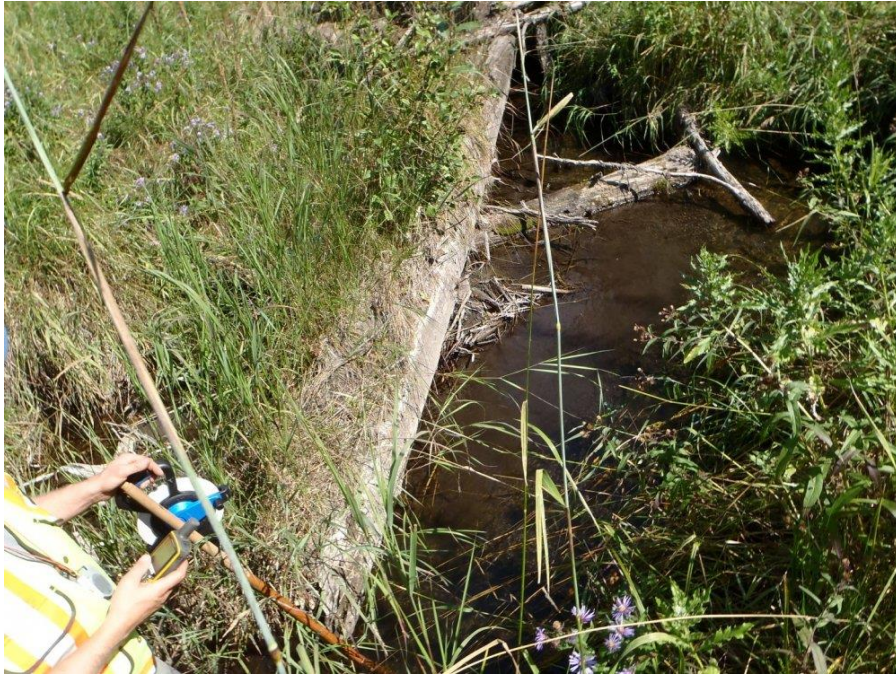
Figure 21. Looking downstream at GRE FHAP Unit 18 on August 26, 2017.
