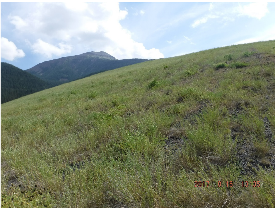
Photo II-19 Upper portion of the downstream slope – looking east. Slope is in good condition with no significant sign of erosion or movement (BTD-2017-15)
