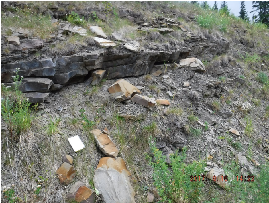
Photo II-26 Typical cut in bedrock on left bank of spillway channel (BTD-2017-21)
