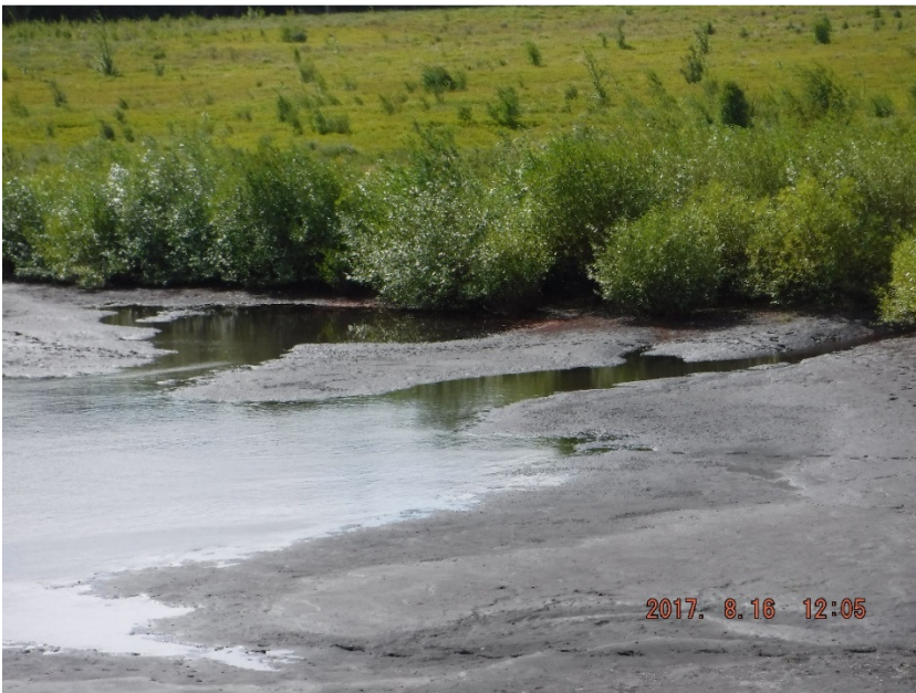
Photo II-6 Localized channels on tailings surface – looking south (BTD-2017-04)
