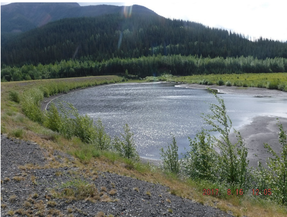
Photo II-5 Overview of vegetated tailings surface and ponded area - looking southeast; pond is smaller than previous year (BTD-2017-04)
