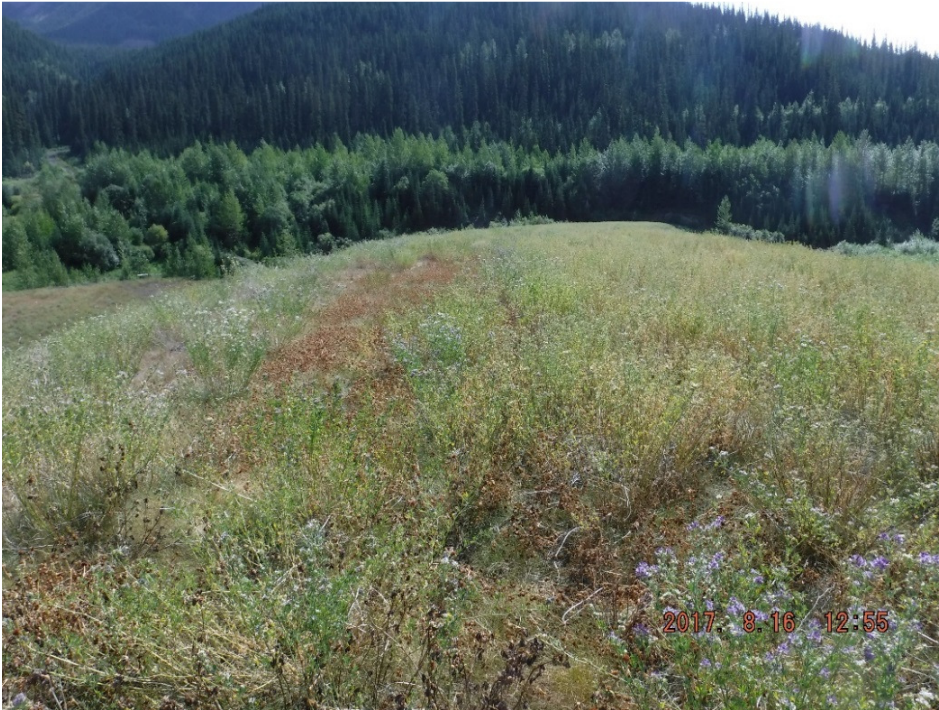
Photo II-10 BTD crest – well vegetated. Minor rutting from vehicle traffic observed (BTD-2017-07)
