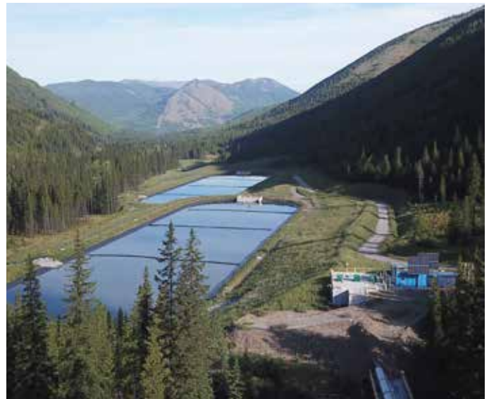
LCO Dry Creek Water Management System Sedimentation Ponds.
