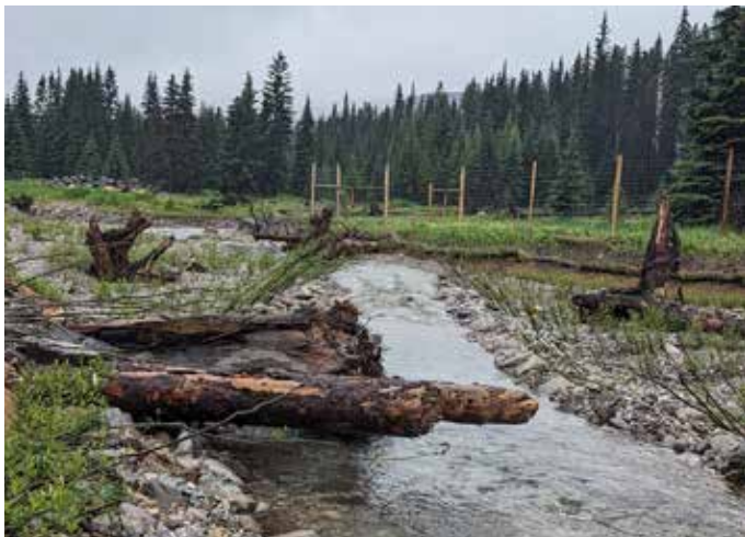
Constructed fish habitat in FRO Clode Creek.
