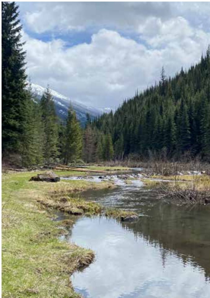
Beaver dam complex upstream of Harmer Dam.
