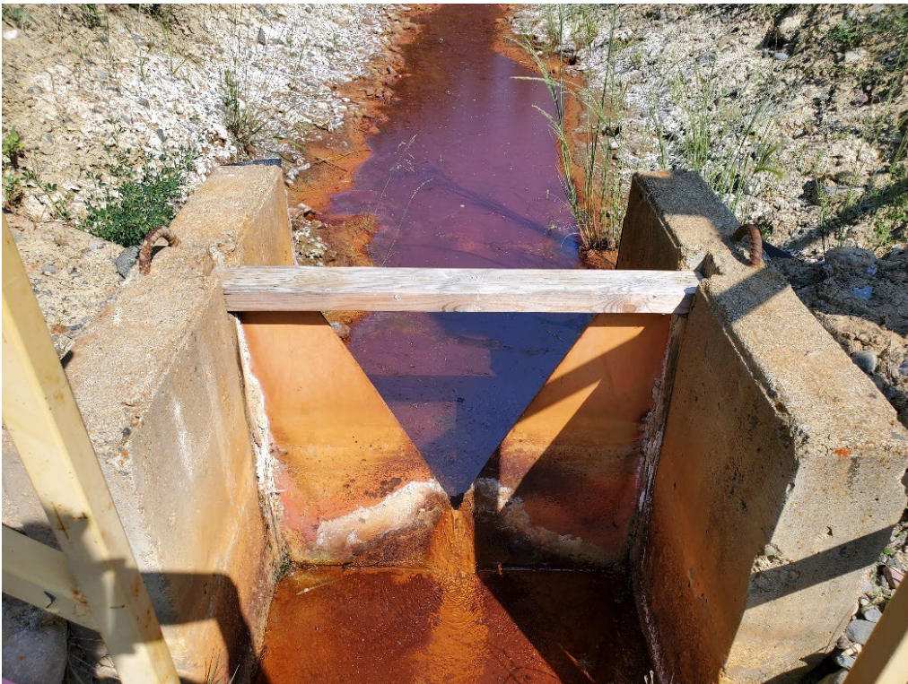
Photo II.16 Weir #4 worn notch
