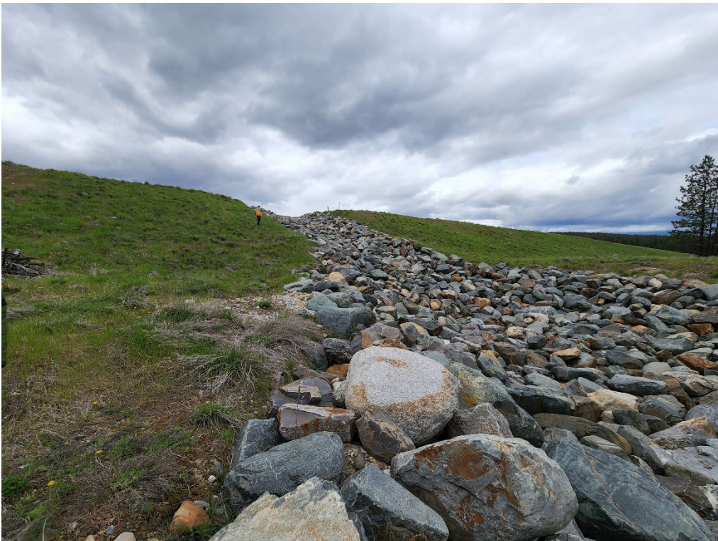
Photo II.26 Siliceous TSF Spillway
