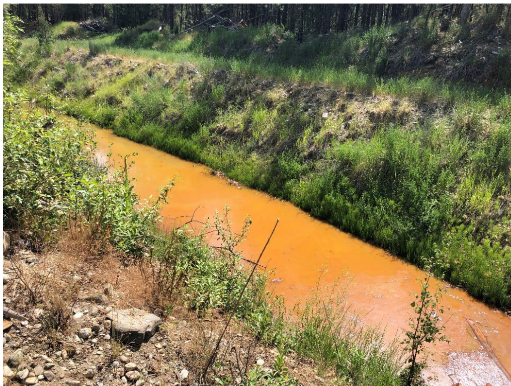
Photo II.24 Seepage downstream of No. 2 Siliceous Dike
