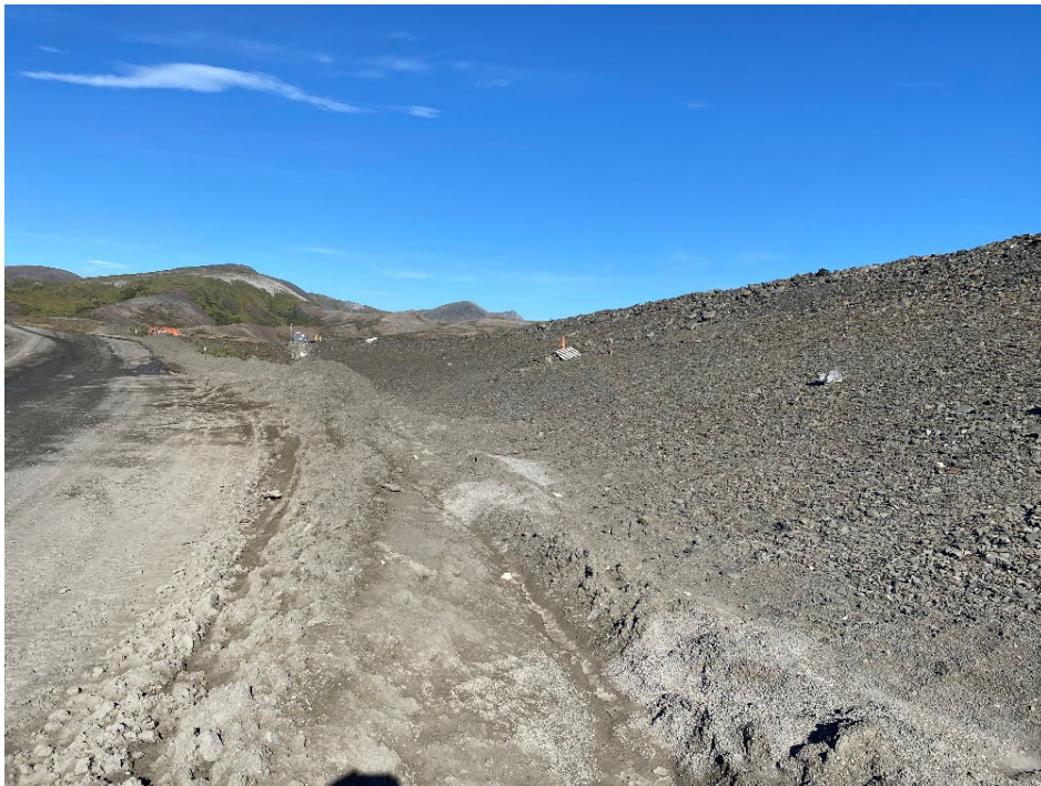
Photo 18: Downstream Slope and Piezometer near Station 39+00
