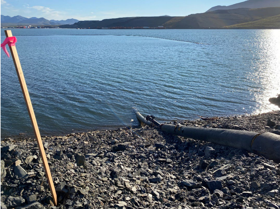
Photo 9: Upstream Slope near Station 10+00 and Subaqueous Tailings Discharge in Pond
