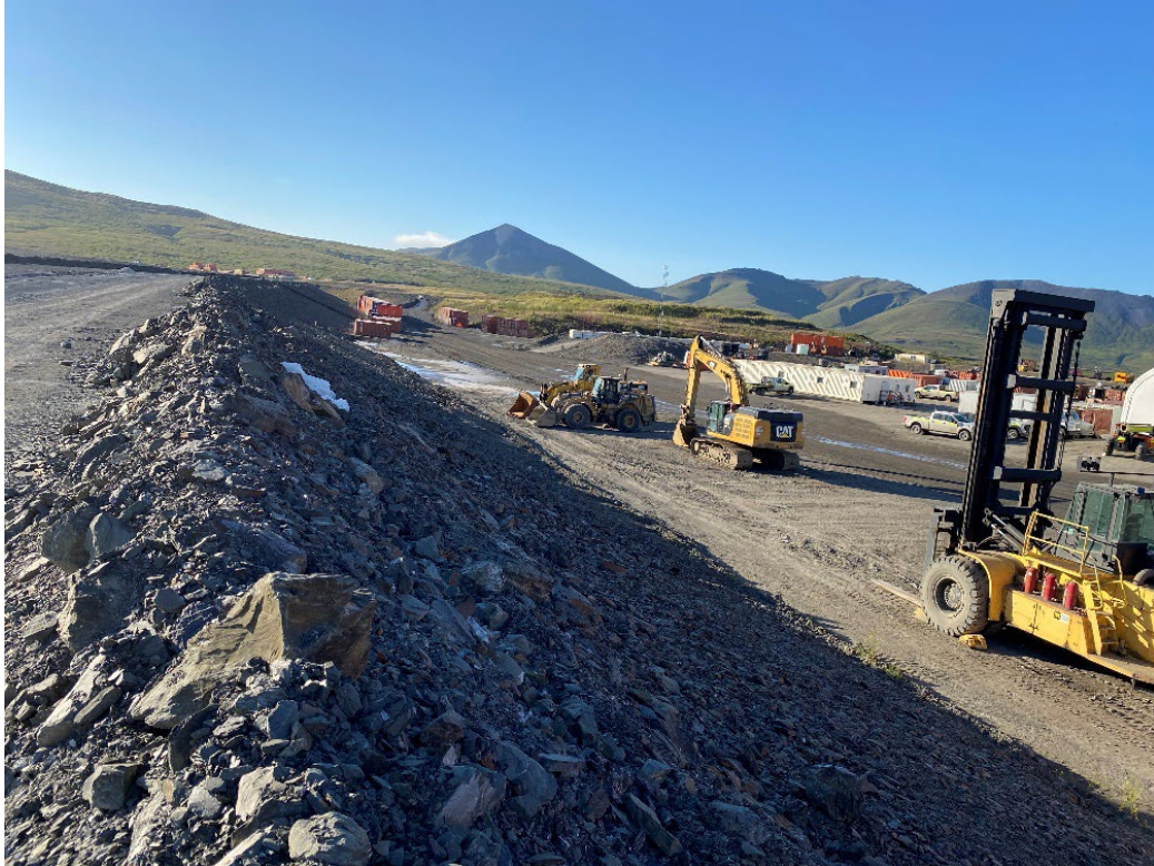
Photo 5: Downstream Slope near Station 2+50
