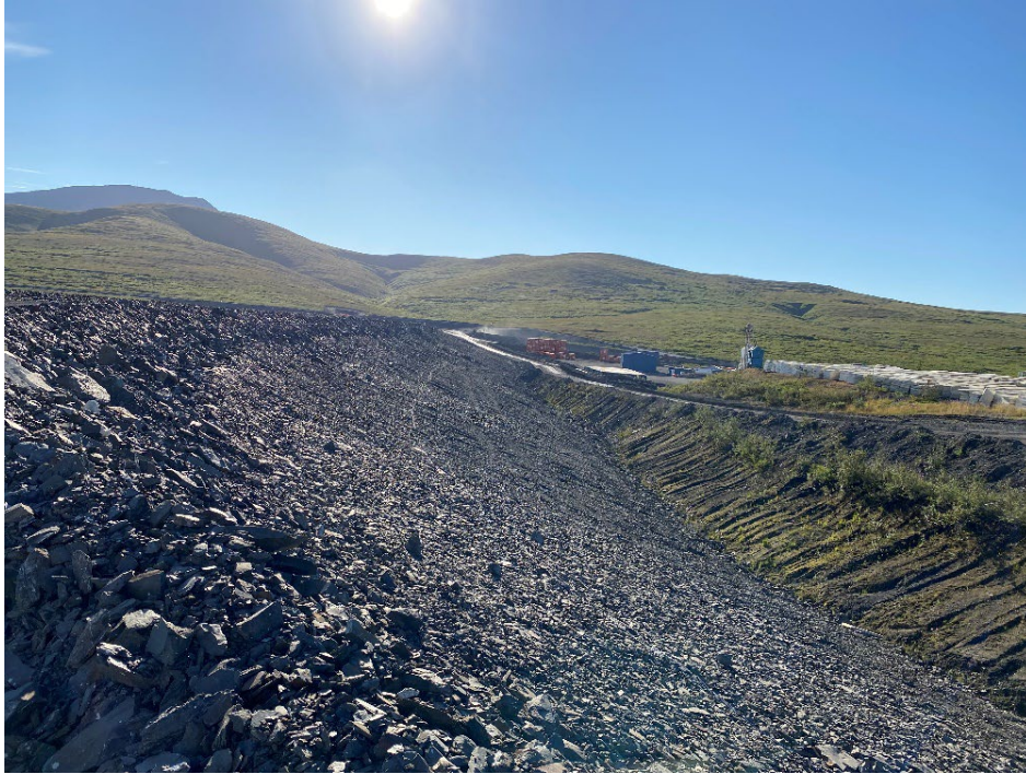
Photo 15: Downstream Slope near Station 27+00
