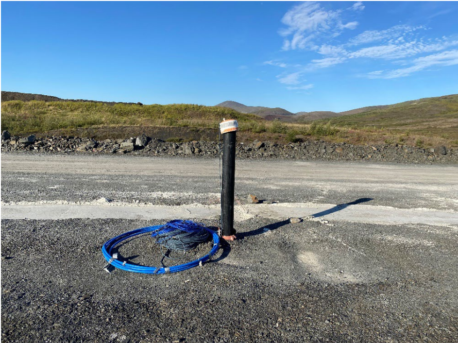
Photo 10: Dam Crest, Cut-off Wall, and SAA Inclinator near Station 14+00
