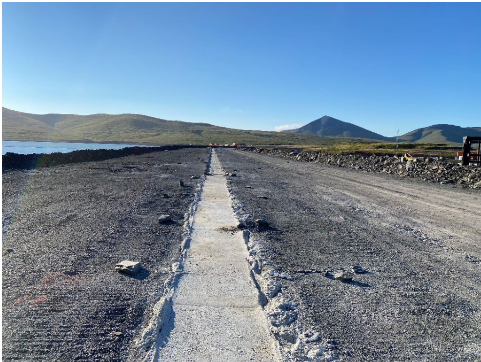
Photo 4: Dam Crest and Cut-off Wall near Station 2+00
