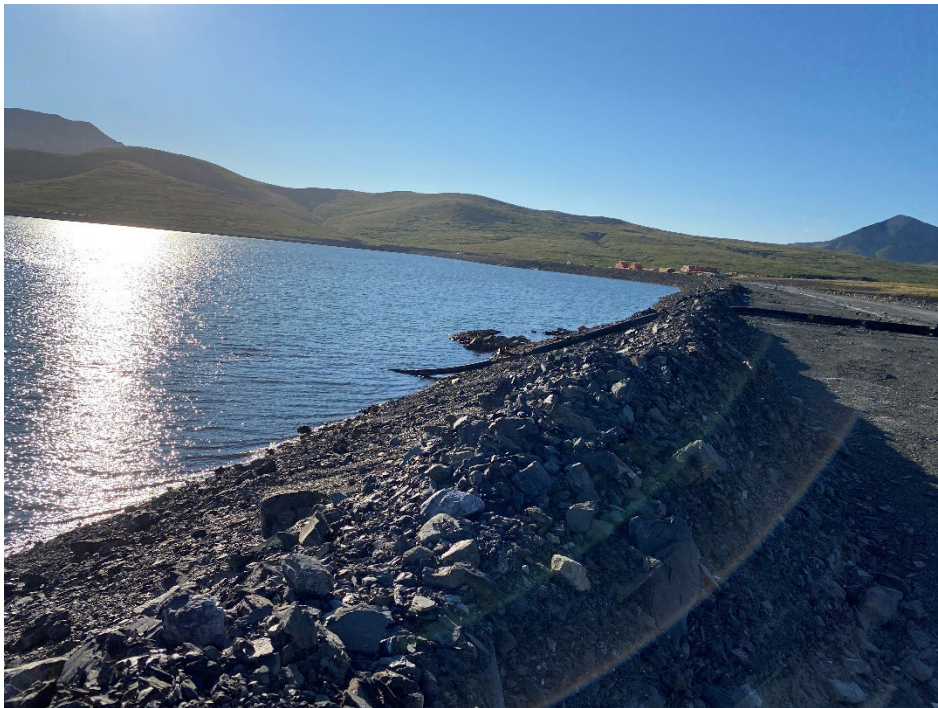
Photo 8: Upstream Slope near Station 9+00
