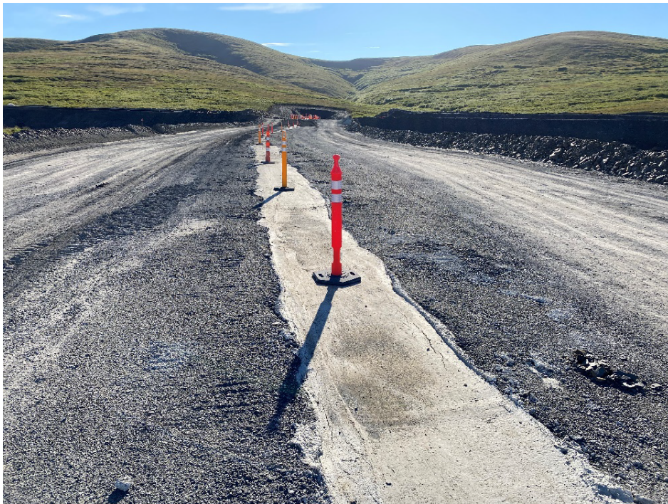
Photo 20: Dam Crest and Cut-off Wall near Station 44+00
