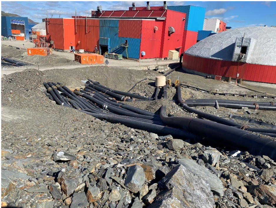
Photo 18: Downstream Slope at Pipeline Corridor
