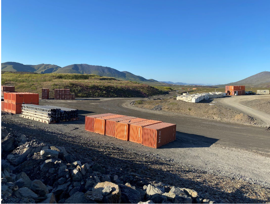
Photo 7: Downstream Slope and Kivalina Overburden Stockpile near Station 9+00
