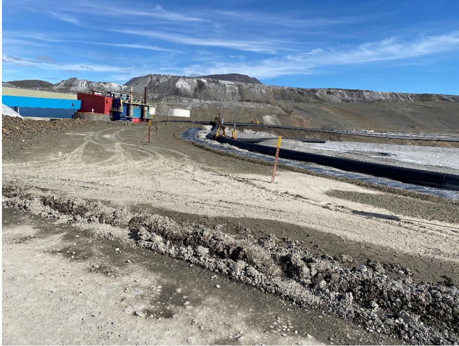
Photo 5: Embankment Crest near Transition to Wing Wall
