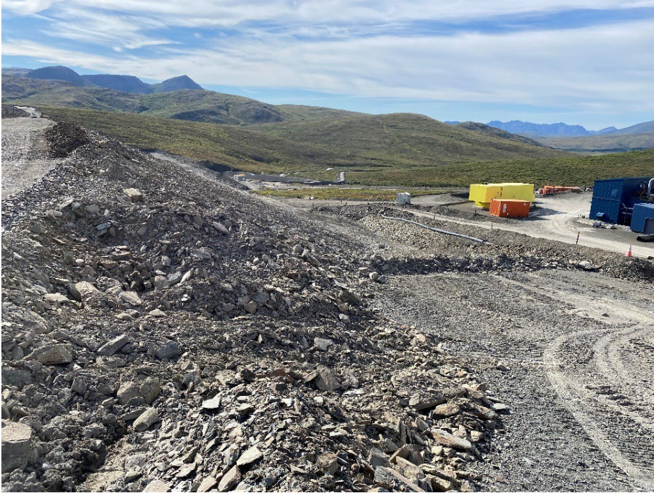
Photo 7: Downstream Slope at East Abutment of Embankment
