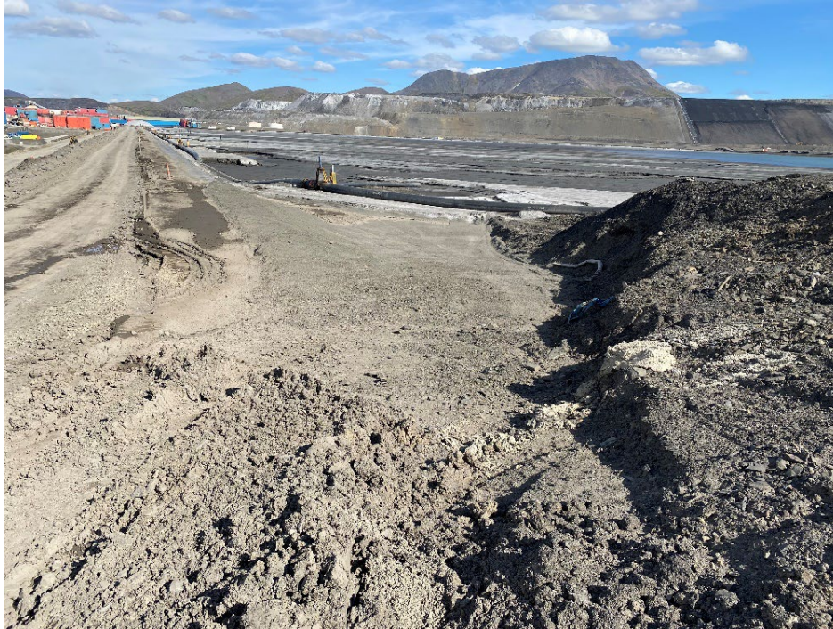
Photo 1: Upstream West Abutment of Embankment
