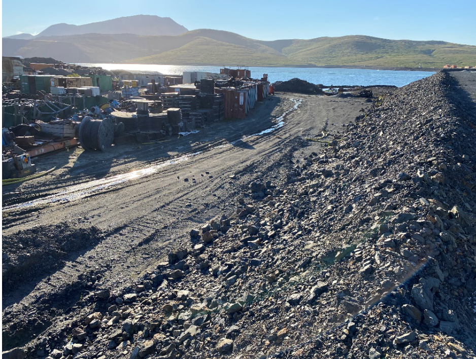
Photo 3: Upstream Slope near West Abutment
