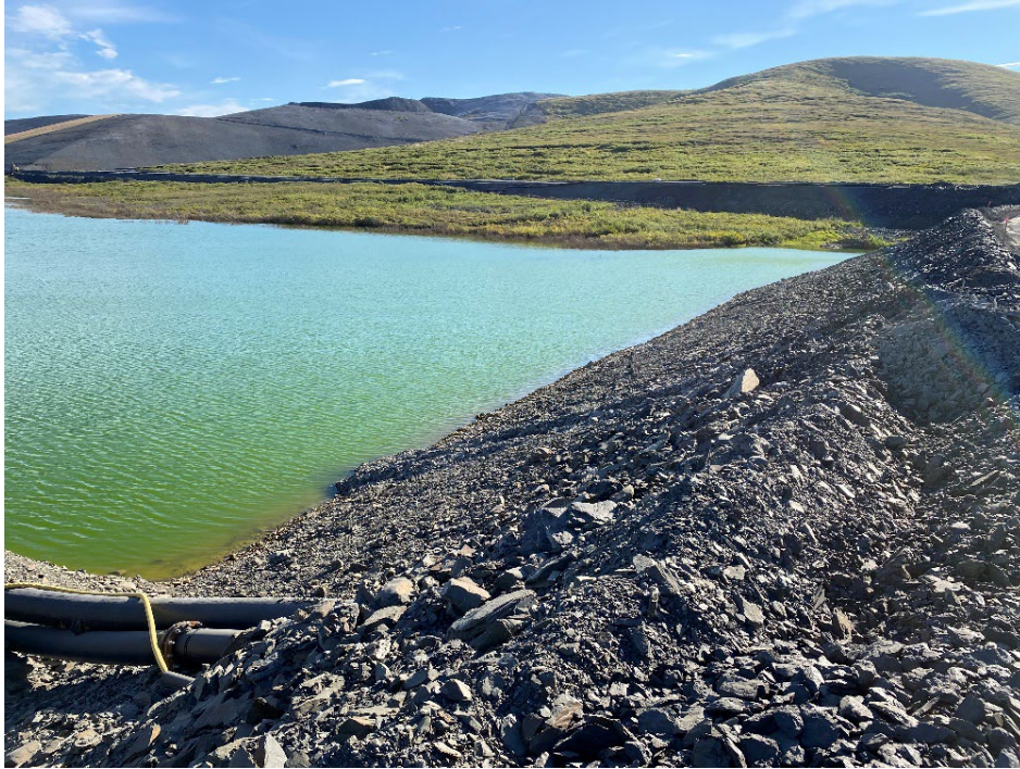
Photo 19: Upstream Slope near Station 43+00
