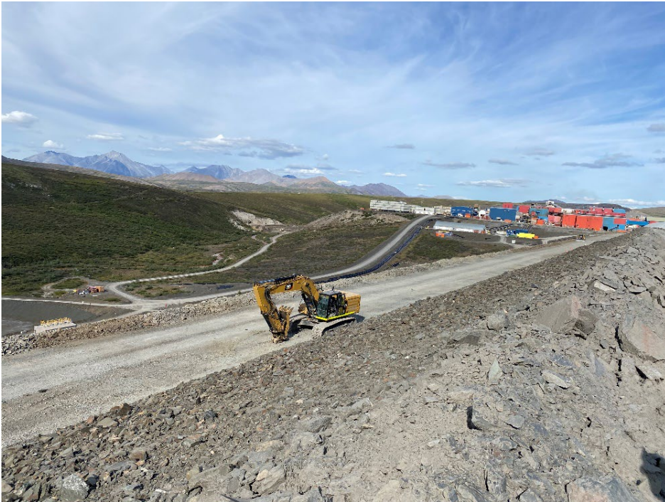
Photo 4: Stage XII Construction Bench and Downstream Embankment Slope
