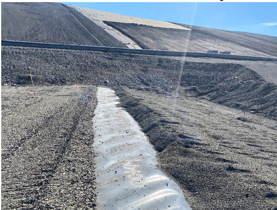
Photo 14: Insulation over Secant Wall at South End of Wing Wall
