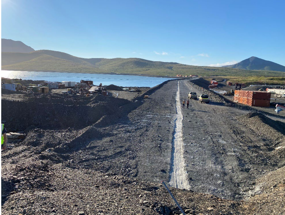
Photo 1: Stage V-A Dam Crest and Cut-off Wall at West Abutment
