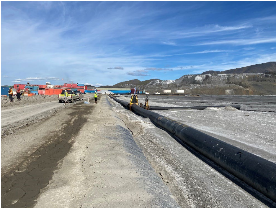
Photo 2: Embankment Crest, Upstream Slope, and Tailings Pipe Bench
