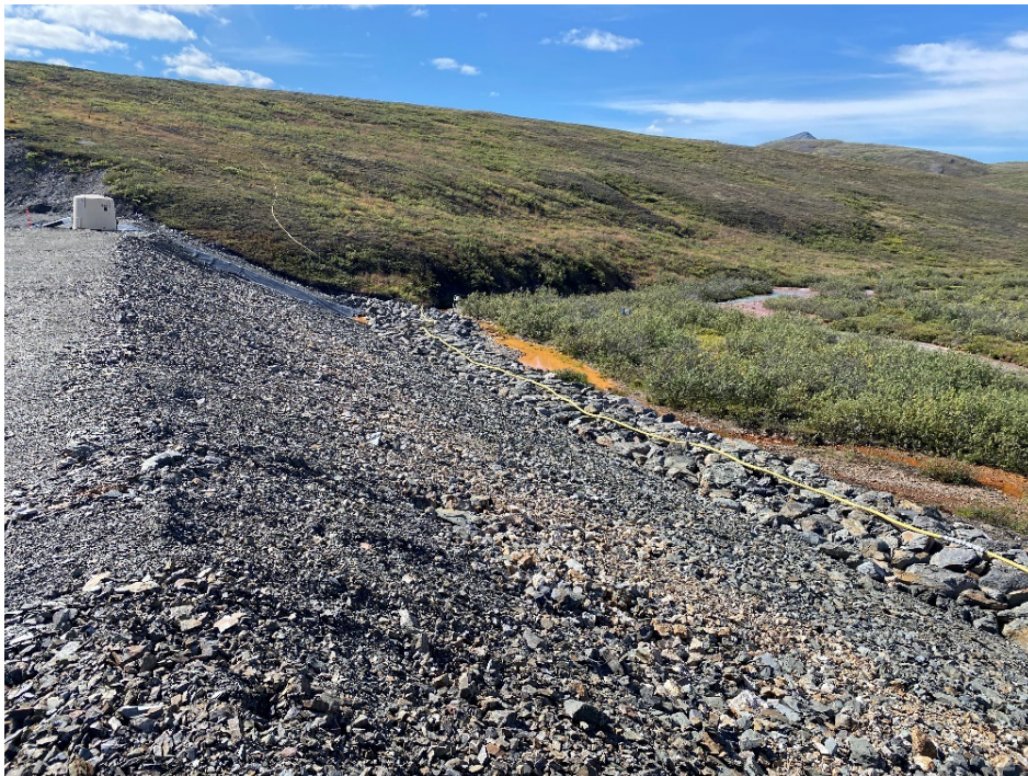
Photo 10: Downstream Slope of Seepage Collection Dam
