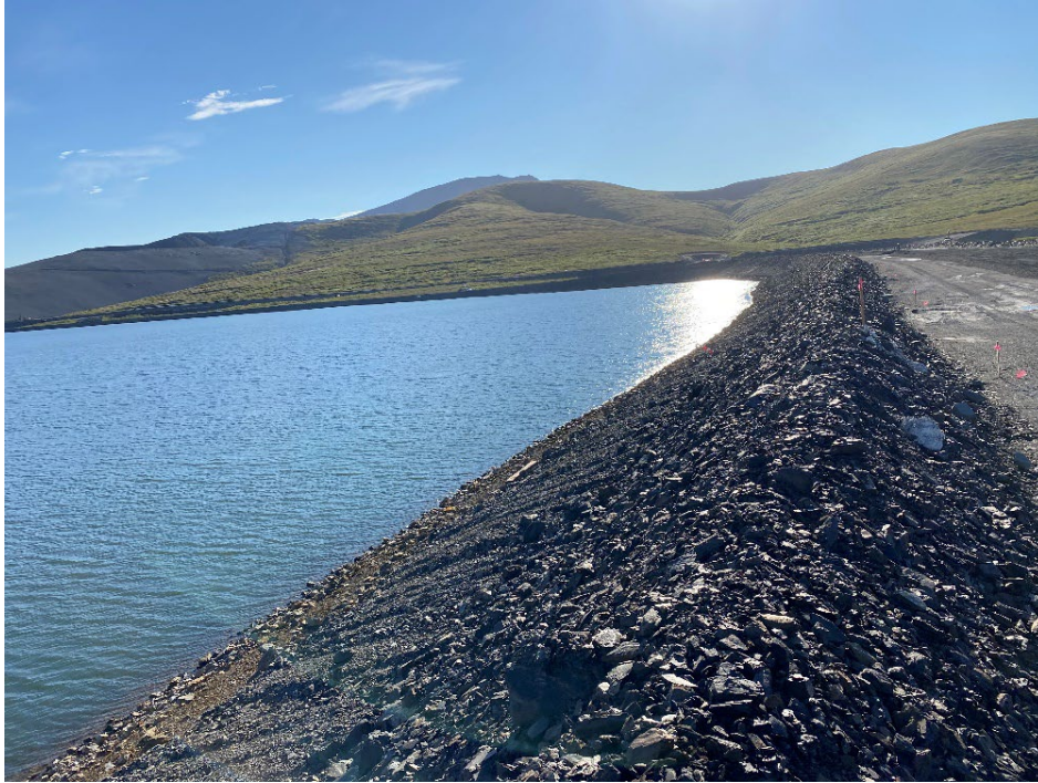
Photo 17: Upstream Slope near Station 30+50
