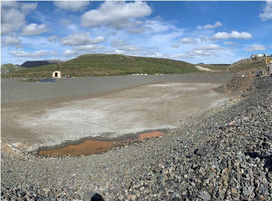
Photo 8: Seepage Collection Pond with Visible Pooled Water
