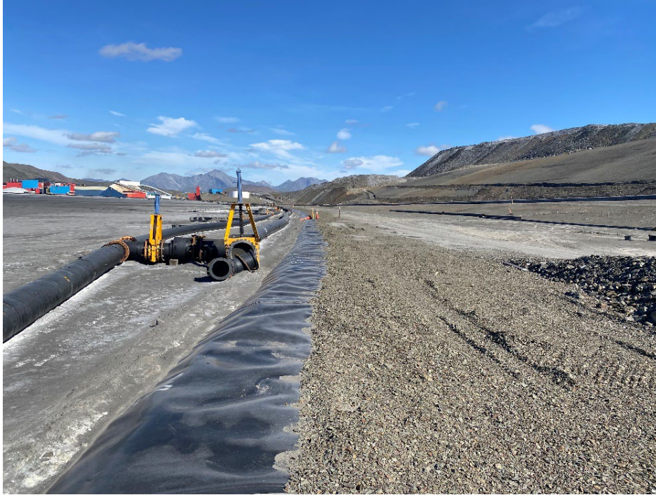
Photo 15: Upstream Slope and Crest at South Leg of Wing Wall
