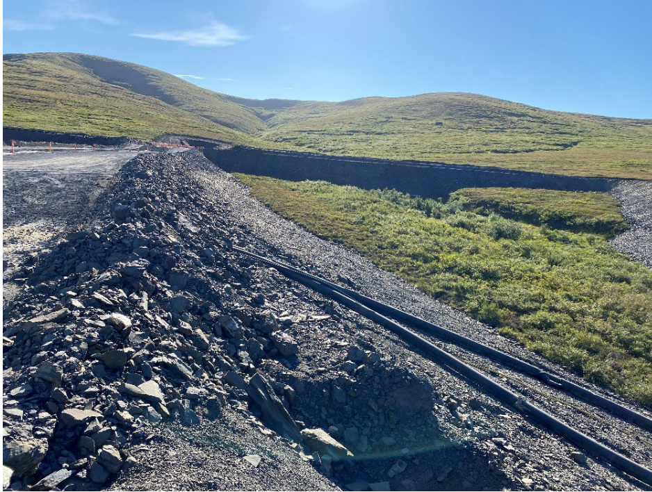
Photo 21: Downstream Slope and Transportation Corridor near Station 43+00
