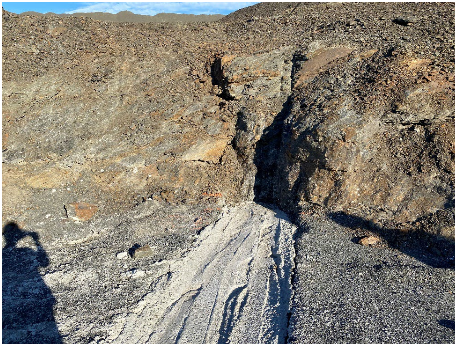
Photo 2: Cut-off Wall Tie-In to Bedrock at West Abutment
