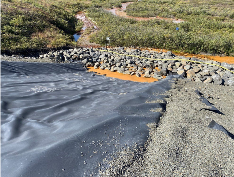
Photo 11: Seepage Collection Dam Spillway
