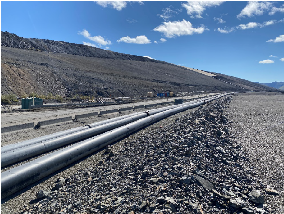
Photo 16: Downstream Slope and Crest at South Leg of TMD Wing Wall
