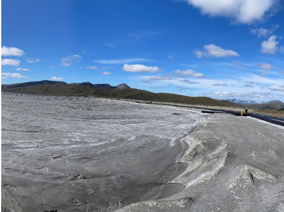
Photo 19: Subaerial Tailings Beach at Embankment
