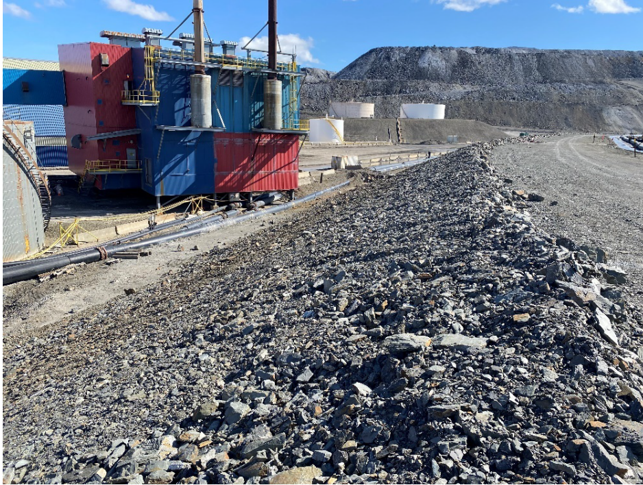
Photo 17: Downstream Slope and Crest at North Leg of TMD Wing Wall
