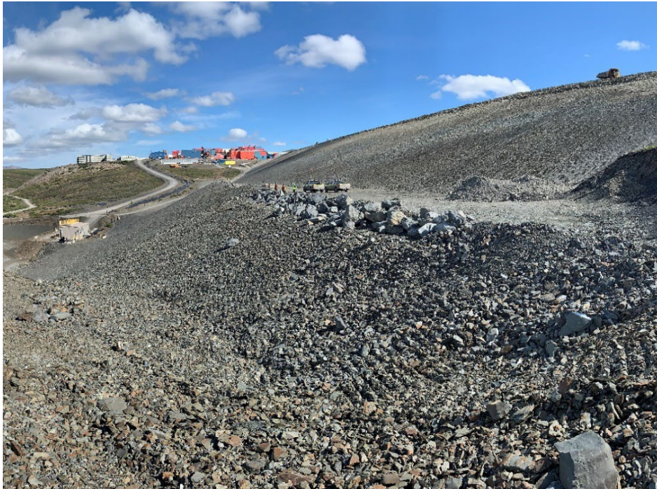
Photo 6: Downstream Slope and Buttress at West Abutment of Embankment
