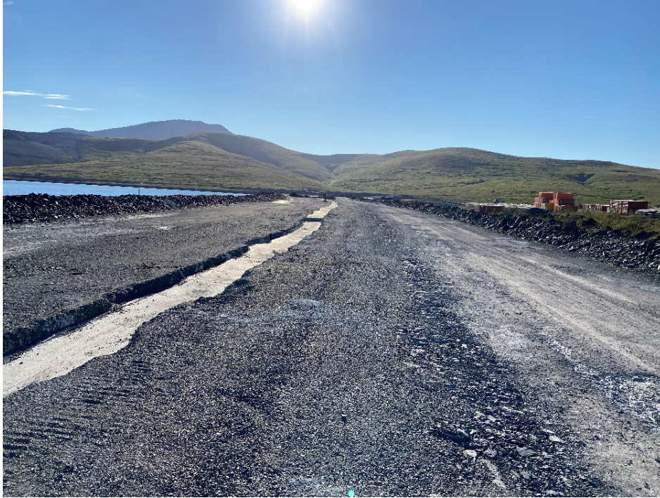
Photo 11: Dam Crest and Cut-off Wall near Station 21+50
