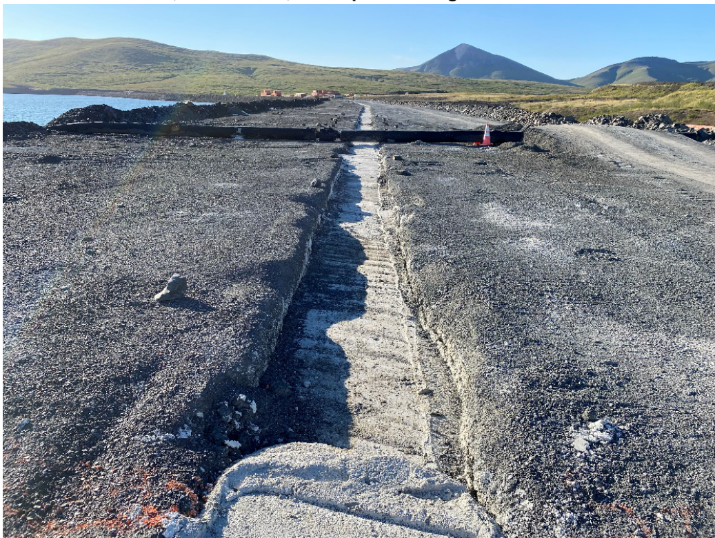
Photo 6: Dam Crest, Cut-off Wall, and Pipe Crossing near Station 10+00
