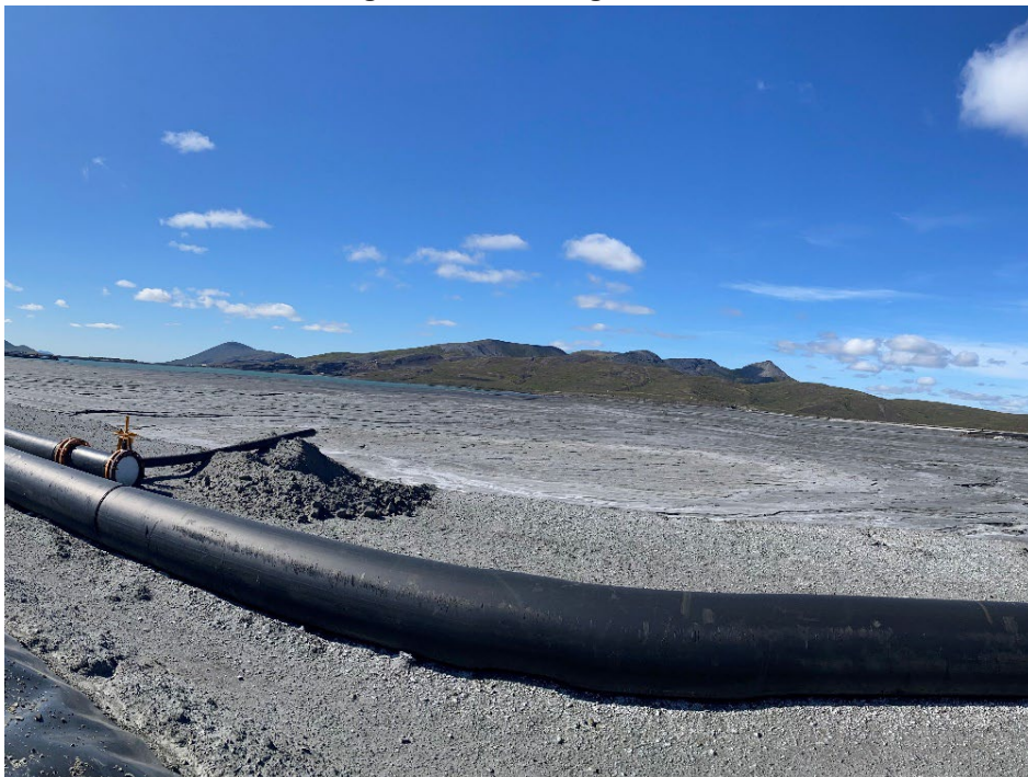
Photo 20: Subaerial Tailings Beach at Wing Wall
