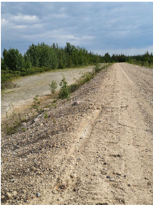
Photo II-2 South Dyke – looking east, minor rills on upstream slope, exposed tailings
