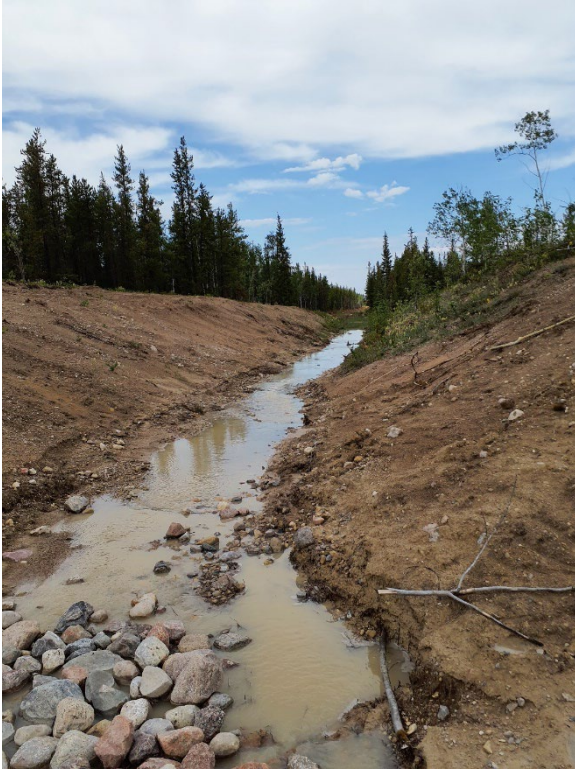
Photo II-39 East Diversion Ditch – looking north at a section of 2021 maintenance
