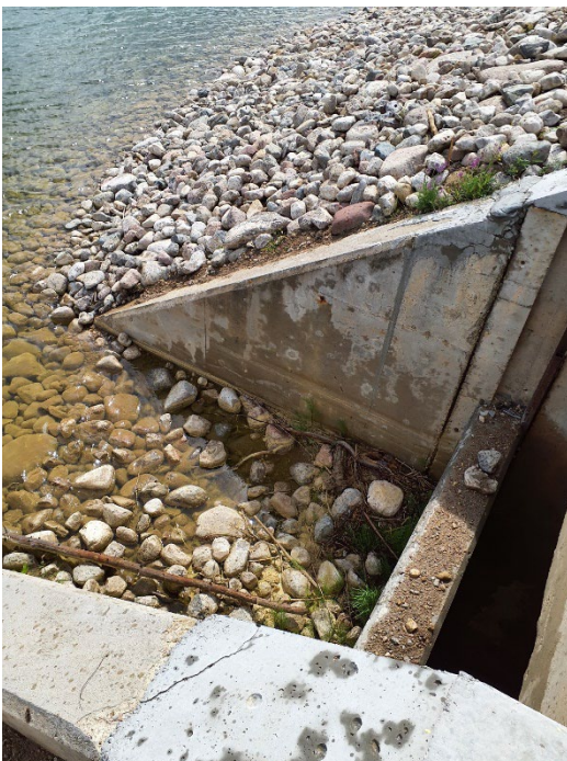
Photo II-24 Main Pond Spillway – looking at the inlet to see the height of the clay plug upstream of the concrete wall
