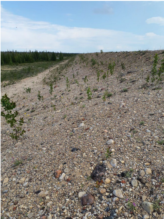
Photo II-16 North Dyke – looking east at the downstream slope
