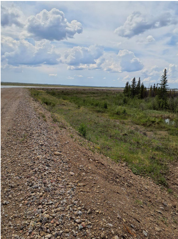
Photo II-21 North Dyke – looking southwest at the downstream slope
