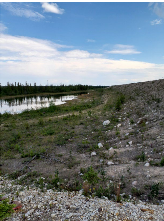
Photo II-14 North Dyke – looking east at the downstream slope and permanent pond at toe
