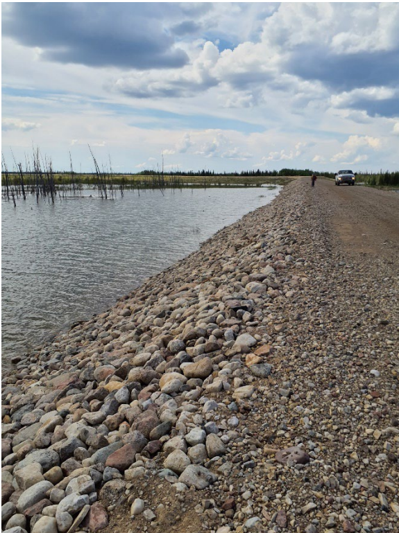
Photo II-18 North Dyke – looking west at the downstream slope where riprap was placed in 2021
