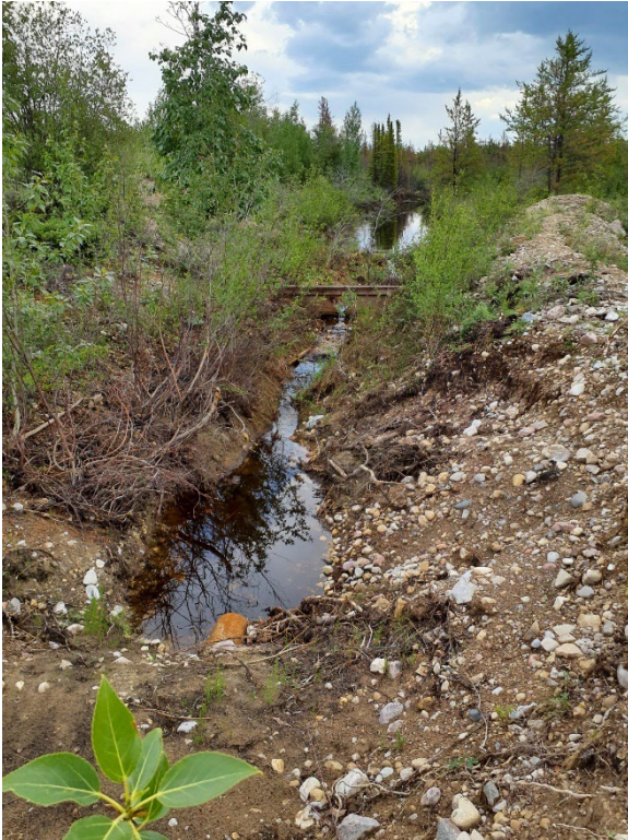
Photo II-36 East Contact Water Ditch – looking south at the weir
