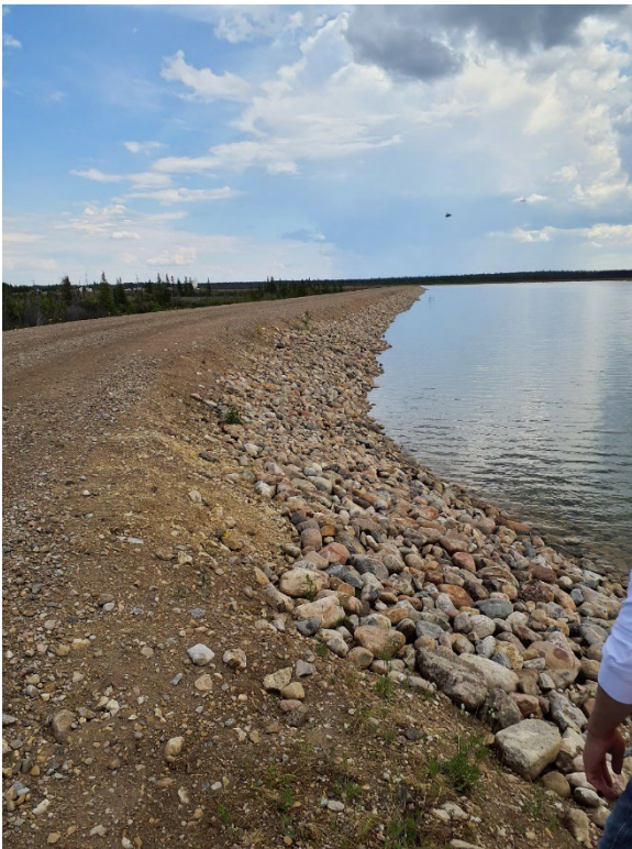
Photo II-20 North Dyke – looking east at the upstream slope and 2021 riprap installation
