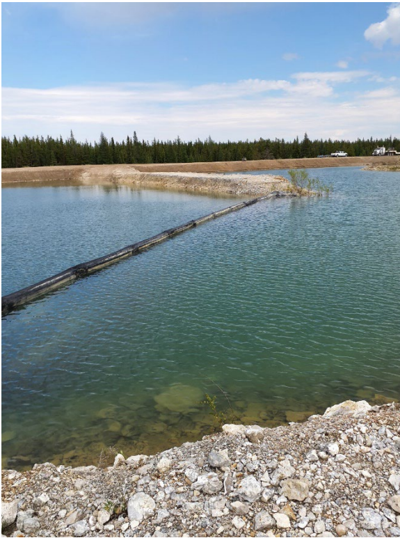
Photo II-29 Polishing Pond – looking east at the southern finger dyke and silt fences
