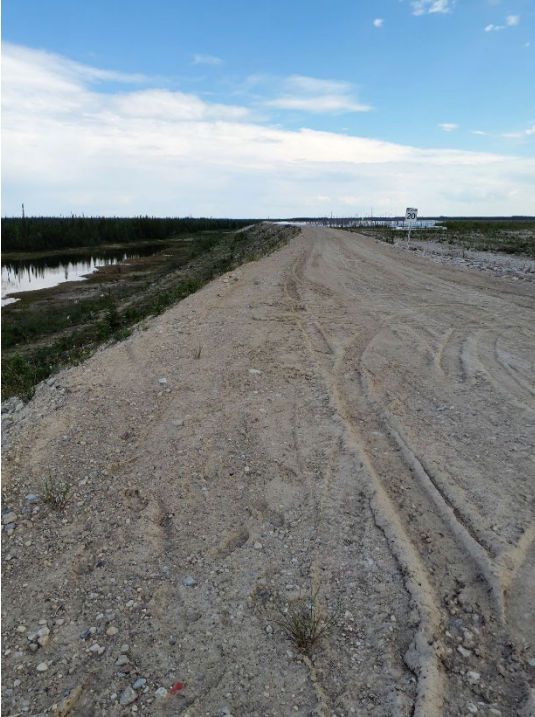
Photo II-14 North Dyke – looking east at the downstream slope and permanent pond at toe
