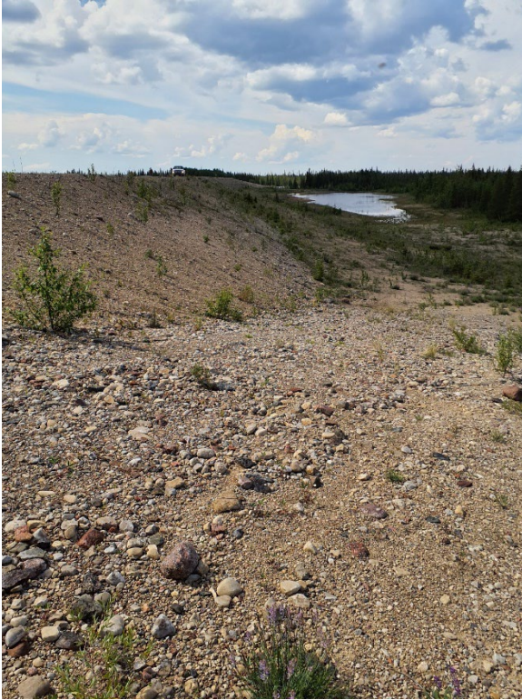
Photo II-18 North Dyke – looking west at the downstream slope where riprap was placed in 2021
