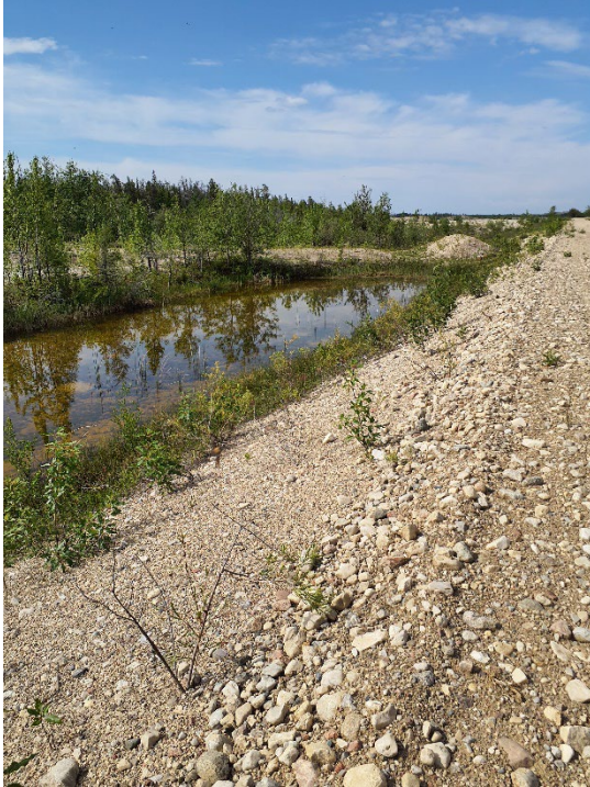
Photo II-2 South Dyke – looking east, minor rills on upstream slope, exposed tailings
