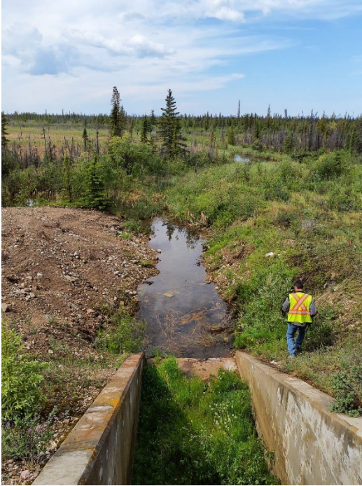
Photo II-24 Main Pond Spillway – looking at the inlet to see the height of the clay plug upstream of the concrete wall
