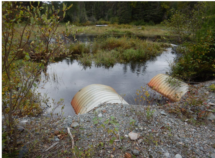
Photo 10 : Culverts on the unnamed creek, northwest of the tailings pond. Water levels were higher than flow in 2021, a possible reflection of significant rainfall on 19 September. No evidence of recent beaver activity in the culverts.
