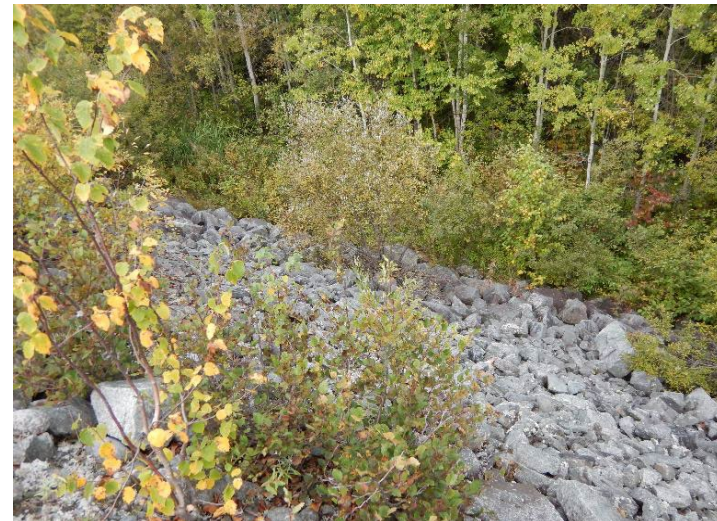
Photo 8 : Typical view of vegetation which is present at the downstream toe of Dams 1 and 2.
