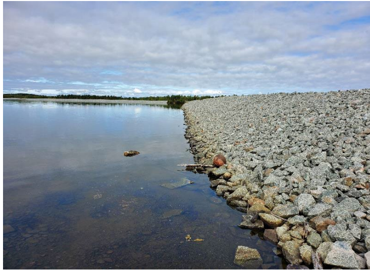
Photo 1 : Dams 1D – View of the upstream slope with riprap replaced.
