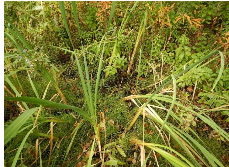
Photo 3 : Flowing water near downstream toe of Dam 1C. Similar flows occur on Dams 1A and 1B.
