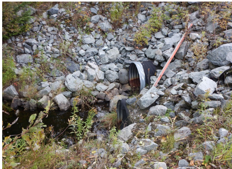
Photo 14 : Outlet channel of the site. Note the limited vegetation upstream of the channel.
