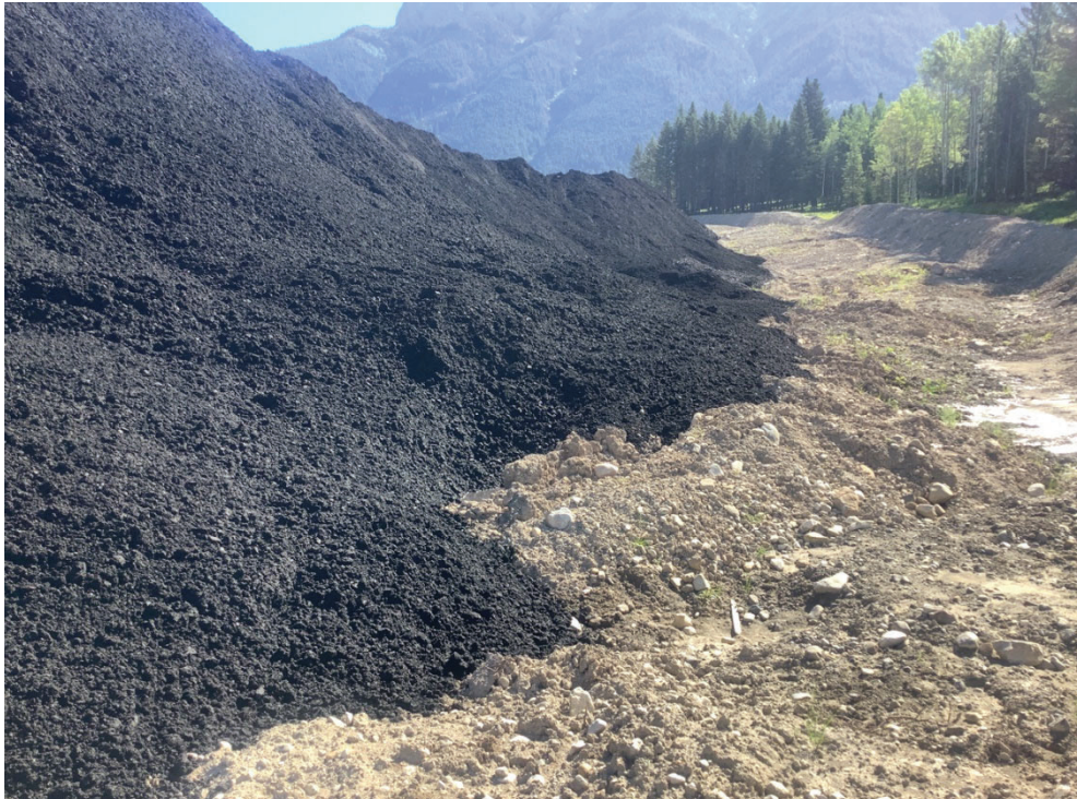
Photo 20. Downstream toe and south runout berm, looking east
