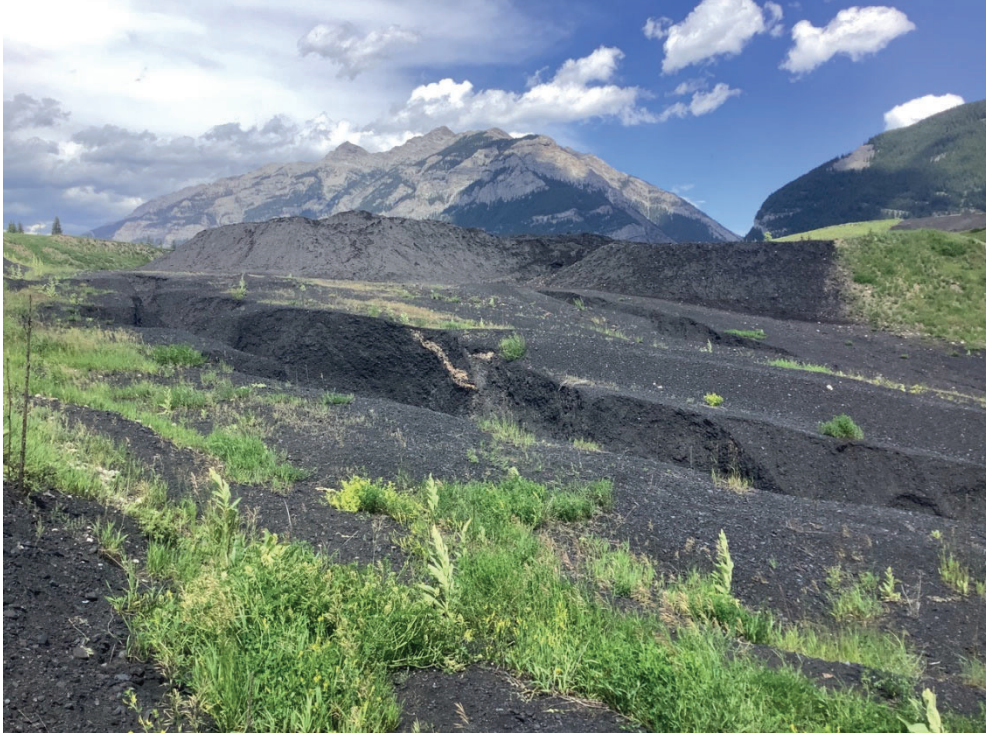
Photo 46. Downstream slope of the Lower Bench, looking northeast
