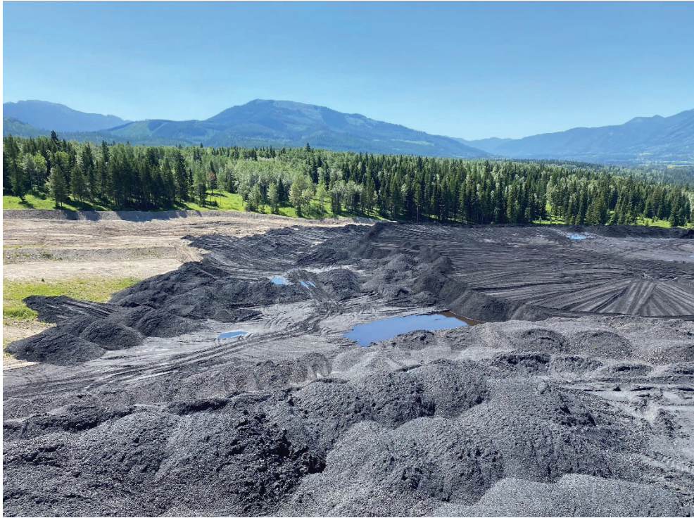
Photo 25. CCR placement on the 1270 m bench, looking south
