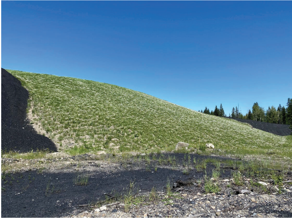
Photo 39. Boundary between progressively reclaimed section of the ERX and recently placed CCR, looking northwest
