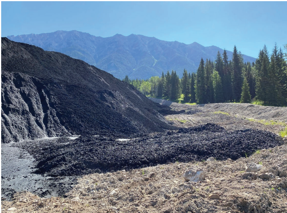
Photo 16. Soft CCR spoils at June 14, 2022 washout event, looking east
