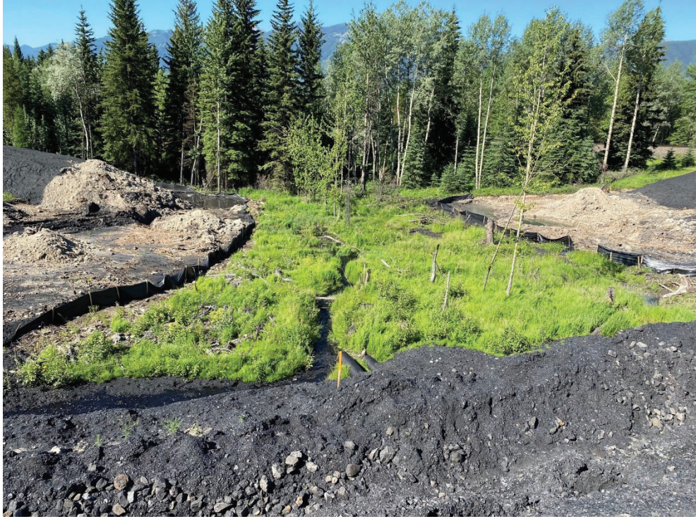
Photo 11. Drainage section in southern downstream area, looking southwest
