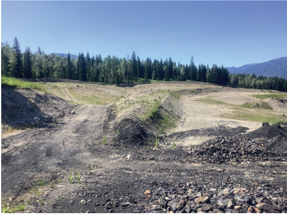
Photo 33. South runout berms constructed from native material, looking south
