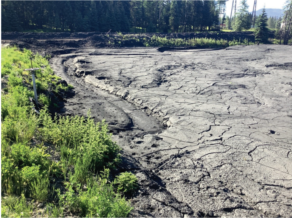
Photo 81. Pond A gated culvert inlet, looking southeast
