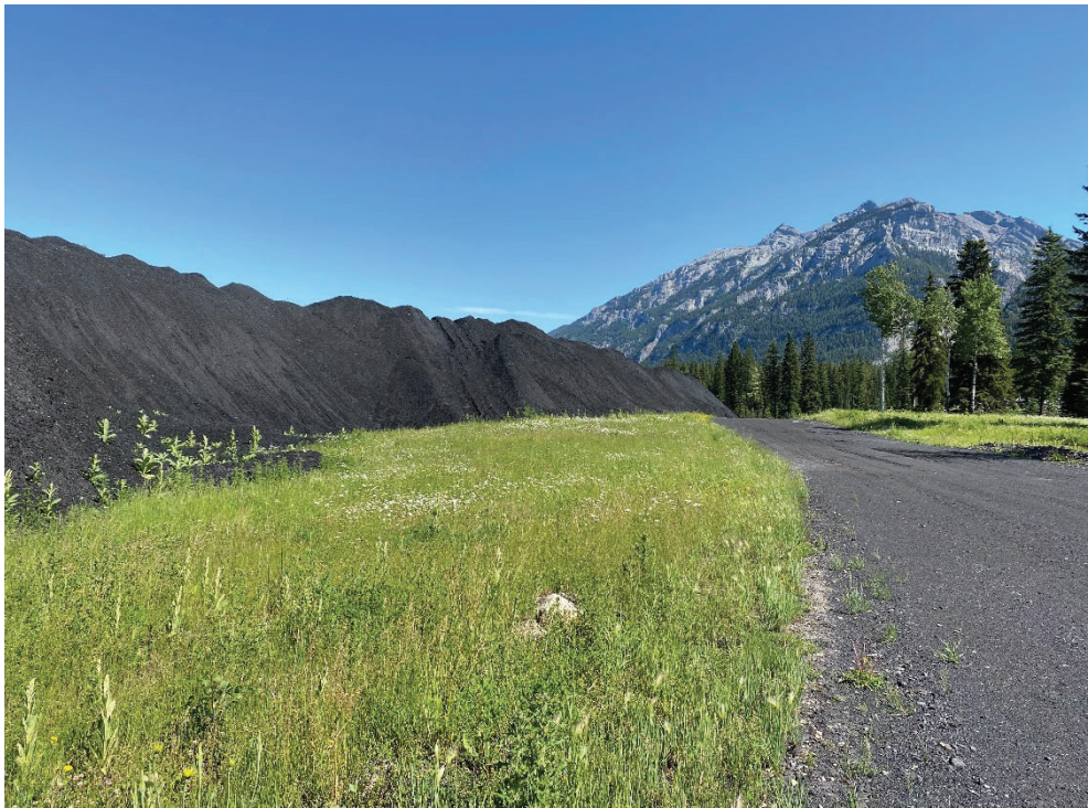
Photo 36. Downstream toe along eastern extents of the ERX, looking north
