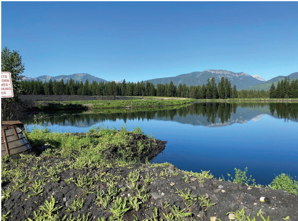
Photo 80. Pond A gated culvert outlet to Pond C, looking southwest
