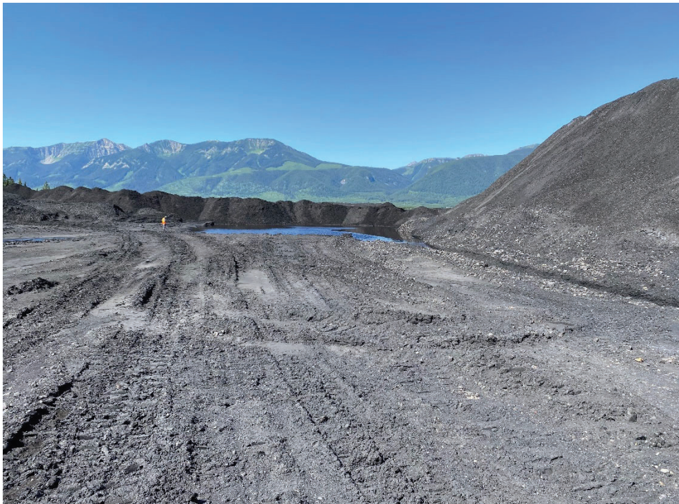
Photo 24. Infiltration sump along toe of the 1285 m bench, looking southwest
