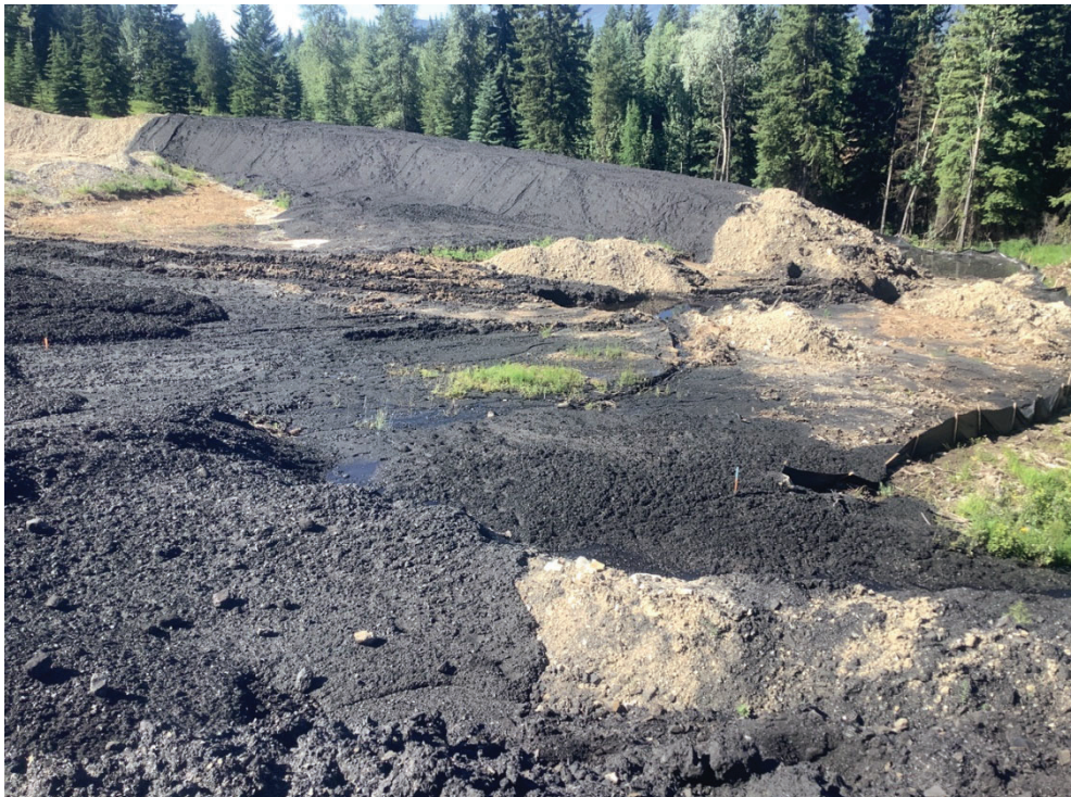
Photo 12. Soft CCR spoils from June 17, 2022 washout event, looking south
