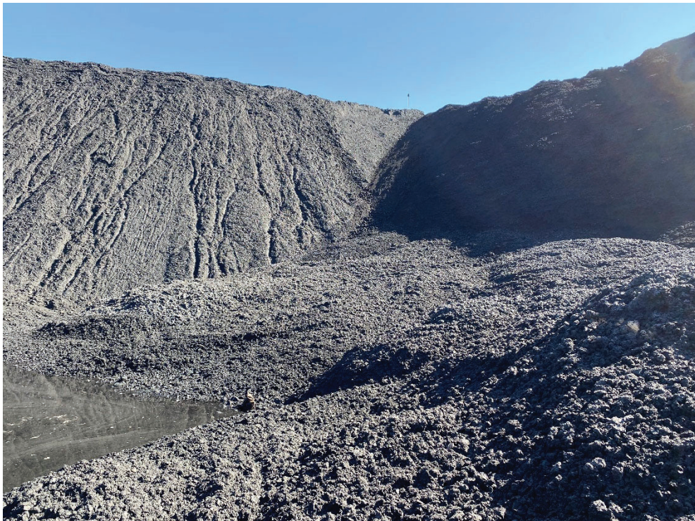
Photo 2. June 17, 2022 washout event location, looking northeast
