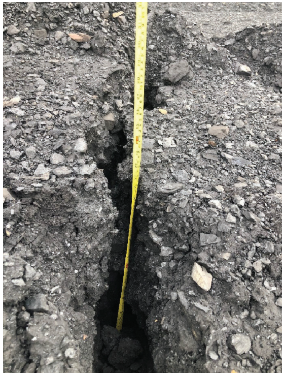
Photo 28. Crack along the 1300 m bench crest, looking east
