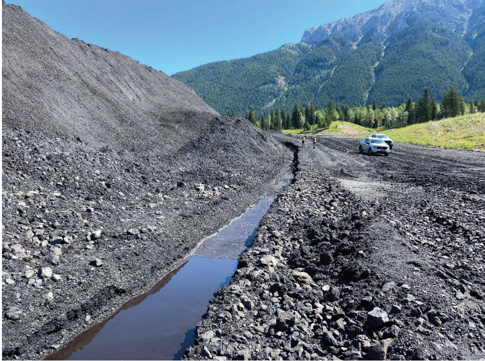
Photo 23. Ditching along toe of the 1285 m bench, looking northeast
