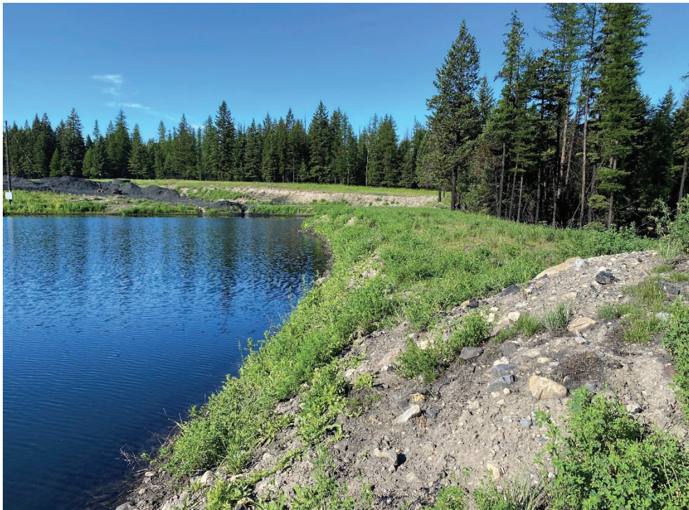
Photo 76. Pond C embankment upstream slope, looking southwest
