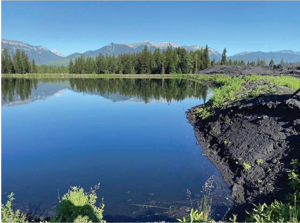
Photo 79. Pond C upstream slope, looking northwest
