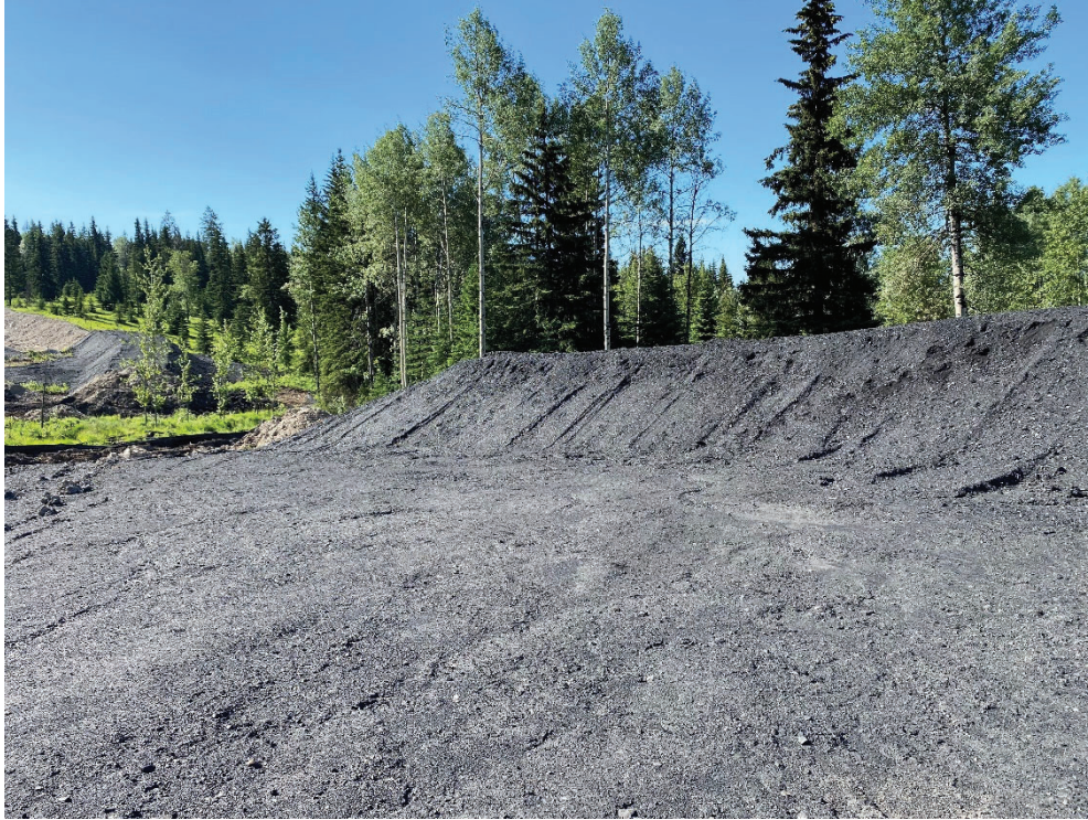
Photo 7. West runout berm constructed out of CCR, looking south
