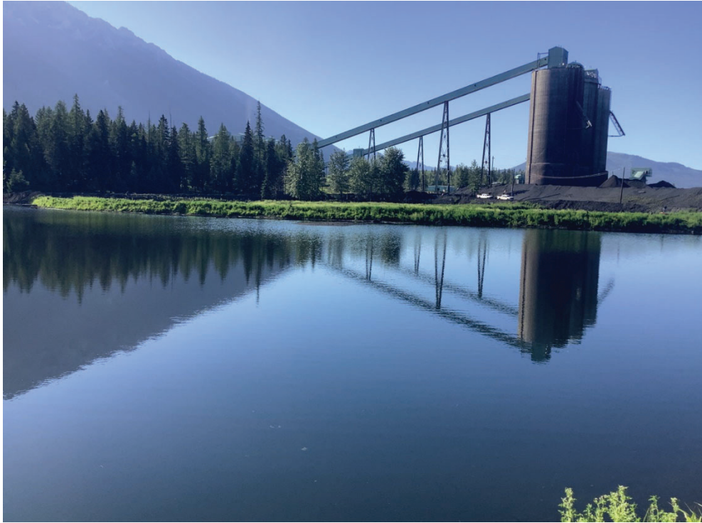
Photo 77. Pond C basin, looking southeast
