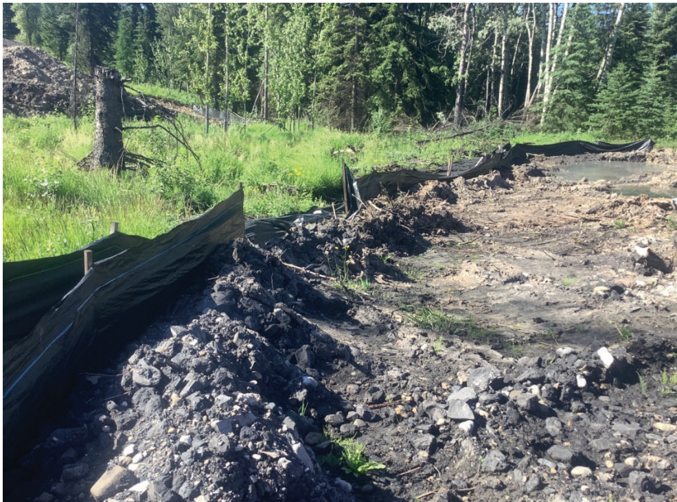
Photo 8. Silt fencing along downstream toe area, looking south
