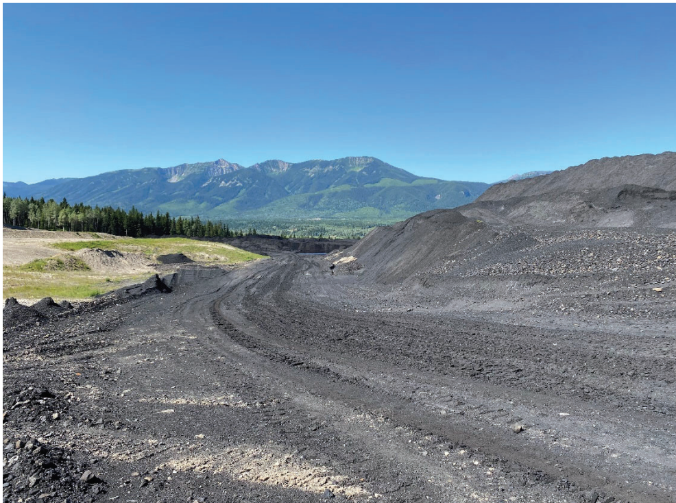
Photo 34. Downstream toe of the 1285 m bench, looking southwest
