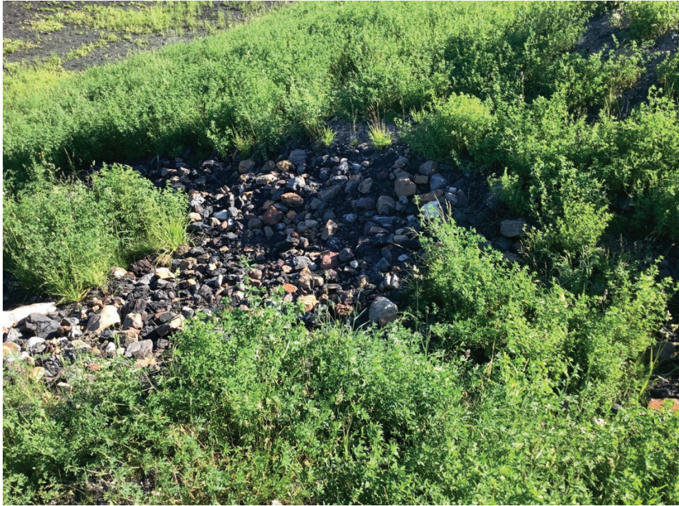
Photo 75. Pond C spillway crest, looking north
