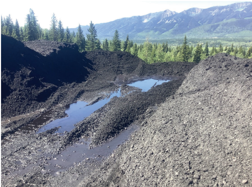
Photo 18. Water pooling near crest of the 1270 m bench, looking south
