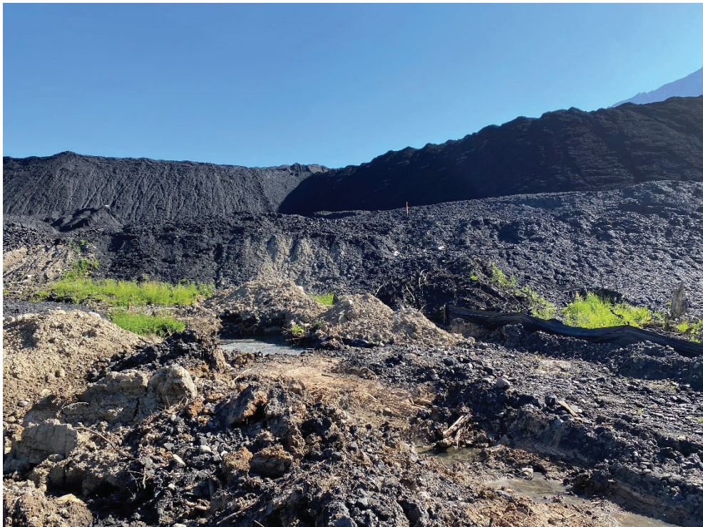
Photo 10. 1270 m bench downstream slope, looking northeast
