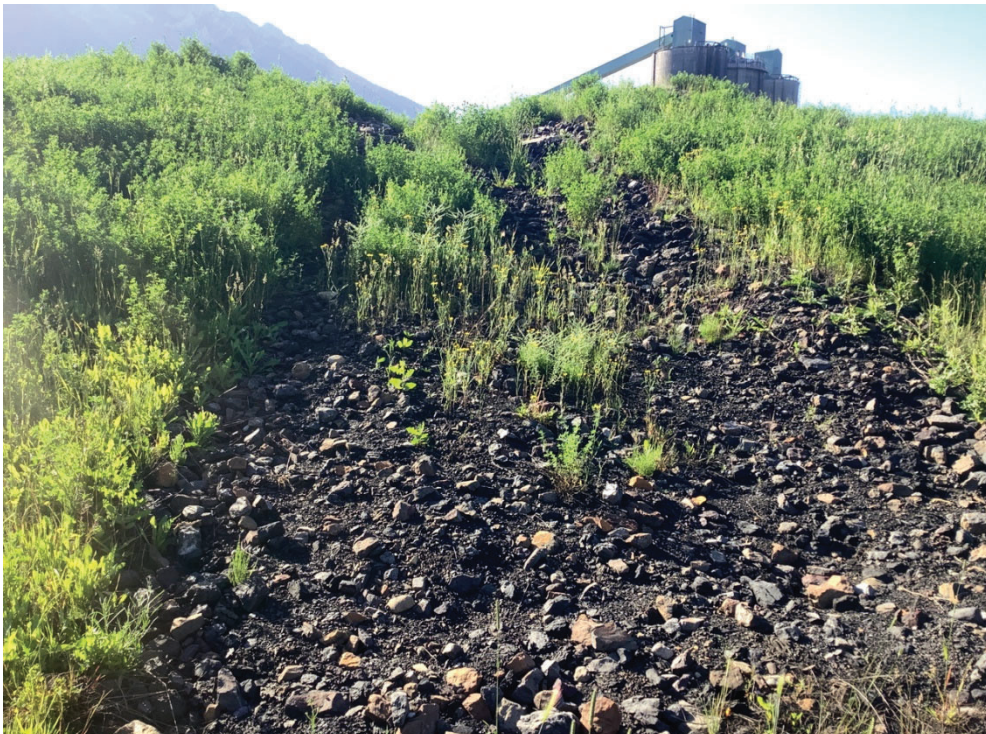
Photo 74. Pond C spillway downstream slope, looking southwest
