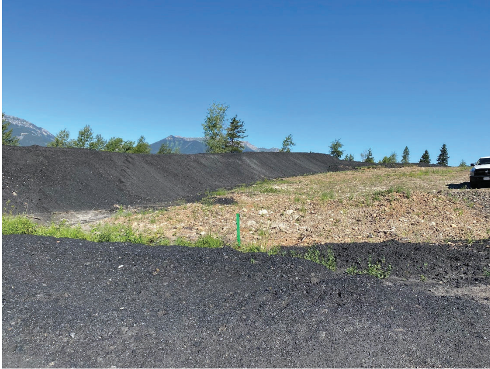
Photo 1. West runout berm constructed out of CCR, looking northwest
