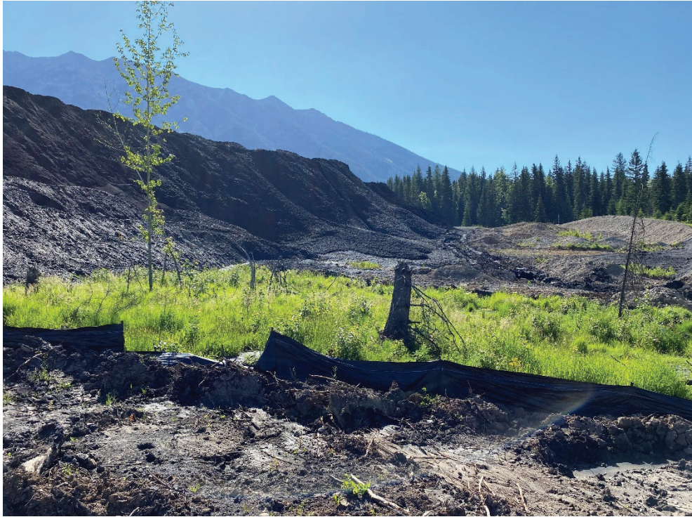
Photo 9. Silt fencing along downstream toe area, looking east
