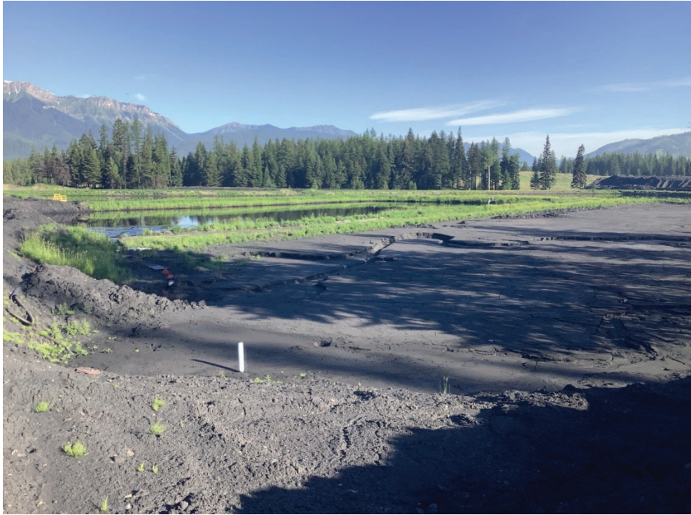
Photo 61. Pond A awaiting cleanout of sediment, looking northwest
