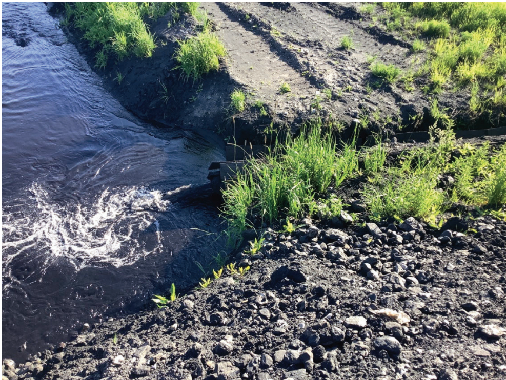
Photo 66. Pond B discharge spigot location, looking northwest
