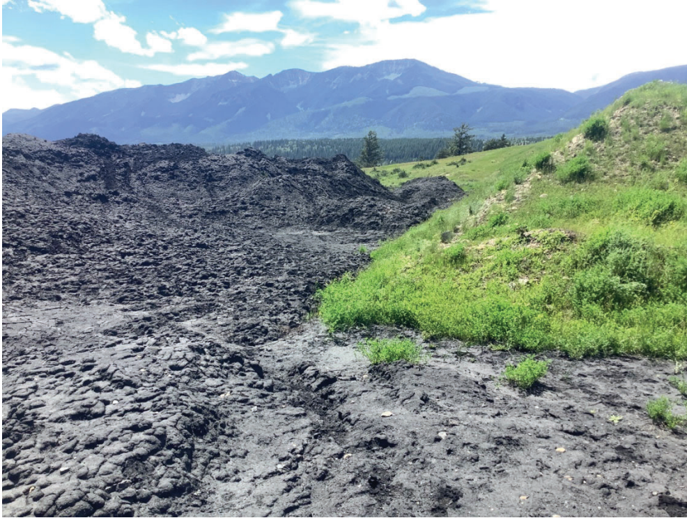
Photo 52. Pond fines deposited along the Lower Exfiltration Basin downstream slope of the Upper Bench, looking southwest
