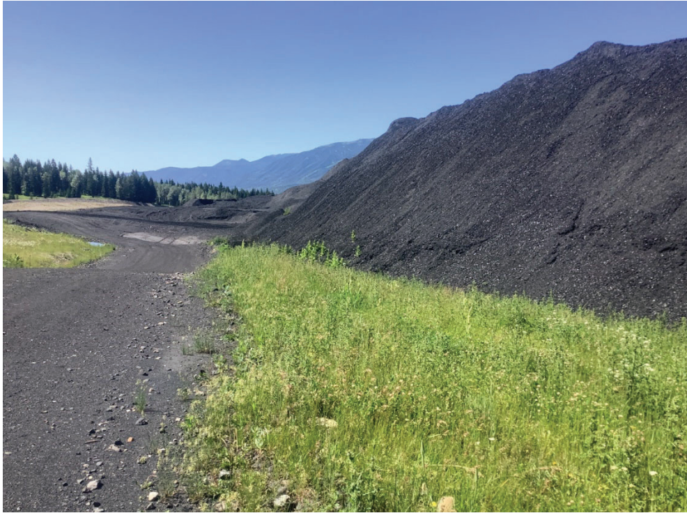
Photo 35. Downstream toe along eastern extents of the ERX, looking south
