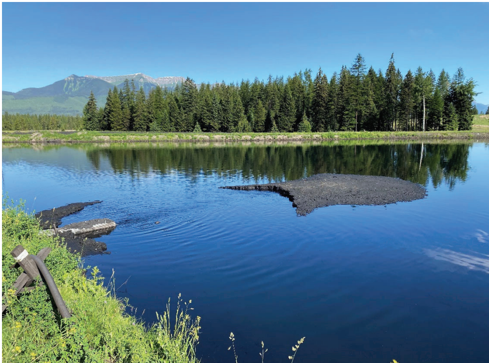
Photo 82. Sediment build up near the Pond B gated culvert outlet to Pond C, looking northwest
