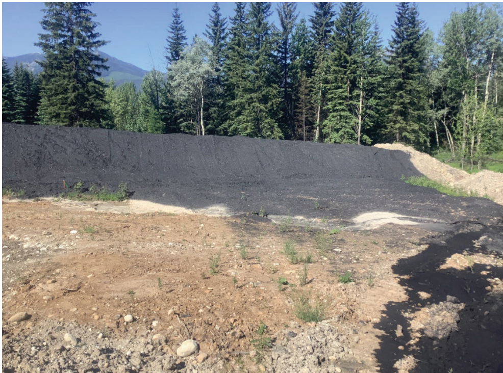
Photo 14. South runout berm section constructed of CCR, looking southwest
