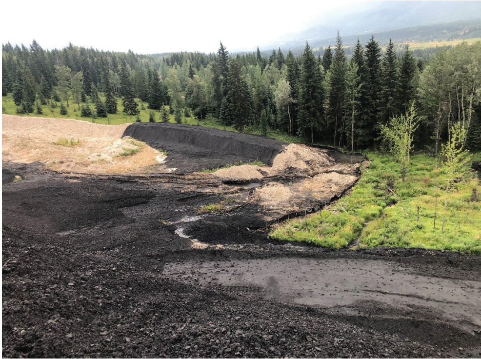
Photo 5. South runout berm repaired with CCR, looking southwest
