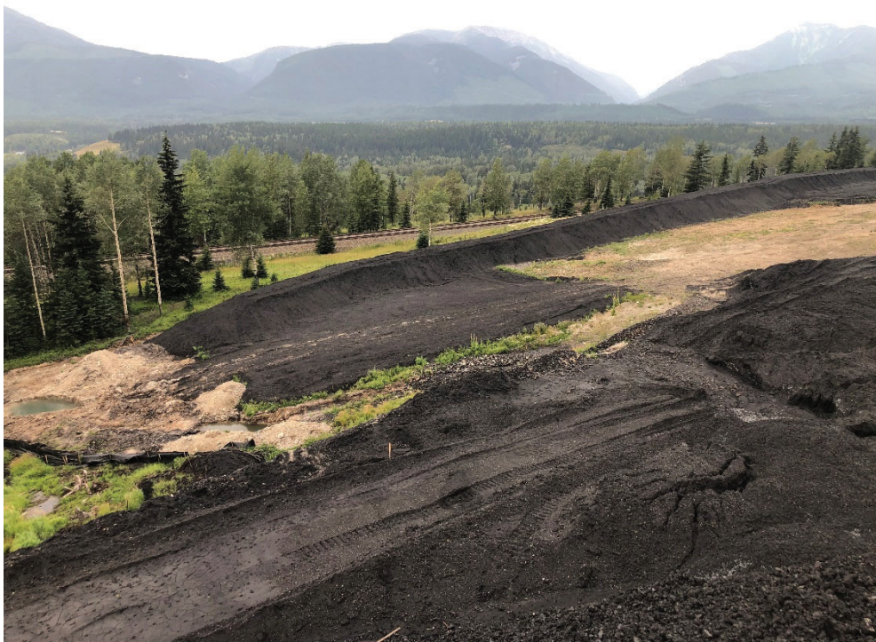
Photo 6. West runout berm constructed out of CCR, looking west
