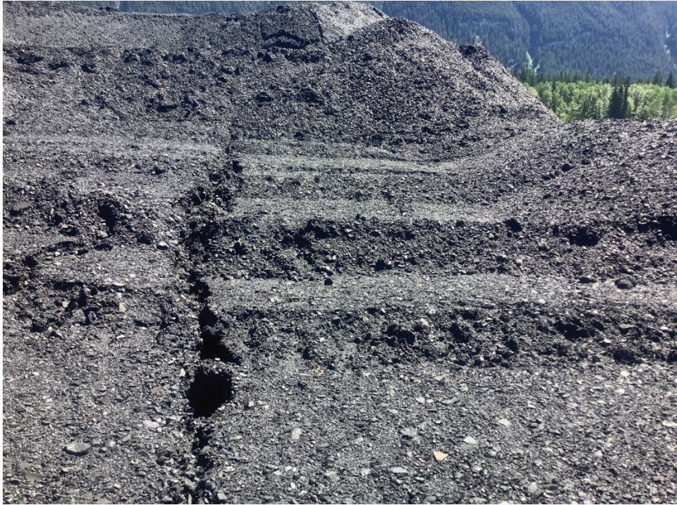
Photo 27. Crack along the 1300 m bench crest, looking east
