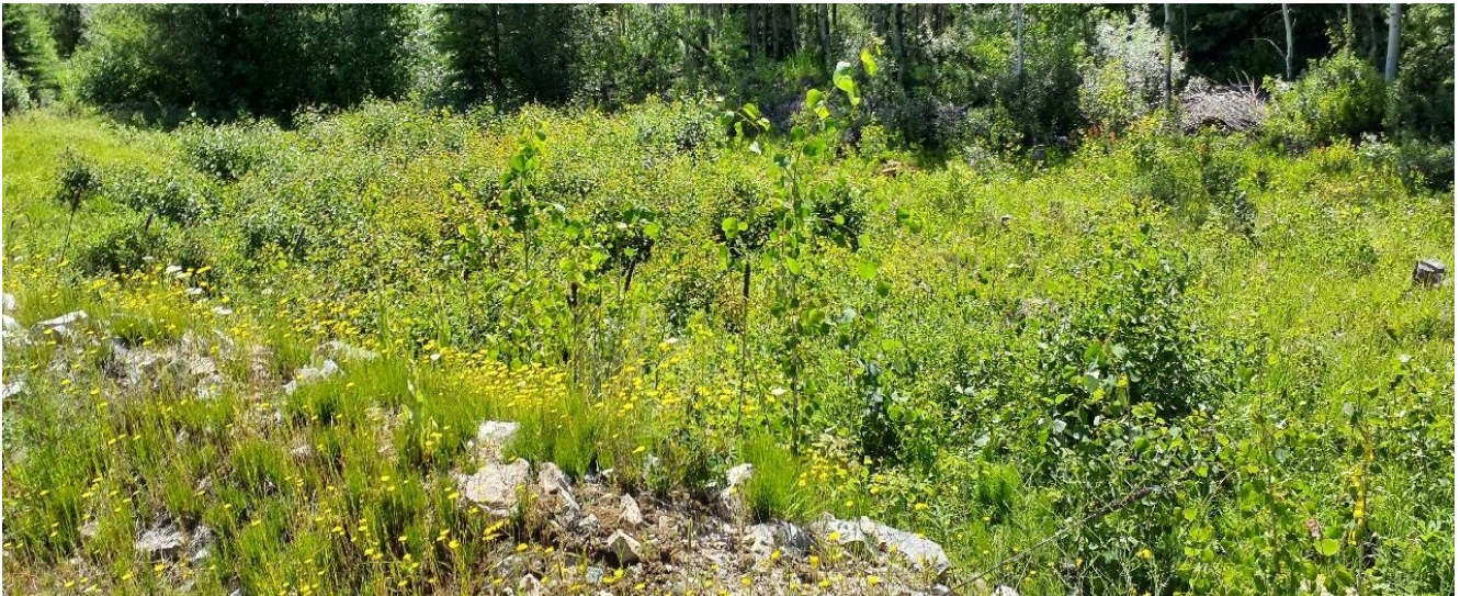
Photo I-C-7 Spillway channel looking toward south. Channel is observed to be >98% vegetated. HVC report that vegetation along the inlet of the spillway channel and inlet were cleared after site visit. (TRJ-2022-09)
