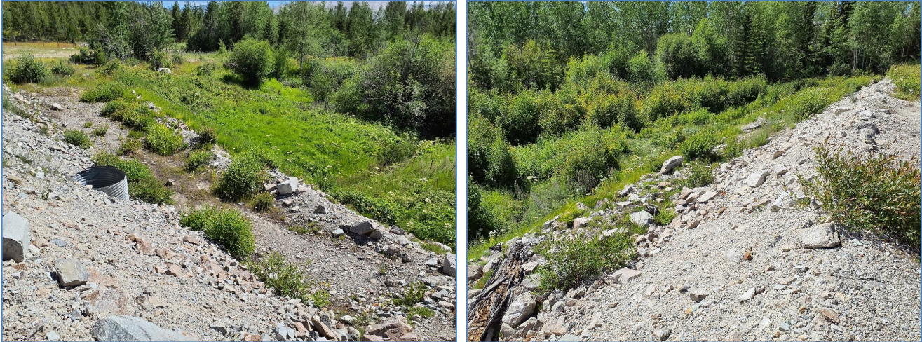
Photo I-C-3 View of downstream slope and outlet of spillway overflow pipe through the dam (TRJ-2022-10)
