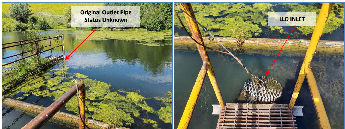
Photo I-B-5 Overview of the pond and LLO inlet which had minor debris that was cleared during inspection (TRJ-2022-08)
