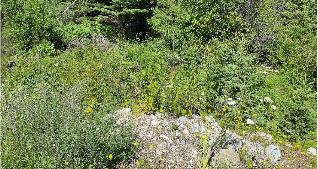
Photo I-C-7 Spillway channel looking toward south. Channel is observed to be >98% vegetated. HVC report that vegetation along the inlet of the spillway channel and inlet were cleared after site visit. (TRJ-2022-09)
