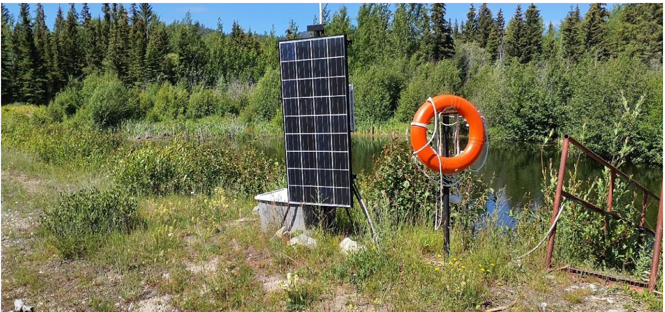
Photo I-C-5 View of solar panel for remote pond level monitoring. Remote monitoring has been effective to trigger inspections when pond levels rise (TRJ-2022-13)
