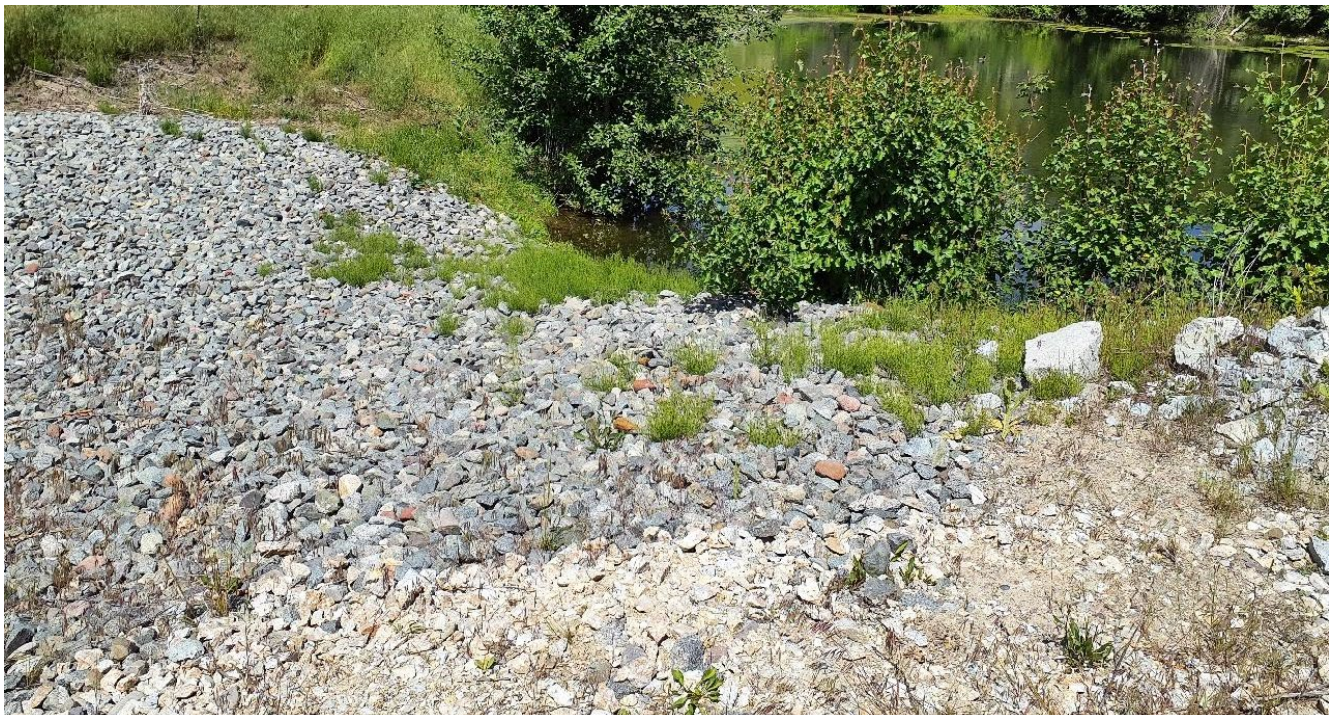
Photo I-B-3 Overview of pond and spillway inlet which has vegetation debris that will be removed during routine maintenance (TRJ-2022-07)
