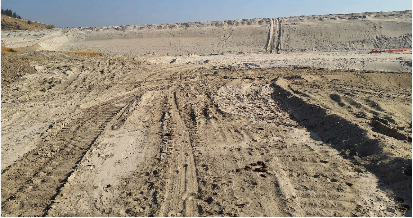
Photo I-A-6 North Dam Bedrock downstream slope (looking northeast). (LL-2022-11)
