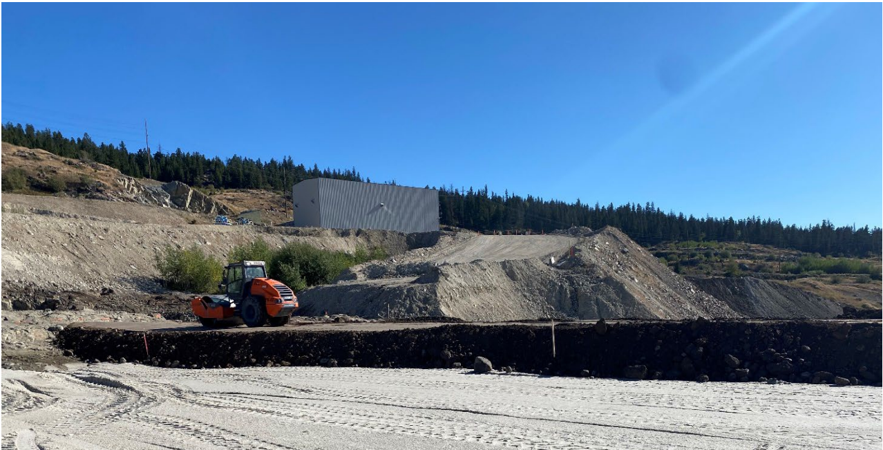
Photo I-A-9 T2 placement of dam core near south abutment. (LL-2022-05)
