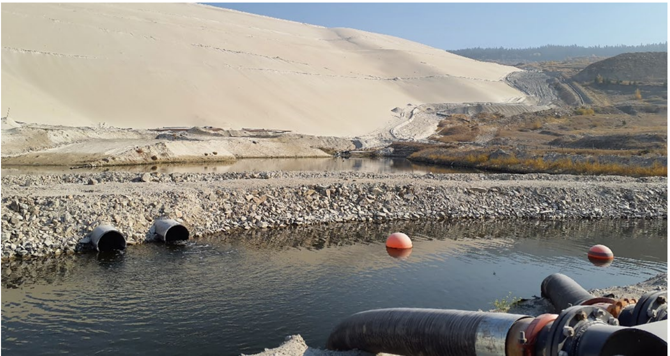
Photo I-A-11 Sediment Pond 1 South Cell and the internal rockfill berm which keeps retained sediments away from pump intakes and Seepage Water Reclaim Pond. (LL-2022-06)
