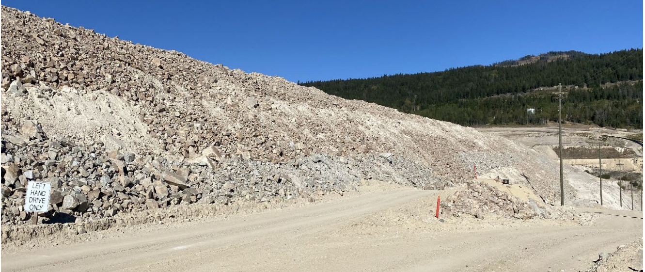
Photo I-B-9 H-H Dam downstream slope and 24 Mile Waste Dump / buttress area looking southwest from north side haul road. Power line along the toe of slope to be relocated out of area to allow 2023 buttress fill placement. Replacement power poles are visible along access road built into downstream slope. (HH-2022-10)
