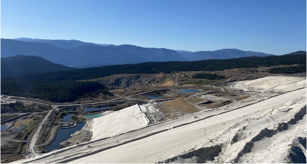
Photo I-A-9 T2 placement of dam core near south abutment. (LL-2022-05)
