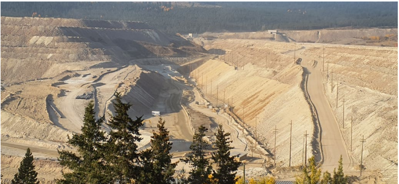
Photo I-B-9 H-H Dam downstream slope and 24 Mile Waste Dump / buttress area looking southwest from north side haul road. Power line along the toe of slope to be relocated out of area to allow 2023 buttress fill placement. Replacement power poles are visible along access road built into downstream slope. (HH-2022-10)
