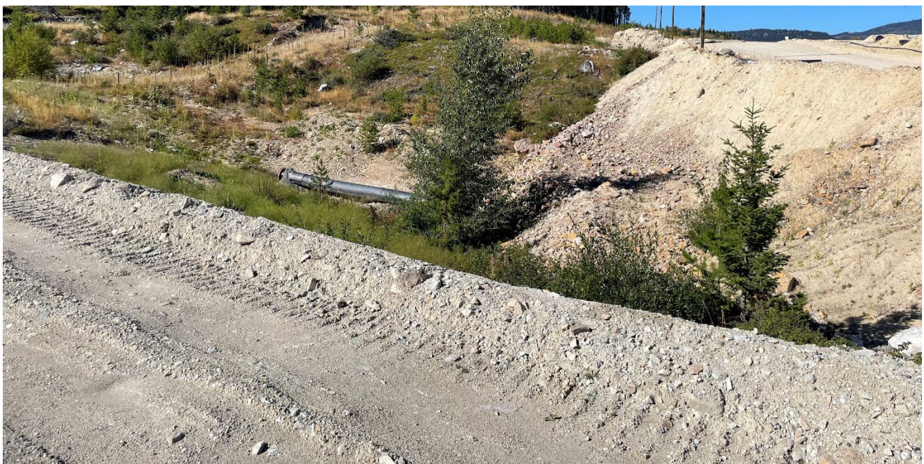
Photo I-B-3 The inlet of the Mystery Creek culvert that extends west of the south side mine road. The pipe was grouted and inlet capped during decommissioning. (HH-2022-11)
