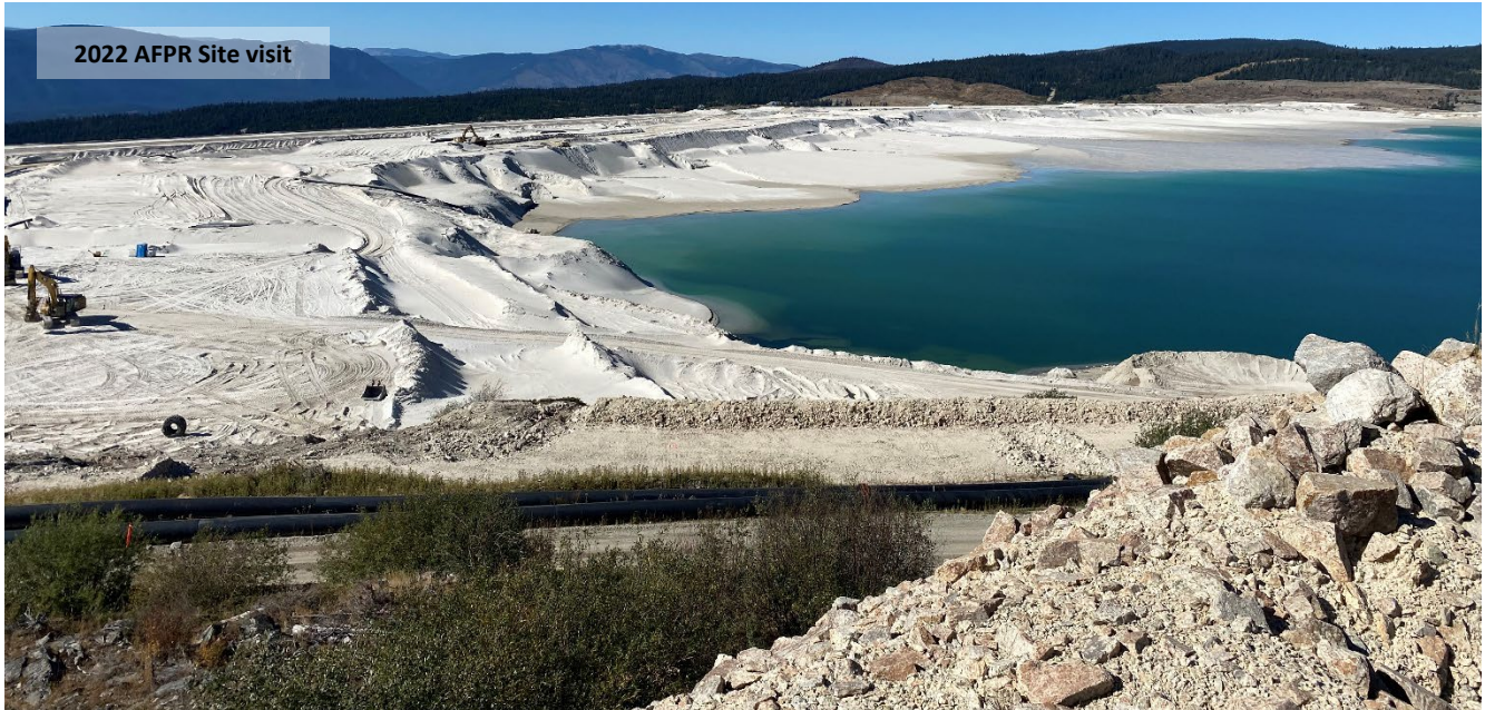
Photo I-A-3 Tailings beach and upstream cycloned sand hydraulic placement cells along South Dam and VBB segments during 2021 and 2022 AFPR site visits. (LL-2022-02)
