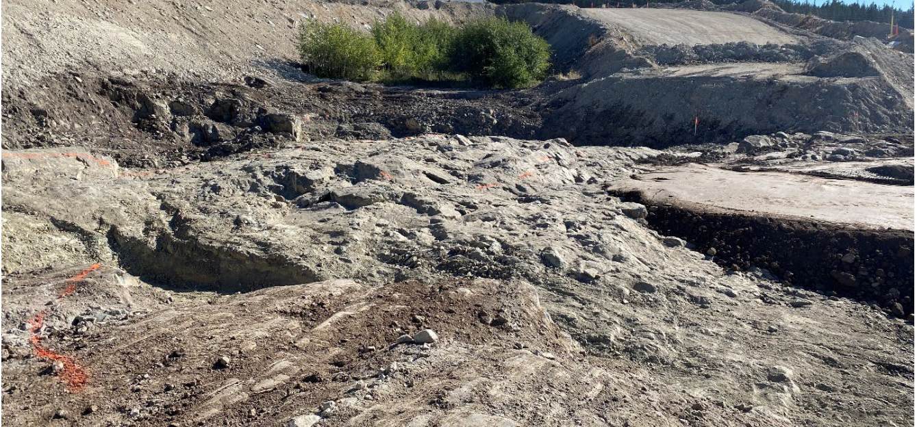
Photo I-A-11 Sediment Pond 1 South Cell and the internal rockfill berm which keeps retained sediments away from pump intakes and Seepage Water Reclaim Pond. (LL-2022-06)
