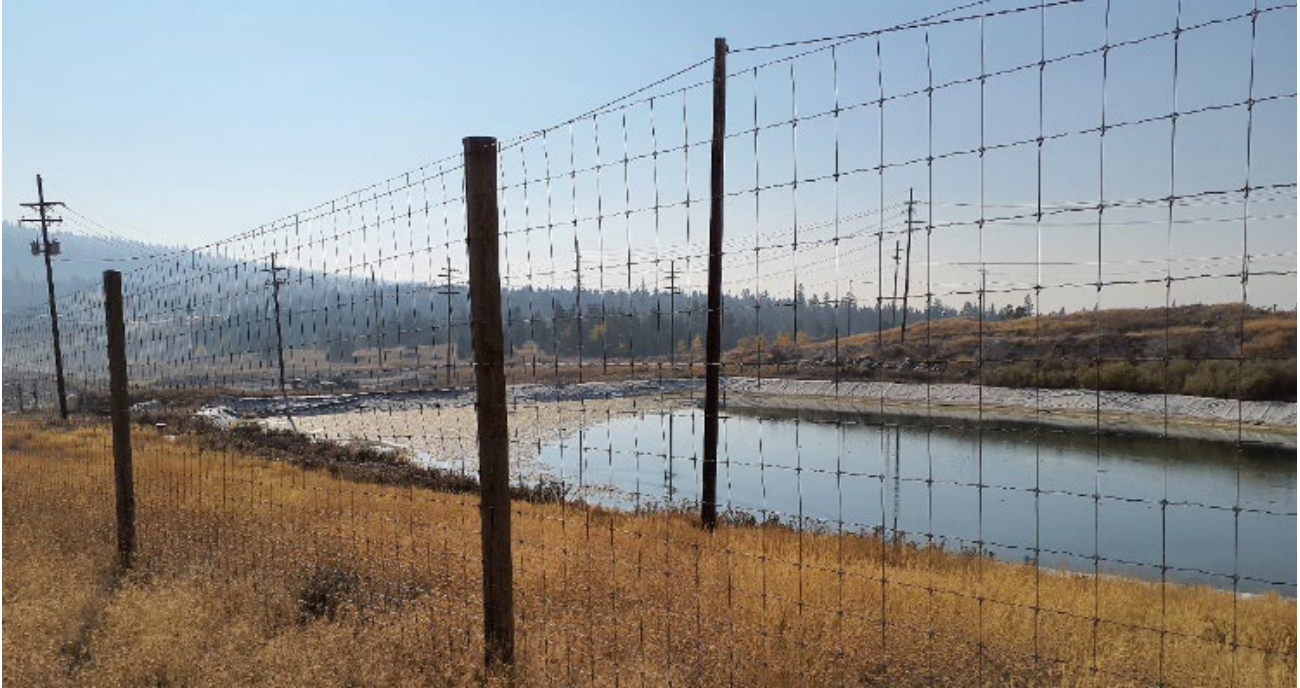
Photo I-A-14 Seepage Pond 2, southern half. Outlet to Seepage Pond 2 was not obstructed during site visit. (LL-2022-08)
