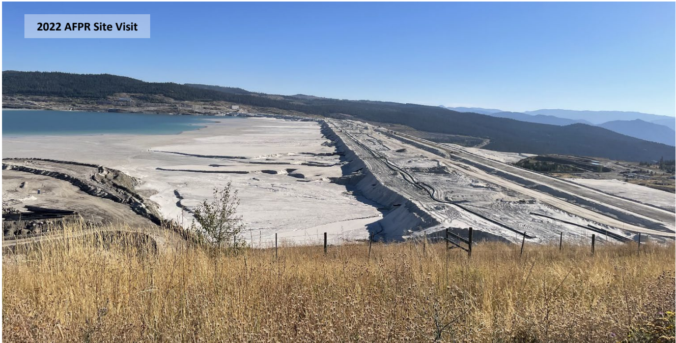
Photo I-A-2 Tailings beach and upstream cycloned sand hydraulic placement cells along North Dam U-GLU and North Dam Bedrock segments during 2021 and 2022 AFPR site visits. (LL-2022-01)
