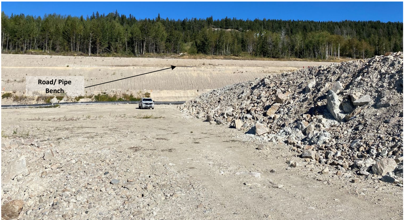
Photo I-B-7 H-H Pipe Bench and access road which crosses dam crest and waste fill platform extended onto tailings beach immediately upstream of west abutment. (HH-2022-05)
