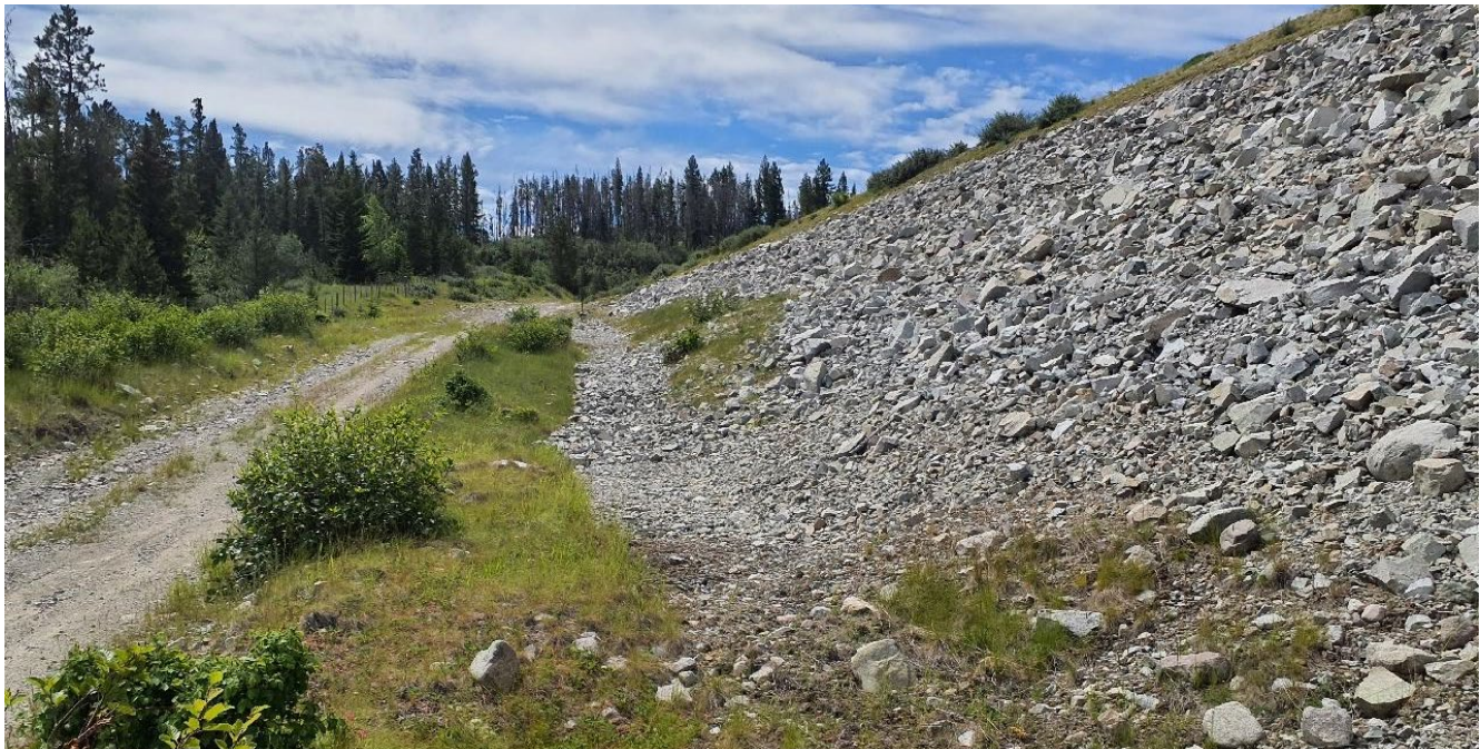
Photo I-B-5 View of downstream slope. Vegetation cover over lower portion of slope suggests this segment of downstream slope is comprised of glacial till fill. No sign of erosion of slope (rock or glacial till) was observed (BTH-2022-10)
