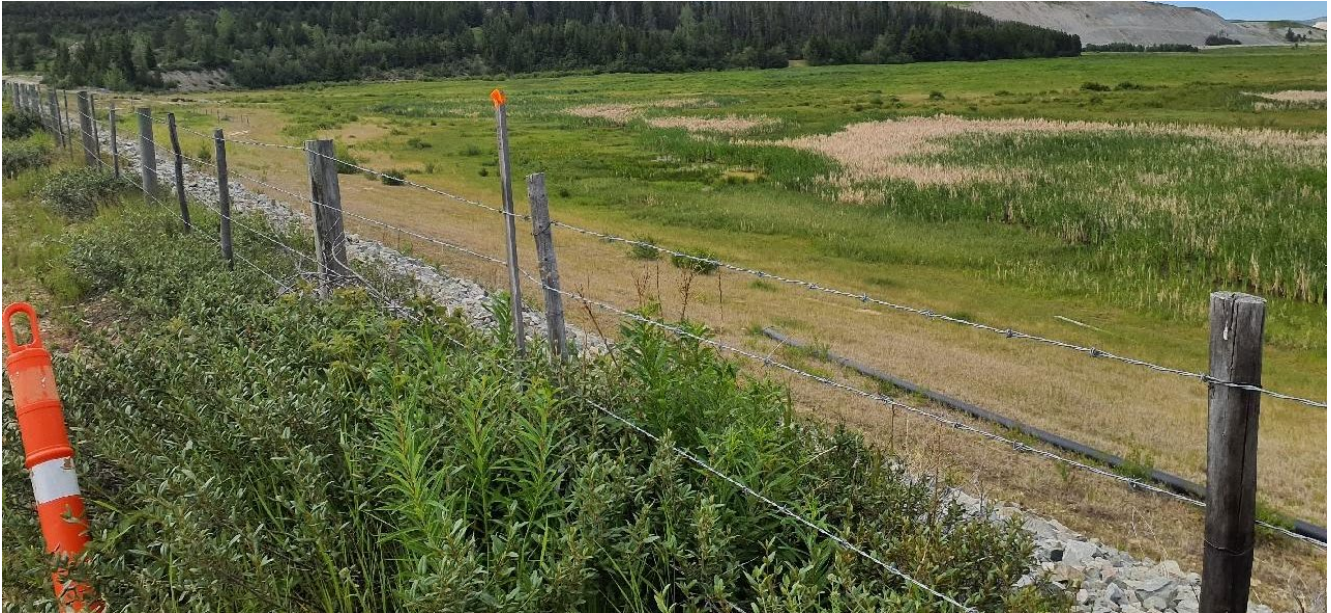
Photo I-B-9 Spillway inlet and approach channel. Channel is vegetated with grass and bushes. Clearing of vegetation is managed as part of routine maintenance (BTH-2022-11)
