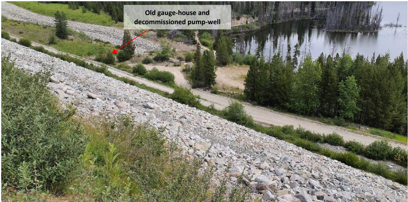
Photo I-B-5 View of downstream slope. Vegetation cover over lower portion of slope suggests this segment of downstream slope is comprised of glacial till fill. No sign of erosion of slope (rock or glacial till) was observed (BTH-2022-10)
