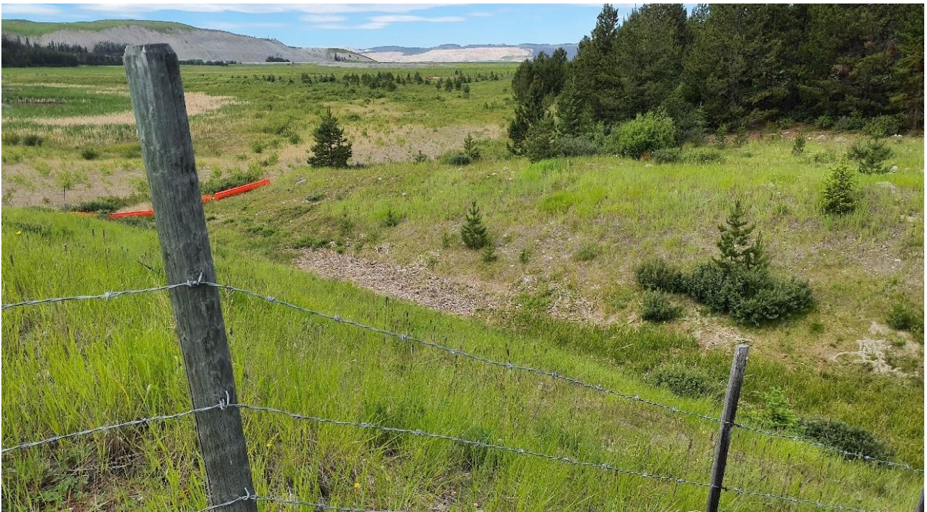
Photo I-B-9 Spillway inlet and approach channel. Channel is vegetated with grass and bushes. Clearing of vegetation is managed as part of routine maintenance (BTH-2022-11)
