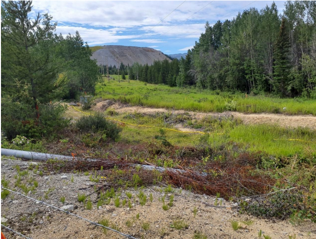
Photo I-C-7 Segment of R3 Seepage Pond LLO pipe that backed up and resulted in spillway discharge, refer to discussion in main text (BTH-2022-16)
