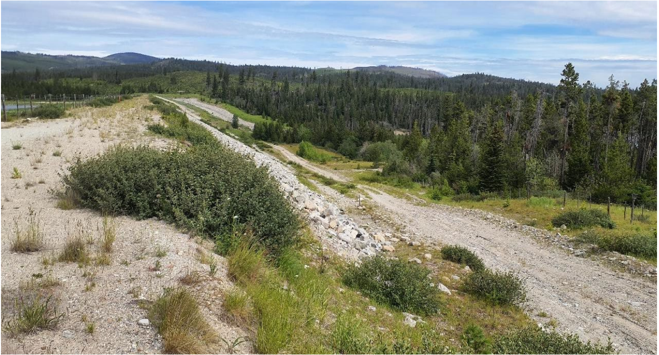
Photo I-B-3 Left abutment with no observation of erosion scours or damage (BTH-2022-09)
