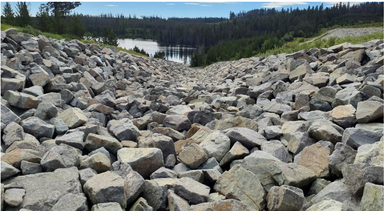
Photo I-B-11 Riprap lined portion of spillway channel looking towards Bose Lake (BTH-2022-12)
