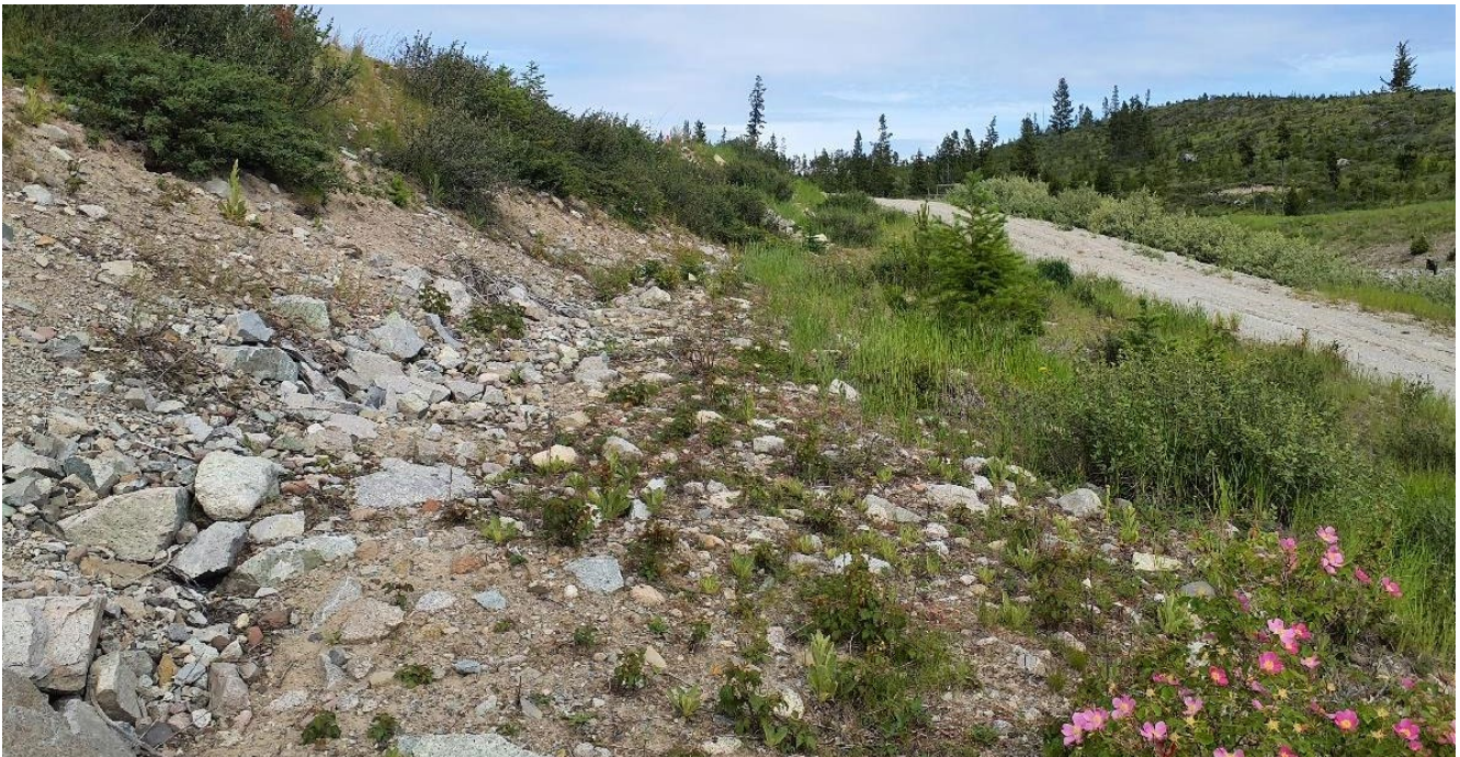
Photo I-B-3 Left abutment with no observation of erosion scours or damage (BTH-2022-09)
