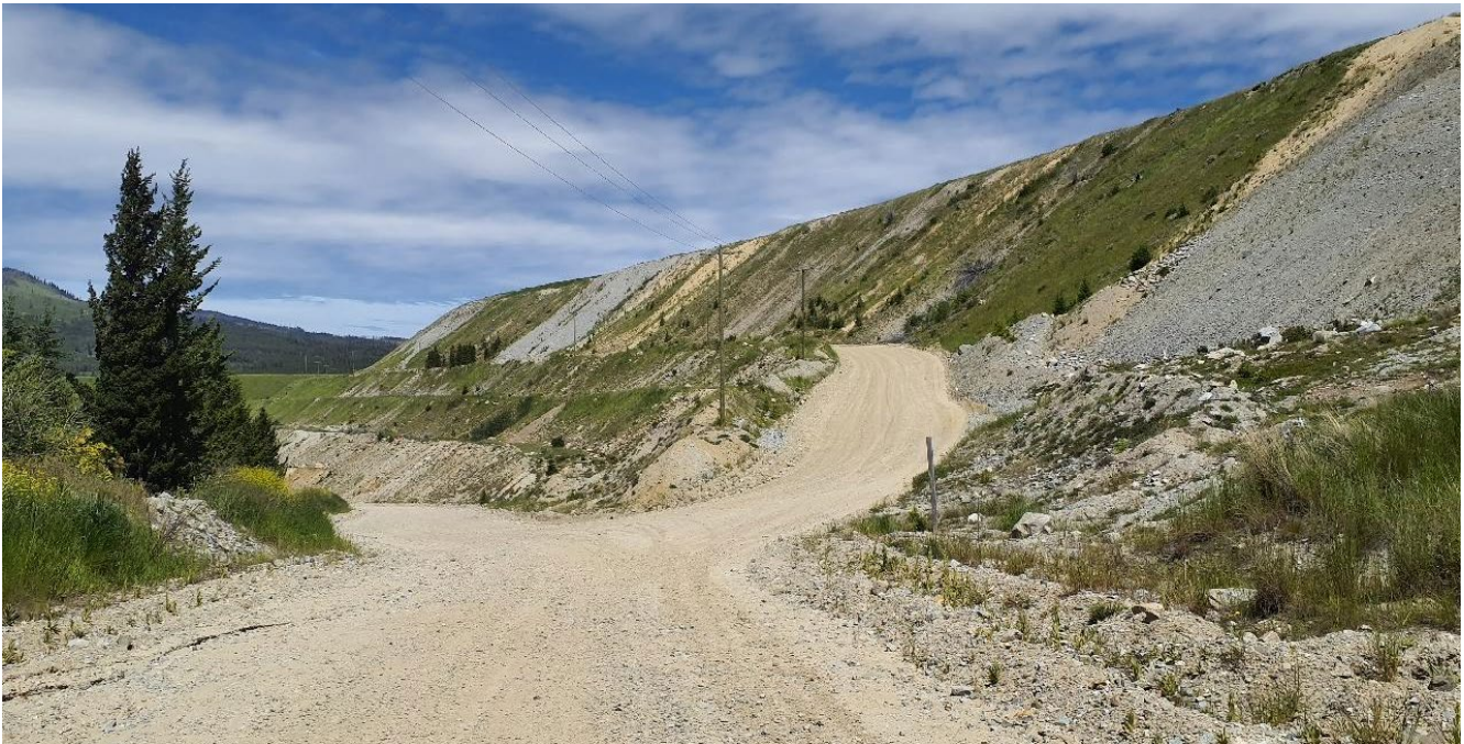
Photo I-A-6 Overview of downstream slope and toe from Trojan Dam. No new erosion areas were observed, and previous repairs are holding up well (BTH-2022-06)
