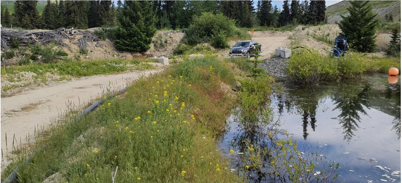
Photo I-C-3 View of R3 Seepage Pond and debris mesh for Low-Level Outlet (LLO). Clear water was flowing at the time of the site visit. The debris mesh is clogged below and above water (BTH-2022-14)
