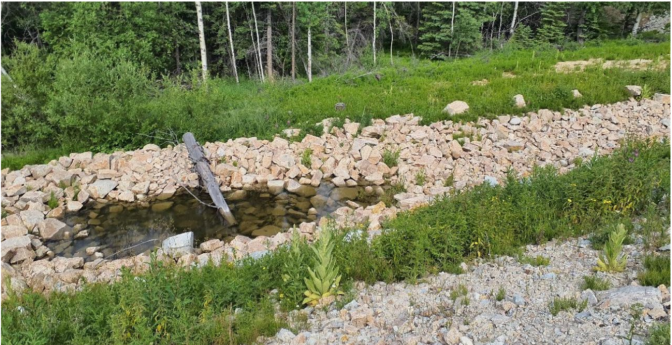
Photo I-C-6 Spillway channel at midpoint, looking downstream (BTH-2022-13)
