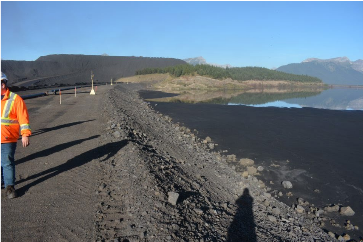
Photograph 10: Main Tailings Dam – Upstream Slope, Crest and Beach, looking Southwest, 30 August 2022
