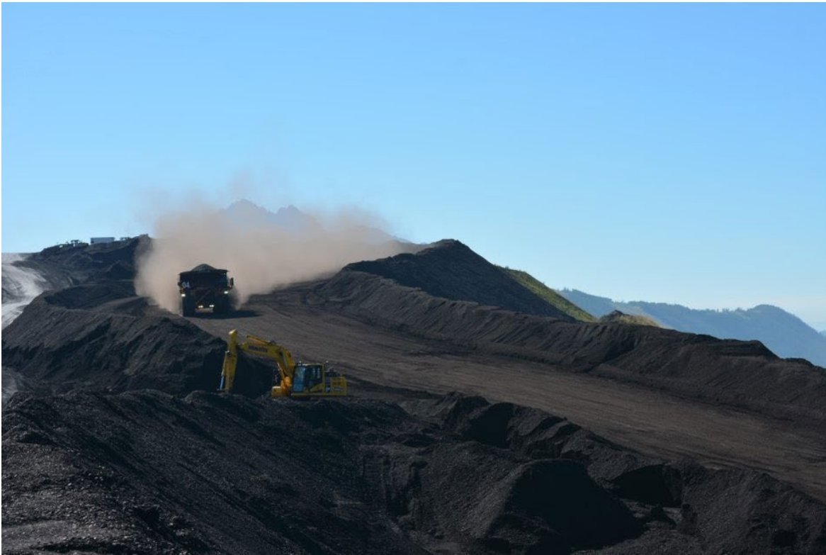
Photograph 21: Construction of Process Plant Light Vehicle Access Road, Looking Southwest, 30 August 2022
