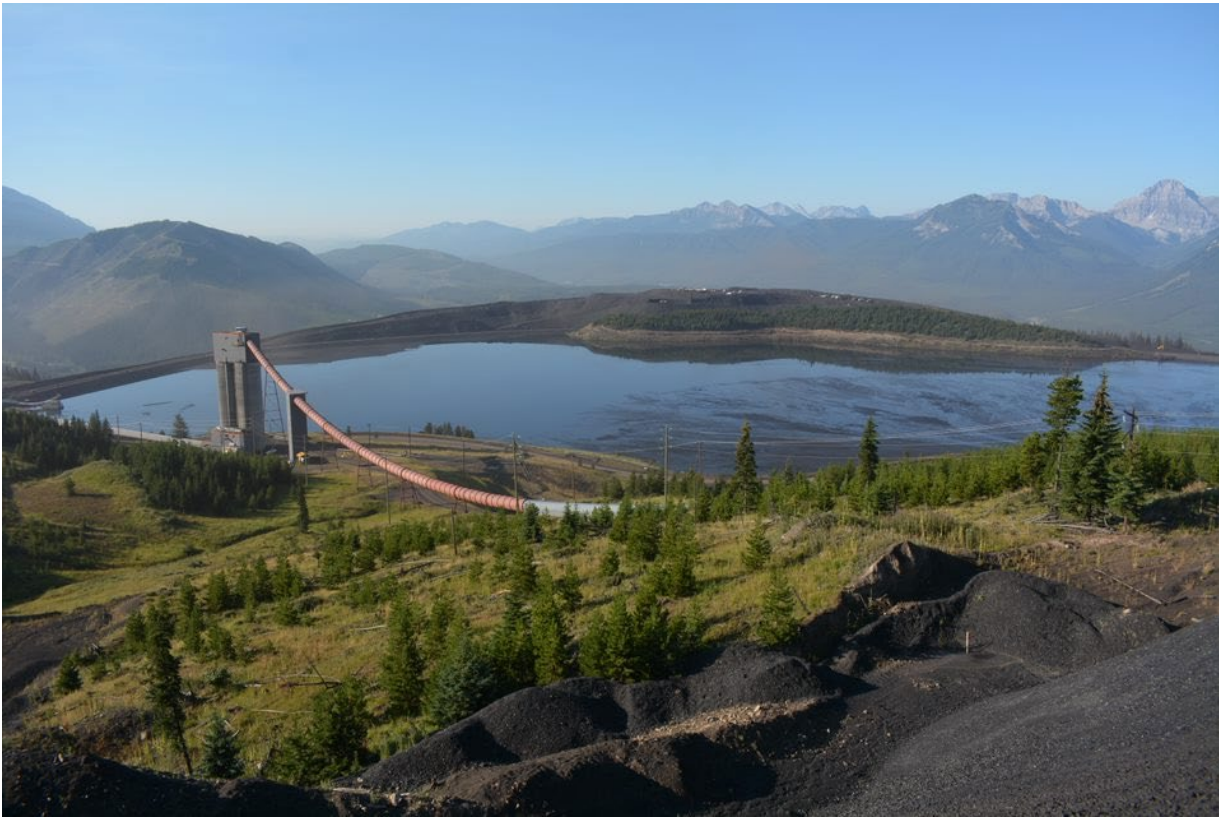
Photograph 1: Tailings Storage Facility – Overview, Looking Southwest, 30 August 2022
