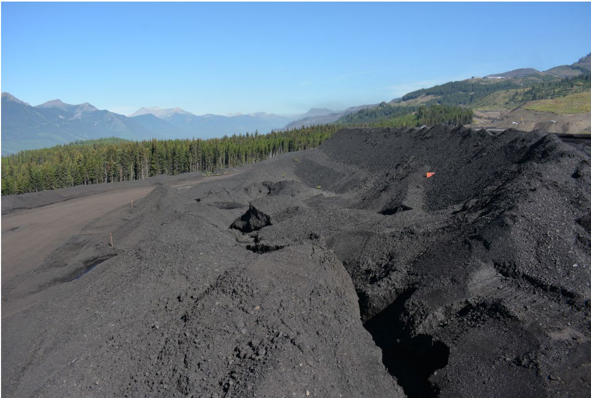
Photograph 23: West Tailings Dam – Downstream Slope; Looking Northwest, 30 August 2022
