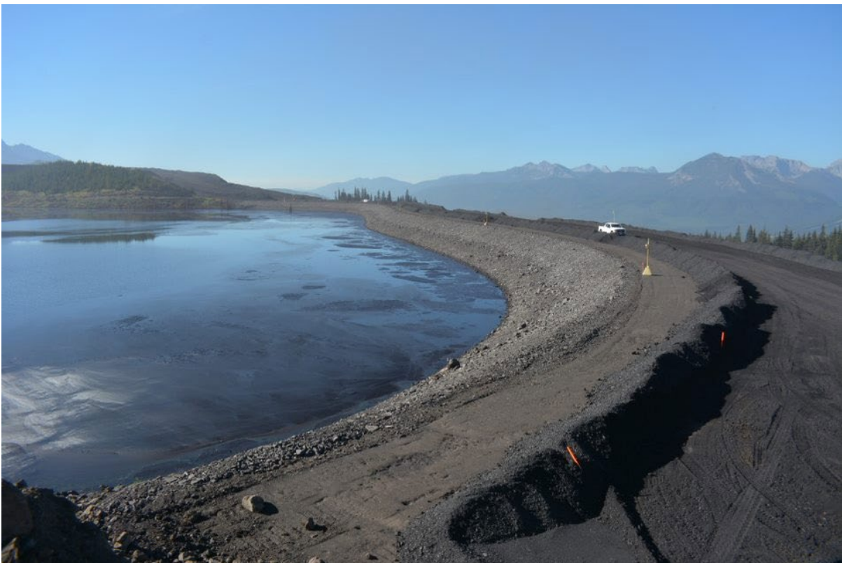
Photograph 16: West Tailings Dam – Upstream Slope and Crest; Looking South, 30 August 2022
