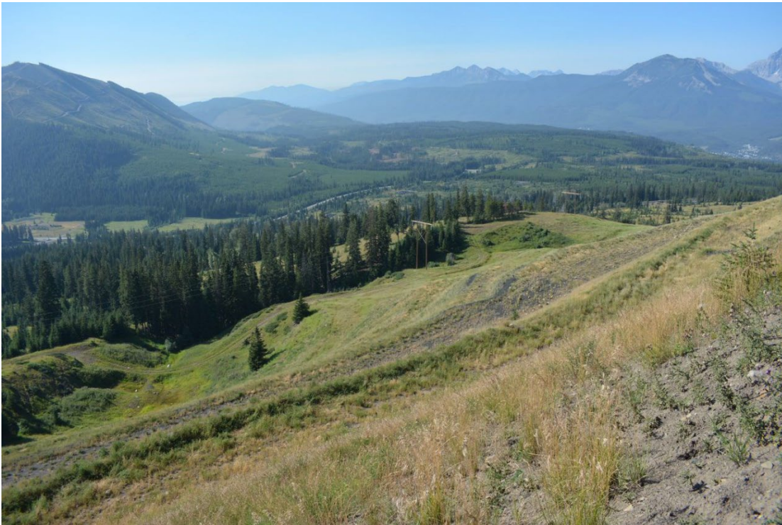
Photograph 37: Site D CCR Facility – Downstream Slope and Toe Area, Looking southwest, 30 August 2022
