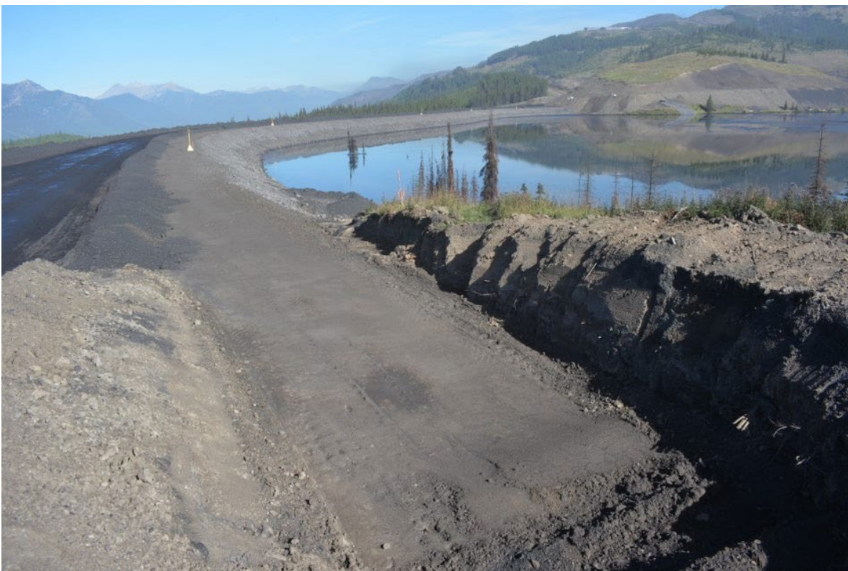
Photograph 20: West Tailings Dam – South Abutment; Looking North, 30 August 2022
