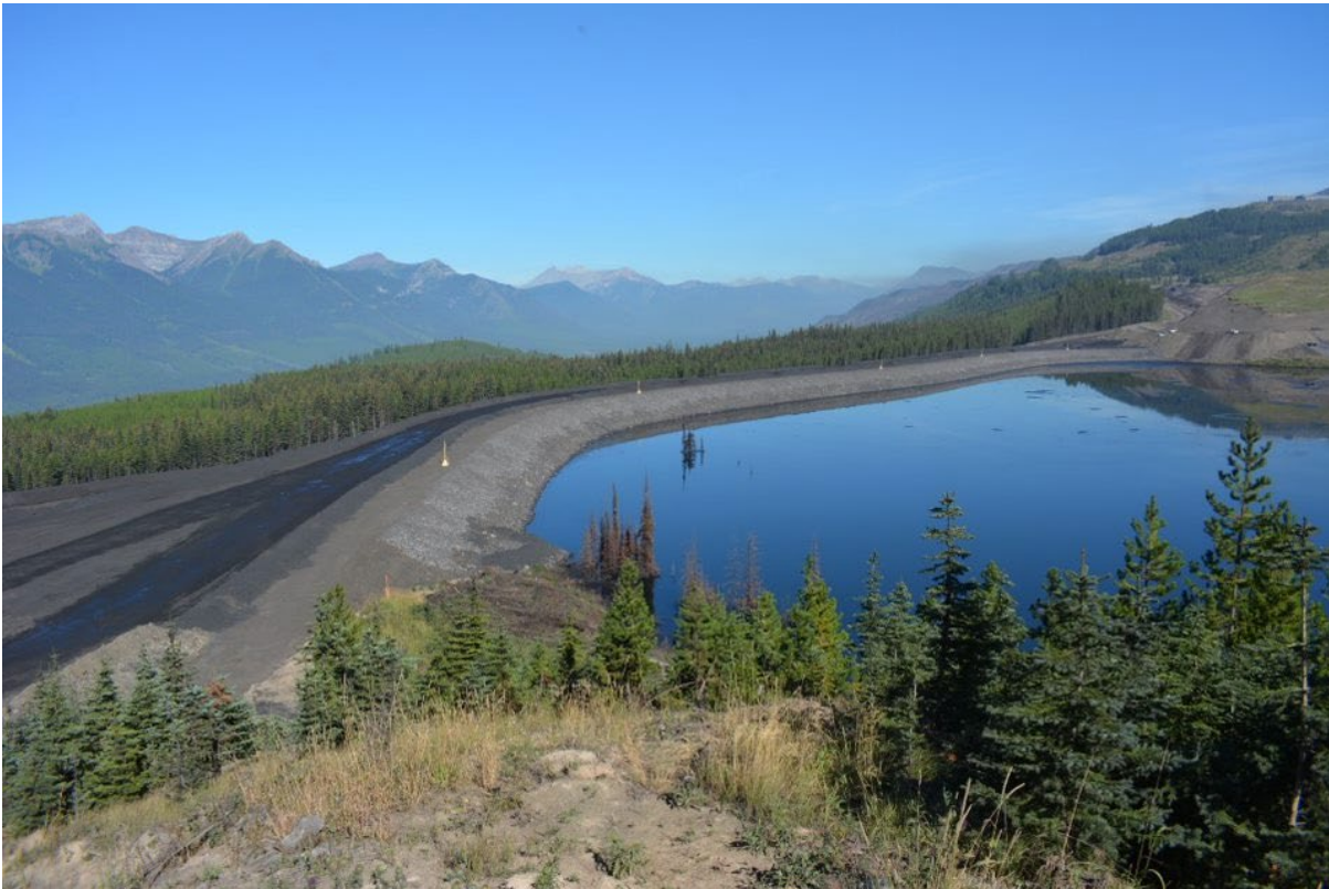
Photograph 15: West Tailings Dam – Overview; Looking North, 30 August 2022
