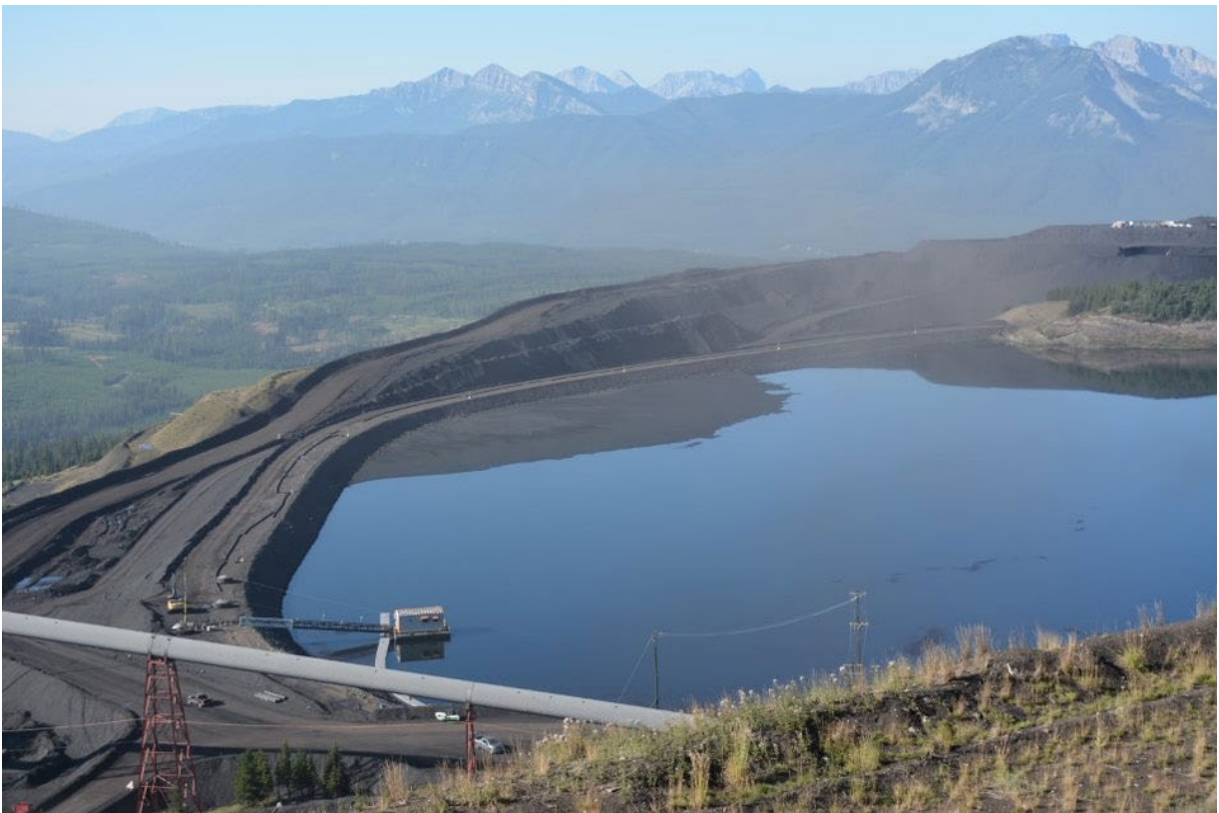
Photograph 2: Main Tailings Dam – Overview, Looking Southwest, 30 August 2022
