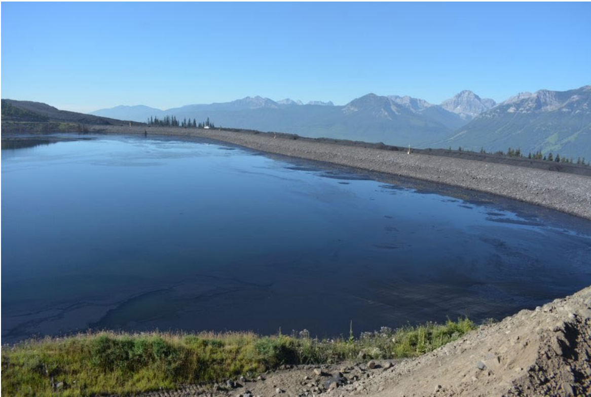
Photograph 17: West Tailings Dam – Upstream Slope and Crest; Looking Southwest, 30 August 2022
