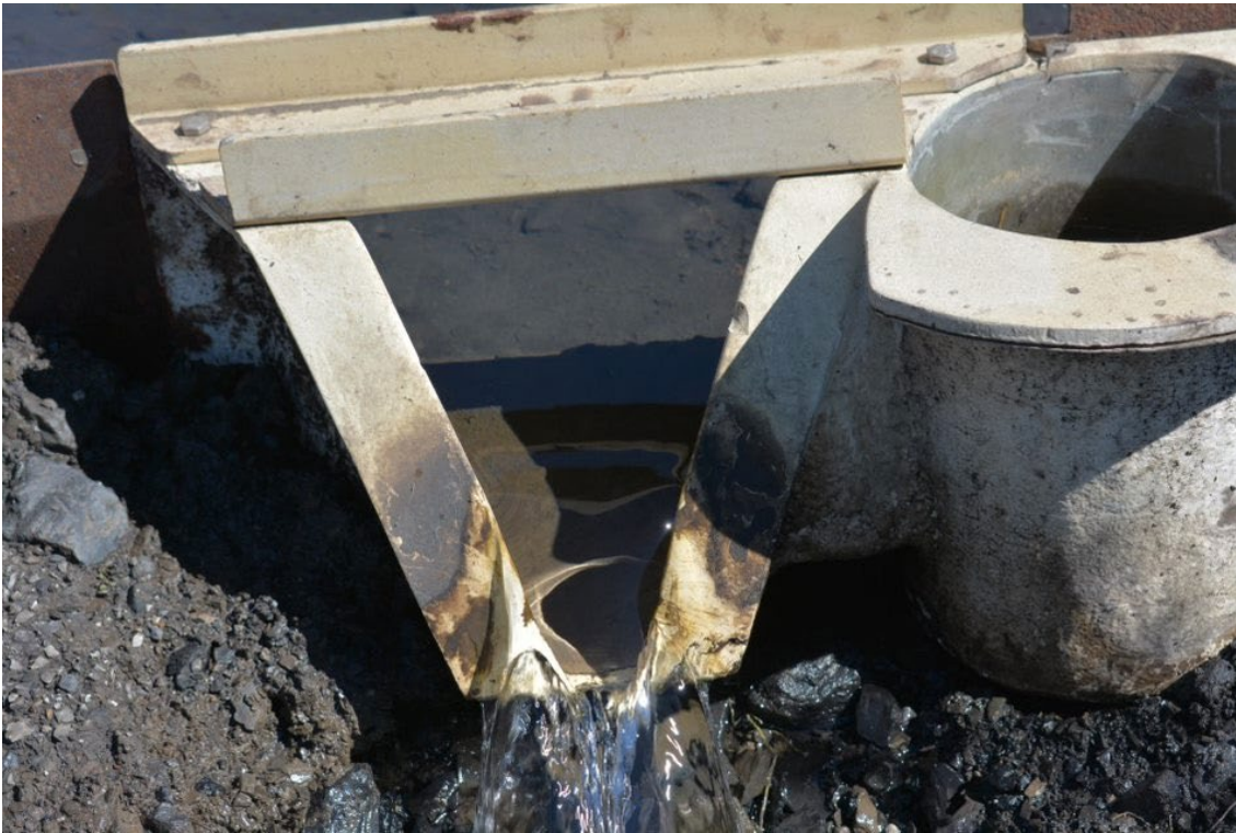
Photograph 25: West Tailings Dam – Seepage Weir, Looking North, 30 August 2022
