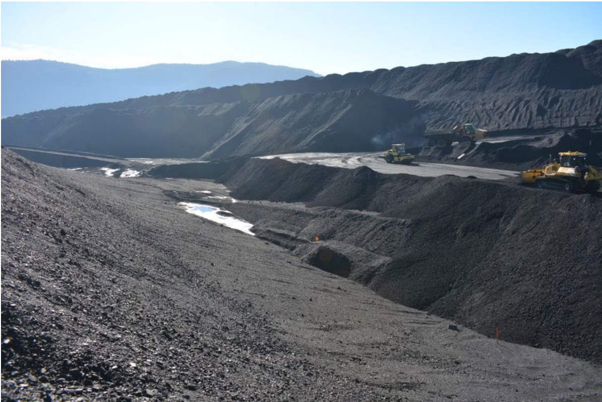
Photograph 13: Main Tailings Dam – Downstream Slope and Toe Area, Looking East, 30 August 2022
