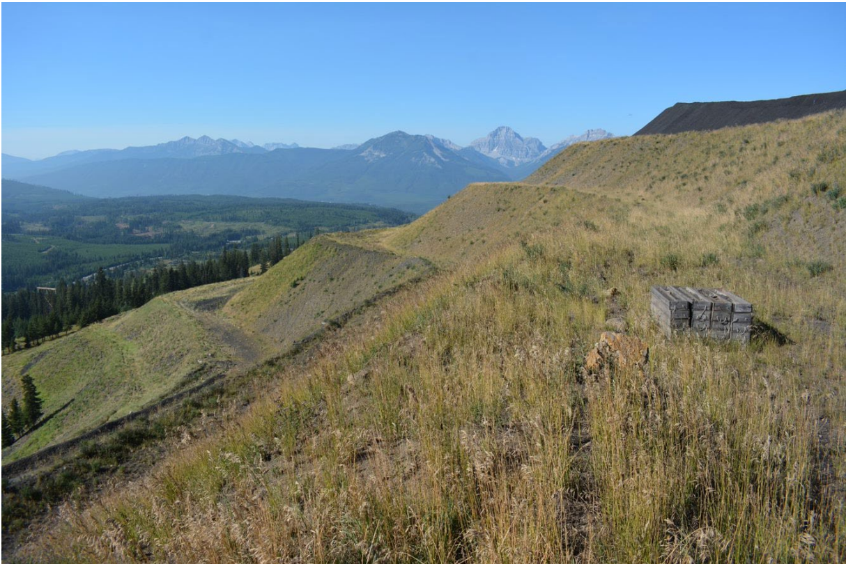
Photograph 33: Site C/D CCR Facility – Downstream Slopes, Looking southwest, 30 August 2022
