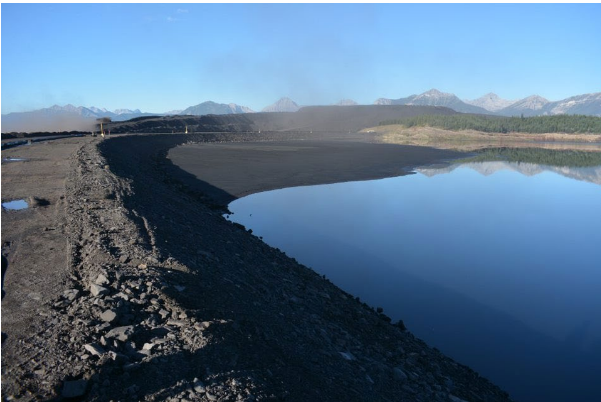
Photograph 8: Main Tailings Dam – Upstream Slope and Crest, Looking Southwest, 30 August 2022
