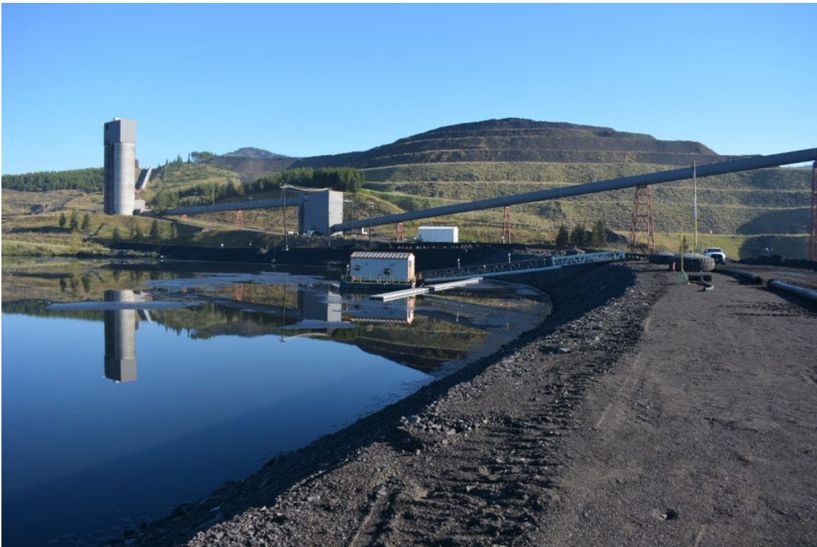
Photograph 6: Main Tailings Dam – Upstream Slope and Crest, Looking North, 30 August 2022
