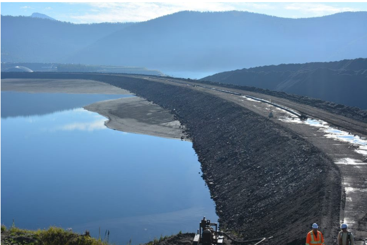
Photograph 12: Main Tailings Dam – Upstream Slope and Crest, Looking Northeast, 30 August 2022
