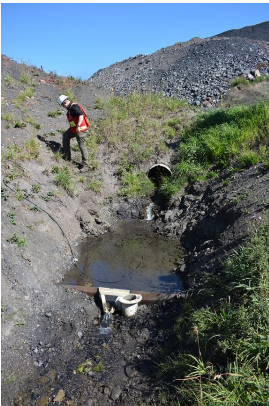
Photograph 24: West Tailings Dam – Seepage Weir, Looking North, 30 August 2022
