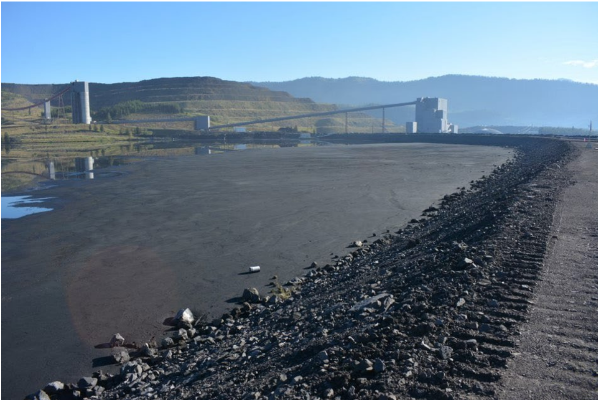
Photograph 11: Main Tailings Dam – Upstream Slope; Looking Northeast, 30 August 2022
