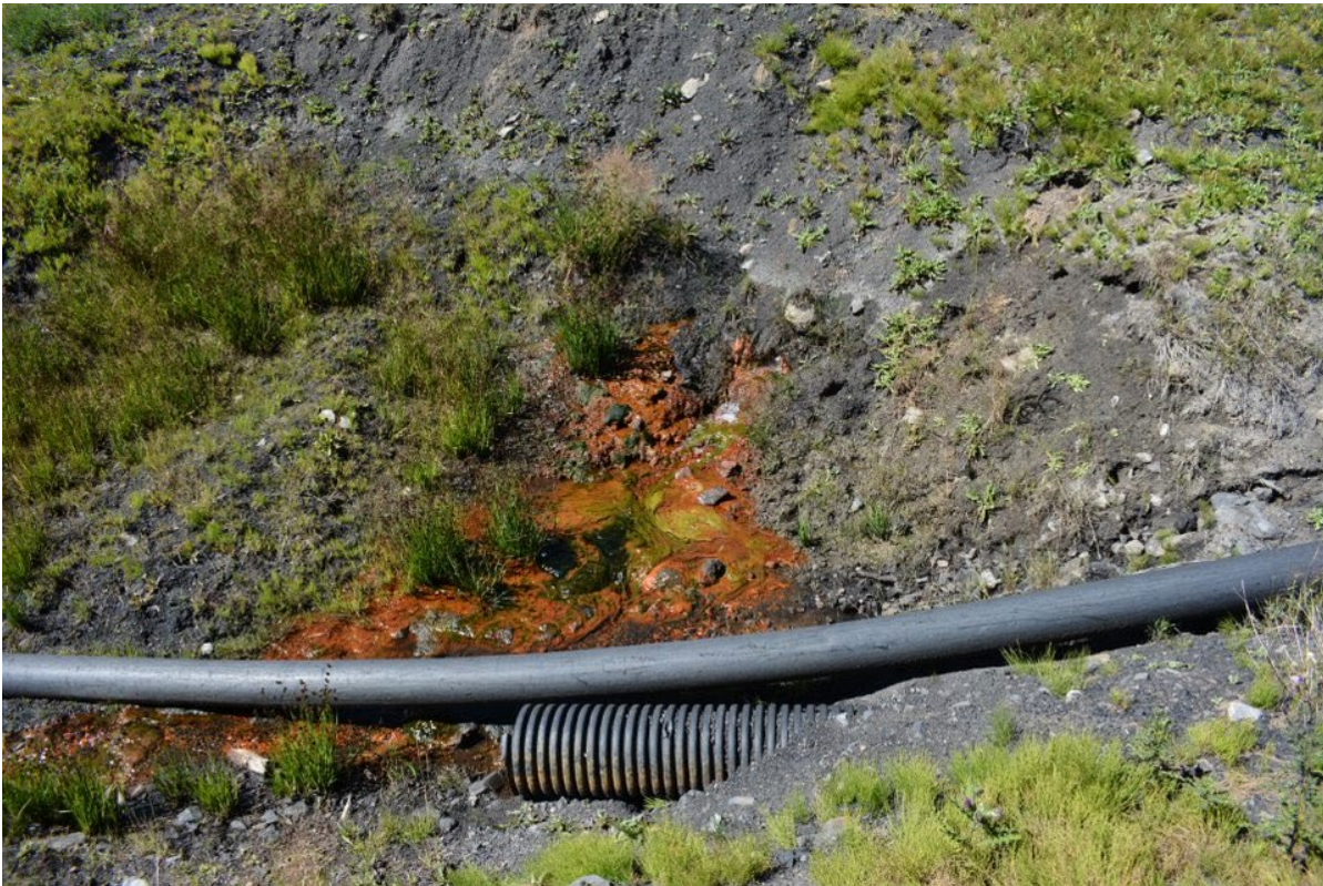
Photograph 29: Site C CCR Facility – Underdrain Seepage Flow, Looking Northwest, 30 August 2022
