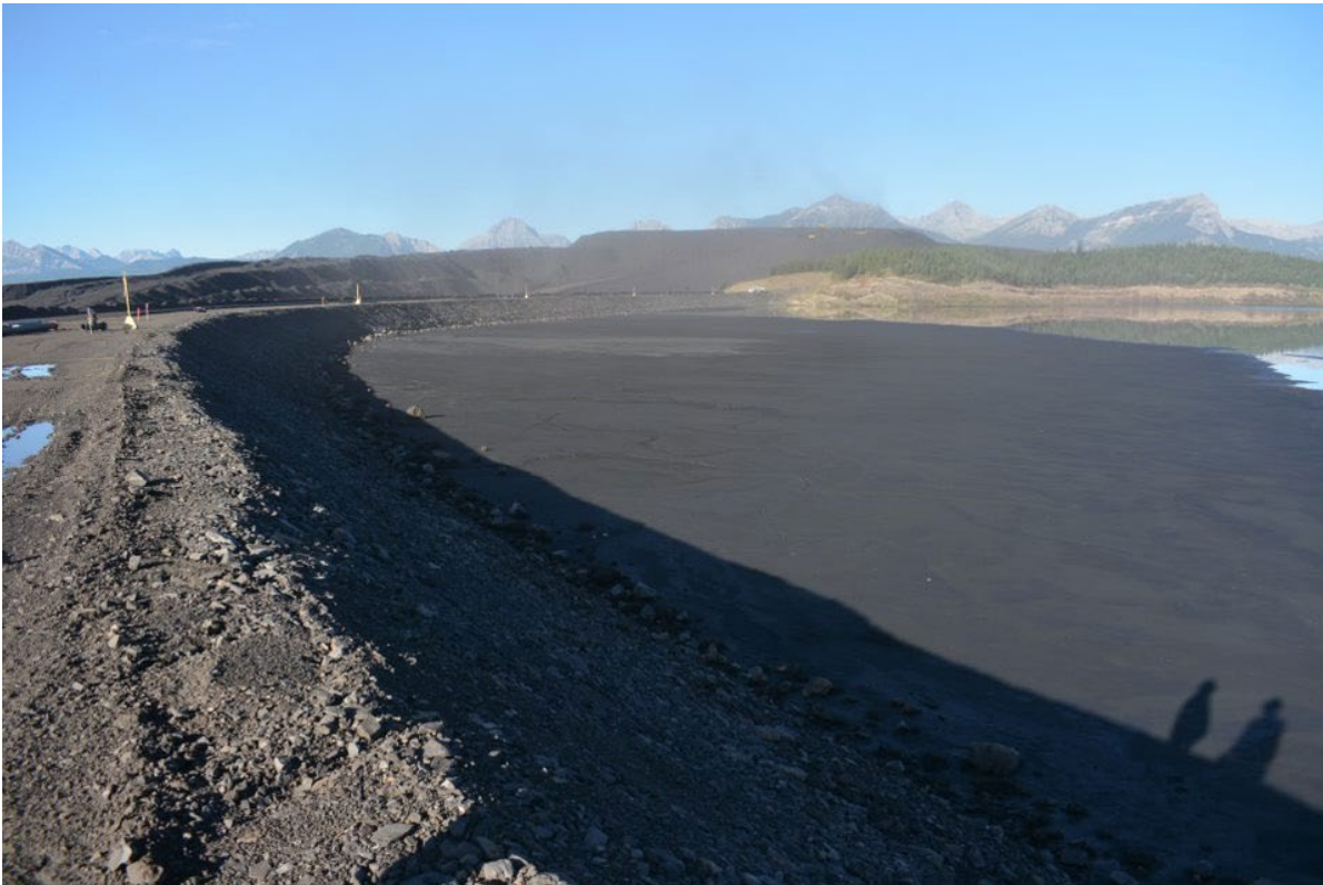
Photograph 9: Main Tailings Dam – Upstream Slope and Beach, Looking Southwest, 30 August 2022
