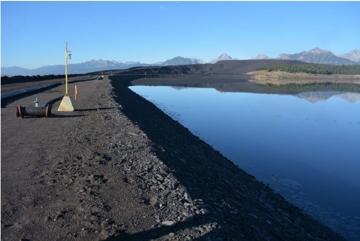
Photograph 7: Main Tailings Dam – Upstream Slope and Crest, Looking Southwest, 30 August 2022
