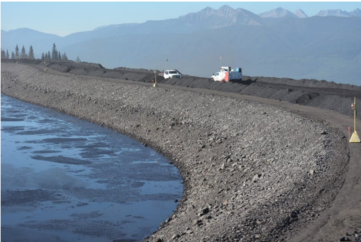
Photograph 18: West Tailings Dam – Upstream Slope and Crest; Looking Southwest, 30 August 2022
