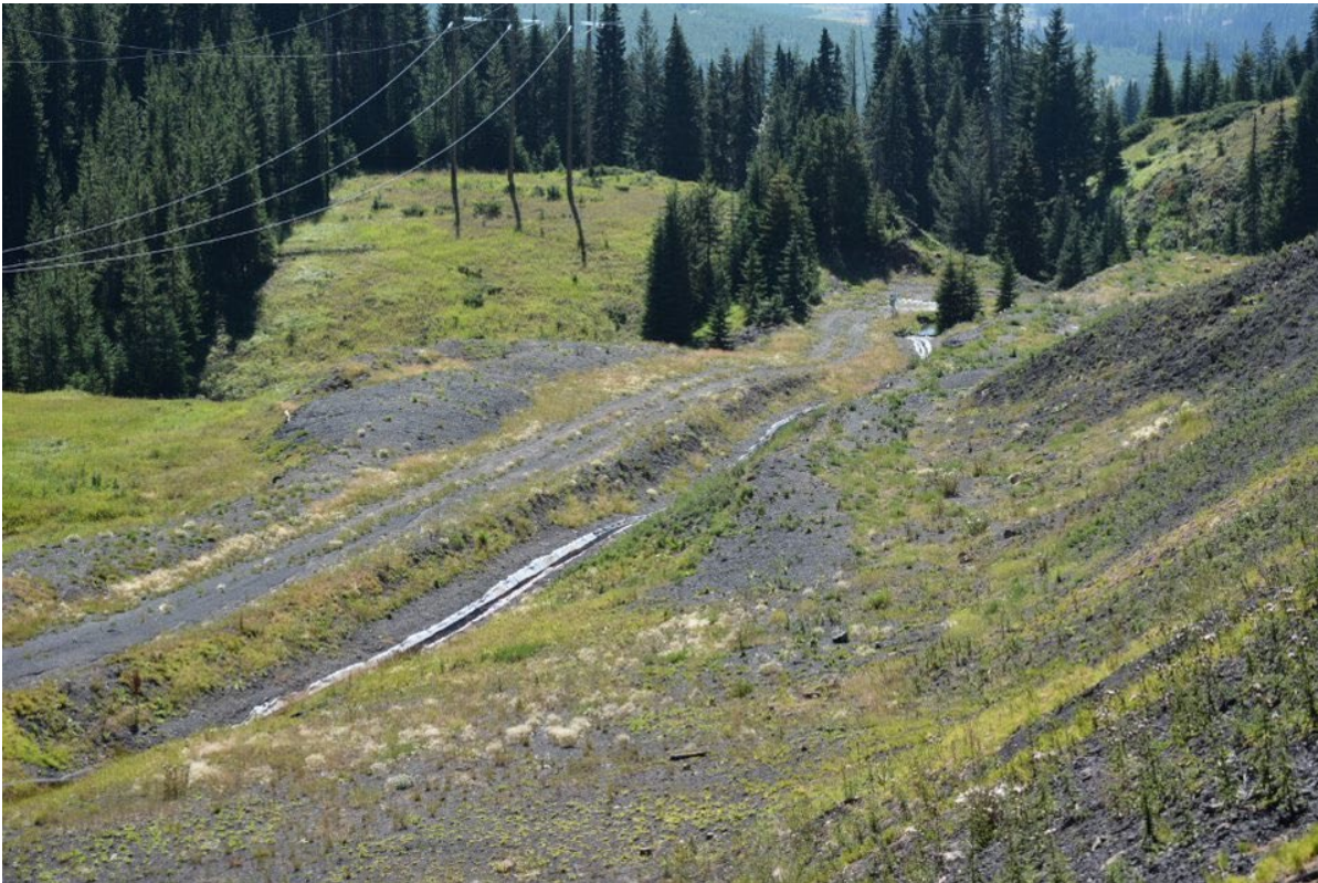
Photograph 27: Site C CCR Facility – Smart Drain at Toe, Looking Southwest, 30 August 2022
