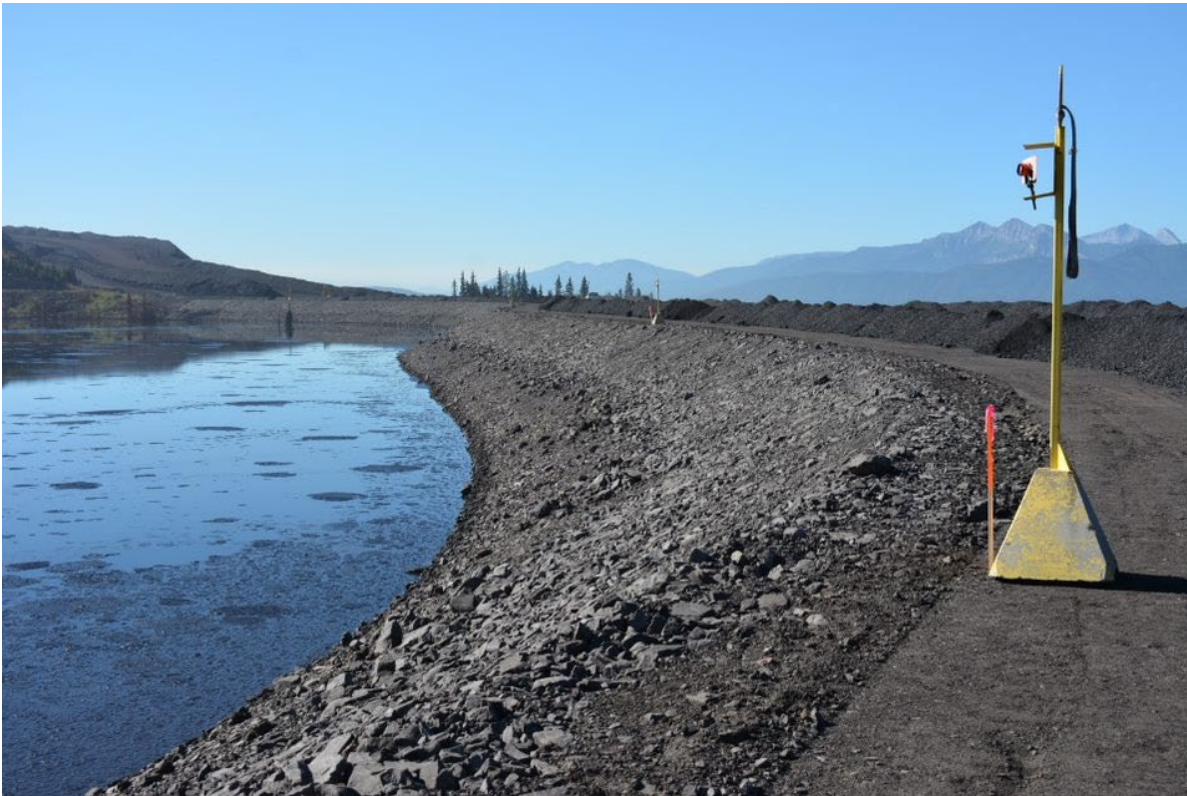
Photograph 19: West Tailings Dam – Upstream Slope, Looking South, 30 August 2022
