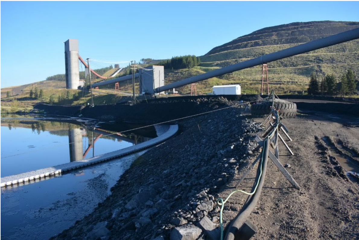
Photograph 5: Main Tailings Dam, North Abutment – Looking North, 30 August 2022
