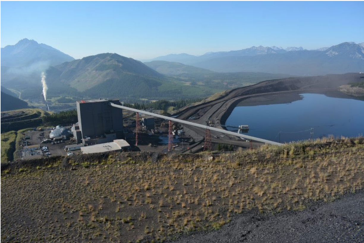
Photograph 3: Main Tailings Dam and Process Plant – Overview, Looking South, 30 August 2022
