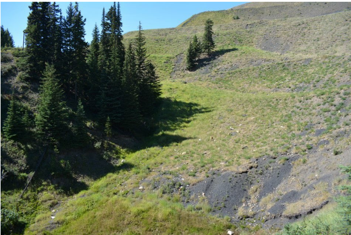
Photograph 32: Site C CCR Facility – Toe Area and Weir Discharge, Looking west, 30 August 2022
