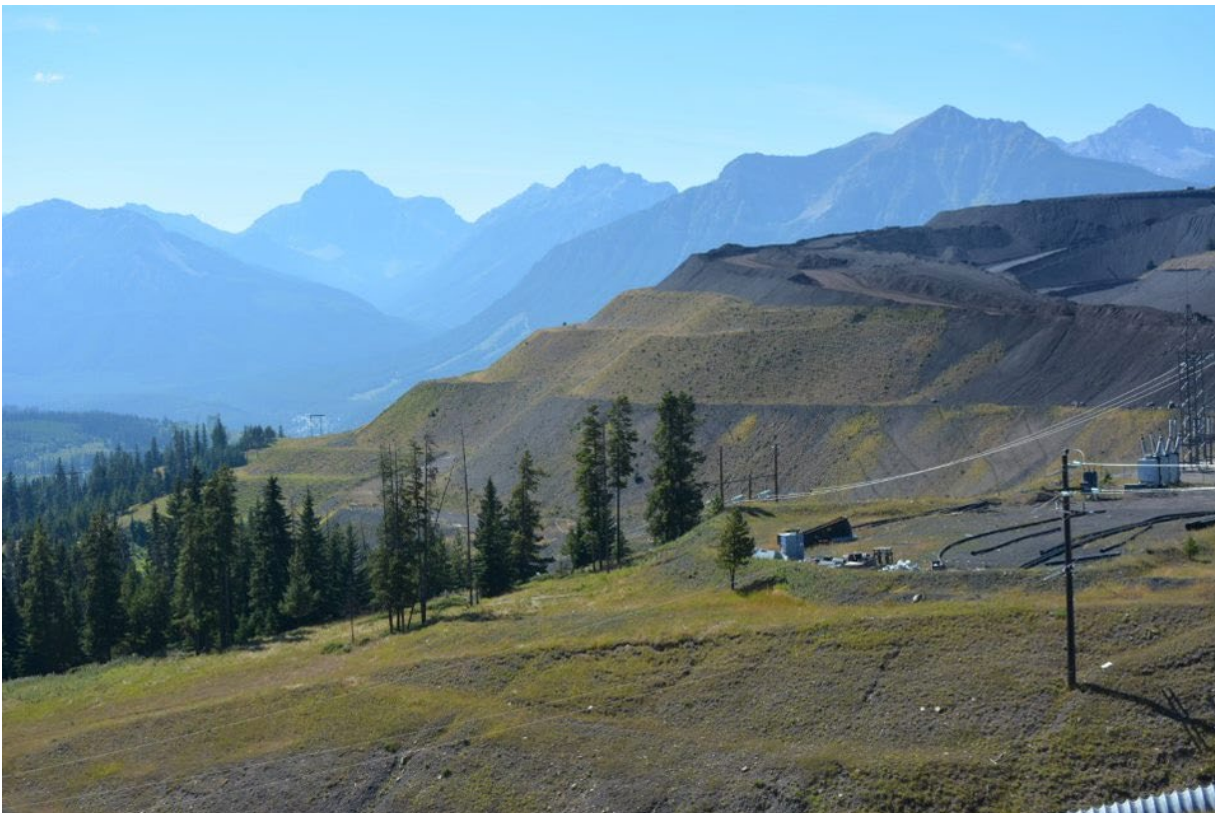
Photograph 26: Site C CCR Facility – Downstream Slope, Looking Southwest, 30 August 2022
