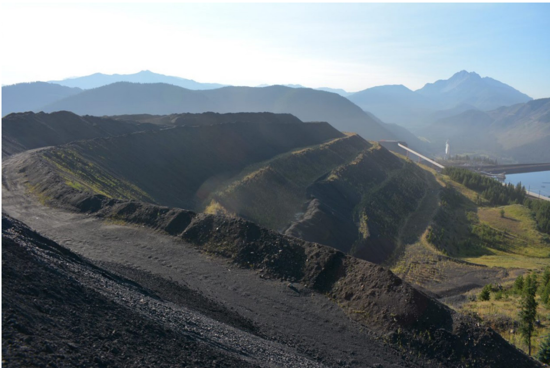
Photograph 18: Site B CCR Facility – West Downstream Slope, Looking Southeast, 31 August 2022
