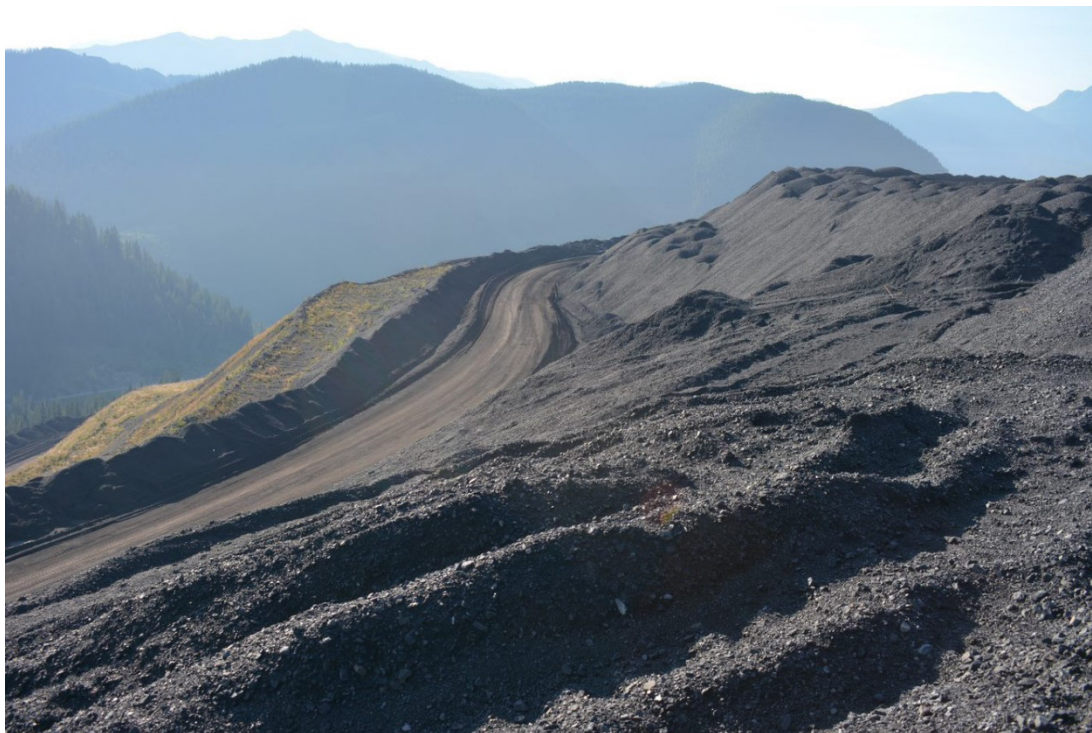
Photograph 13: Site B CCR Facility – Haul Road, Looking South, 31 August 2022
