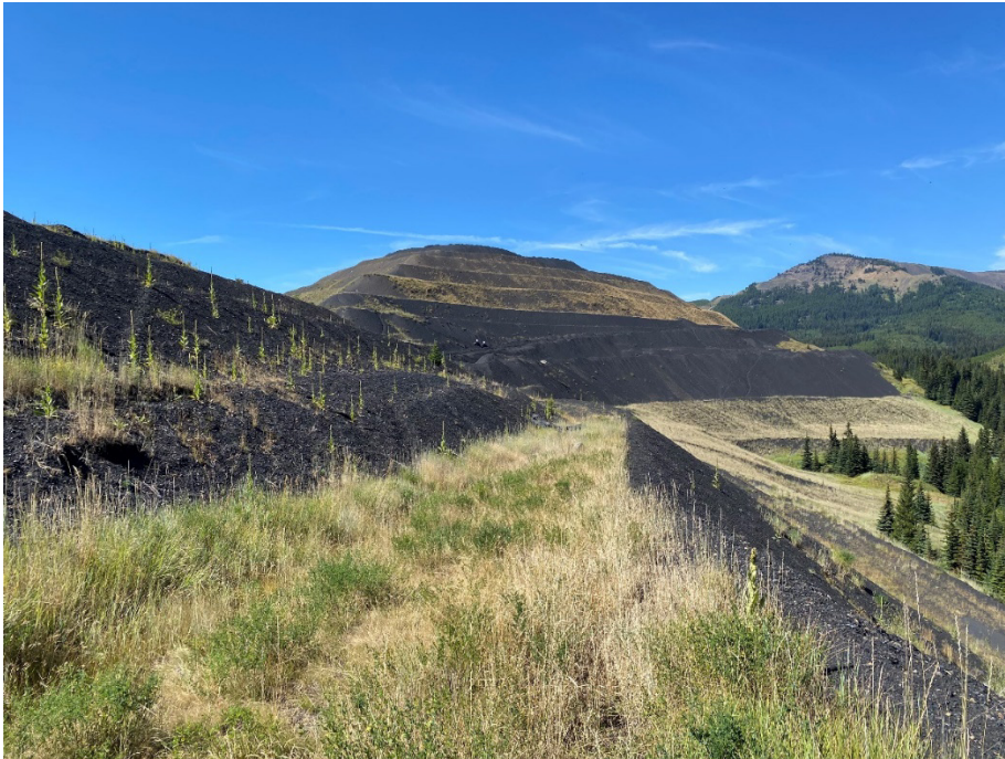
Photograph 5: Site A CCR Facility – East Slope; Looking Northwest (Site B CCR Facility in background), 30 August 2022
