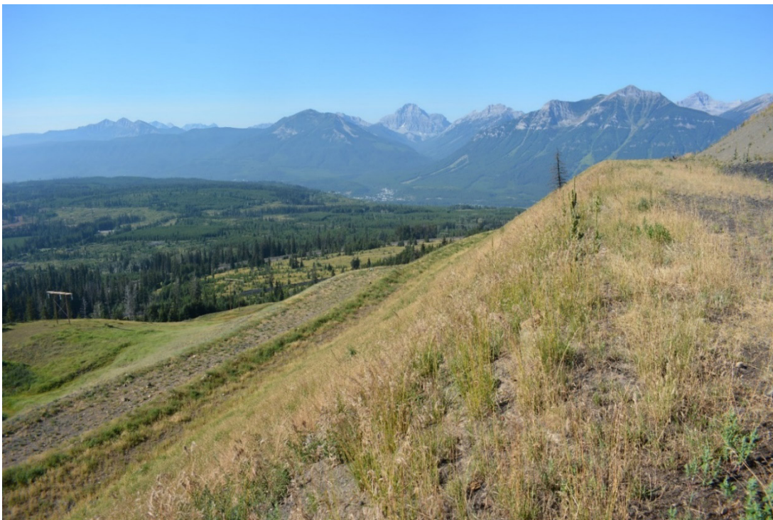
Photograph 21: Site E CCR Facility – Downstream Slope, Looking Southwest, 31 August 2022
