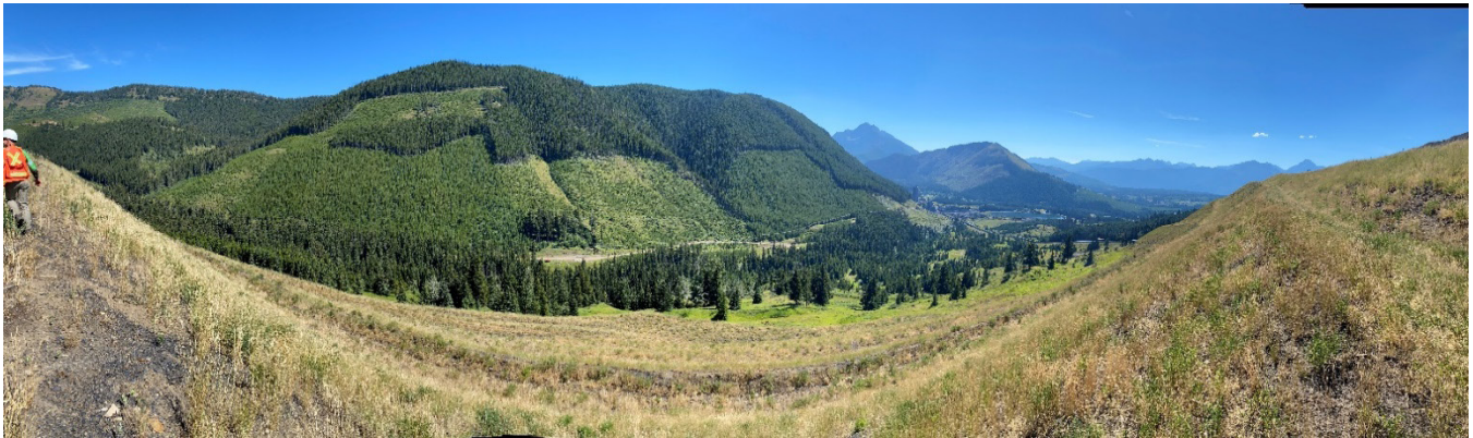
Photograph 4: Site A CCR Facility – Downstream Slope Near Relict Landslide; Looking South, 30 August 2022
