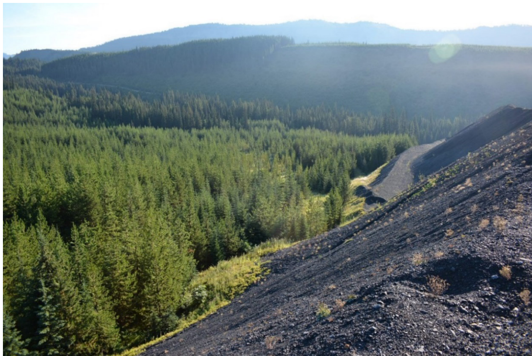
Photograph 15: Site B CCR Facility – North and East Extension Toe Area, Looking East, 31 August 2022
