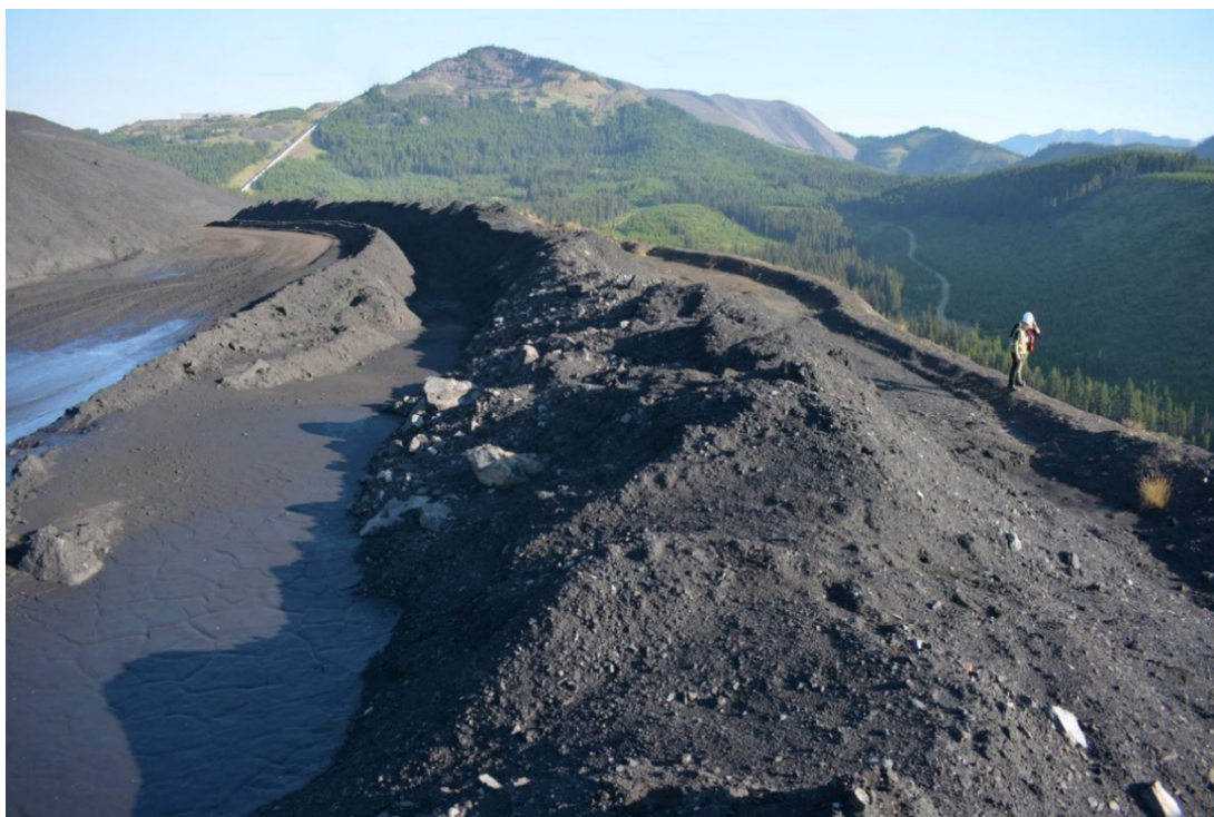
Photograph 10: Site B CCR Facility – Repaired Erosion Area on east side of haul road, Looking North, 31 August 2022
