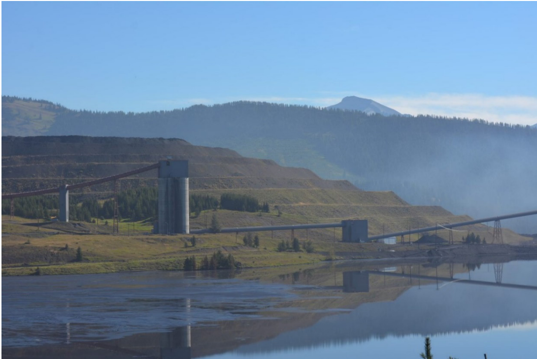
Photograph 7: Site B CCR Facility – Overview from Main Tailings Dam; Looking Northeast, 31 August 2022
