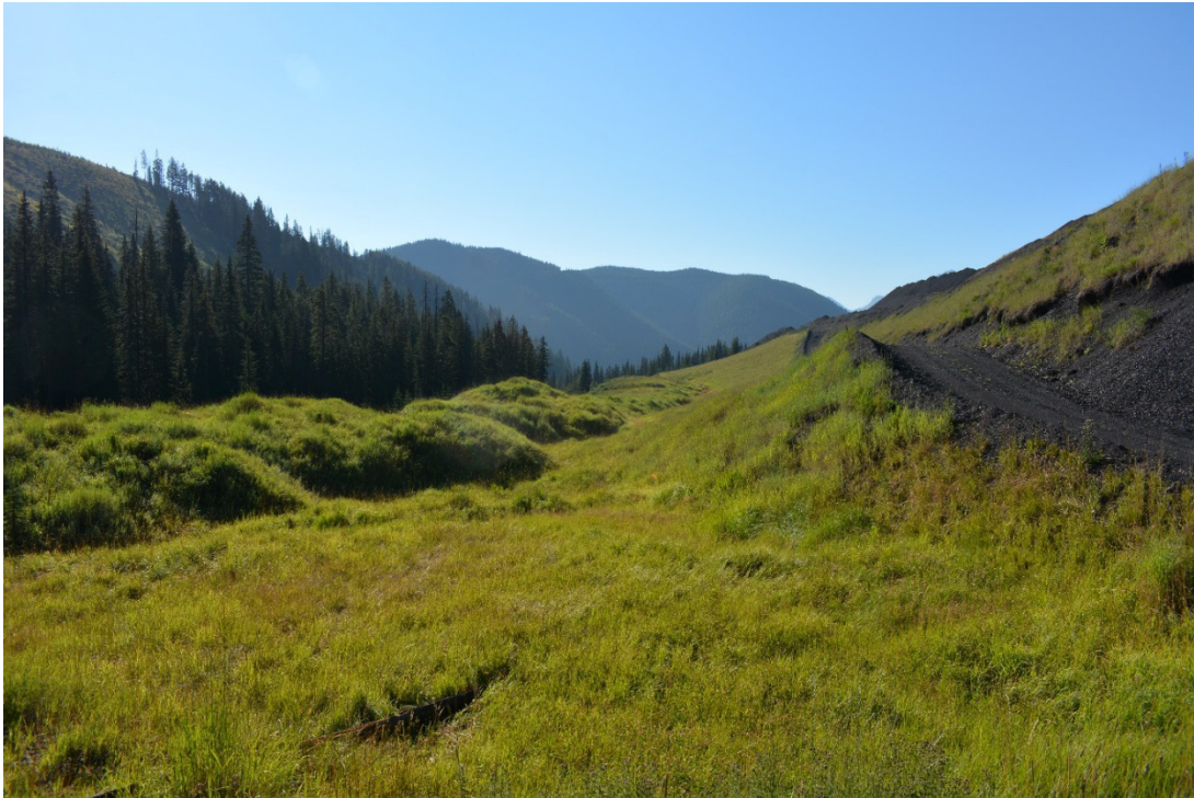
Photograph 17: Site B CCR Facility East Toe Area, Looking East, 31 August 2022
