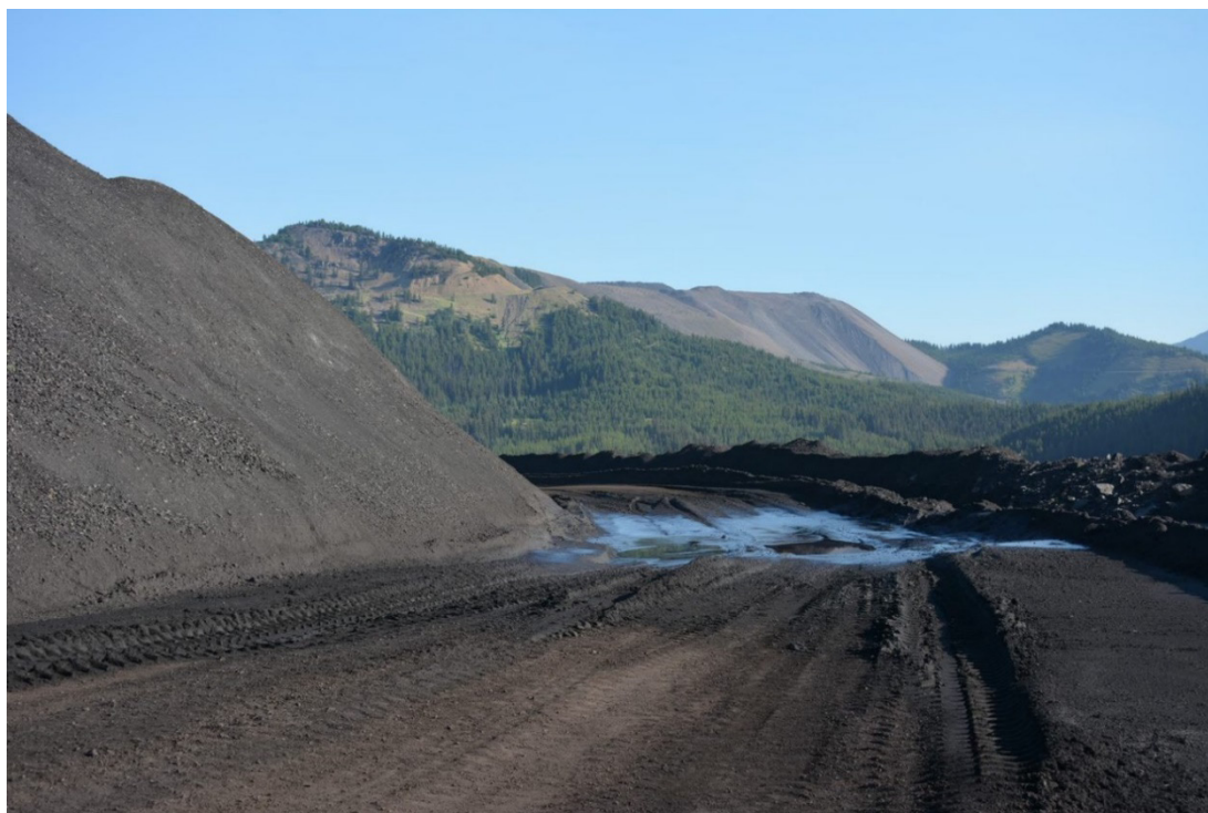
Photograph 12: Site B CCR Facility – Low Spot in haul road, Looking Northeast, 31 August 2022
