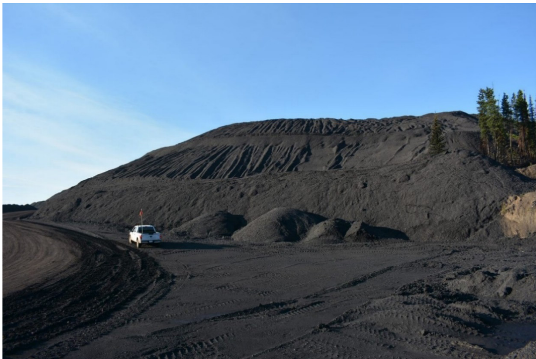
Photograph 9: Site B CCR Facility – Reprofiled Slope at Haul Road Switchback, Looking West, 31 August 2022
