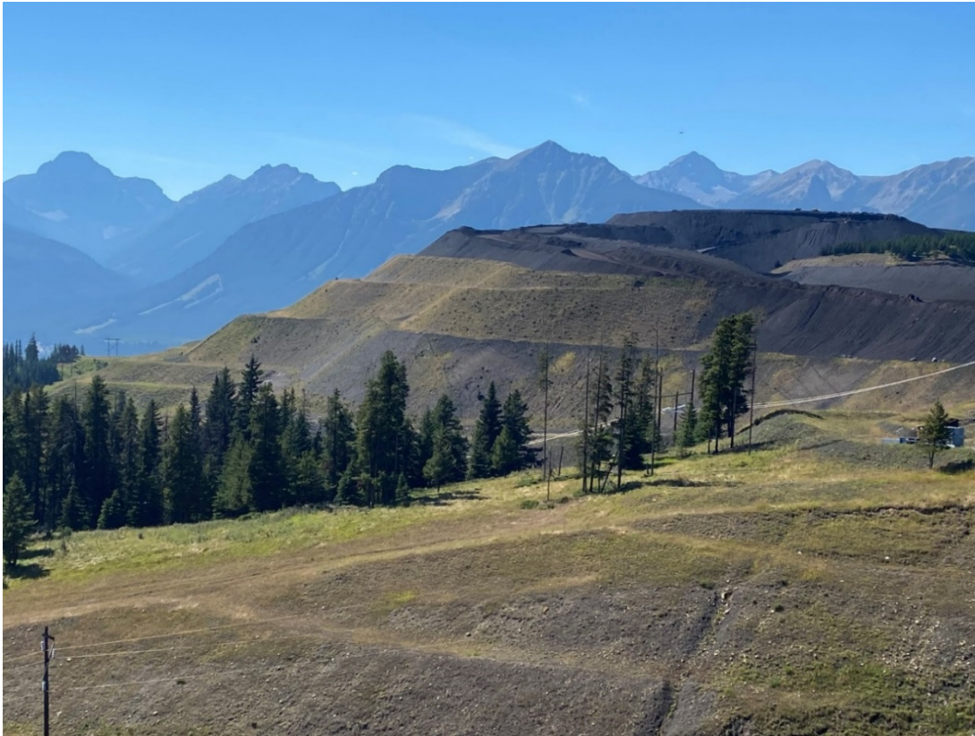
Photograph 19: Site E CCR Facility – Overview from Site A CCR Facility; Looking West, 30 August 2022
