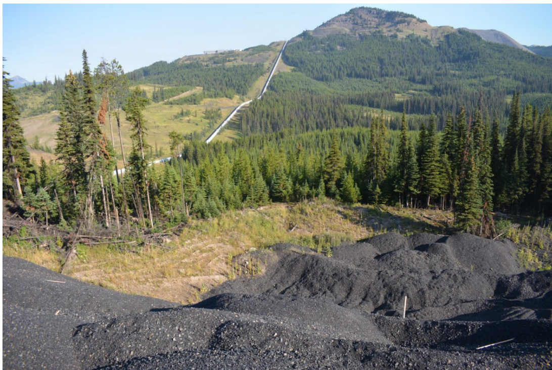
Photograph 14: Site B CCR Facility North Extension Abutment Area, Looking North, 31 August 2022
