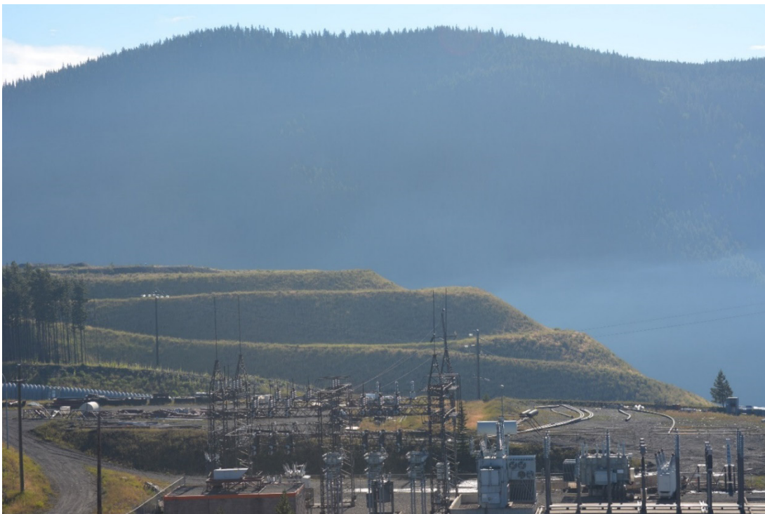
Photograph 2: Site A CCR Facility – Overview from Site C CCR Facility, Looking East, 30 August 2022
