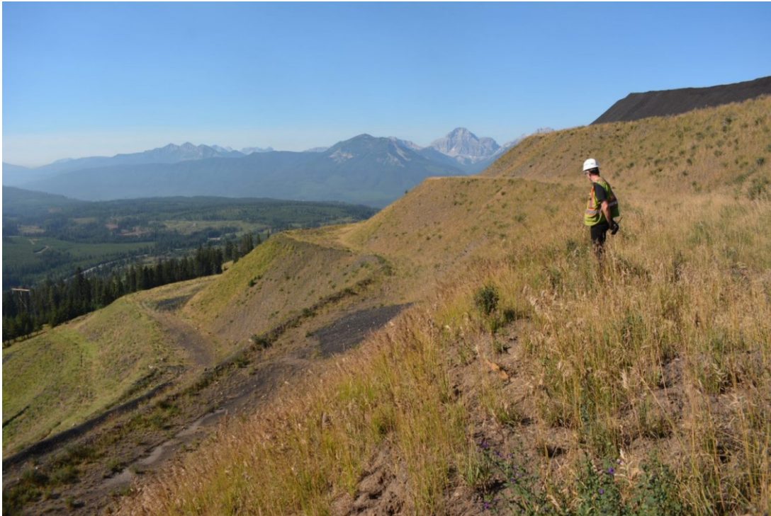
Photograph 20: Site E CCR Facility – Downstream Slopes, Looking West, 31 August 2022
