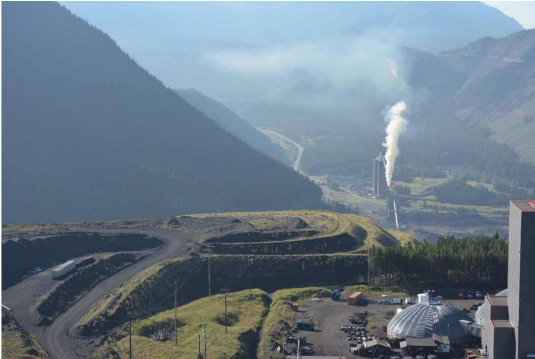
Photograph 3: Site A CCR Facility – Overview from Site B; Looking Southeast, 30 August 2022
