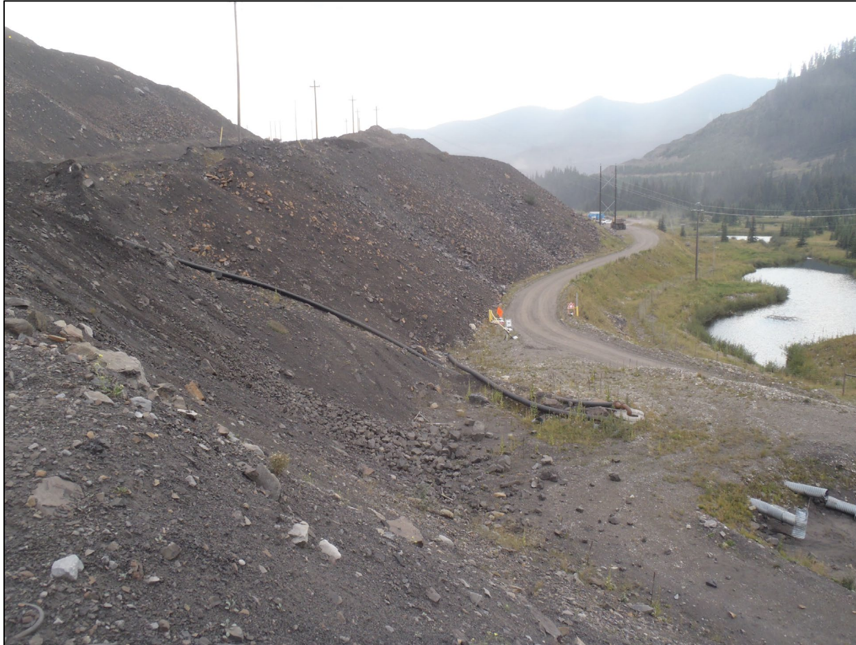
Turnbull TSF: View of the downstream slope and toe of the low point area waste rockfill, looking southwest.
