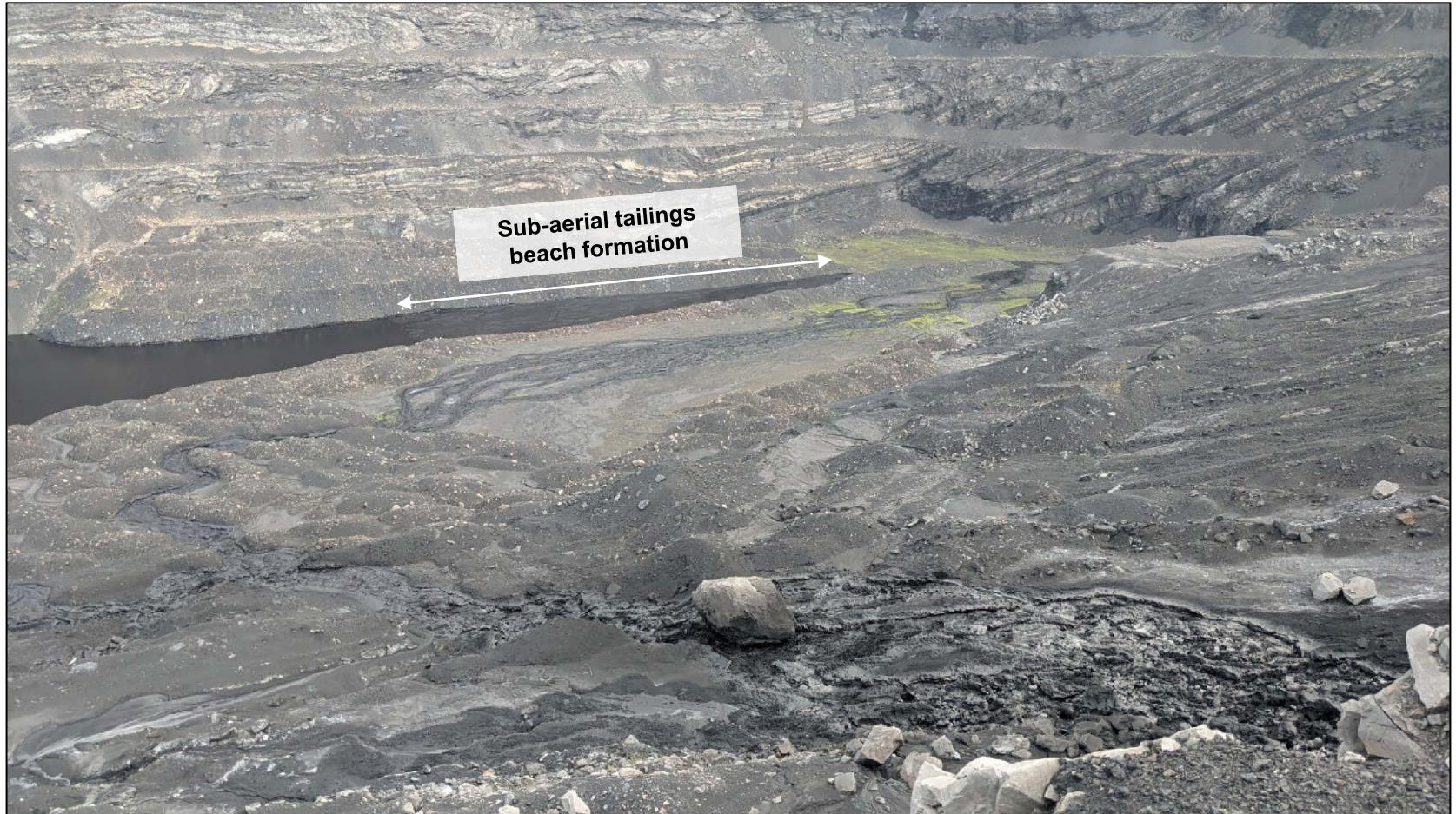
Tailings deposition and in-pit spoils below the tailings pipeline end of the pipe outlet, looking east.
