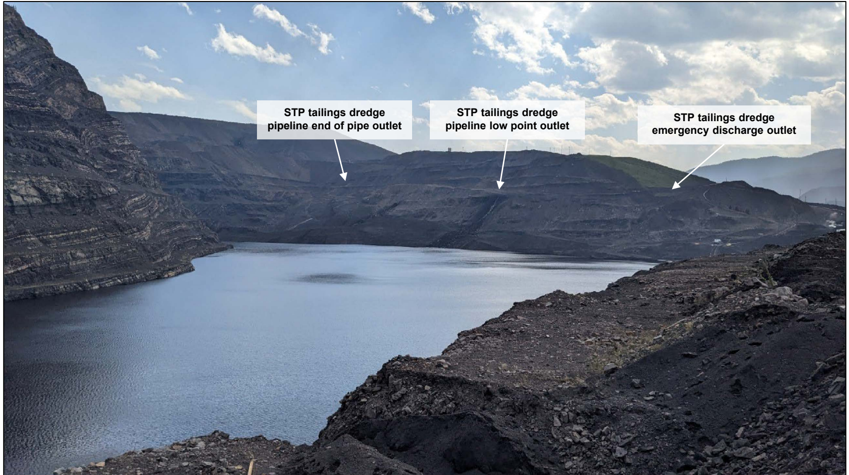
Turnbull TSF: Overview from north endwall, looking south.
