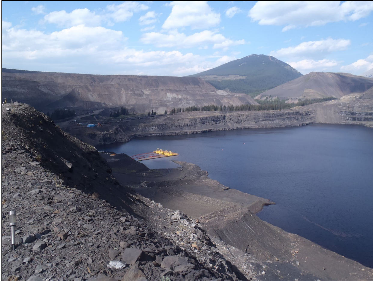
Turnbull TSF pond, reclaim water intakes, and pipelines, looking north.
