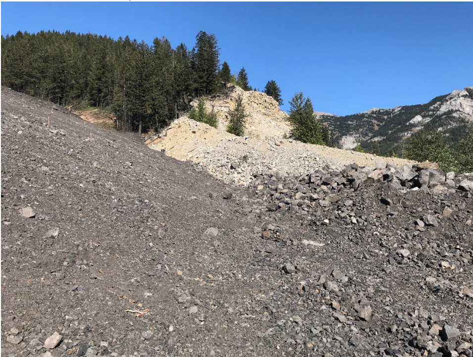
Photo IW-12 WFTF downstream slope at east abutment. (Looking South – Taken 21 September 2022)
