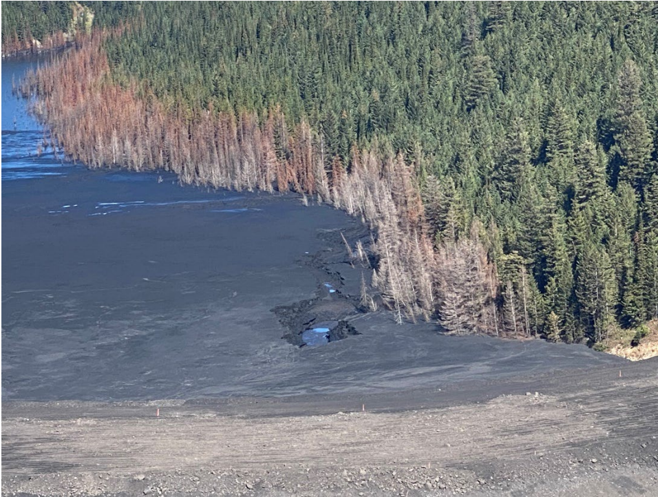
Photo IW-17 WFTF receding incised channel. (Looking north, from Sunshine Dump crest – Taken 21 September 2022)
