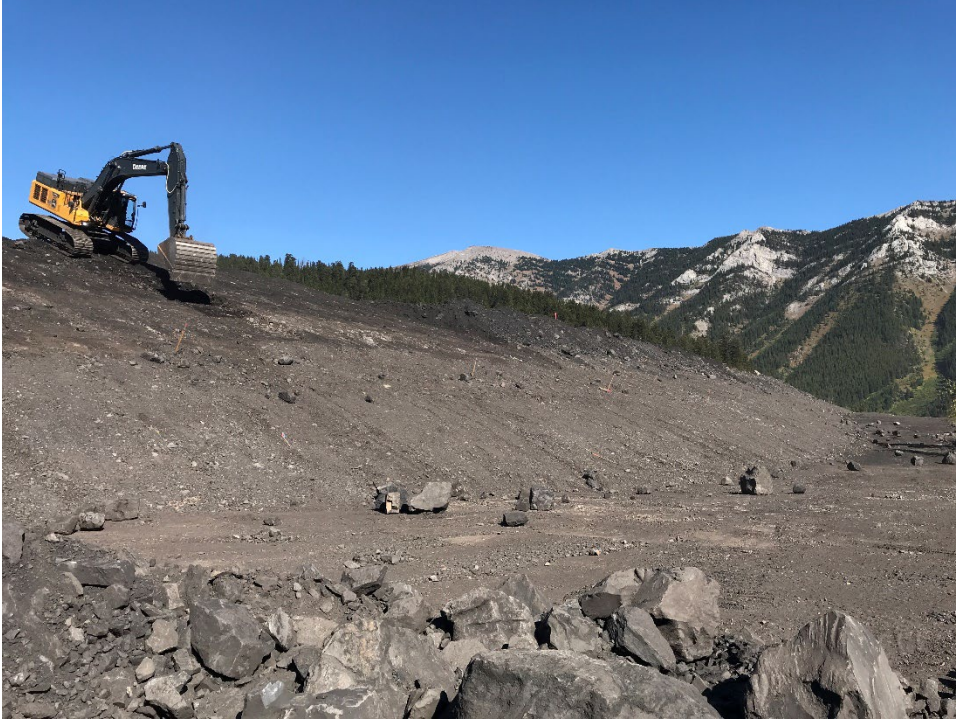
Photo IW-15 WFTF typical downstream slope. (Looking NE – Taken 21 September 2022)
