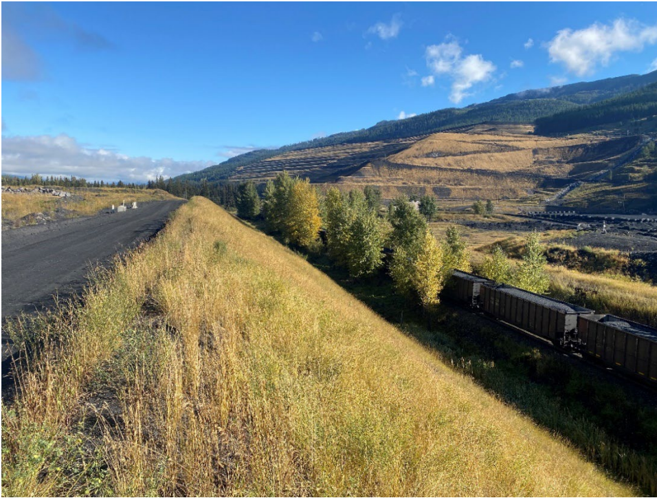
Photo IC-3 Lagoon C crest and embankment typical conditions. (Looking north – Taken 20 September 2022)
