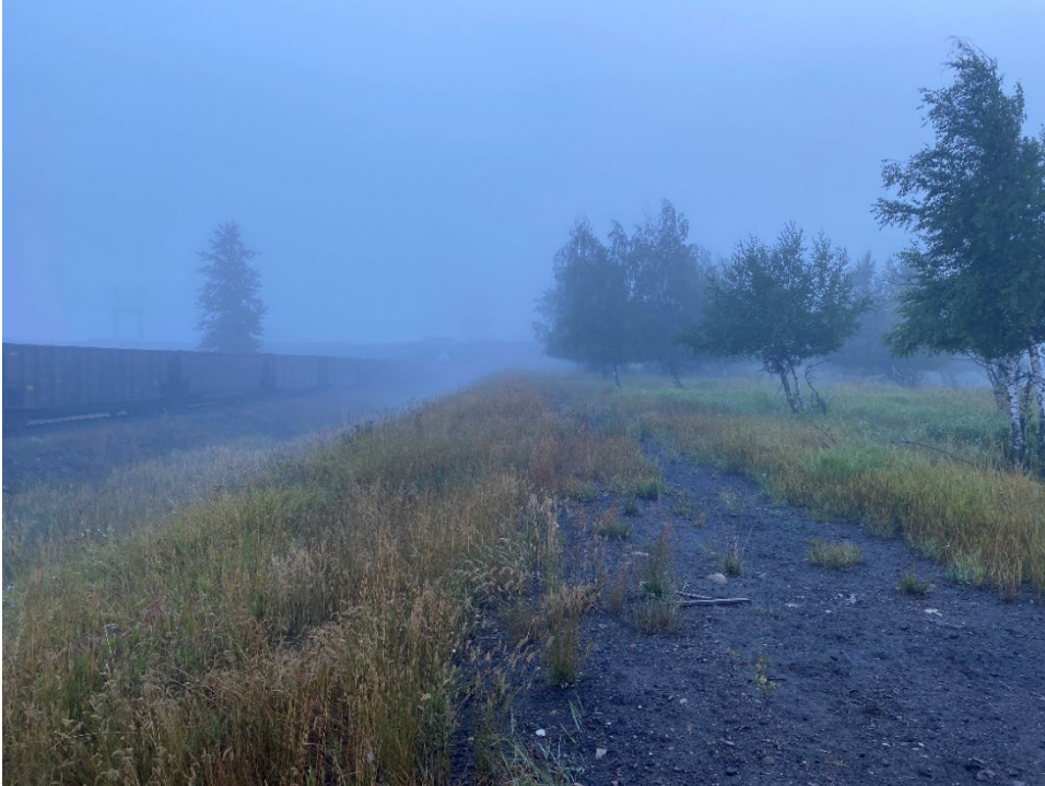
Photo IA-5 Lagoon A crest typical conditions. (Looking NE – Taken 20 September 2022)
