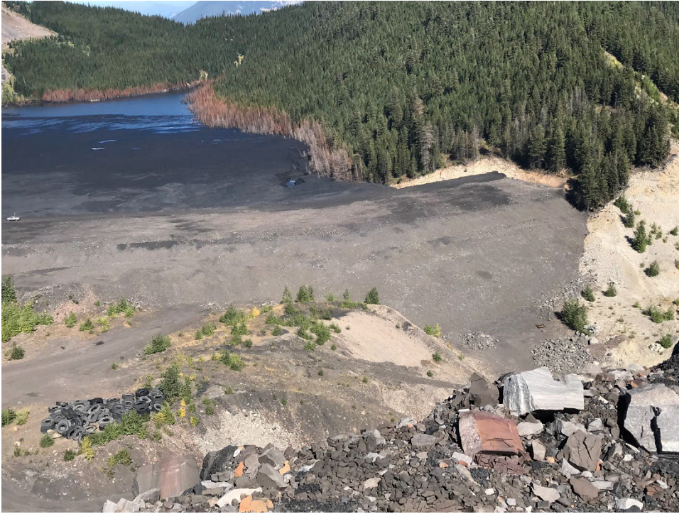
Photo IW-3 WFTF south embankment and east abutment overview. (Looking NE, from Sunshine Dump crest – Taken 21 September 2022)
