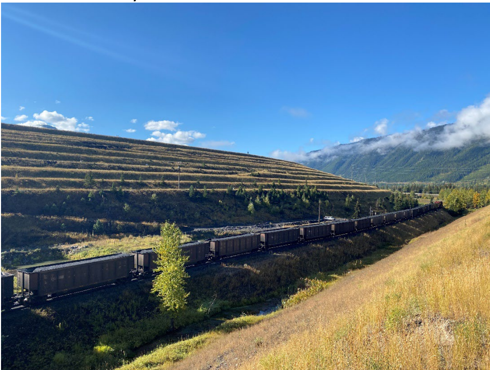
Photo ID-2 Lagoon D embankment. (Looking SW, from Lagoon C crest – Taken 20 September 2022)
