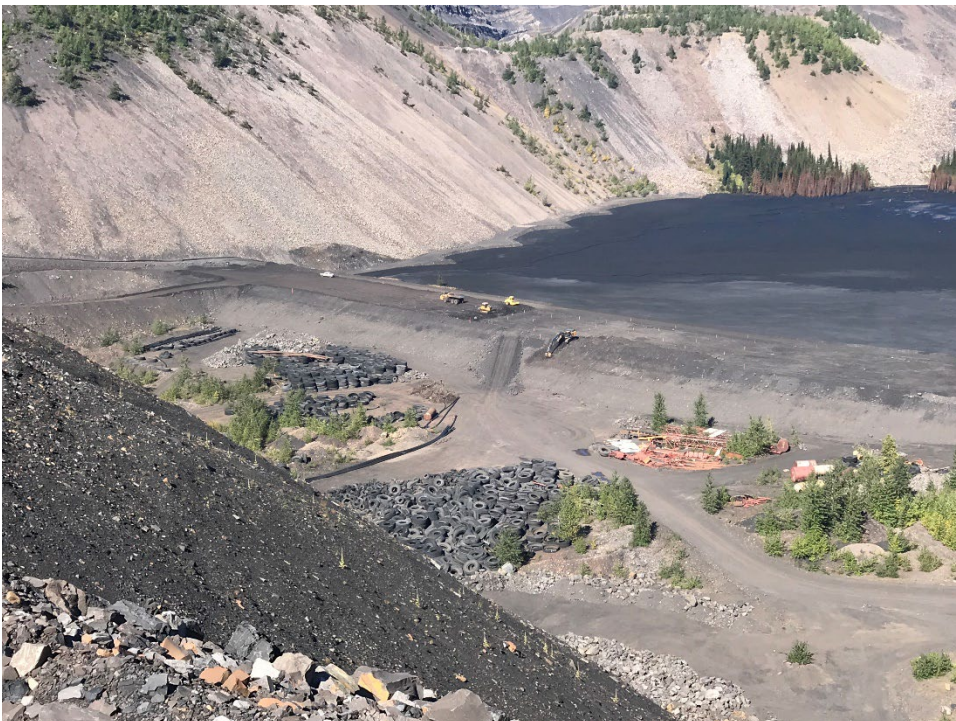
Photo IW-2 WFTF south embankment and west abutment overview. Adit Filter Berm (AFB) in background. (Looking NW, from Sunshine Dump crest – Taken 21 September 2022)
