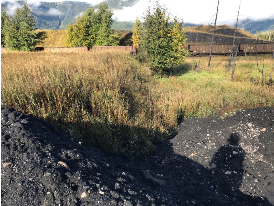
Photo IB-6 Lagoon B crest and embankment. (Looking west – Taken 20 September 2022)
