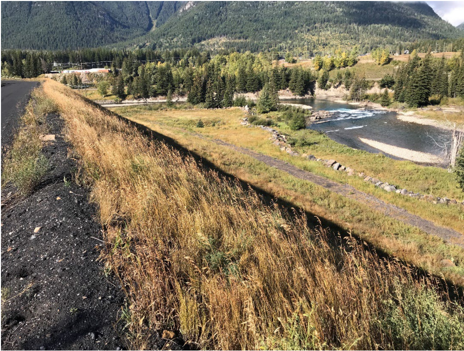
Photo IC-7 Lagoon C downstream slope and toe riprap. (Looking west – Taken 20 September 2022)
