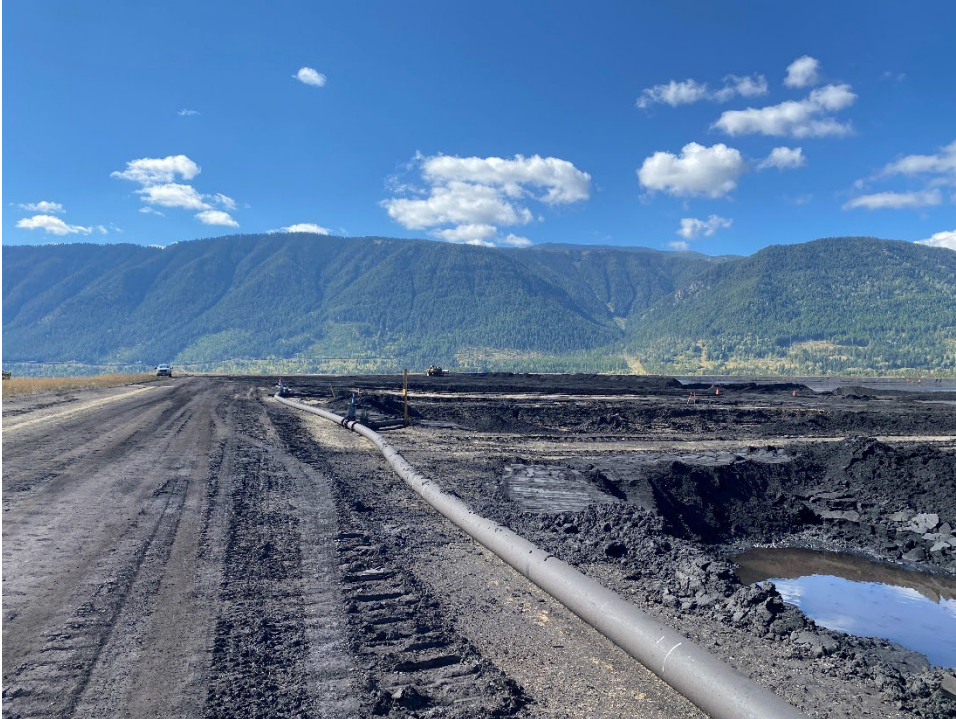
Photo ID-20 Lagoon D south tailings cells. (Looking west – Taken 20 September 2022)
