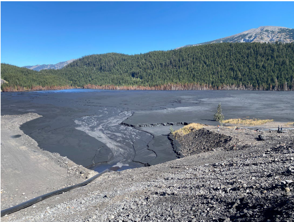
Photo IW-4 WFTF tailings beach, spigot, and WFTF embankment-AFB tie-in. (Looking NE – Taken 21 September 2022)
