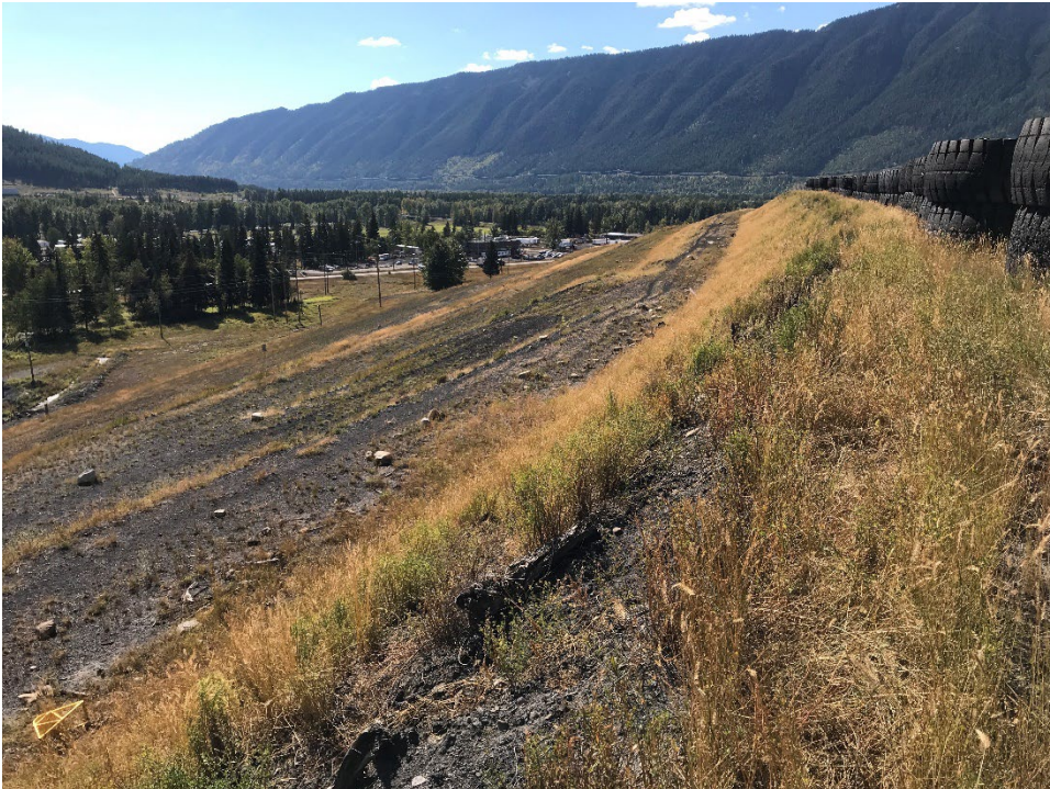
Photo ID-14 Lagoon D crest and embankment slope. (Looking SW – Taken 20 September 2022)
