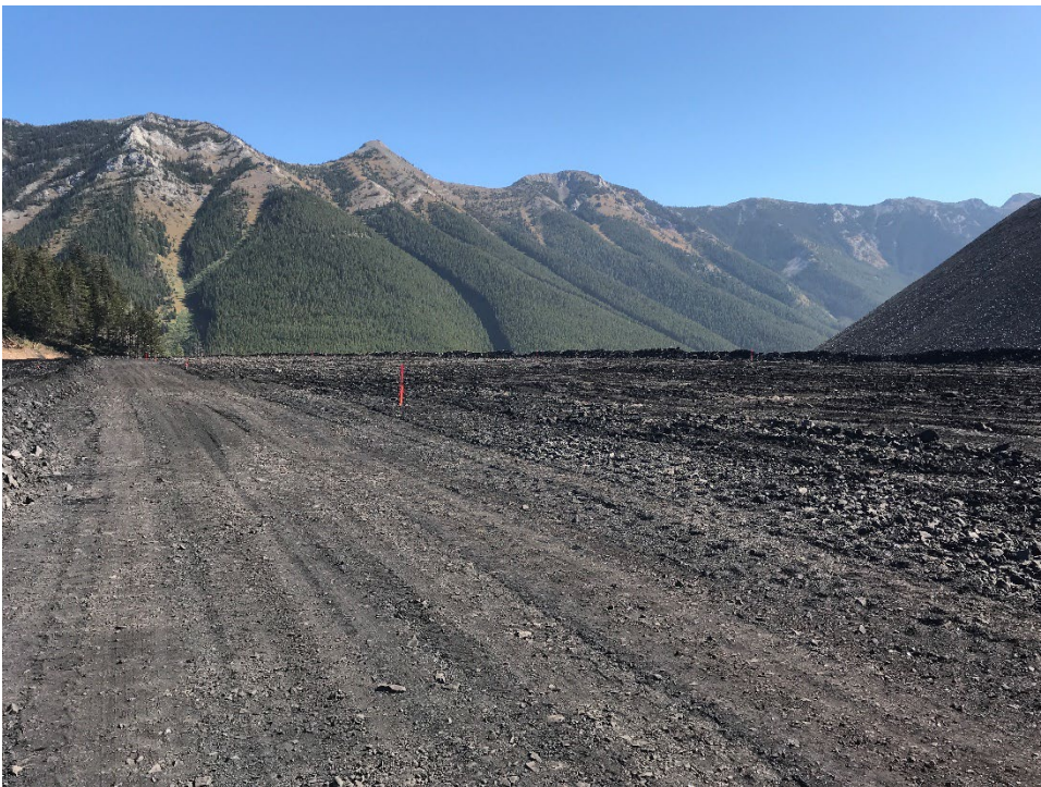
Photo IW-10 WFTF crest typical condition. (Looking SE – Taken 21 September 2022)
