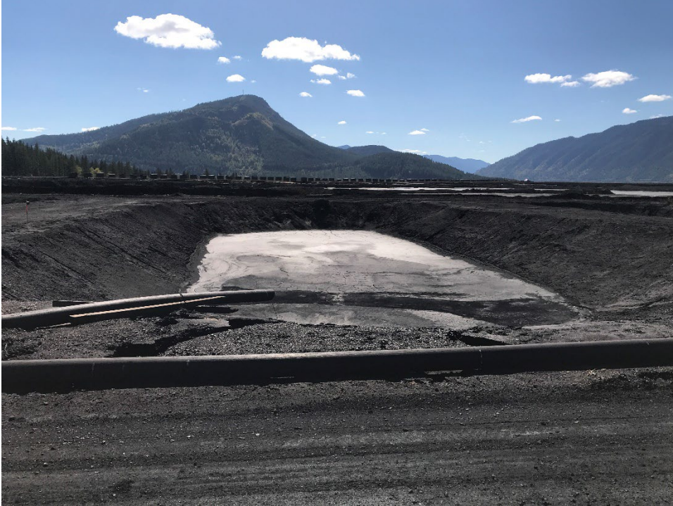
Photo ID-19 Lagoon D north tailings cells. (Looking south – Taken 20 September 2022)
