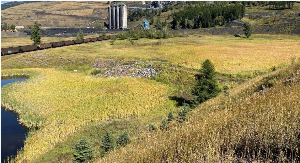
Photo IA-1 Lagoon A general conditions and overview. (From Lagoon D, looking NE – Taken 20 September 2022)
