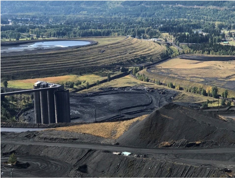
Photo IB-1 Lagoon B overview. (Looking SE, from Coarse Coal Refuse (CCR) Dump crest – Taken 20 September 2021)
