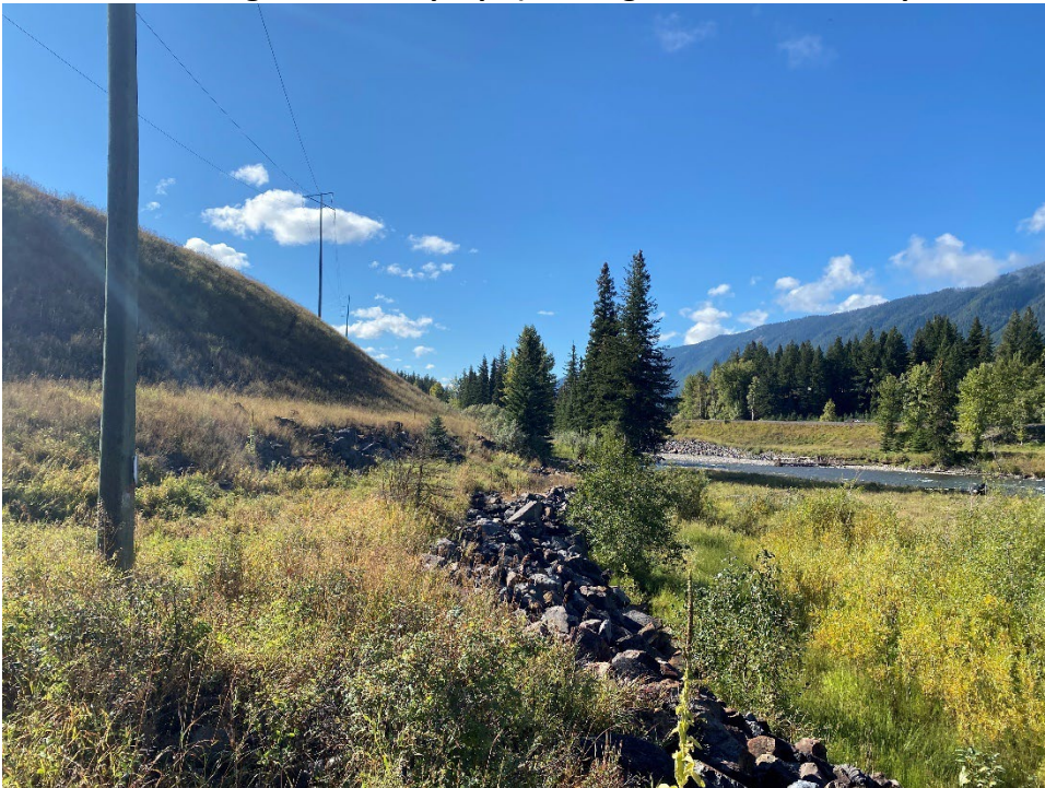
Photo IC-8 Lagoon C toe riprap. (Looking SW – Taken 20 September 2022)
