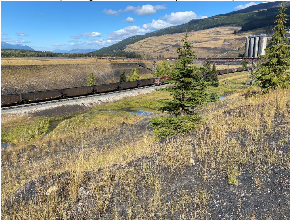
Photo ID-6 Lagoon D ponding at the embankment toe (Otto Creek) adjacent to the rail line. (Looking north – Taken 20 September 2022)
