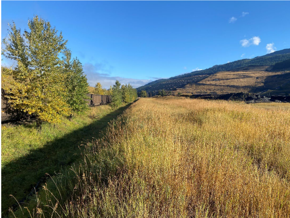
Photo IB-4 Lagoon B crest typical condition. (Looking north – Taken 20 September 2022)
