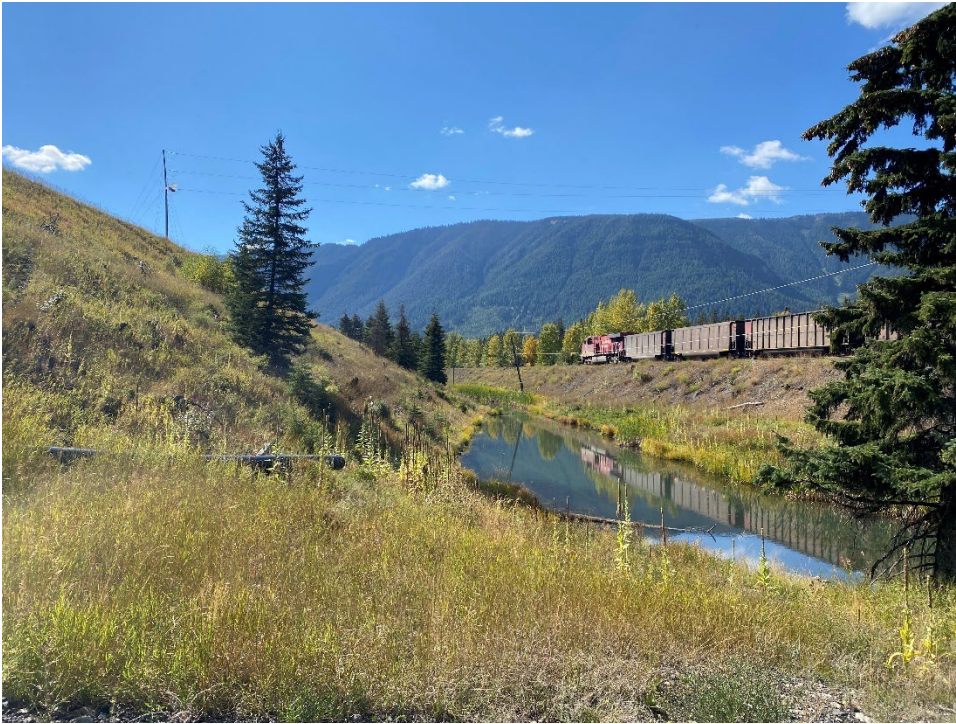
Photo ID-5 Lagoon D ponding at the embankment toe (Otto Ponds) adjacent to the rail line. (Looking SW – Taken 20 September 2022)
