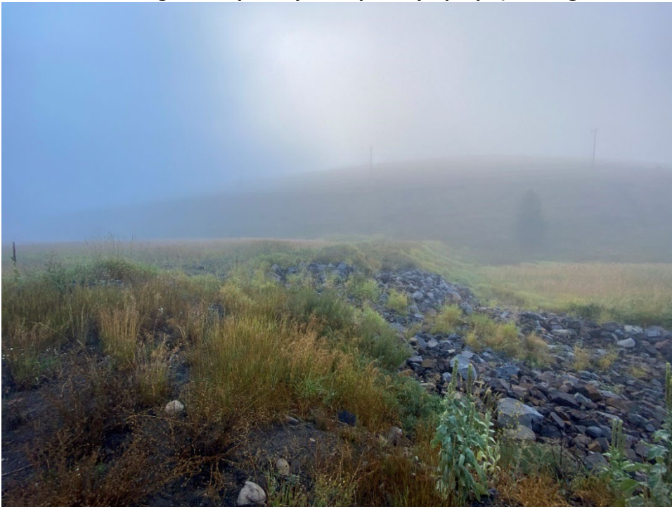
Photo IA-4 Lagoon A spillway and spillway riprap. (Looking south – Taken 20 September 2022)
