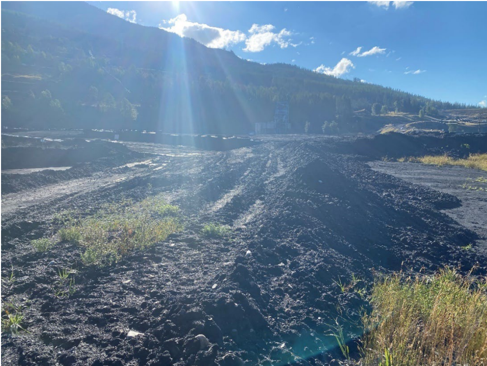
Photo IB-8 Lagoon B embankment resloping. (Looking SE – Taken 20 September 2022)
