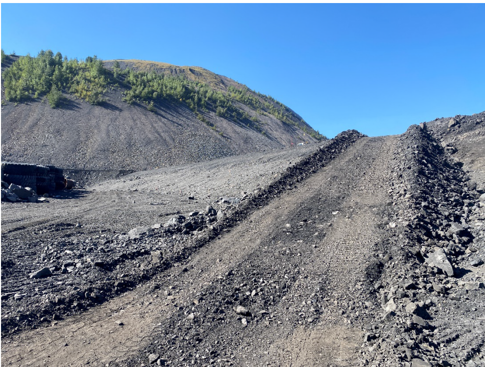
Photo IW-16 WFTF typical downstream slope. (Looking NW – Taken 21 September 2022)
