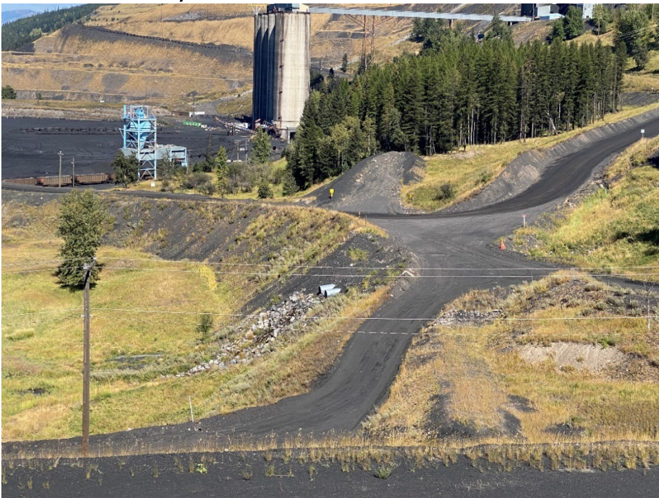
Photo IA-6 Cossarini Creek culvert outlets. (From Lagoon D, looking north – Taken 20 September 2022)
