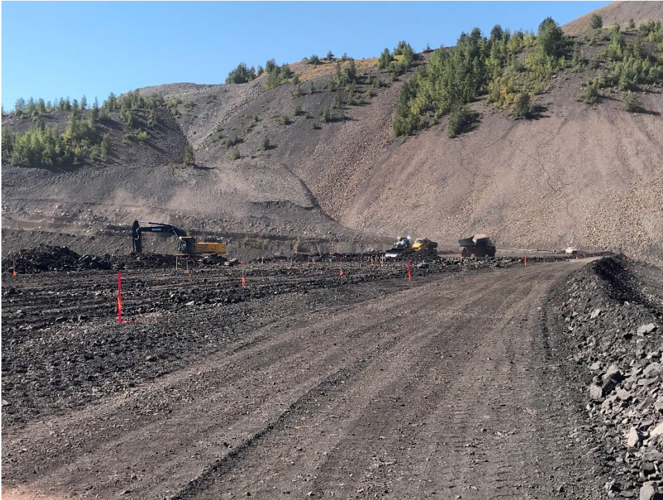
Photo IW-9 WFTF construction raise progress. (Looking west – Taken 21 September 2022)
