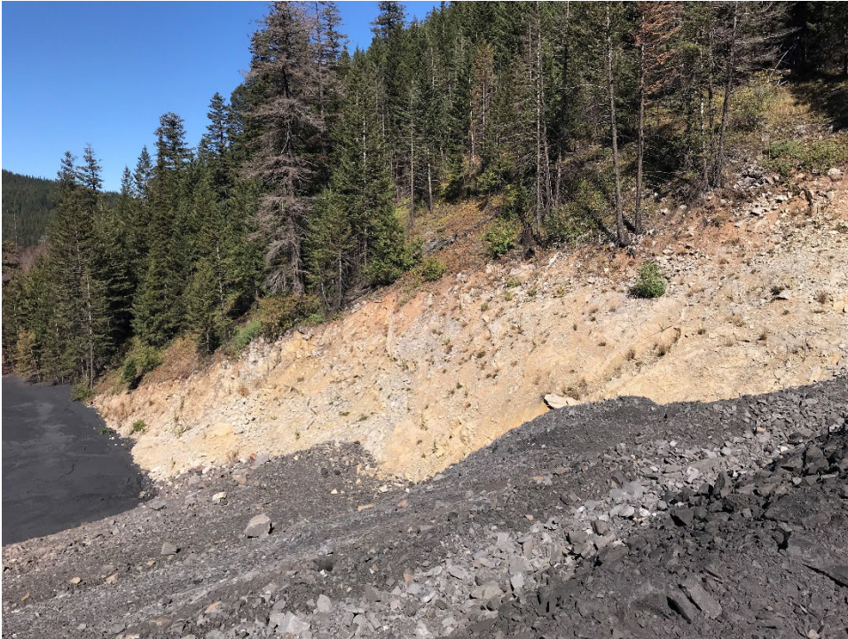
Photo IW-11 WFTF upstream slope at east abutment. (Looking west – Taken 21 September 2022)
