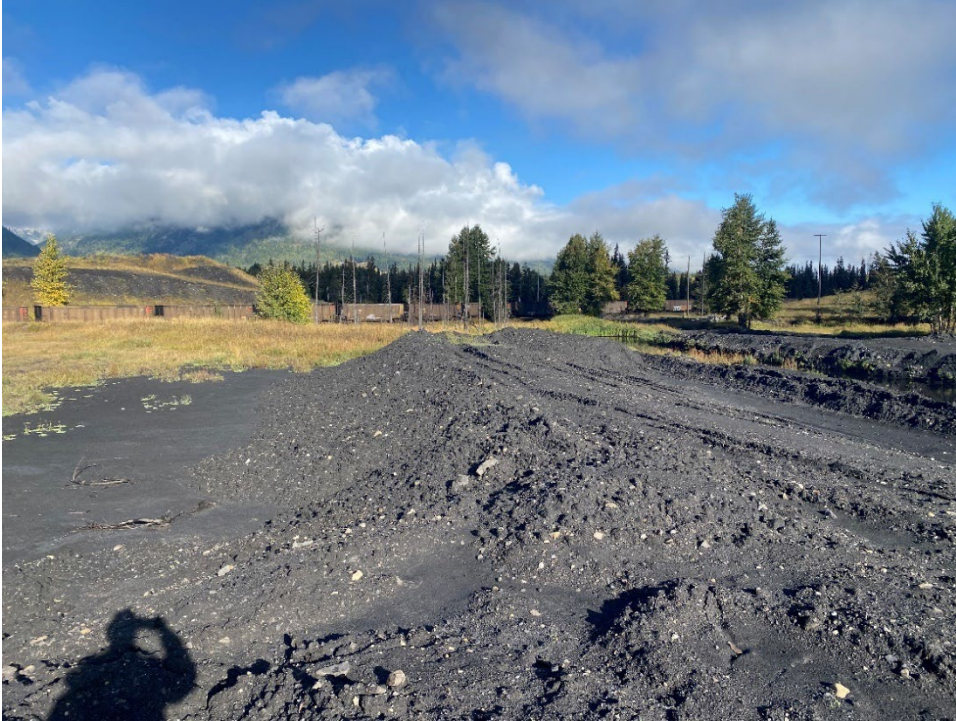
Photo IB-7 Lagoon B embankment resloping. (Looking NW – Taken 20 September 2022)
