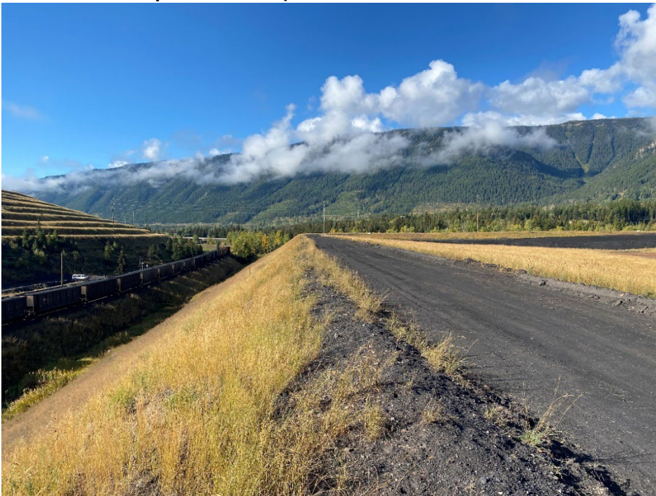
Photo IC-4 Lagoon C crest and embankment typical conditions. (Looking SW – Taken 20 September 2022)
