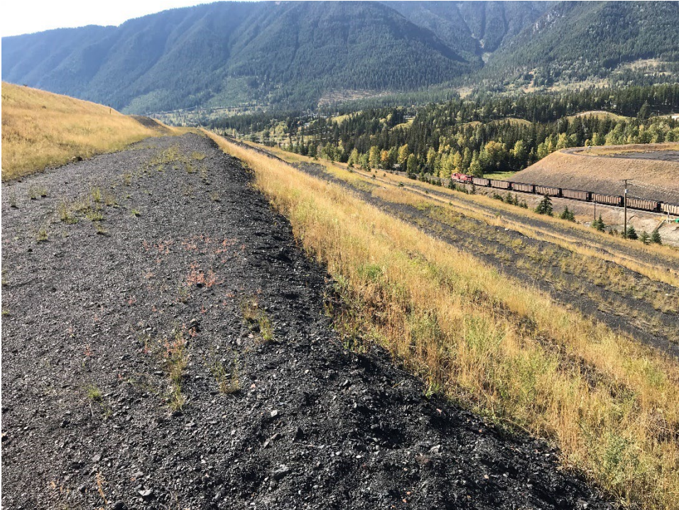
Photo ID-8 Lagoon D bench typical conditions. (Looking west – Taken 20 September 2022)
