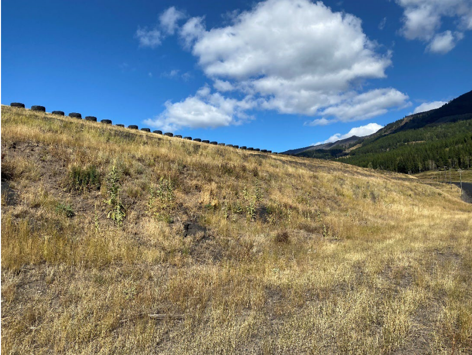
Photo ID-13 Lagoon D embankment. (Looking NE – Taken 20 September 2022)
