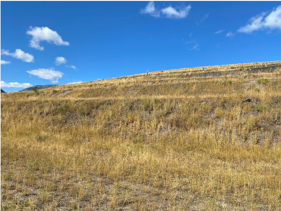
Photo ID-12 Lagoon D embankment. (Looking north – Taken 20 September 2022)
