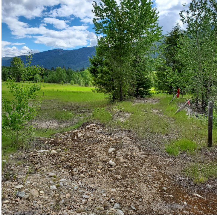
Photo 9: South TSF –Cell 5 Crest and Tailings, Looking North from Cell 1. Jun 22, 2022
