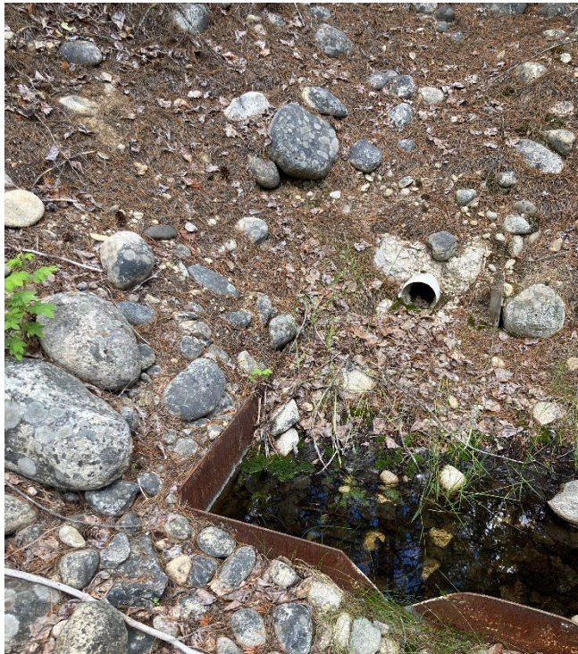
Photo 24: North TSF –Cell 6 Decant Outlet. Jun 22, 2022
