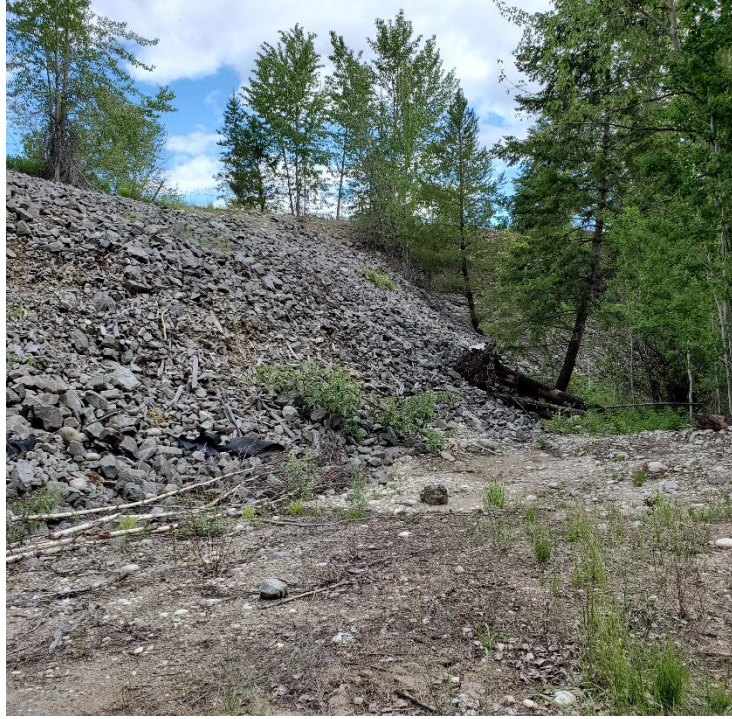
Photo 3: South TSF –Cell 5 South Side Downstream Slope with Rockfill, Looking Northeast. Jun 22, 2022
