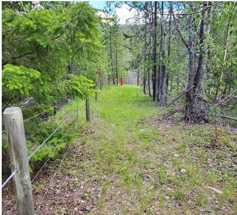
Photo 28: North TSF –Cell 7 North Embankment Crest, Looking East. Jun 22, 2022
