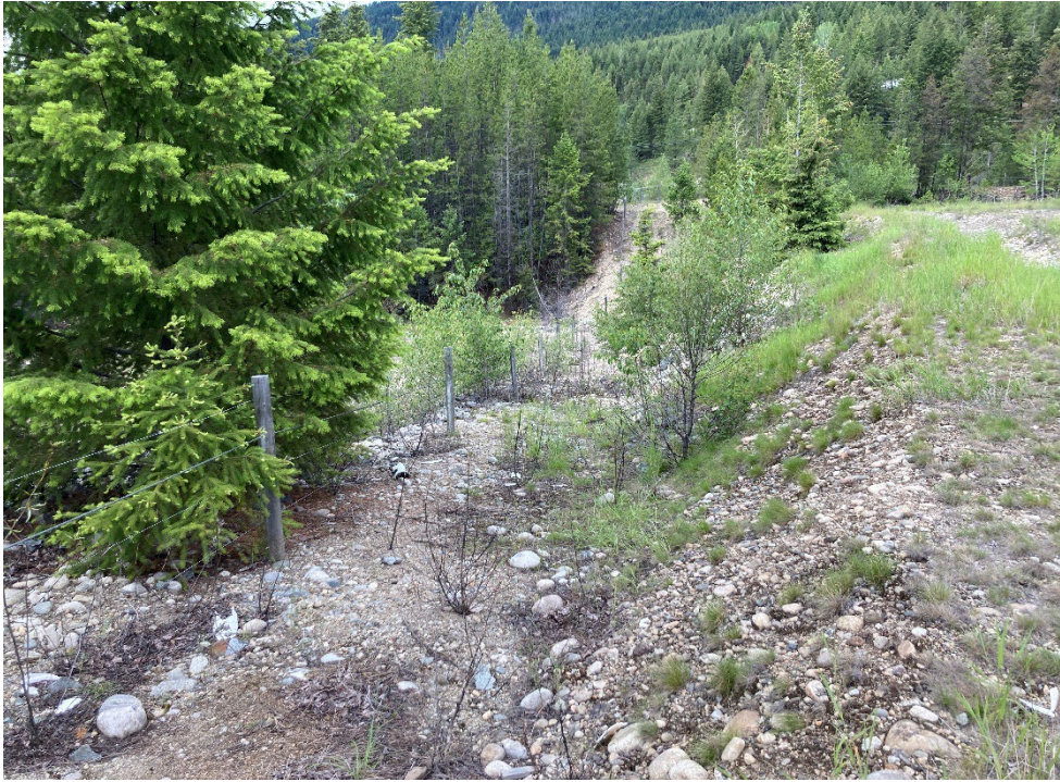
Photo 4: South TSF –Cell 1 Crest and Downstream Slope, Looking Southwest. Jun 22, 2022
