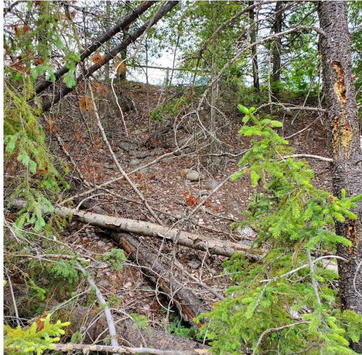
Photo 2: South TSF –Cell 5 Southeast Corner Downstream Embankment Slope, Looking Northeast. Jun 22, 2022
