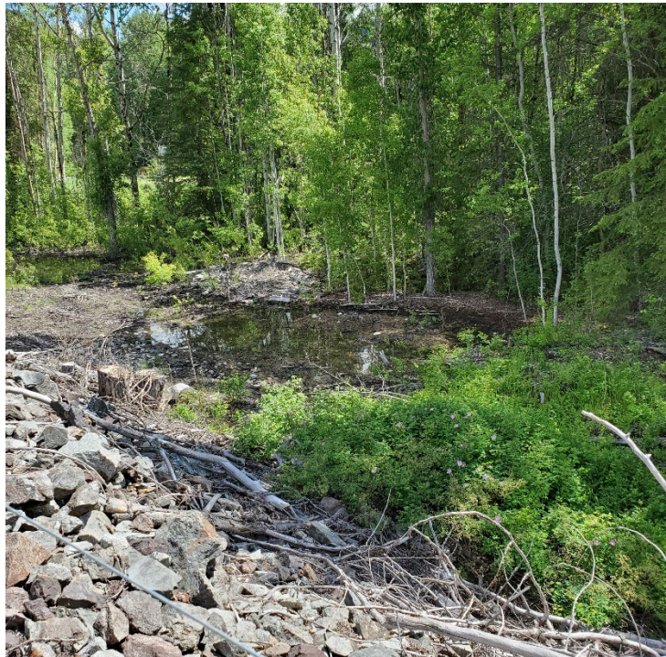
Photo 14: South TSF –Ponding at Cell 3 Downstream Toe, Looking Northeast. Jun 22, 2022
