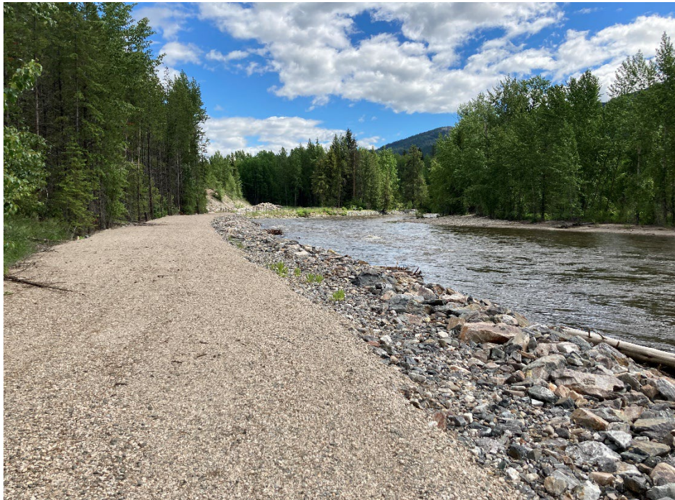
Photo 1: South TSF - Cells 4 and 5 Embankment Toe Erosion Protection Riprap, Looking North. Jun 22, 2022
