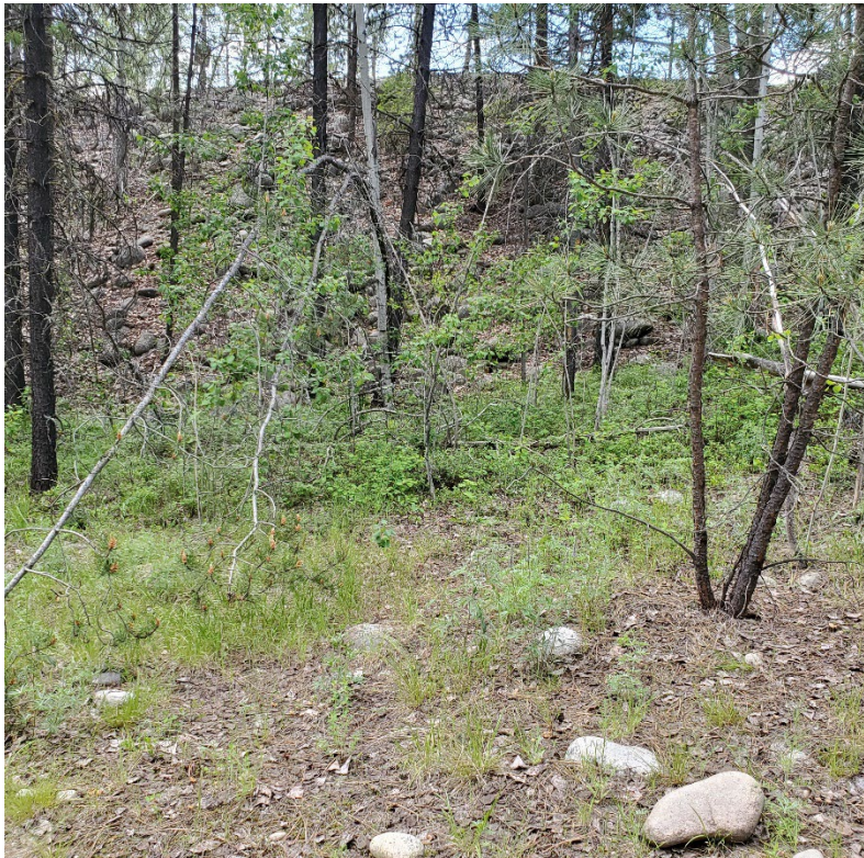
Photo 22: North TSF –Cell 6 Downstream Slope and Toe, Looking West. Jun 22, 2022
