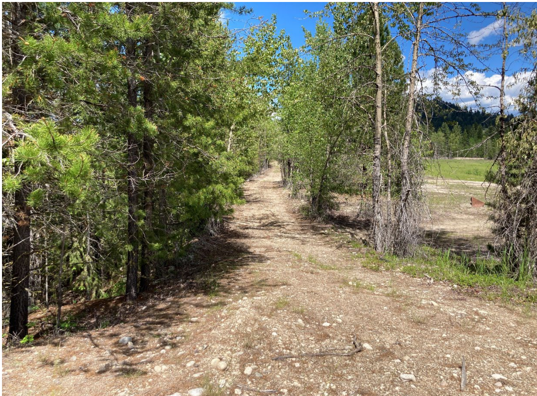
Photo 32: North TSF –Divider Dyke Between Cell 6 and Cell 7, Looking North. Jun 22, 2022
