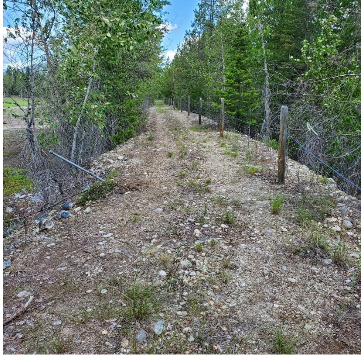
Photo 19: North TSF –Cell 6 East Embankment Crest, Looking North. Jun 22, 2022
