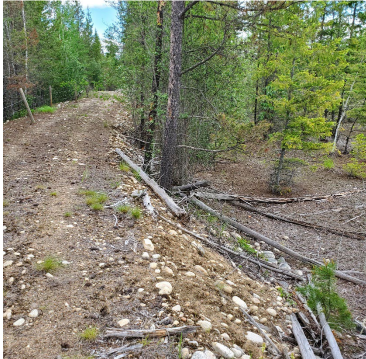
Photo 6: South TSF –Cell 1 West Embankment, Looking North. Jun 22, 2022
