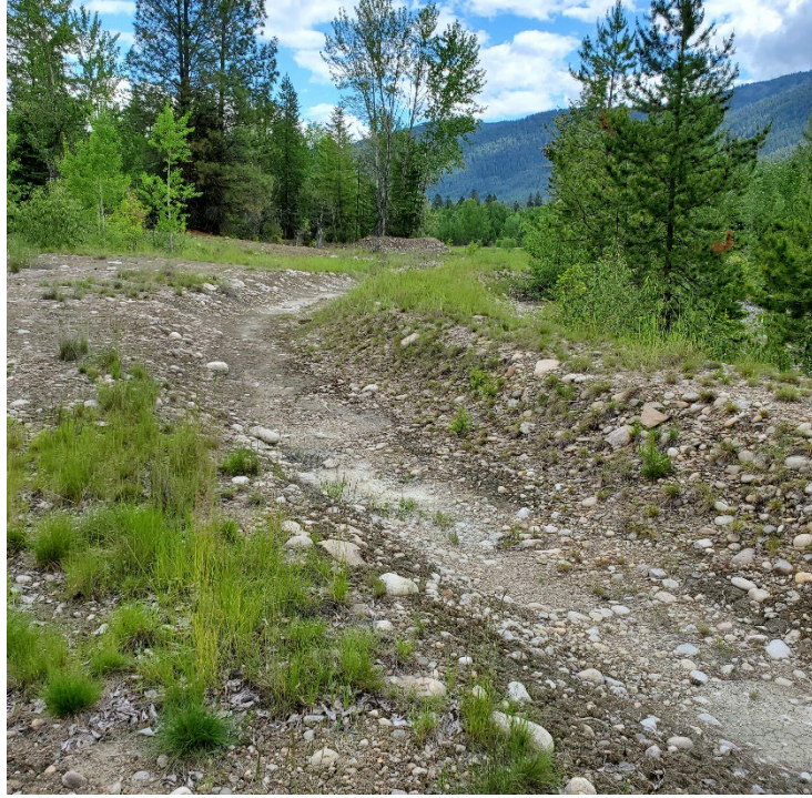
Photo 5: South TSF –Cell 1 Crest and Upstream Ditch to Cell 5, Looking Northeast. Jun 22, 2022
