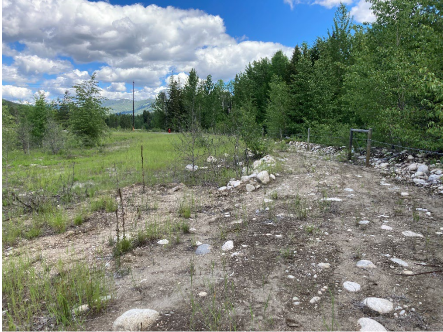
Photo 11: South TSF –Cell 4 Embankment Crest and Tailings, Looking North. Jun 22, 2022
