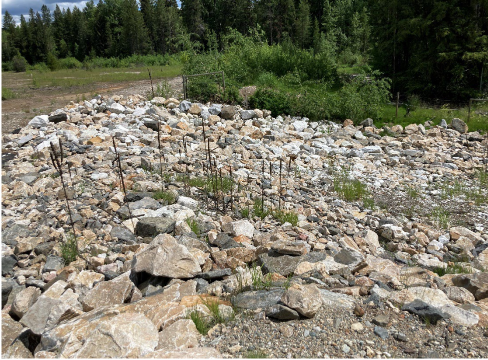
Photo 15: South TSF –Cell 3 Spillway, Looking South. Jun 22, 2022
