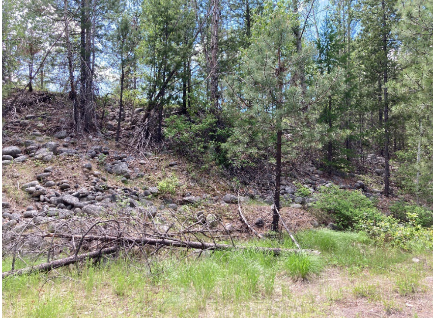
Photo 23: North TSF –Cell 6 Downstream Slope and Toe. Looking Southwest. Jun 22, 2022
