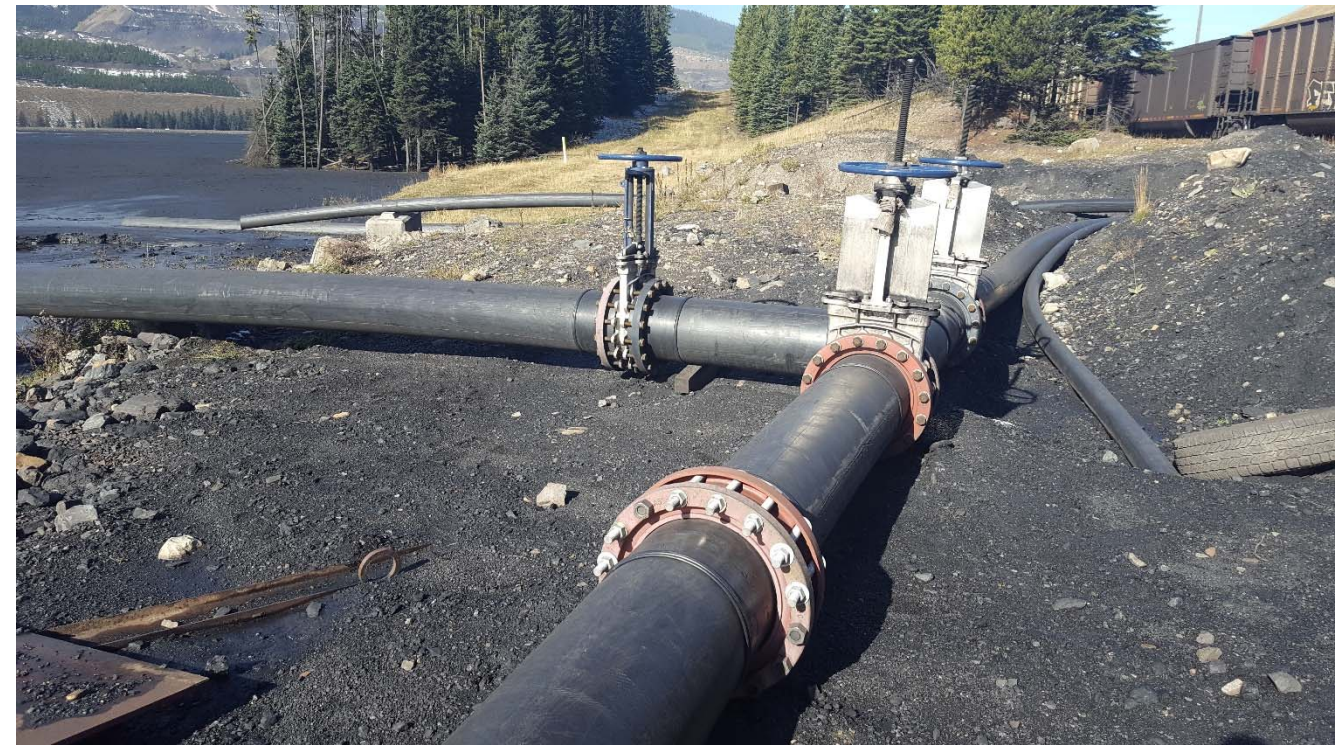
Photograph 24: Natural ground adjacent to railway line and emergency tailings dredge bypass, looking northwest. 4 October 2017.
