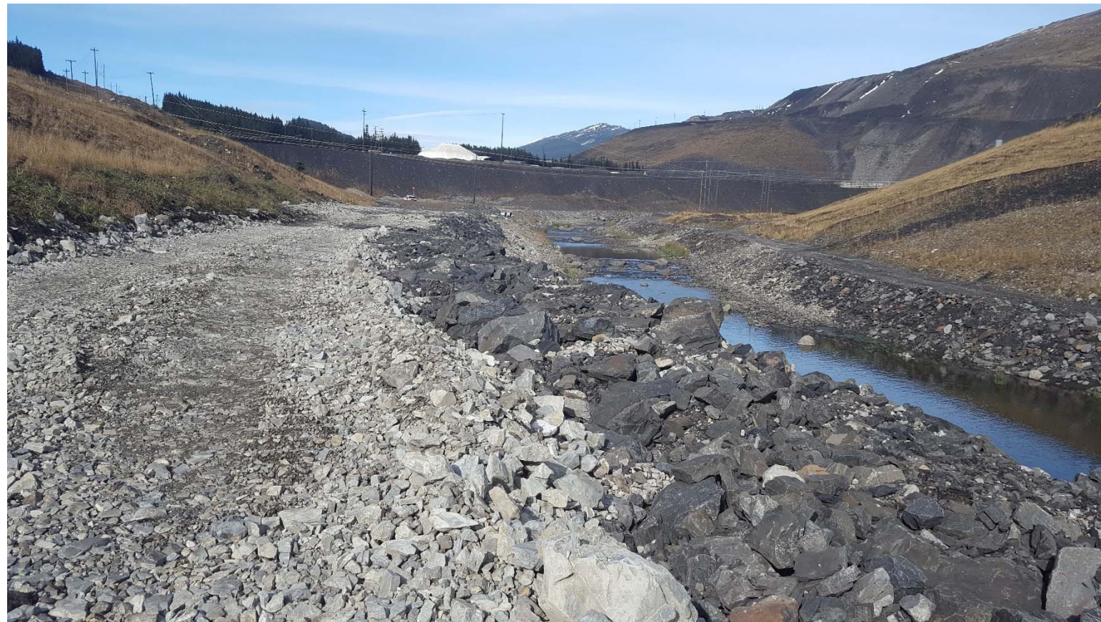
Photograph 21: NTP dam toe, downstream riprap recently raised, looking north. 4 October 2017.
