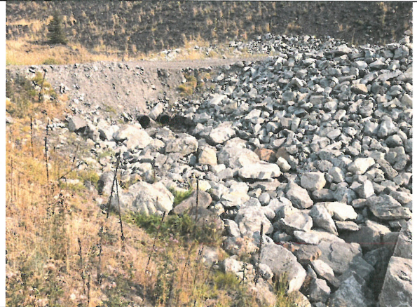
Photo 8: Looking upstream at STP riprap and drainage culverts along Maxam Creek (approx. Sta. 0+240 to 0+250)
