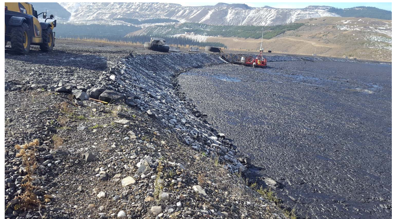
Photograph 29: STP Main Dam, new upstream constructed riprap 1.4H:1V, looking west. 4 October 2017.
