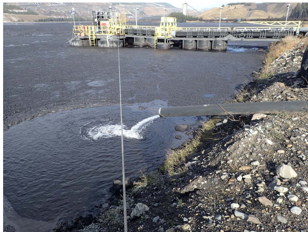
Photograph 28: STP Main Dam, barge at south end of pond and reclaim from seepage return wells, looking north. 4 October 2017.
