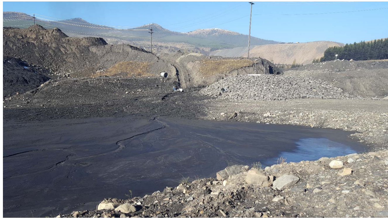
Photograph 18: NTP, surface runoff from haul road ditch reporting to tailings beach, looking west. 5 October 2017.
