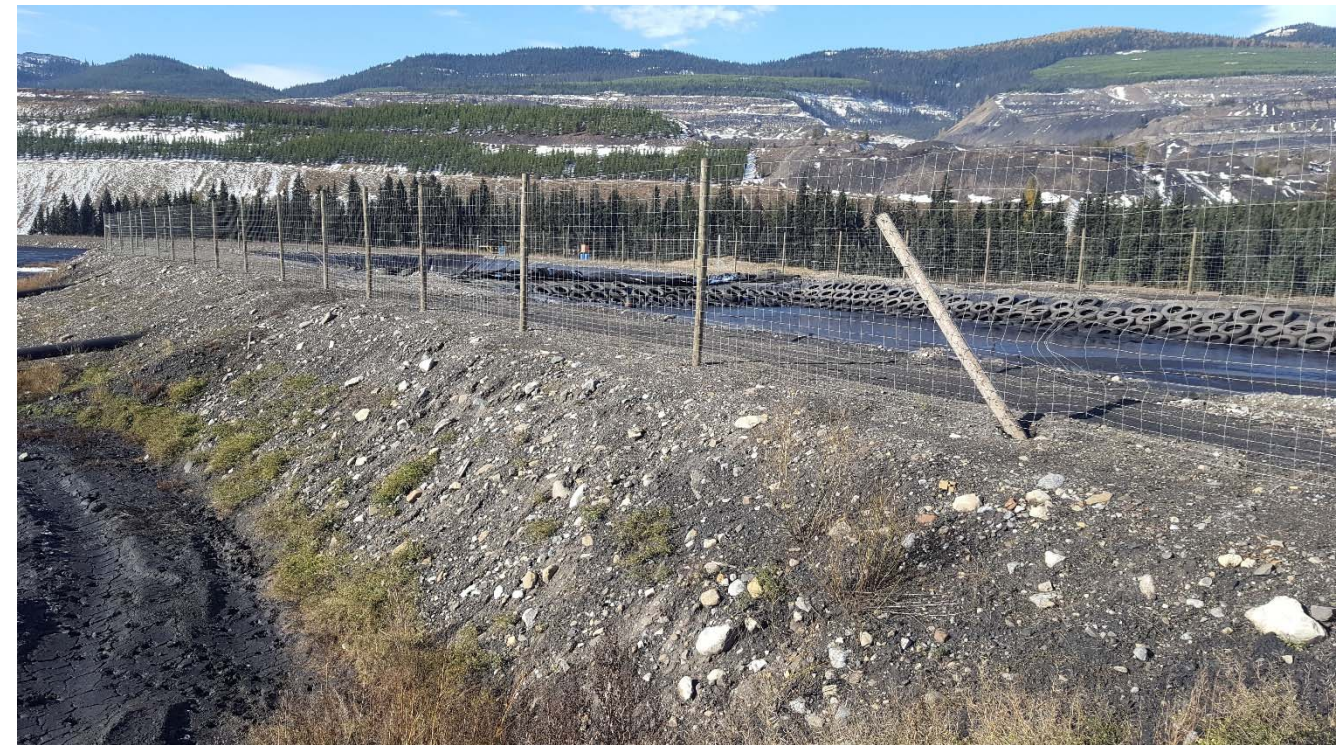
Photograph 54: STP north abutment, waste water cells, looking southwest. 4 October 2017.
