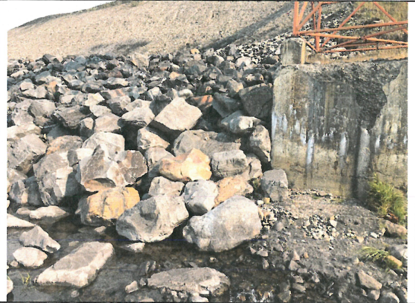
Photo 14: Looking at downstream extent of riprap (approx. Sta. 0+680)
