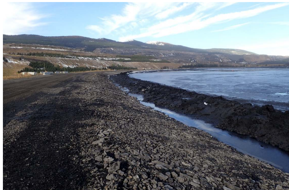
Photograph 36: STP West Dam, upstream slope with new riprap, looking northwest. Note tailings were pushed into pond to place riprap. 4 October 2017.
