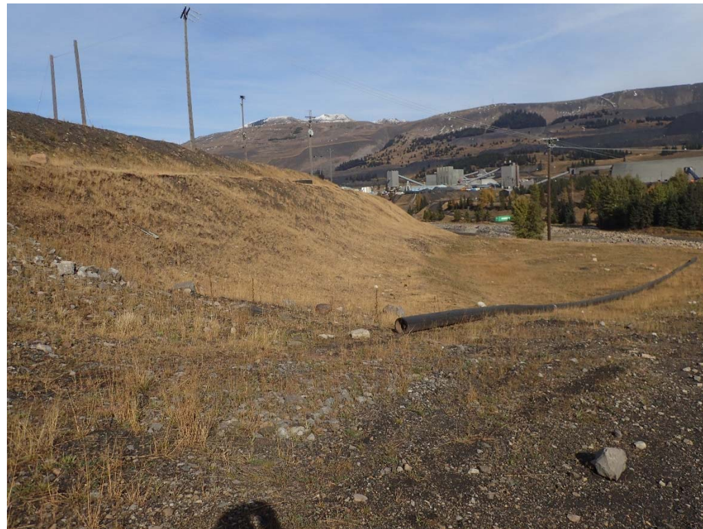
Photograph 2: NTP dam downstream slope overview from south abutment, looking northeast. 4 October 2017.
