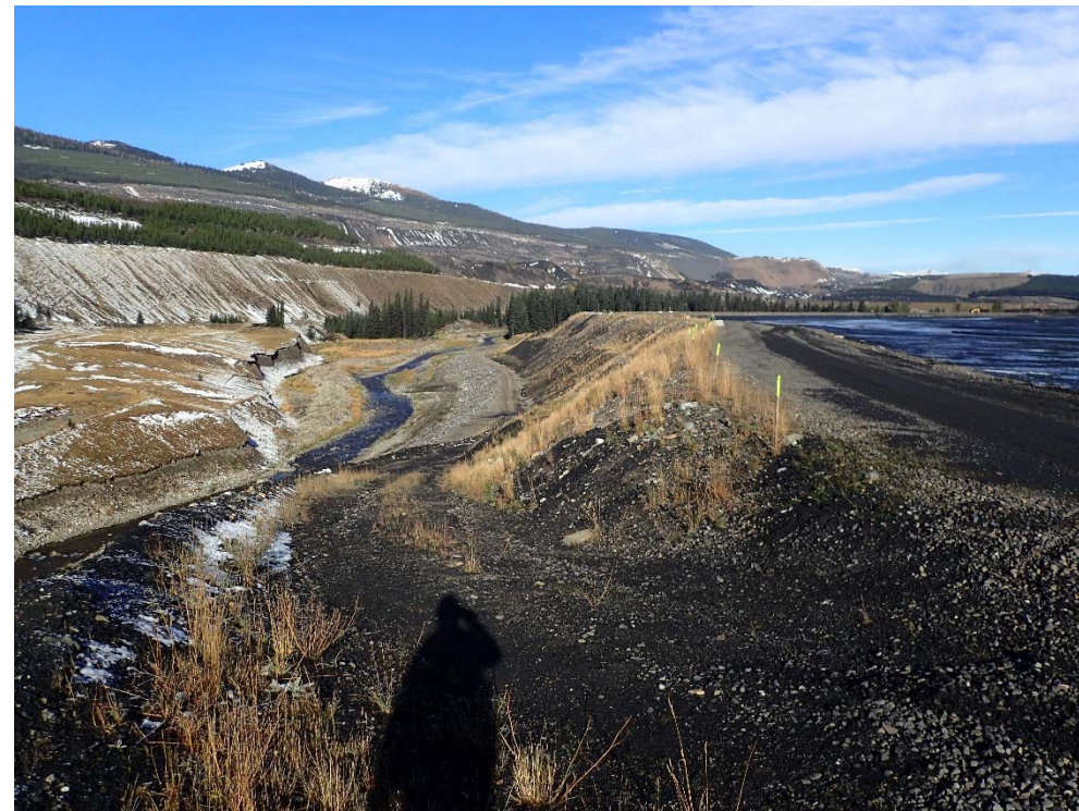
Photograph 46: STP West Dam, downstream slope overview and Fording River, looking northwest. 4 October 2017.
