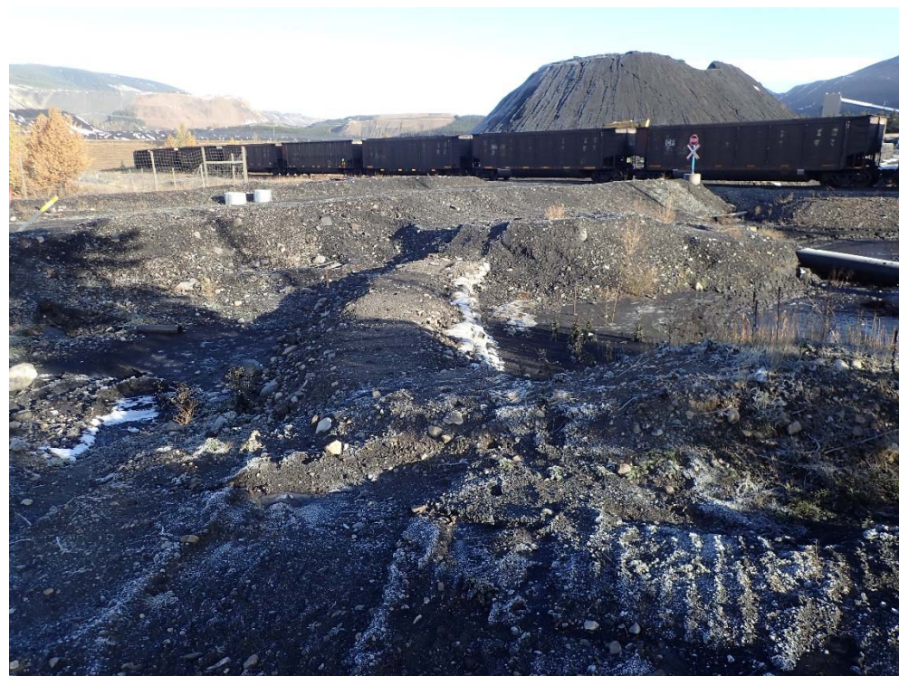
Photograph 55: STP north abutment, recently constructed upstream till berm, looking northeast. 4 October 2017.
