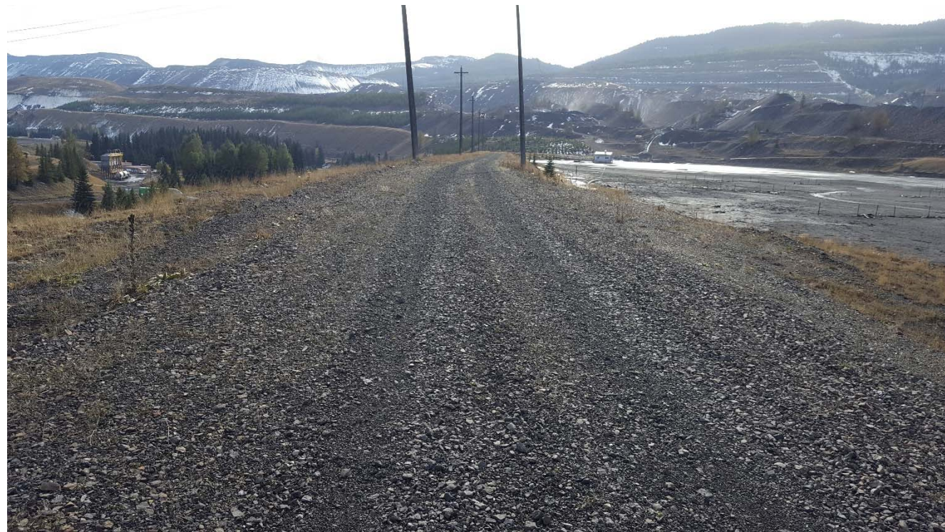
Photograph 11 : NTP crest, looking southwest. 4 October 2017.
