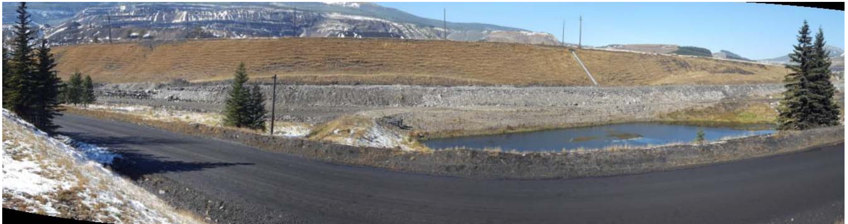
Photograph 10: NTP dam downstream slope and riprap overview from North Loop Pond, looking northwest. 3 October 2017.
