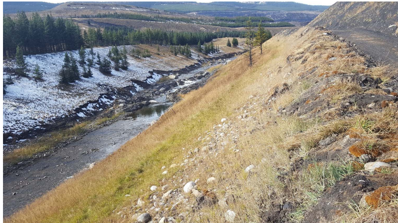
Photograph 38: STP West Dam, downstream slope, looking northwest. 4 October 2017.
