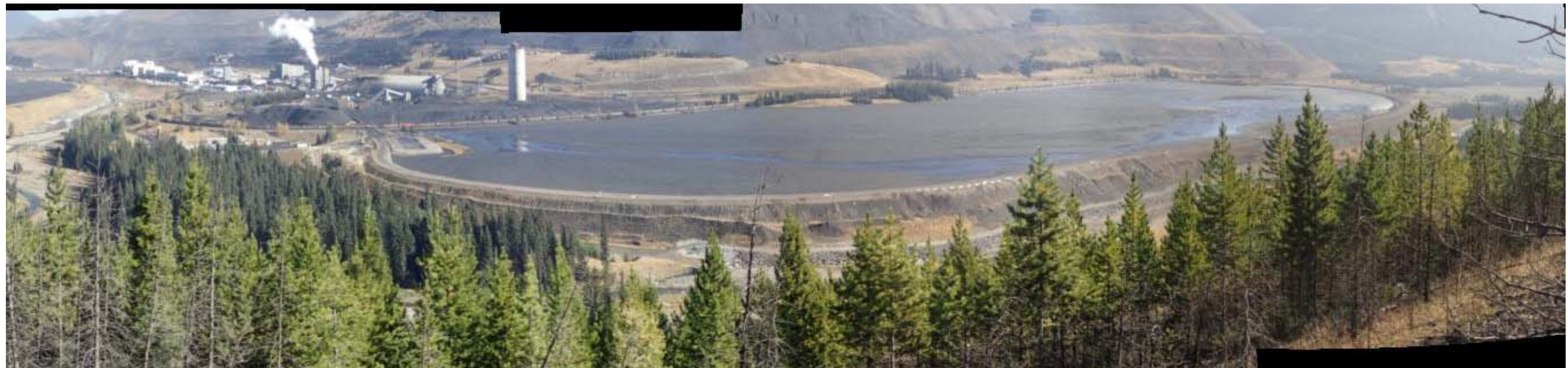
Photograph 22: South Tailings Pond (STP) overview from west side of Fording River, looking southeast. 5 October 2017.
