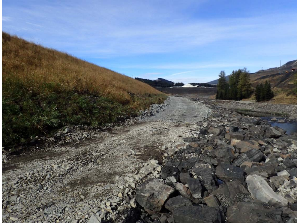
Photograph 15: NTP downstream slope and riprap along Fording River, looking north. 4 October 2017.
