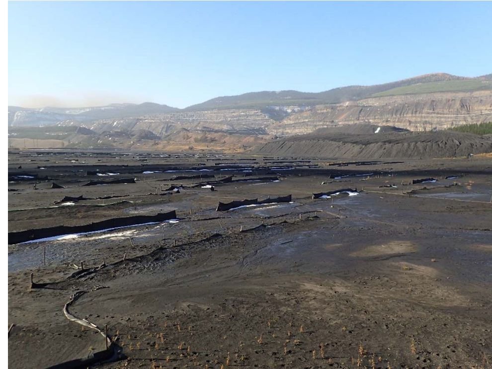
Photograph 16: NTP, tailings surface with silt fencing for dust control, looking southwest. 5 October 2017.
