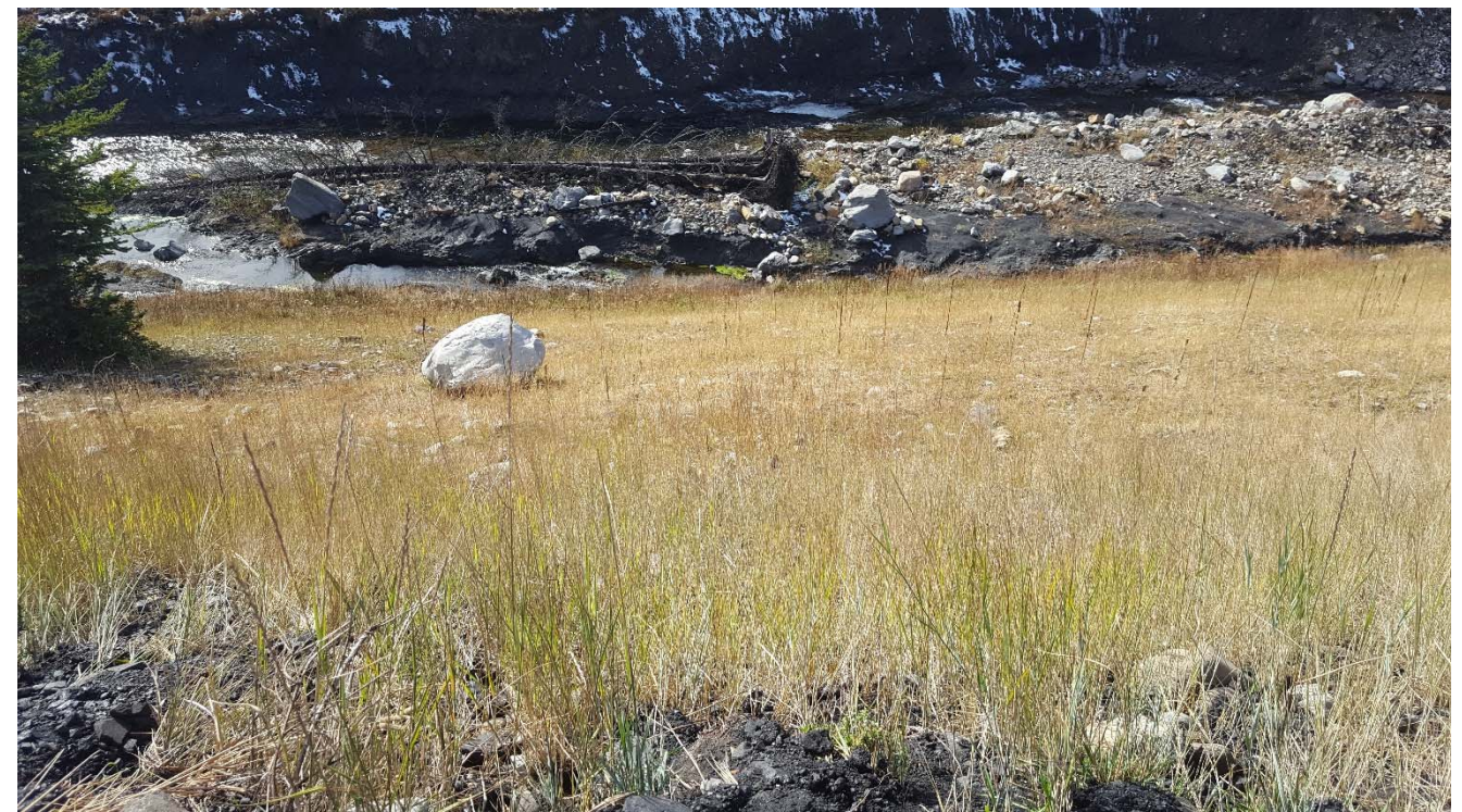
Photograph 42: STP West Dam, downstream slope and Fording River, looking southwest. 4 October 2017.
