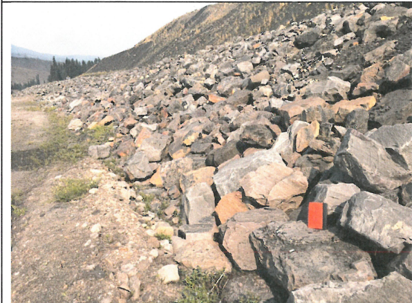
Photo 11: Looking upstream at STP riprap (approx. Sta. 0+360 to 0+460)
