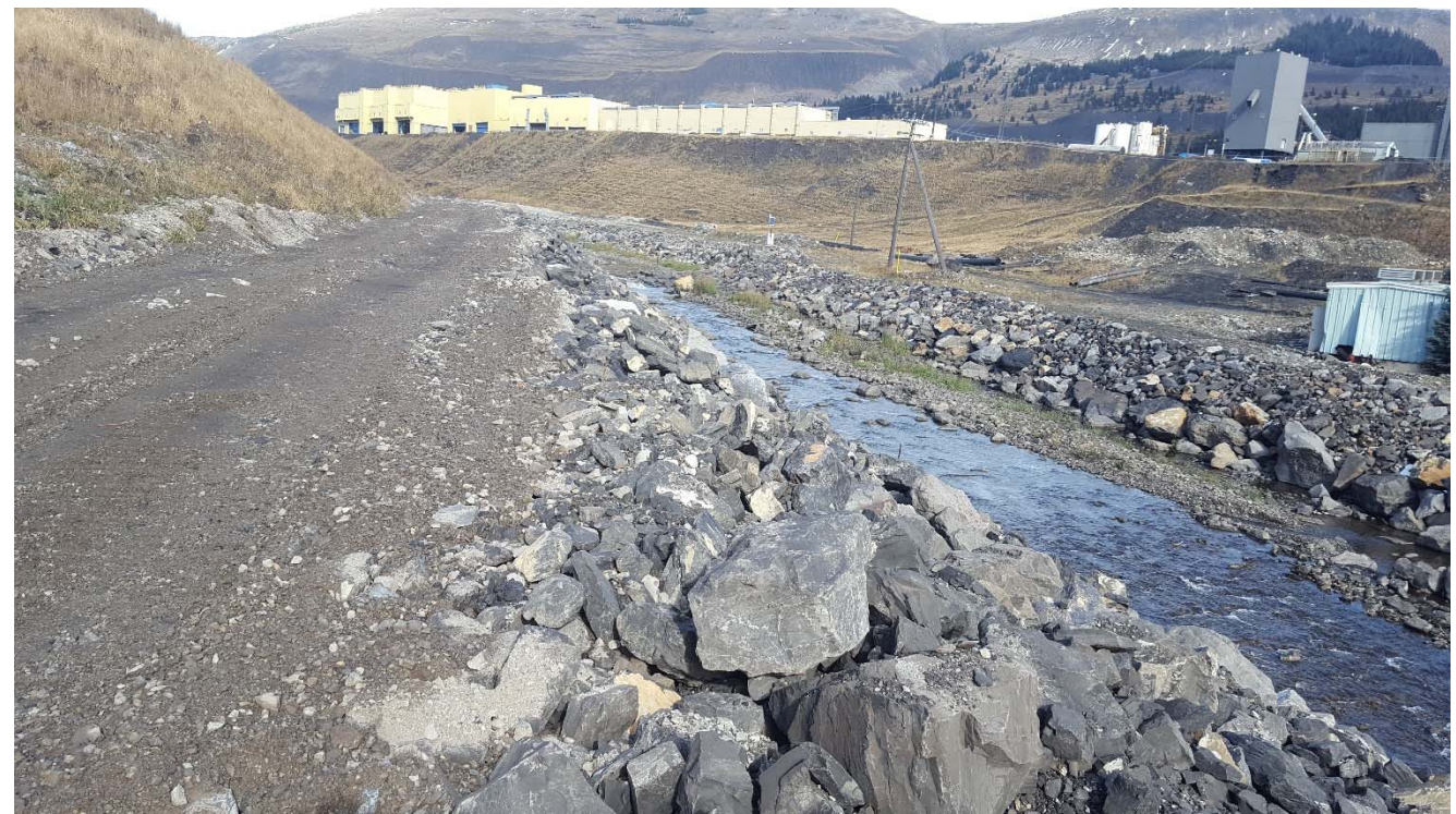
Photograph 12 : NTP toe, riprap along Fording River, looking northeast. 4 October 2017.
