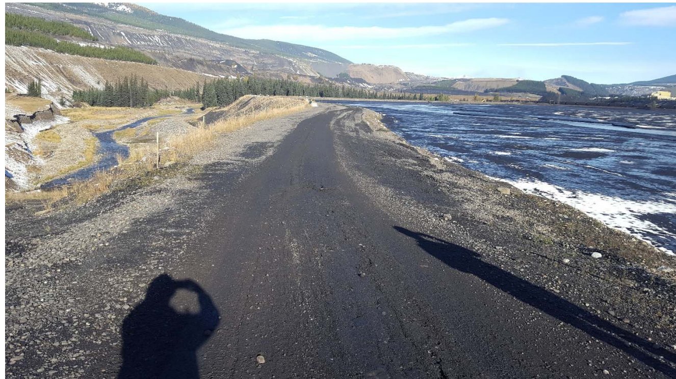
Photograph 45: STP West Dam crest and tailings pond overview, looking northwest. 4 October 2017.
