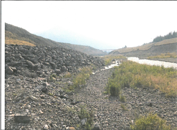
Photo 9: Looking downstream at STP riprap (approx. Sta. 0+280 to 0+360)
