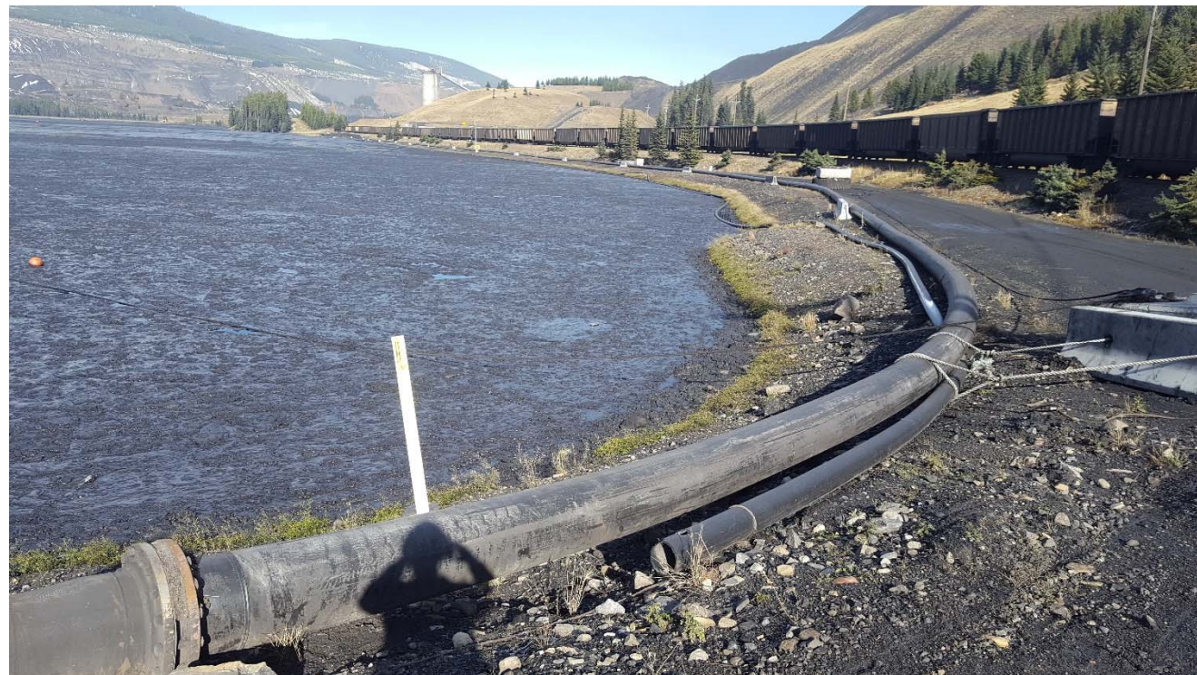
Photograph 25: STP south abutment till blanket area and gas line crossing location, looking northeast. 4 October 2017.
