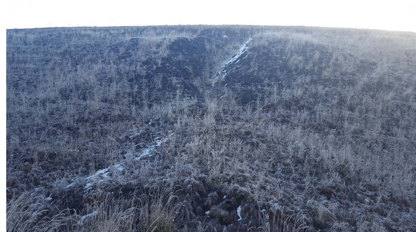
Photograph 52: STP West Dam, erosion gully, looking east. 4 October 2017.
