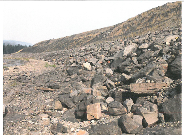
Photo 12: Looking upstream at STP riprap (approx. Sta. 0+360 to 0+580)
