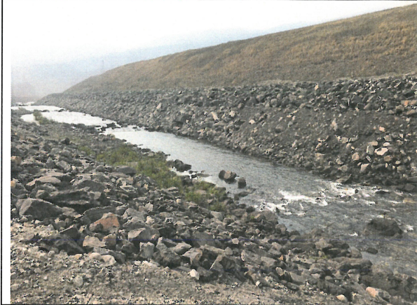
Photo 5: Looking downstream at NTP riprap (far bank) covered by gravel (approx. Sta. 0+620 to 0+800)
