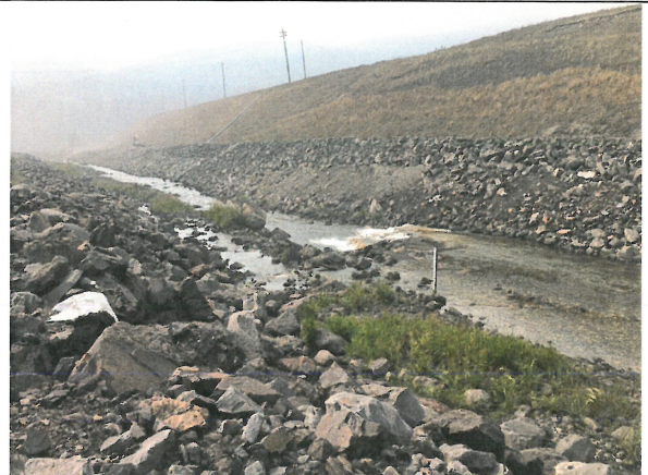
Photo 6: Looking downstream at NTP riprap (far bank) covered by gravel (approx. Sta. 0+840 to 0+940)
