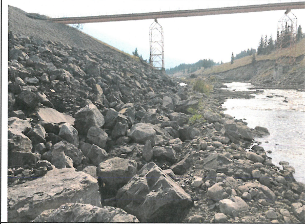
Photo 13: Looking downstream at STP riprap (approx. Sta. 0+580 to 0+680)
