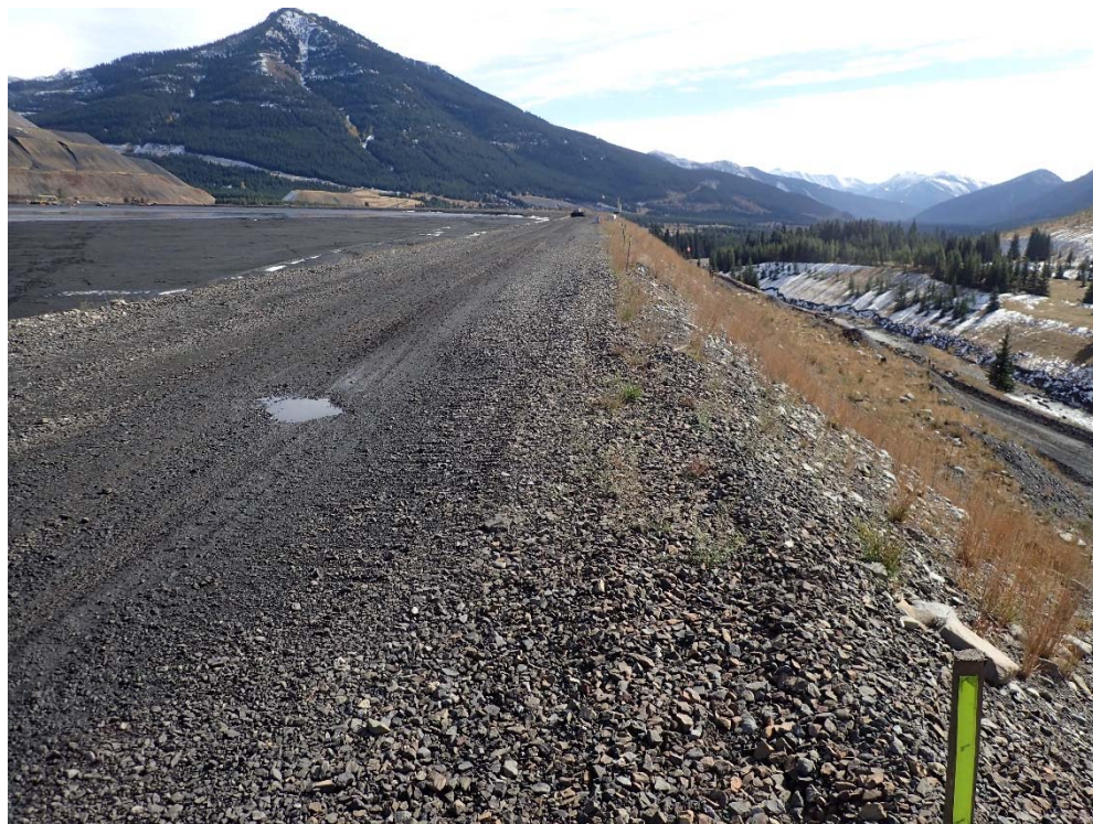
Photograph 41: STP West Dam crest overview, looking southeast. Note crest regraded. 4 October 2017.
