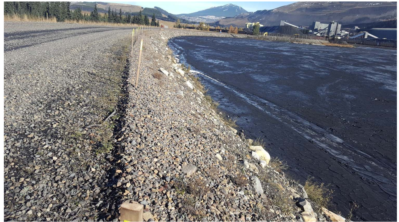
Photograph 50: STP upstream slope and crest, looking north. 4 October 2017.
