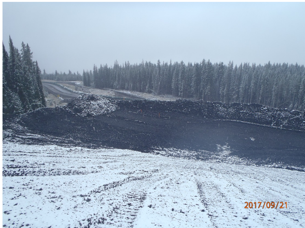
Photograph 23: West Dam – downstream slope at south abutment, looking west.
