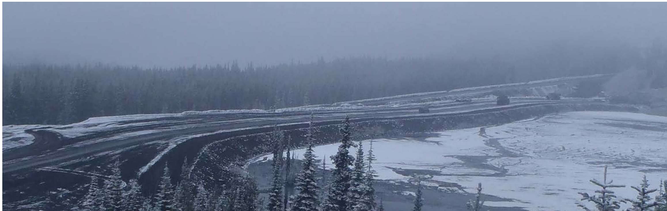
Photograph 18: West Dam – overview of upstream slope, looking northwest. 21 September 2017.
