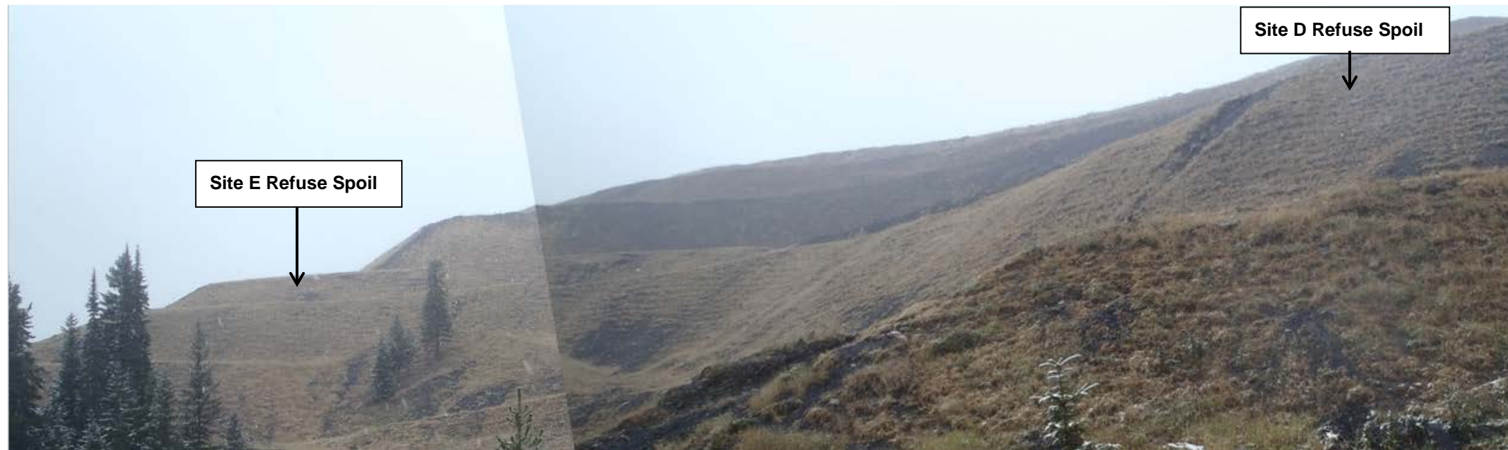
Photograph 10: Site D and E – overview of Site D and Site E coarse coal refuse spoils, looking northwest. 21 September 2017.
