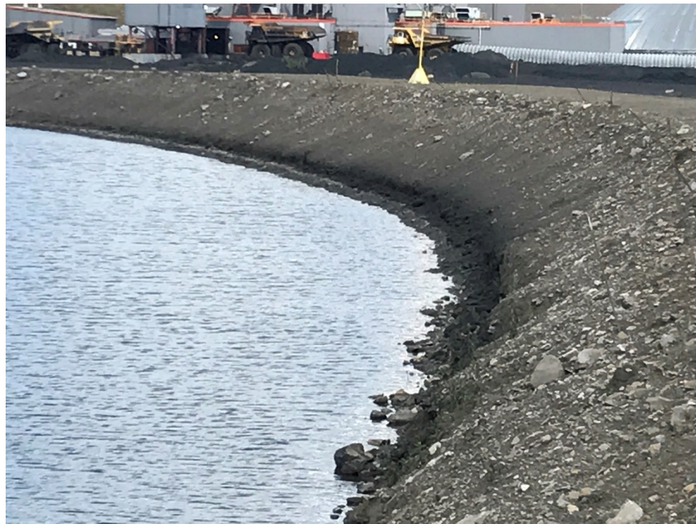
Photograph 6: Main Dam – upstream slope, looking northeast. 30 July 2017.
