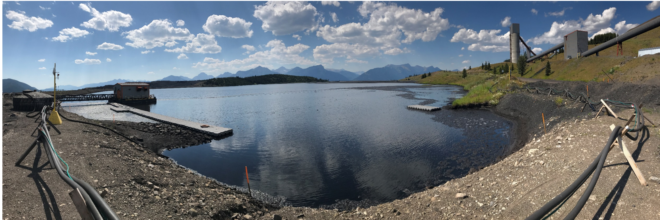
Photograph 3: Main Dam – overview of barge, looking southwest. 30 July 2017.
