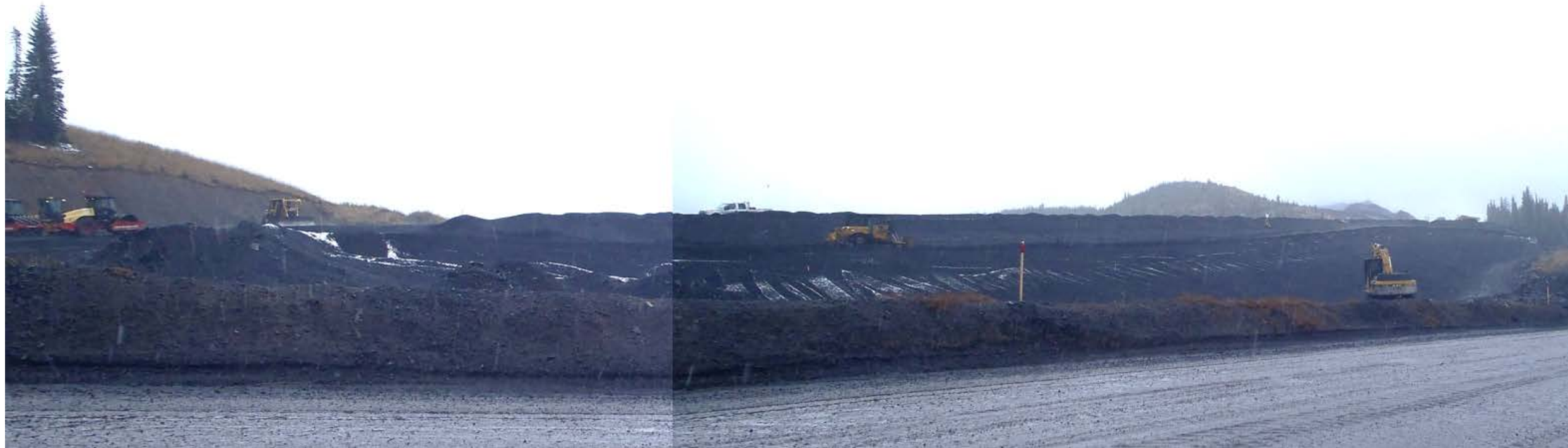
Photograph 19: West Dam – overview of downstream slope under construction, looking southeast. 21 September 2017.
