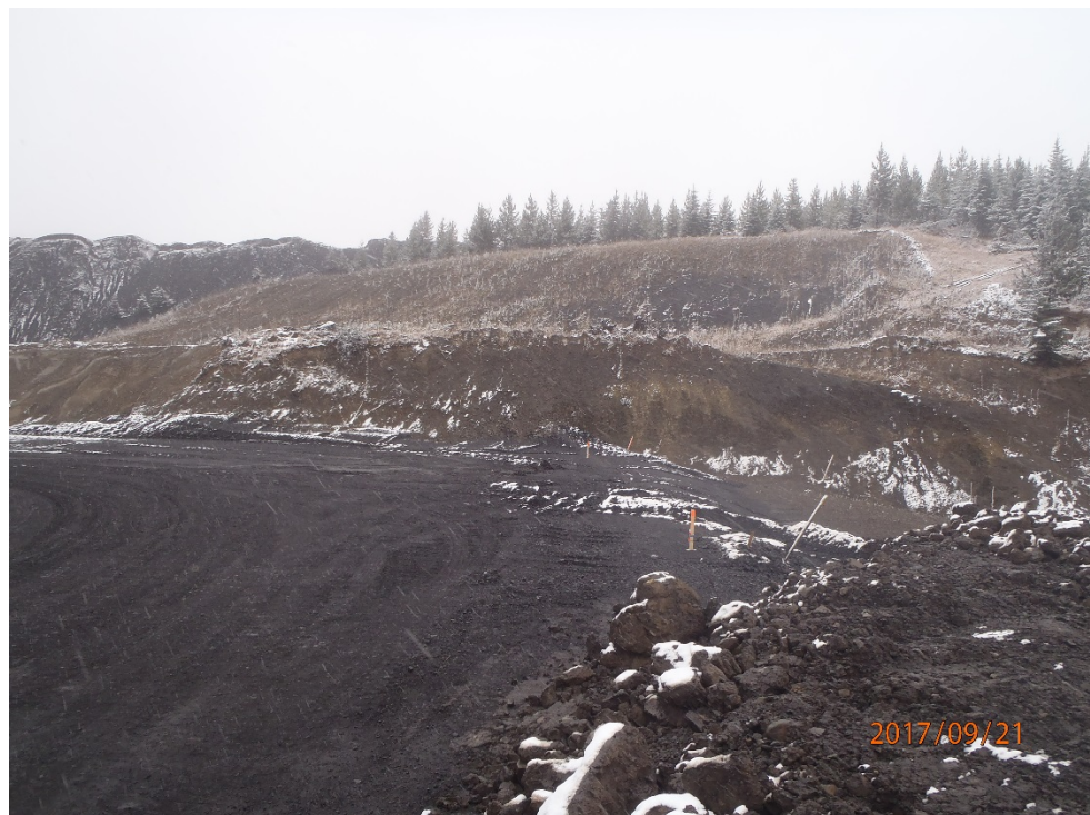
Photograph 8: Main Dam – west abutment, looking west. 21 September 2017.
