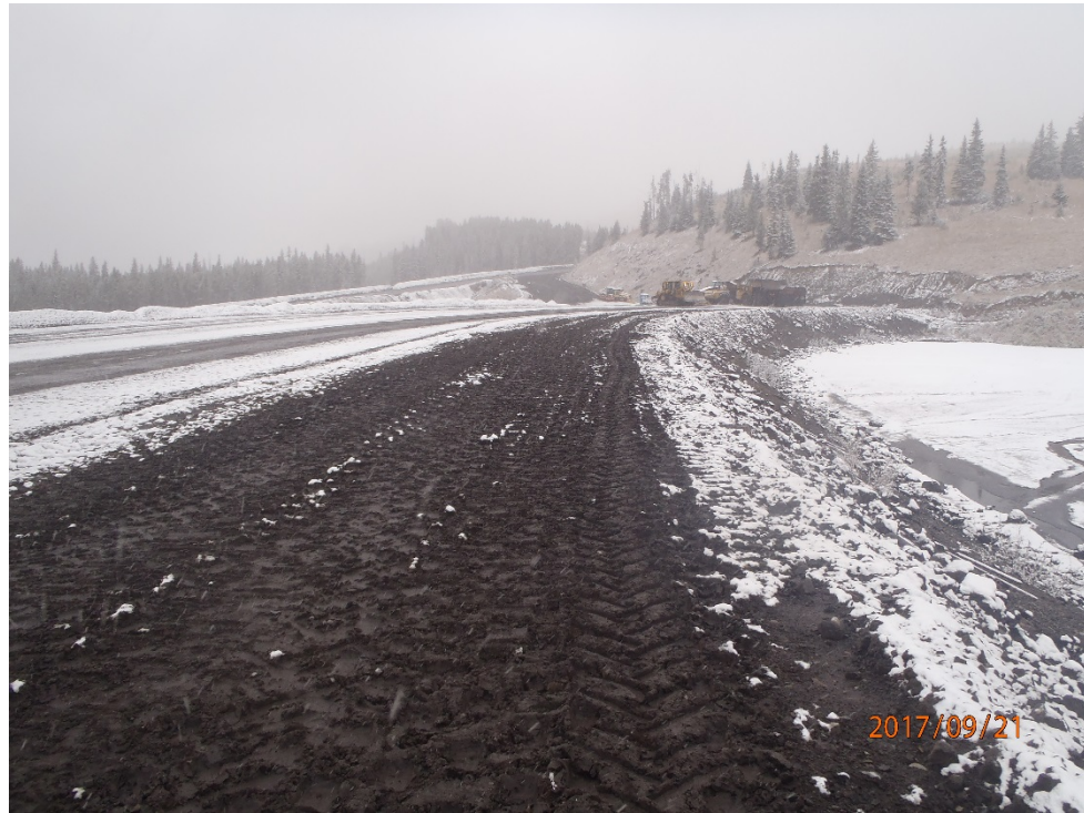
Photograph 21: West Dam – upstream slope, crest and north abutment looking north. 21 September 2017.
