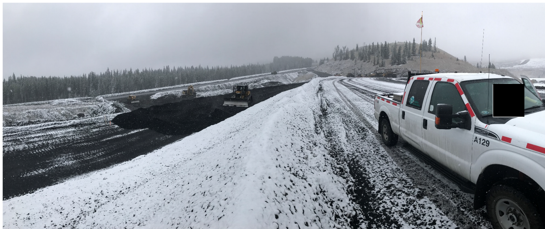
Photograph 20: West Dam – downstream slope under construction, looking north. 21 September 2017.
