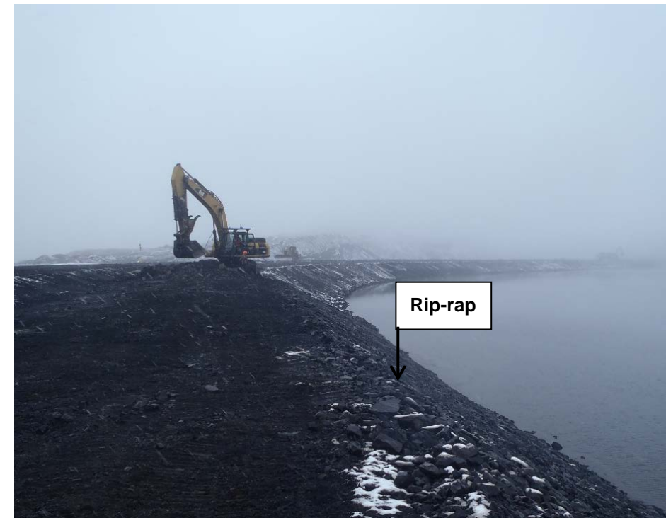
Photograph 5: Main Dam – upstream slope and crest, looking southwest. 21 September 2017.
