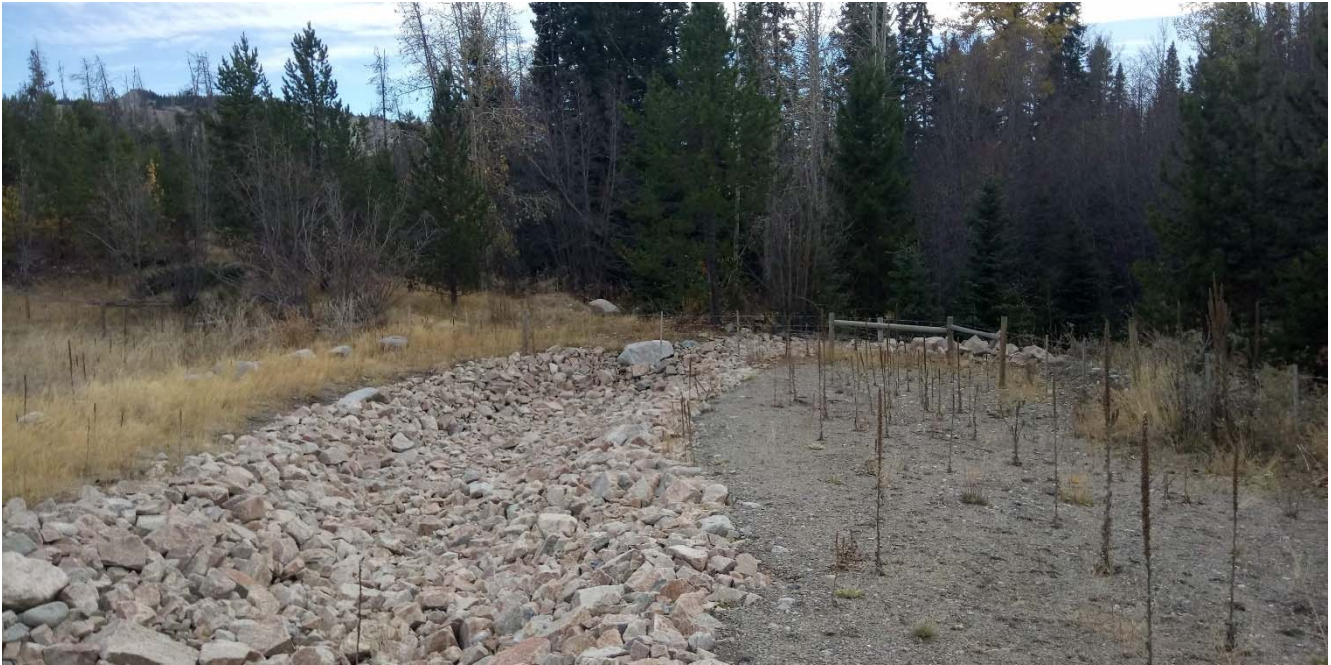
Photo II-B- 7 Final portion of spillway riprap, view downstream towards outfall (TRJ-2017-19)
