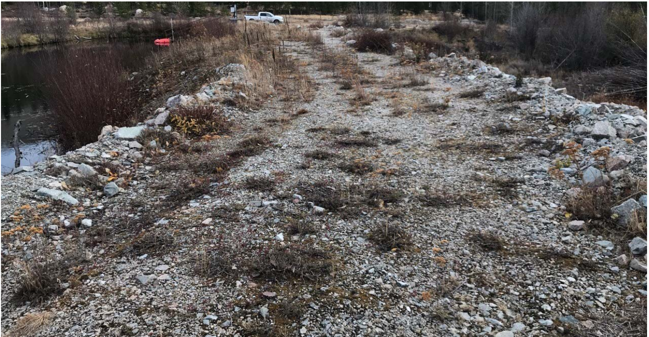
Photo II-C- 3 Overflow near right abutment. Heavy vegetation in front of pipe which could lead to an obstruction. Flow discharges to the dam's right toe (TRJ-2017-23)
