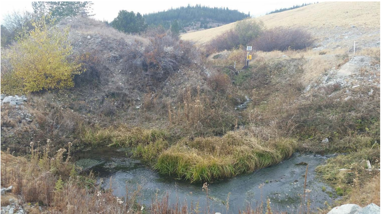
Photo II-A- 28 Weir for right abutment seepage toe drain, flow observed (TRJ-2017-06)
