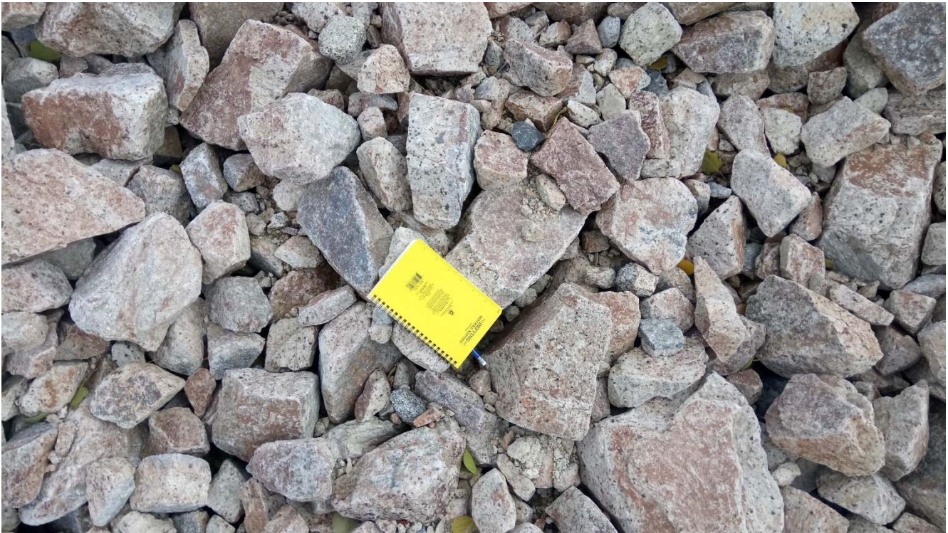
Photo II-B- 9 Downstream slope, no signs of erosion, view from spillway (TRJ-2017-17)
