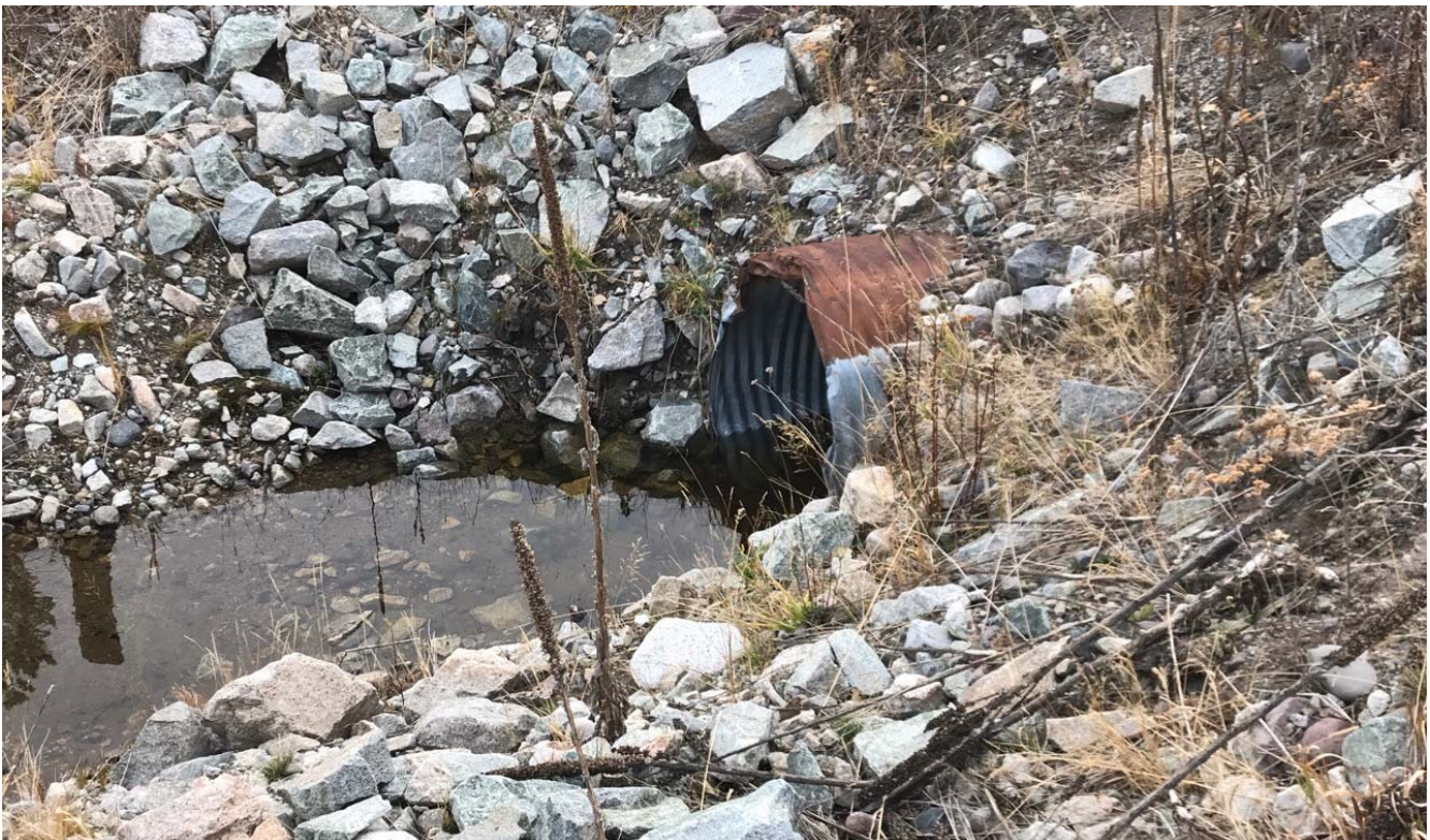
Photo II-A- 32 Diversion channel intersection point, road culvert free of obstructions (TRJ-2017-28)
