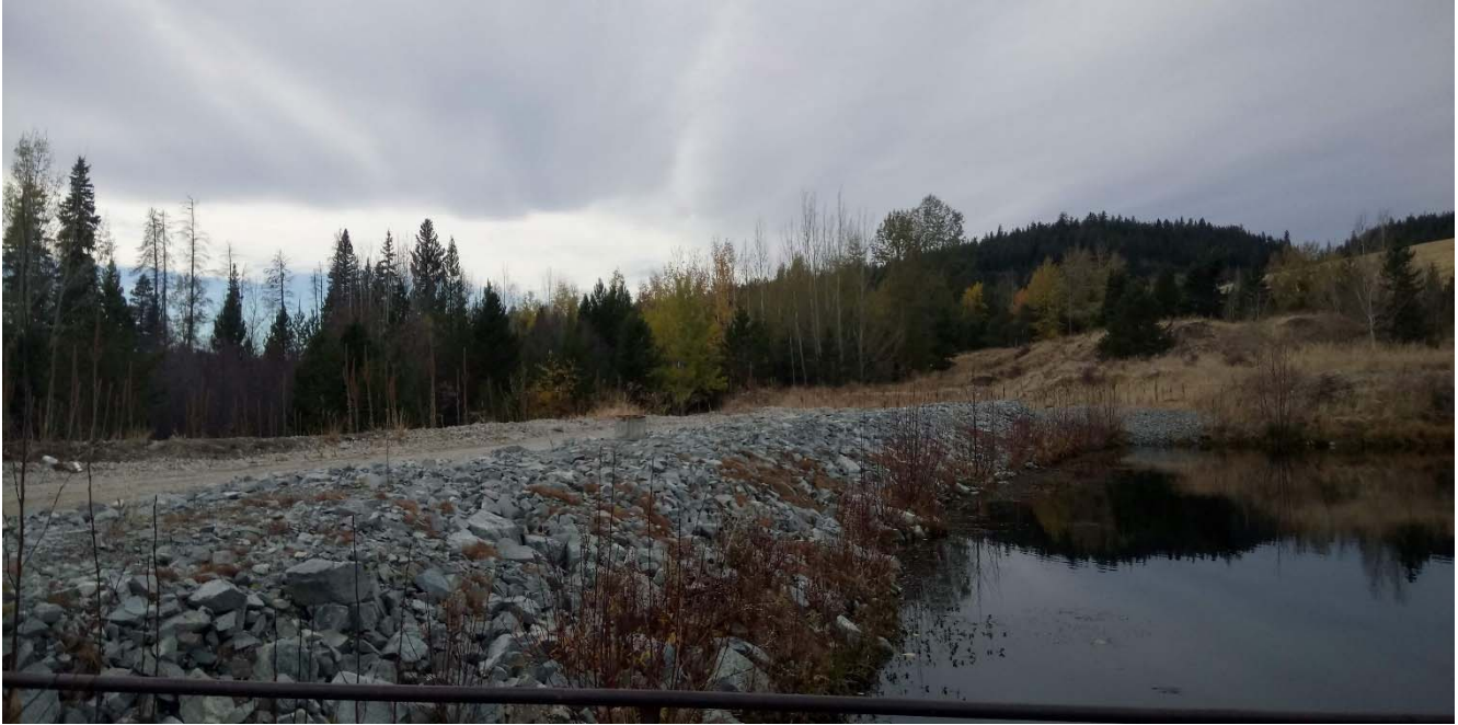
Photo II-B- 3 Low-level outlet to Witches Brook (via Lower Trojan Dam) and wooden debris boom. Debris boom has minimal vegetation, and minor obstructions present in trash rack, therefore material was cleared since 2016 inspection (TRJ-2017-15)
