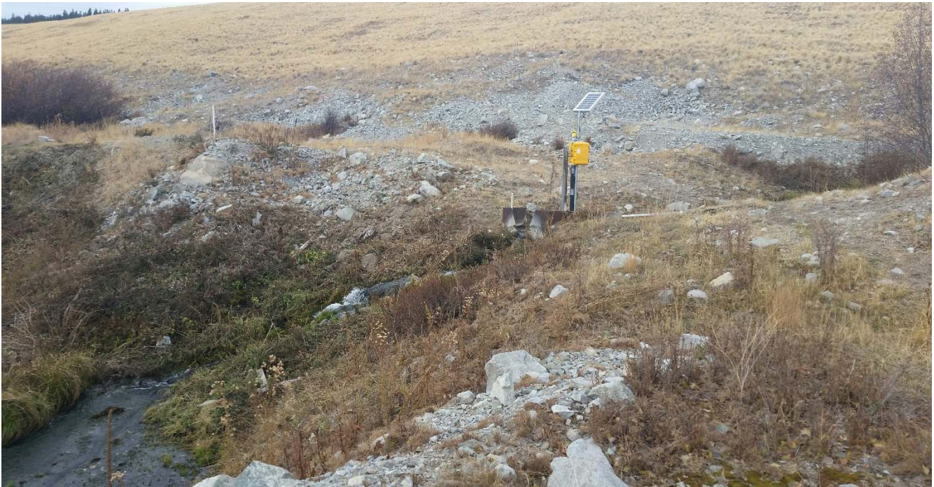
Photo II-A- 28 Weir for right abutment seepage toe drain, flow observed (TRJ-2017-06)
