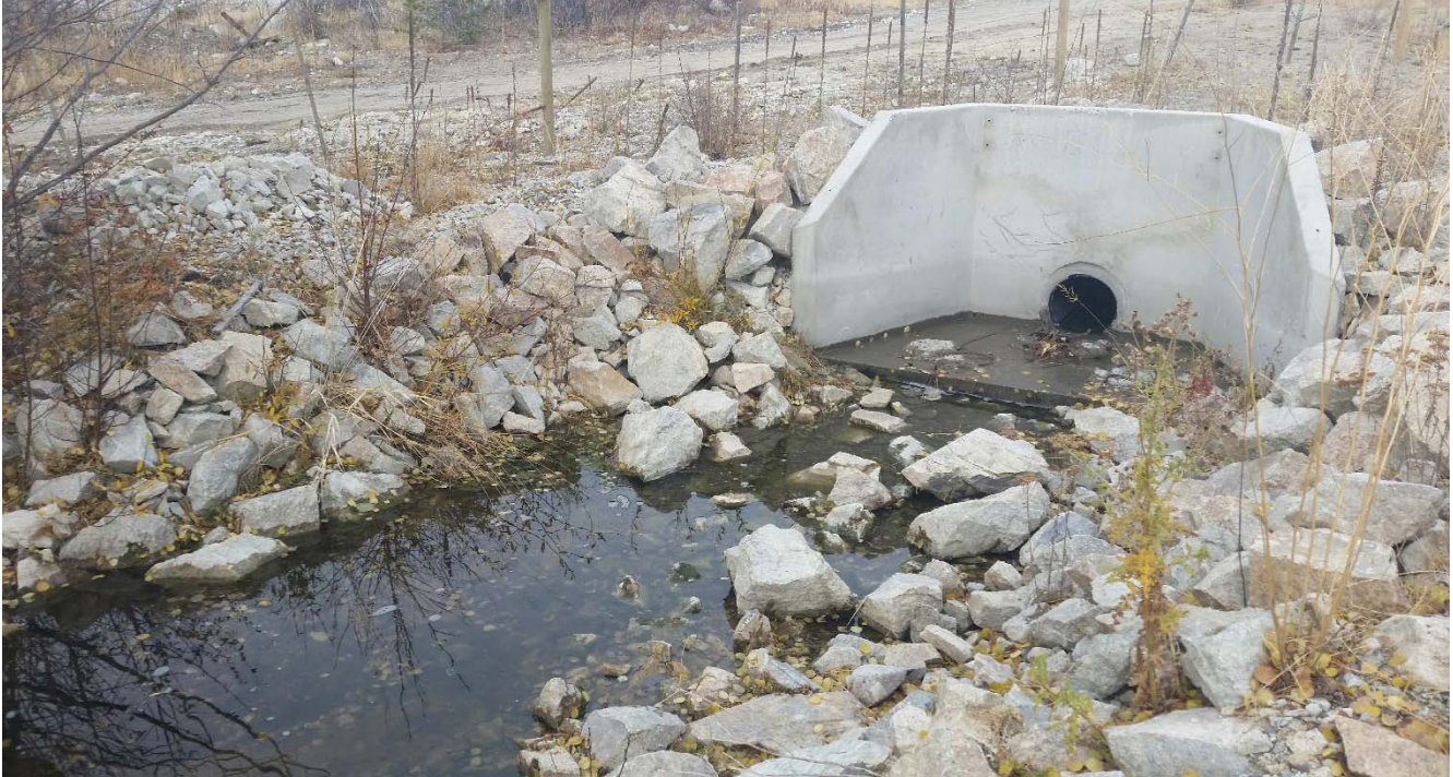
Photo II-C- 12 Inflow culvert from Trojan Diversion Ditch (TRJ-2017-25)
