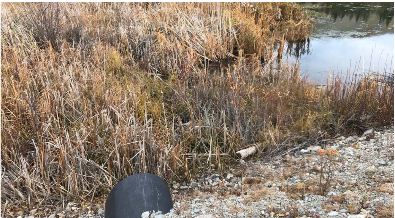
Photo II-C- 3 Overflow near right abutment. Heavy vegetation in front of pipe which could lead to an obstruction. Flow discharges to the dam's right toe (TRJ-2017-23)
