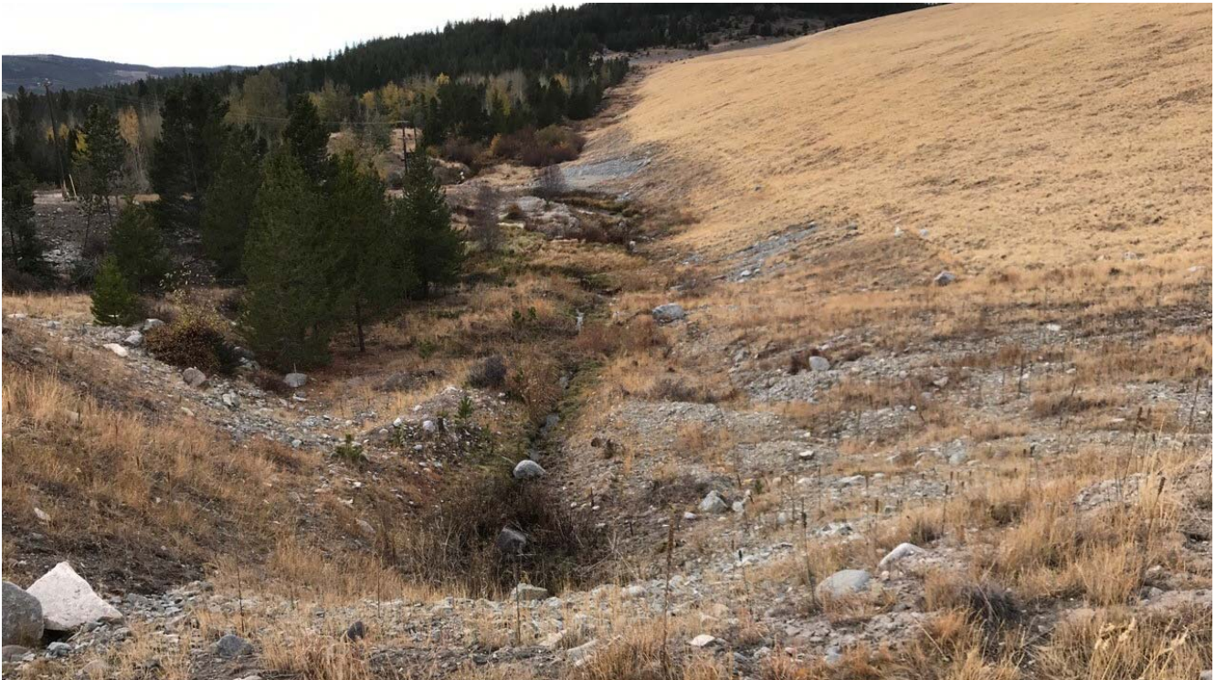
Photo II-A- 26 Seepage collection ditch view towards right abutment, flow observed (TRJ-2017-07)
