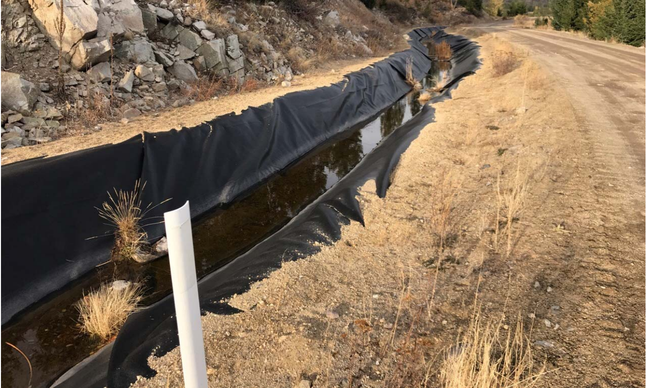
Photo II-A- 30 Damage to liner observed on diversion channel (TRJ-2017-26)
