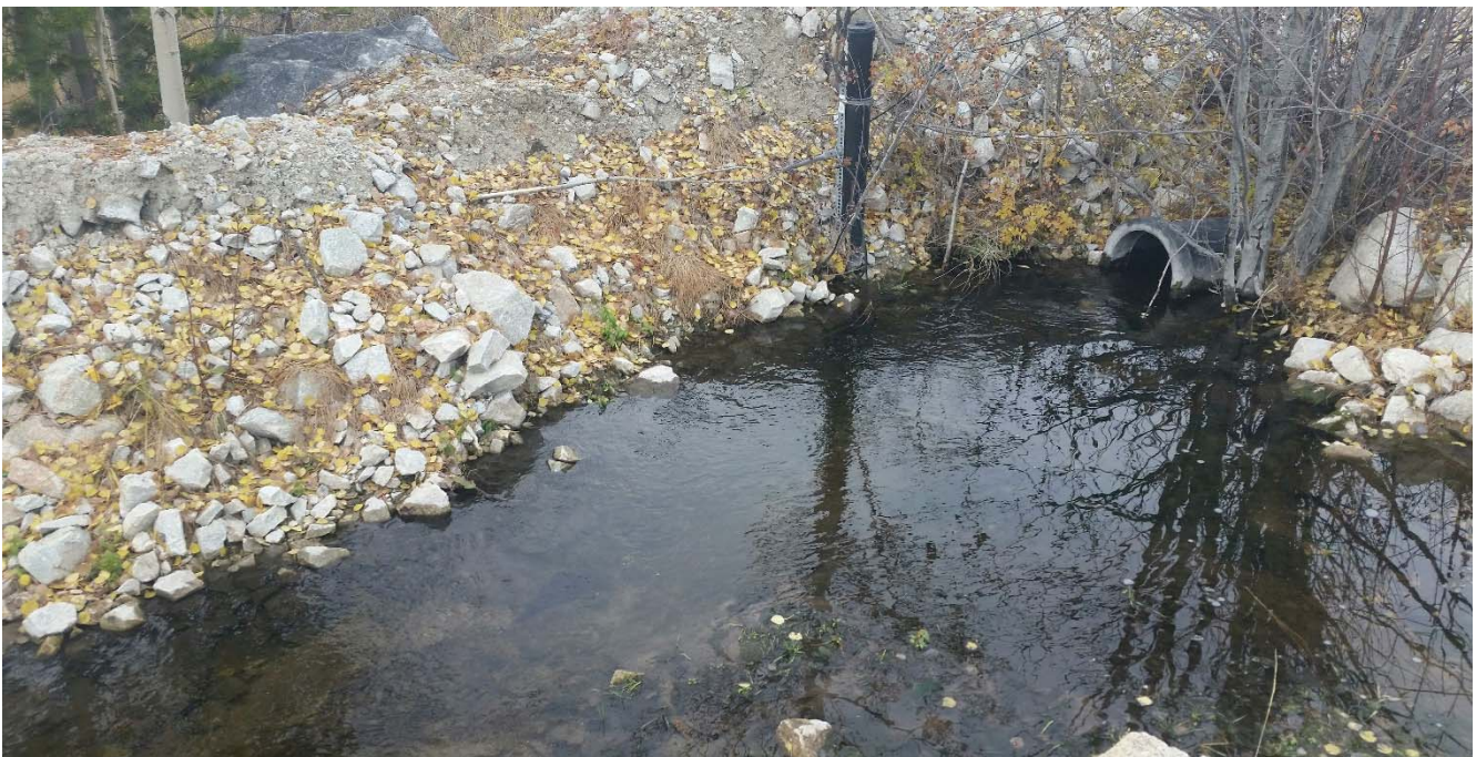
Photo II-C- 11 Low-level outlet discharge pipe, no obstructions present (TRJ-2017-25)
