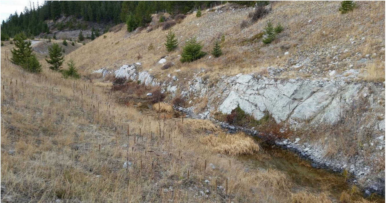
Photo II-A- 17 Spillway channel with exposed bedrock and pooled water view upstream (TRJ-2017-09)
