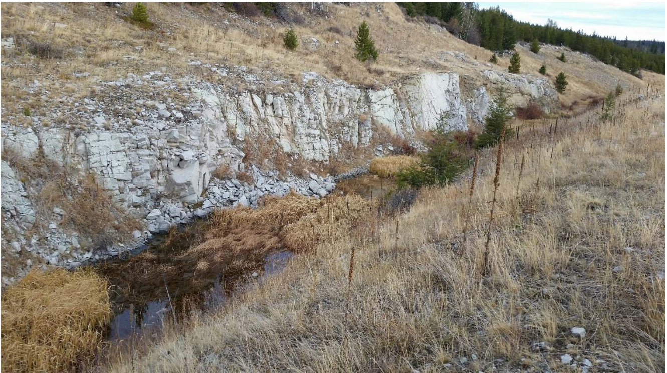
Photo II-A- 17 Spillway channel with exposed bedrock and pooled water view upstream (TRJ-2017-09)
