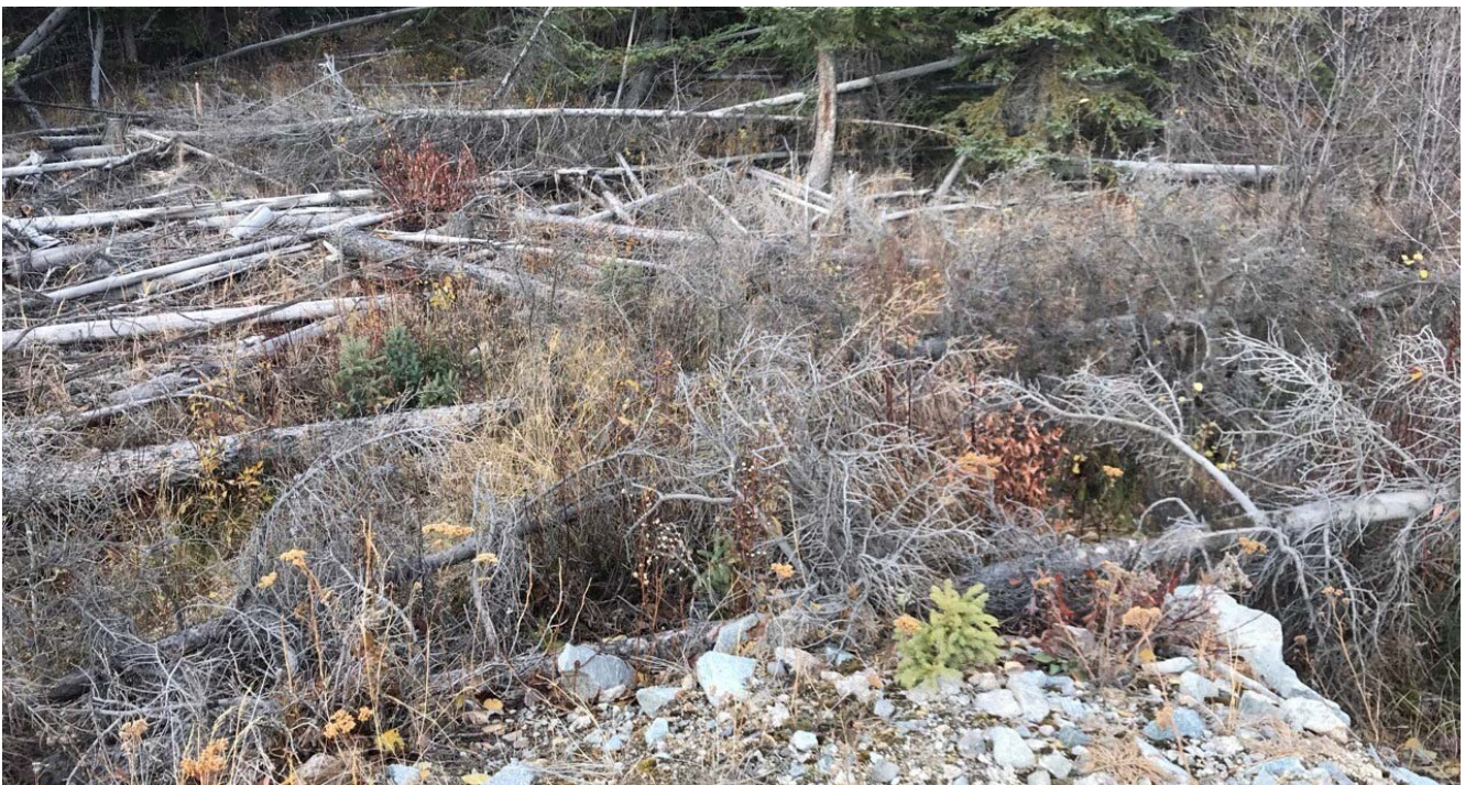
Photo II-C- 5 Spillway route filled with debris, no visible channel or flow path (TRJ-2017-24)
