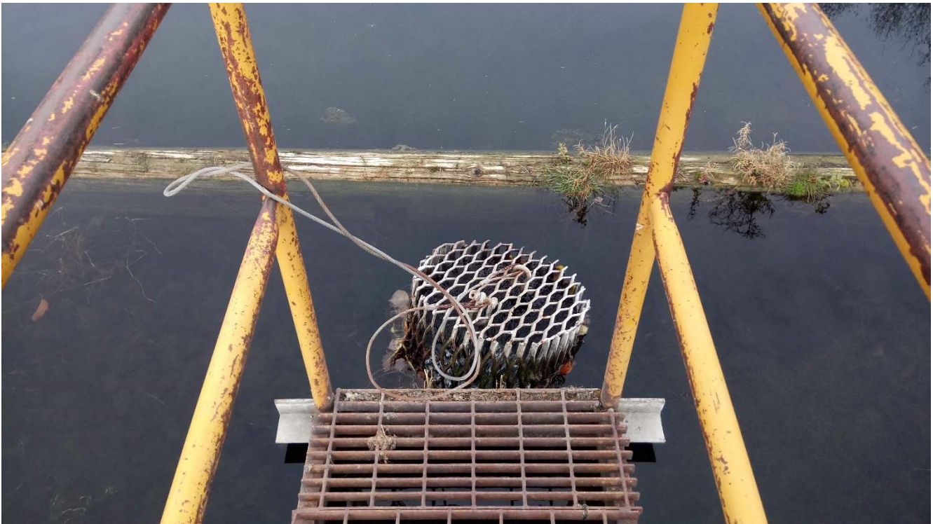
Photo II-B- 3 Low-level outlet to Witches Brook (via Lower Trojan Dam) and wooden debris boom. Debris boom has minimal vegetation, and minor obstructions present in trash rack, therefore material was cleared since 2016 inspection (TRJ-2017-15)
