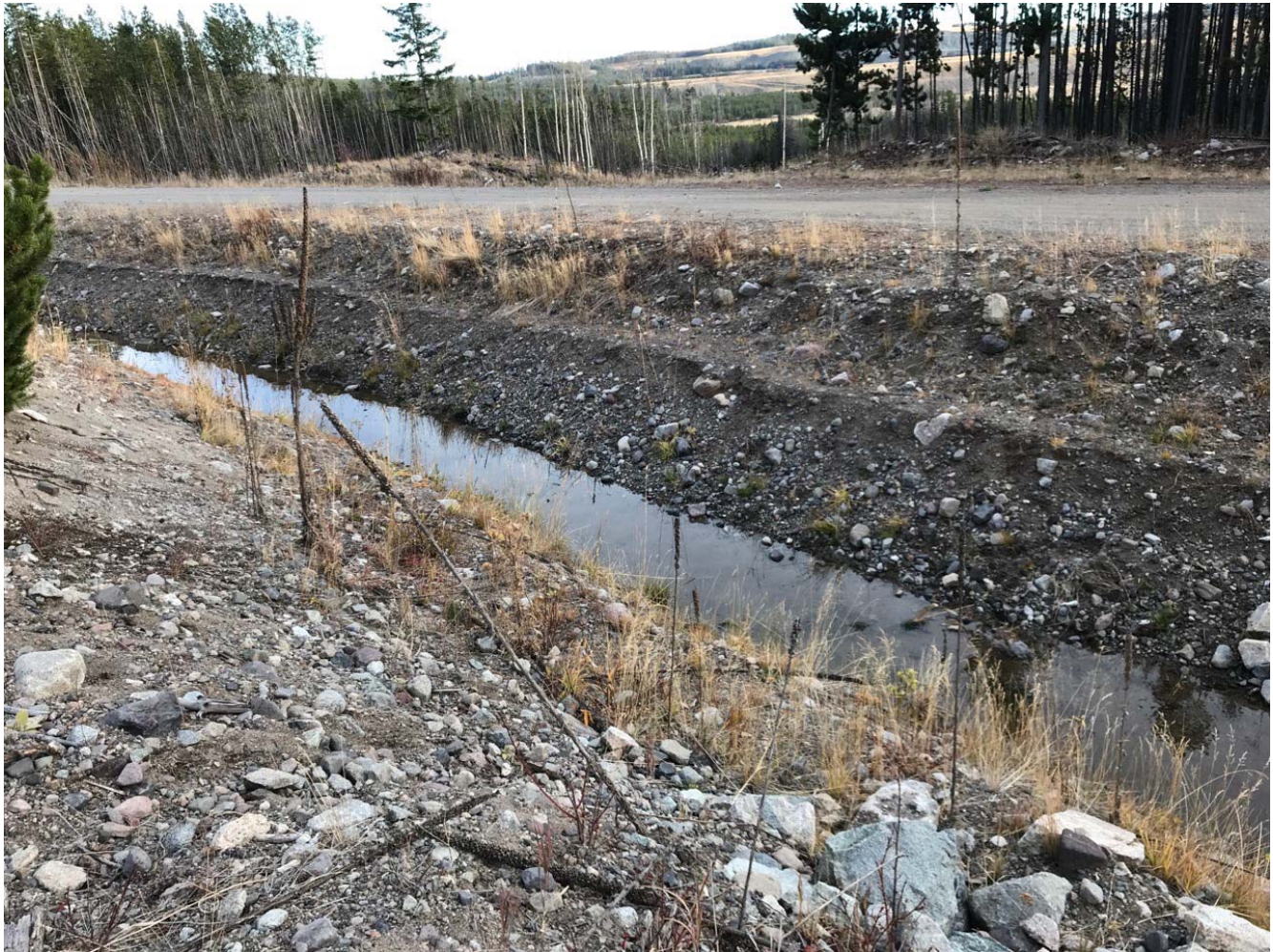
Photo II-A- 33 Continuation of till lined section of diversion channel (TRJ-2017-28)
