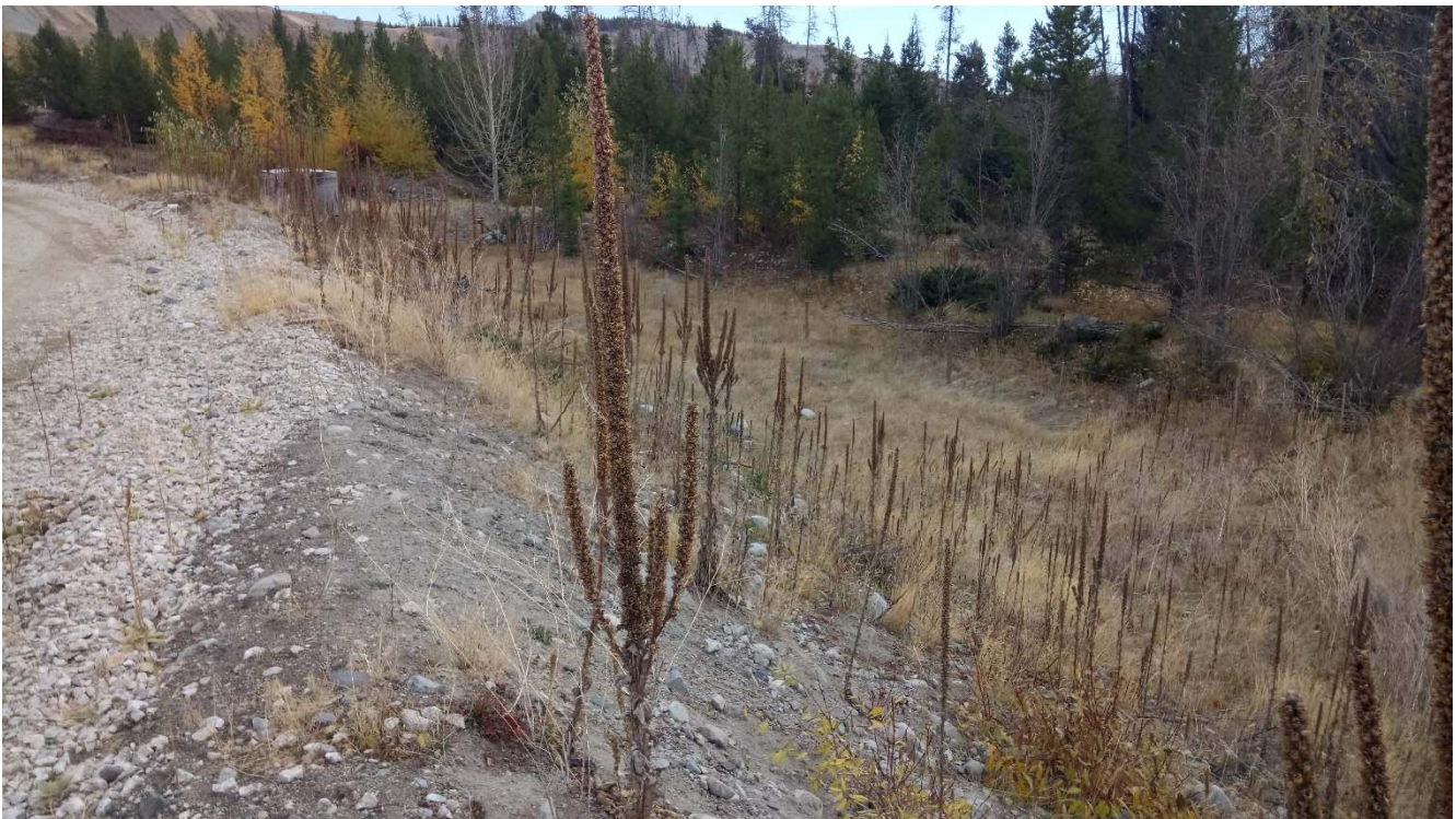
Photo II-B- 9 Downstream slope, no signs of erosion, view from spillway (TRJ-2017-17)
