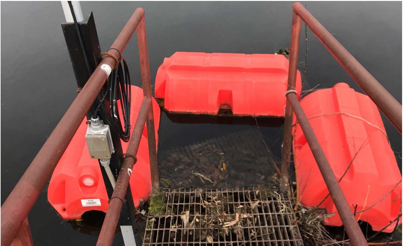
Photo II-C- 11 Low-level outlet discharge pipe, no obstructions present (TRJ-2017-25)
