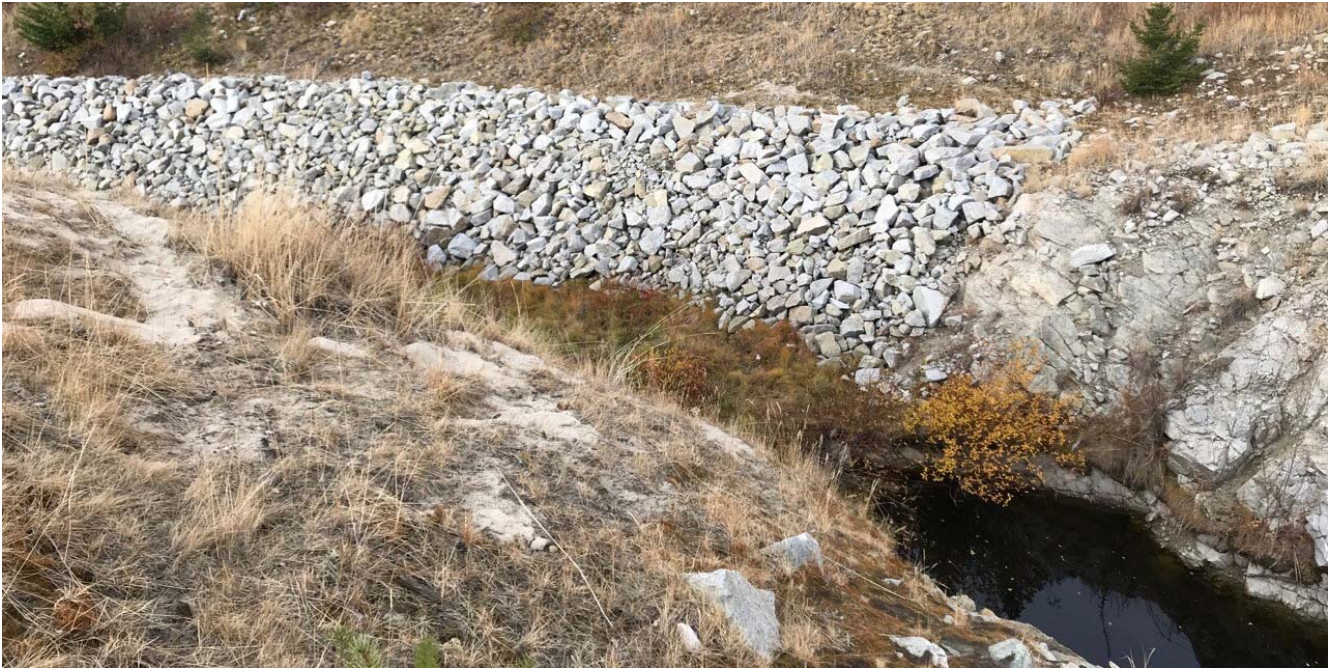
Photo II-A- 21 Transition from small rip rap to large riprap at this point where the channel grade steepens, view downstream (TRJ-2017-04)
