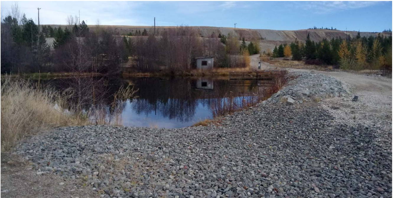
Photo II-B- 5 Transition from smaller riprap to coarser riprap as grade steepens, view upstream (TRJ-2017-16)
