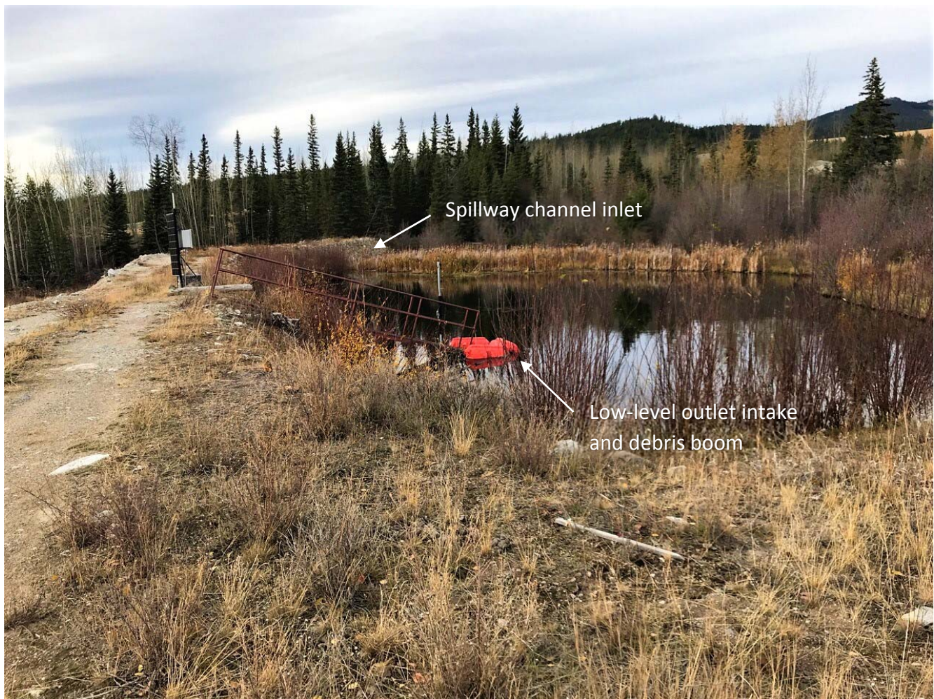
Photo II-C- 1 Overview of R4 seepage pond (TRJ-2017-20)
