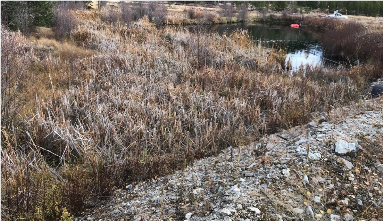
Photo II-C- 5 Spillway route filled with debris, no visible channel or flow path (TRJ-2017-24)
