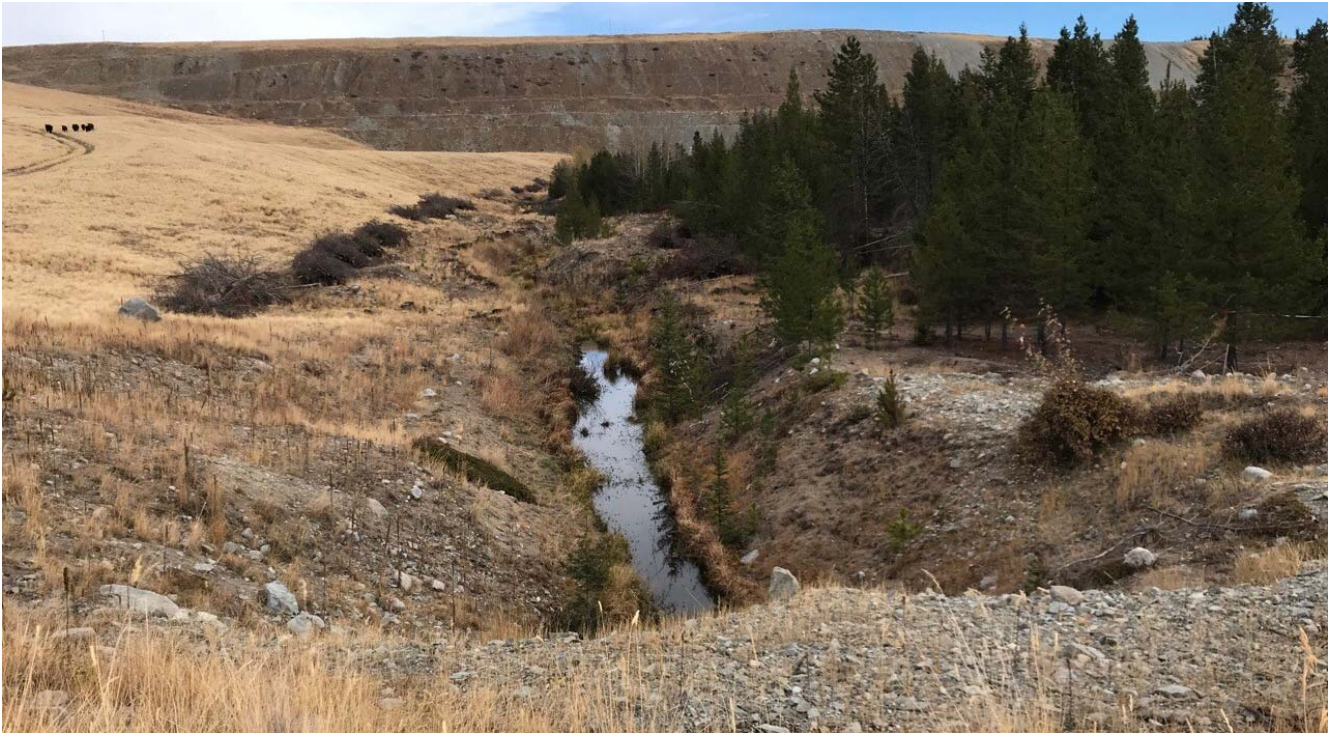
Photo II-A- 26 Seepage collection ditch view towards right abutment, flow observed (TRJ-2017-07)
