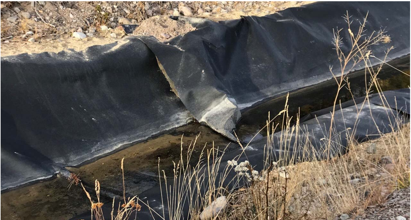
Photo II-A- 30 Damage to liner observed on diversion channel (TRJ-2017-26)
