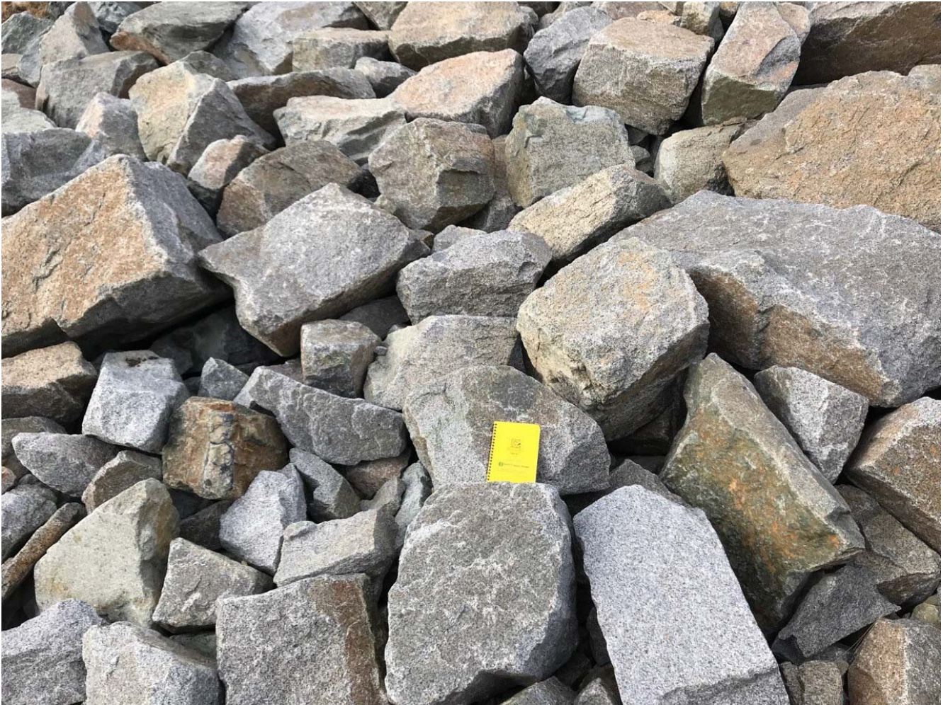
Photo II-A- 22 Overview of large riprap at transition point from large to small. Small riprap ~100mm, Coarser riprap ~150-1200mm (TRJ-2017-04)
