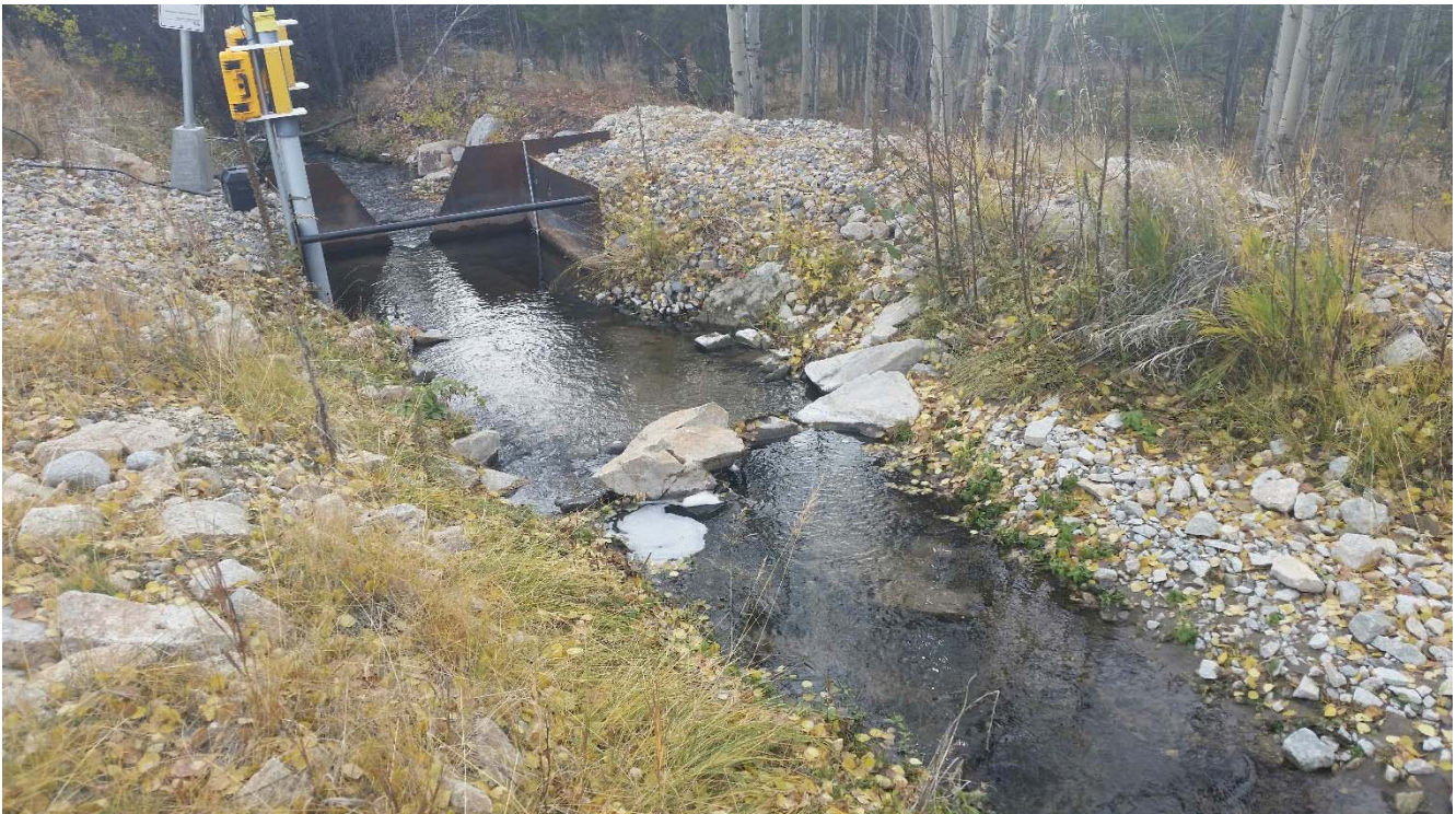
Photo II-C- 13 Discharge channel to weir, obstruction from large rocks present in channel (TRJ-2017-25)
