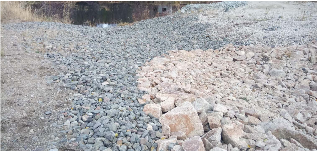
Photo II-B- 5 Transition from smaller riprap to coarser riprap as grade steepens, view upstream (TRJ-2017-16)
