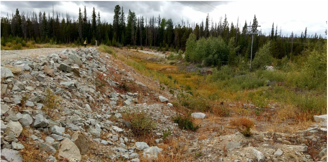
Photo II-B-5 S2: downstream slope looking from right abutment. (HGH-2017-15)
