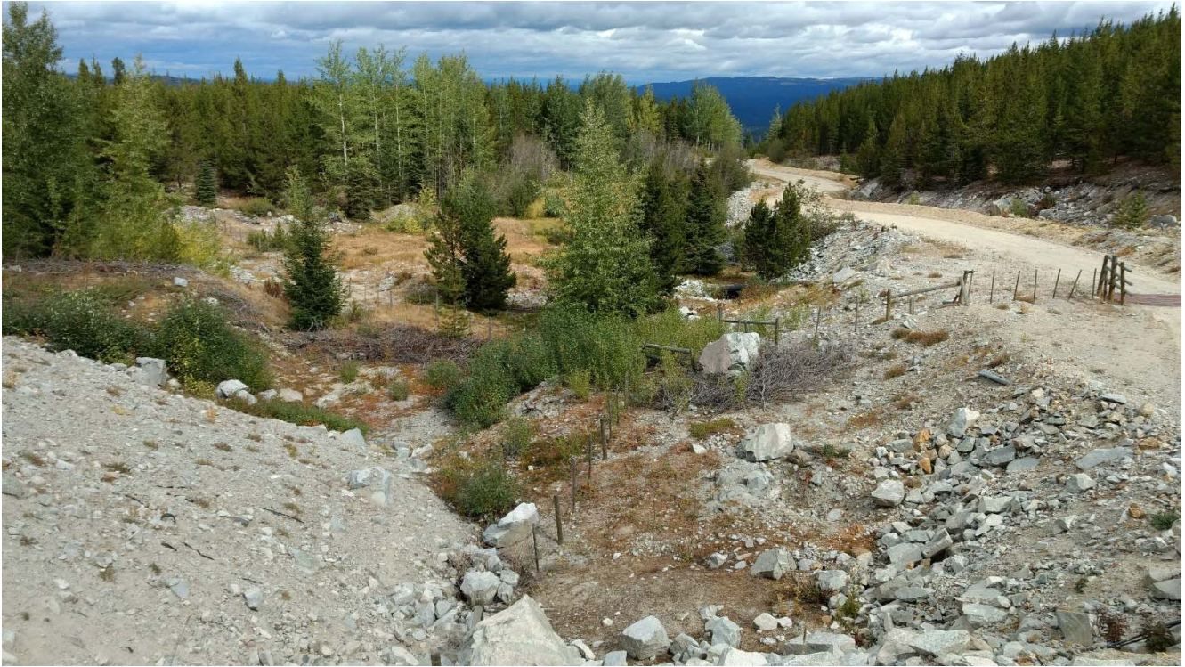
Photo II-B-18 S1: spillway outlet. (HGH-2017-27)
