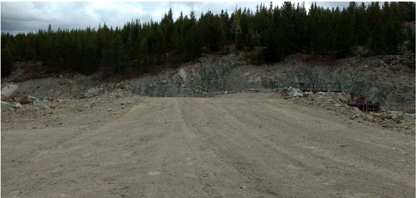
Photo II-B-15 S1: dam crest looking East towards right abutment. (HGH-2017-24)
