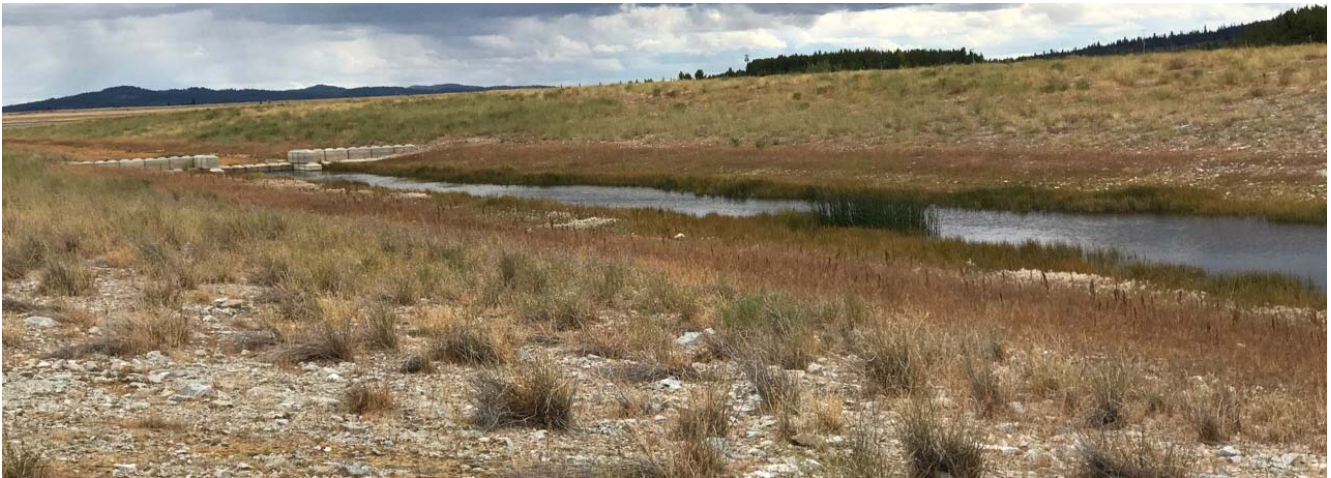
Photo II-A-4 Spillway upstream of crest, concrete lock-block control sill (HGH-2017-01)
