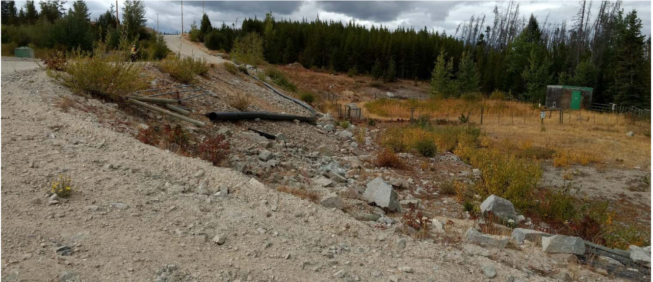
Photo II-B-11 S8: downstream slope looking West from right abutment. (HGH-2017-18)
