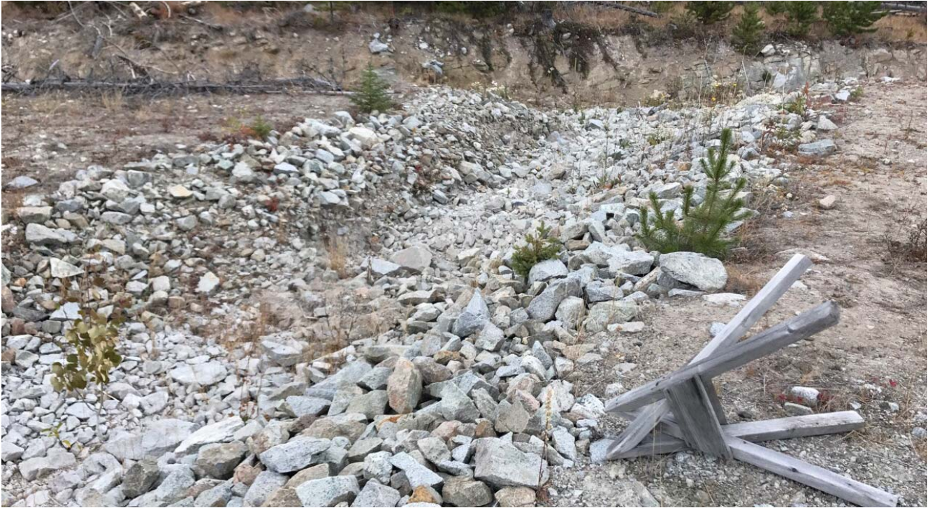
Photo II-B-8 S2: spillway looking downstream to tie-in with Highmont spillway. (HGH-2017-13)
