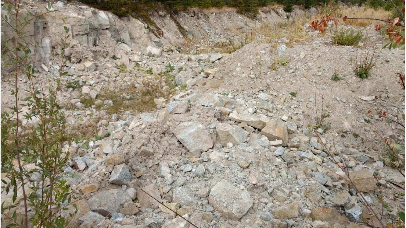
Photo II-A-14 Spillway channel till plug (HGH-2017-12)
