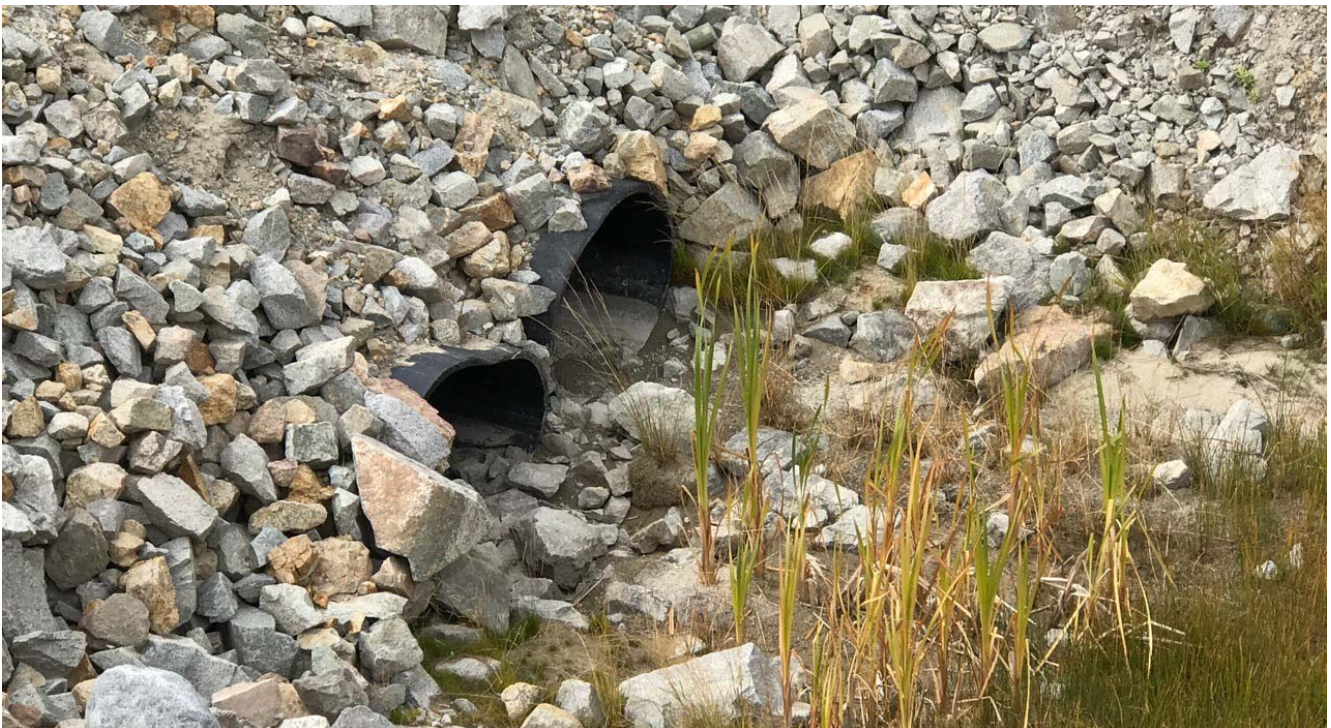
Photo II-A-12 Downstream side of 33" ID spillway road culverts, showing vegetation (HGH-2017-09)
