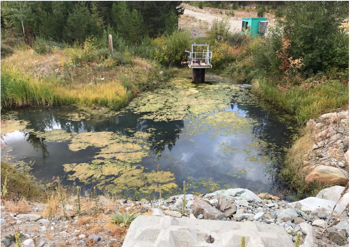
Photo II-B-21 S5: pumping cell with outlet pump to S1 pond. (HGH-2017-36)
