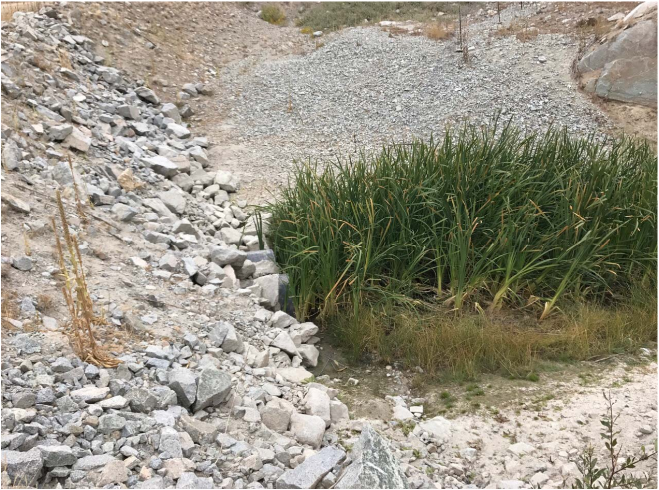
Photo II-A-6 Spillway culverts, downstream side of crest, vegetated (HGH-2017-02)
