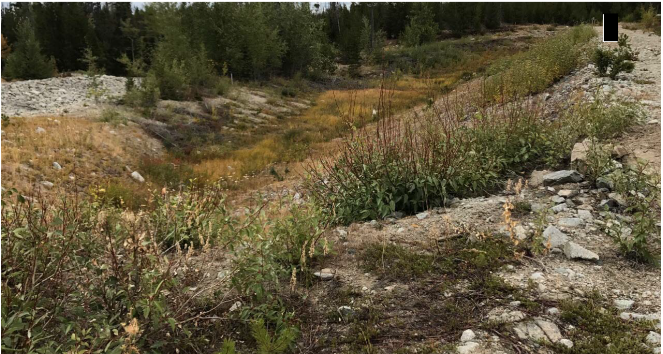
Photo II-B-3 S2: downstream slope looking from left abutment. (HGH-2017-13)
