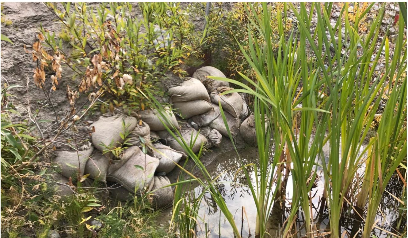
Photo II-B-26 S5: spillway pipes (2x), inlet currently blocked with sand bags. (HGH-2017-37)
