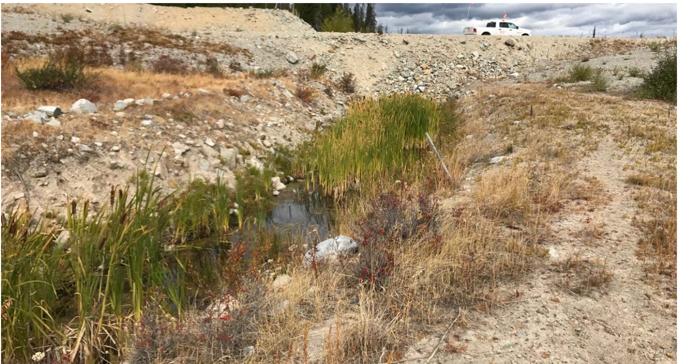
Photo II-A-10 Spillway channel looking downstream, vegetated showing standing water (HGH-2017-06)
