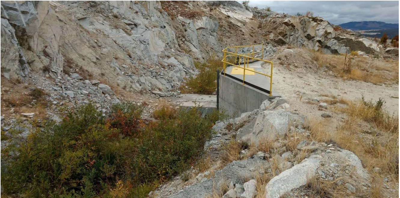
Photo II-A-9 Spillway channel looking downstream at inlet to Seepage Recovery Pond S1 pipeline division, showing trashrack on invert (HGH-2017-04)
