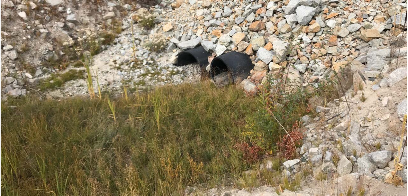
Photo II-A-12 Downstream side of 33" ID spillway road culverts, showing vegetation (HGH-2017-09)
