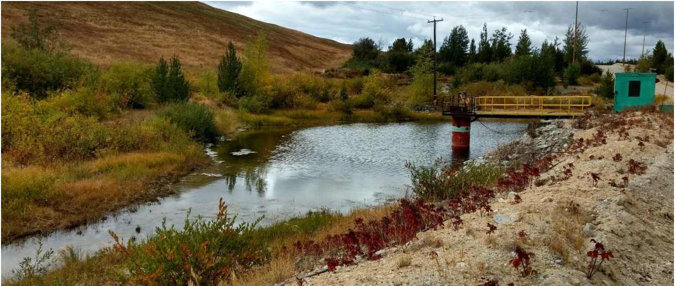
Photo II-B-9 S8: pond overview with pumphouse to S1 pond (right of photo) and North Dam downstream slope in background. (HGH-2017-18)
