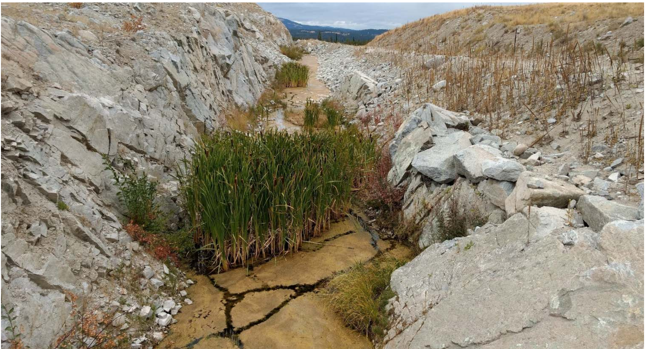
Photo II-A-8 Spillway channel looking downstream from the flow control gate (HGH-2017-03)
