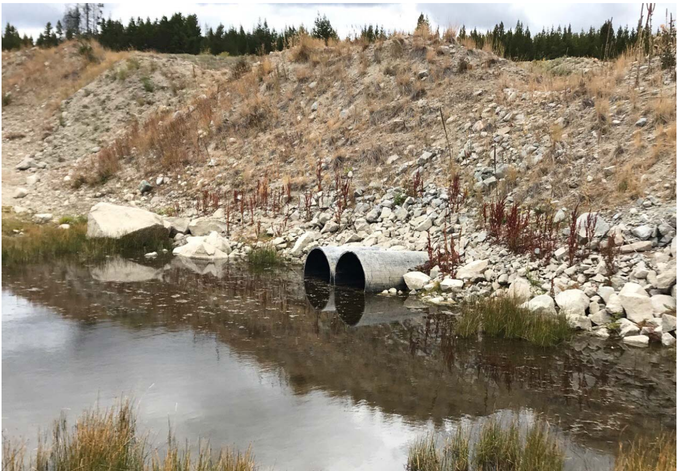
Photo II-A-5 Spillway culverts, upstream side of crest, submerged (HGH-2017-01)
