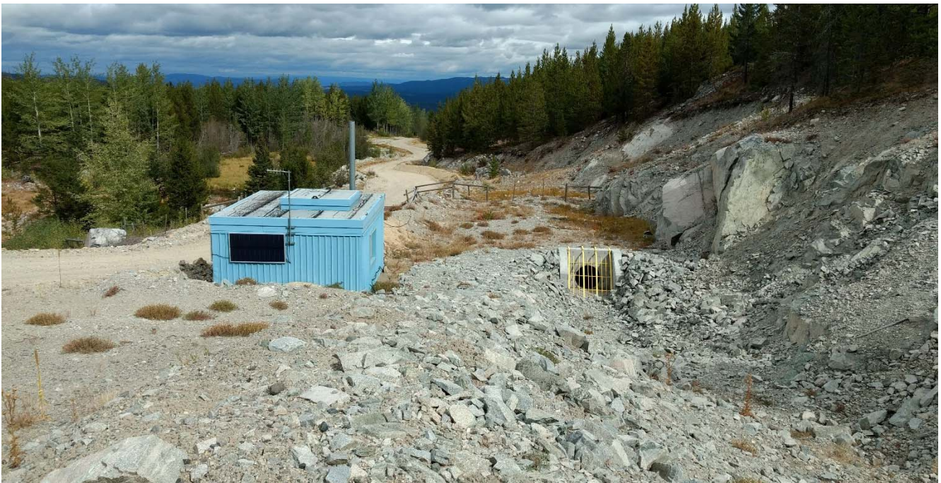
Photo II-B-17 S1: spillway channel and pipe intake looking downstream. (HGH-2017-28)
