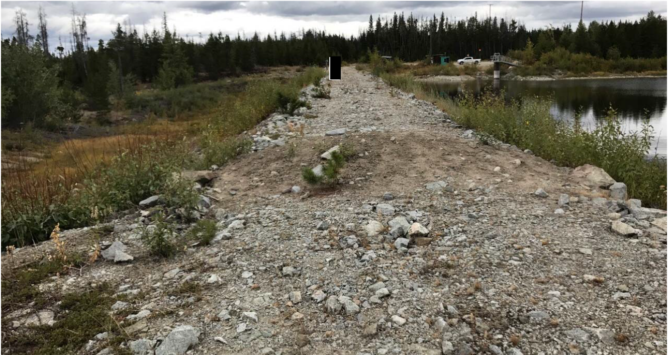
Photo II-B-2 S2: dam crest, looking from left abutment. (HGH-2017-13)
