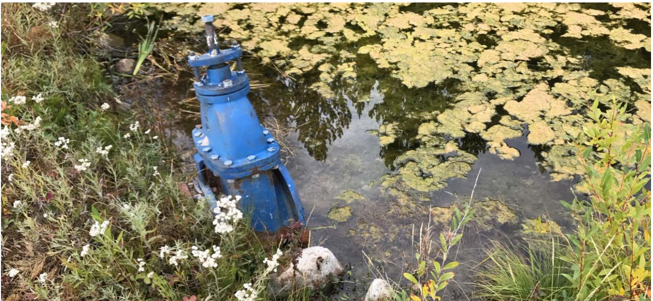
Photo II-B-24 S5: intake of pipe connecting perimeter pond to pumping cell. (HGH-2017-34)
