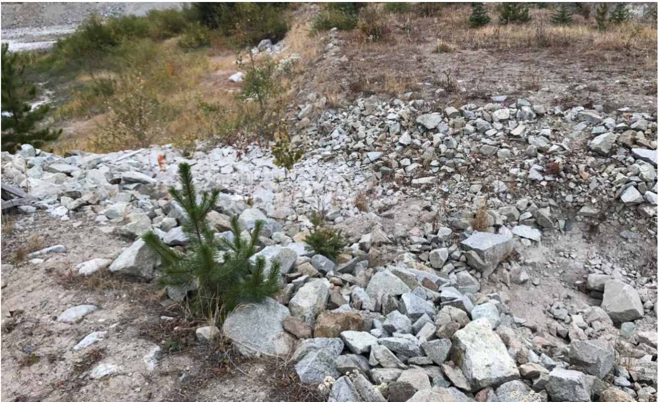
Photo II-B-7 S2: spillway looking upstream towards pond. (HGH-2017-13)
