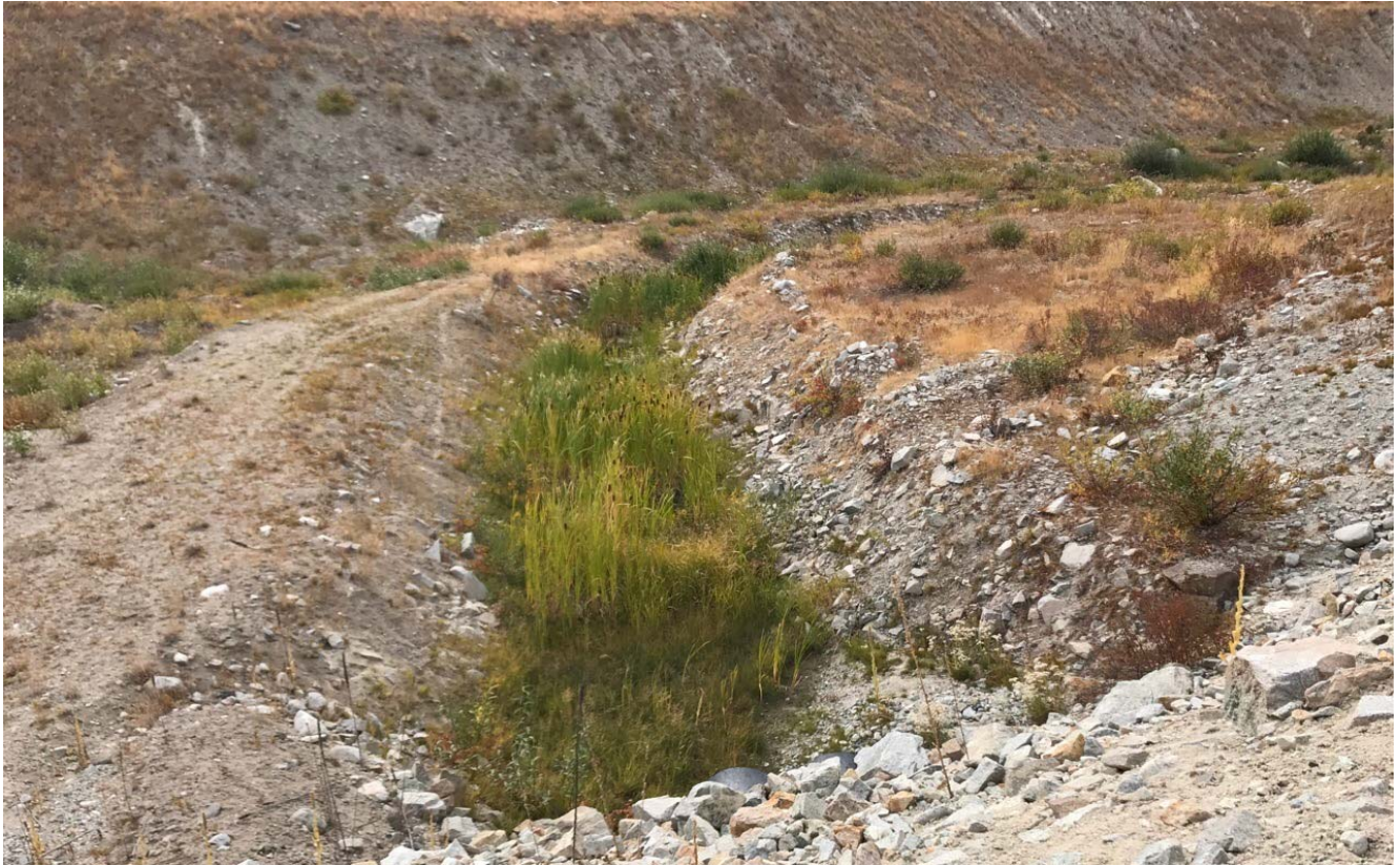
Photo II-A-13 Spillway channel looking downstream from road (HGH-2017-09)
