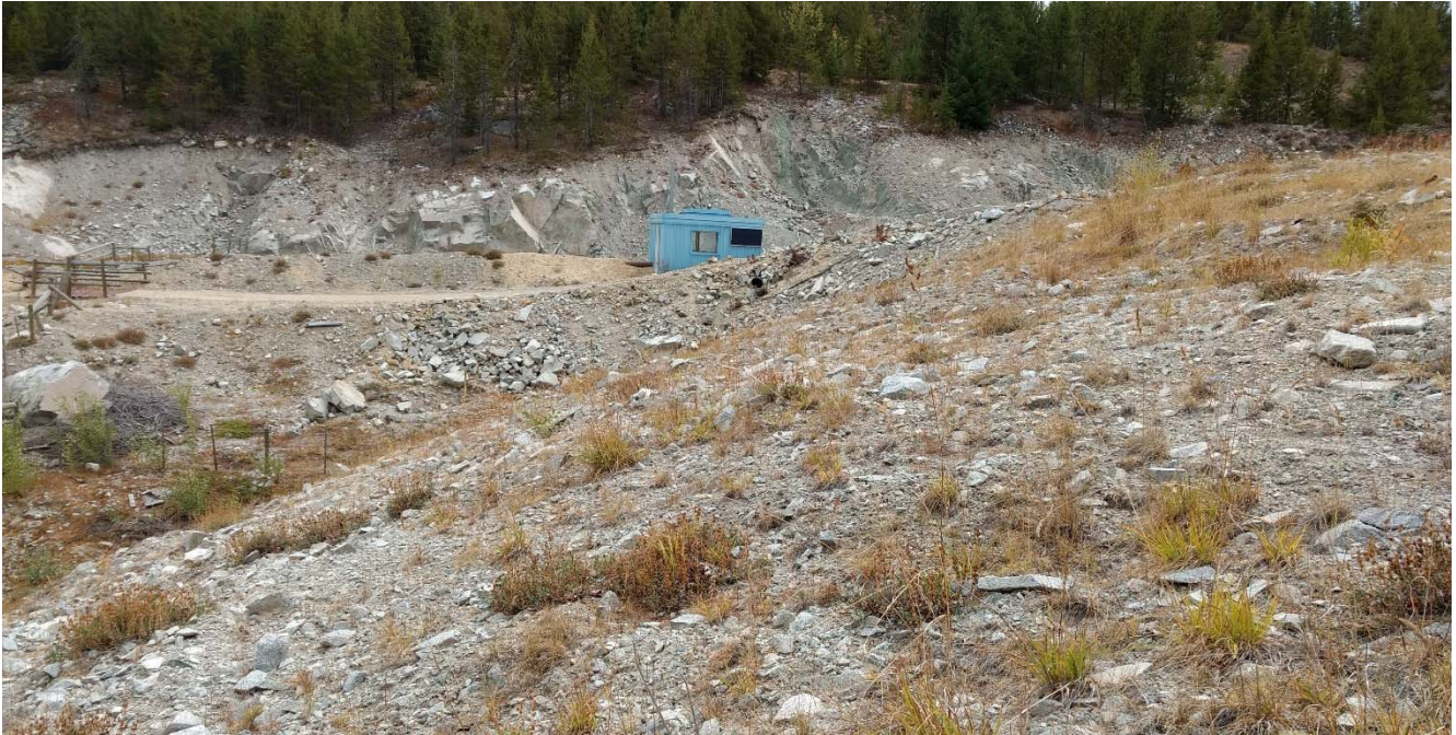
Photo II-B-16 S1: downstream slope looking East toward spillway. (HGH-2017-29)
