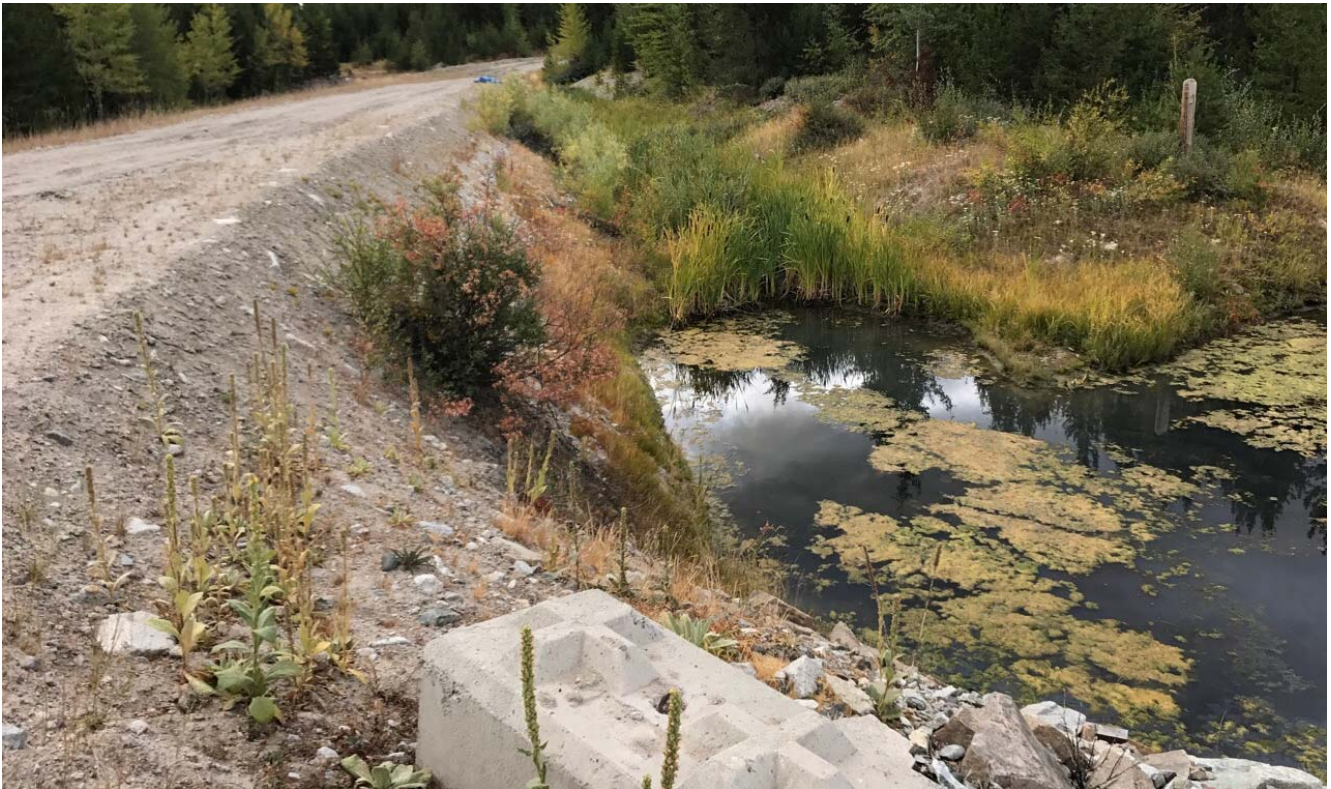
Photo II-B-23 S5: pumping cell looking South towards outlet channel and spillway. (HGH-2017-36)
