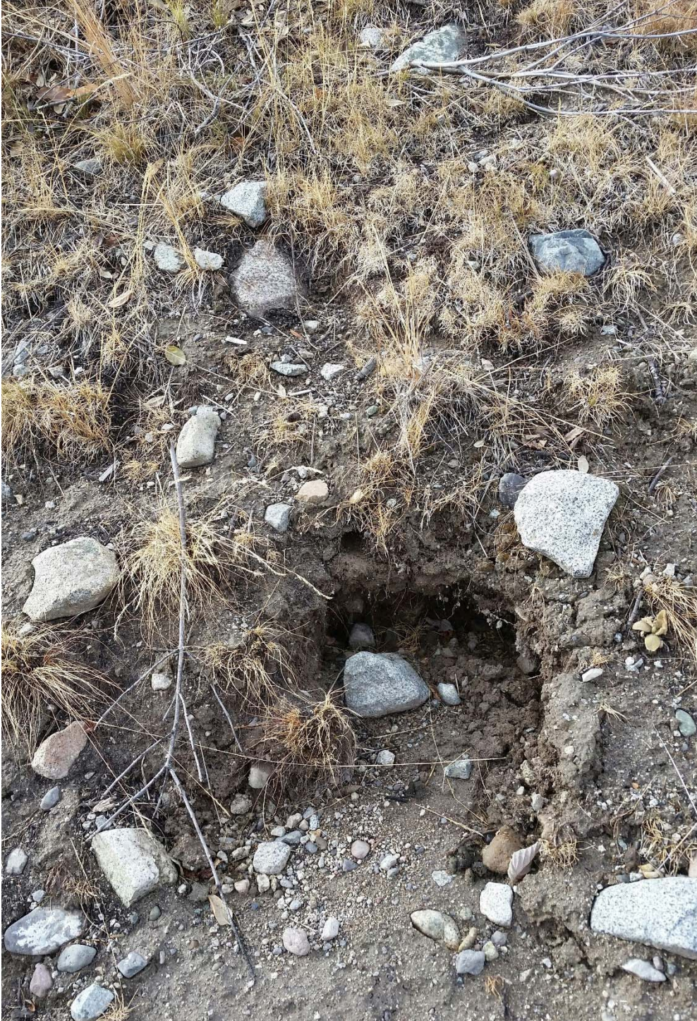
Photo II-B-23 Possible animal burrow site near right dam abutment. (BTH-2017-09)
