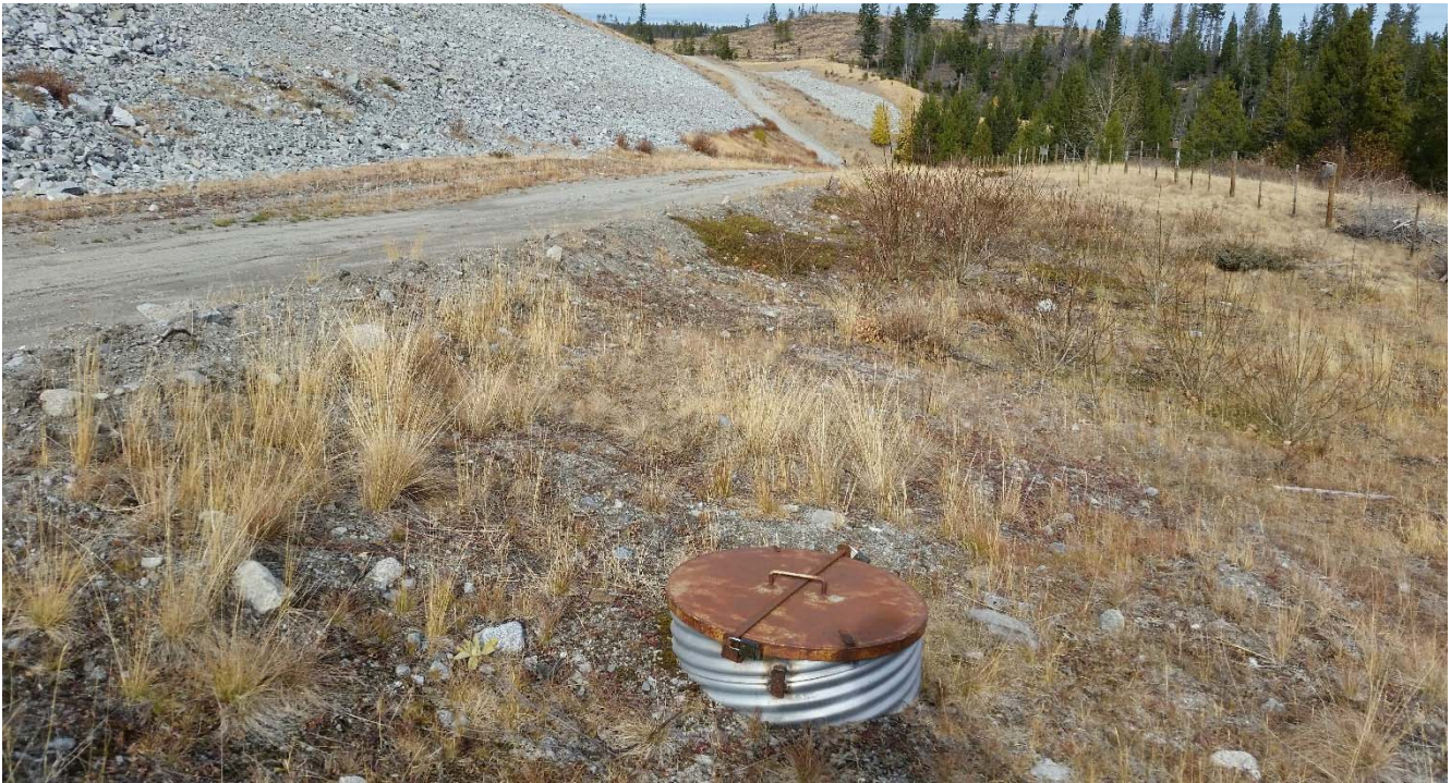
Photo II-B-6 Toe drain, no visible damage, view towards left abutment (BTH-2017-11)
