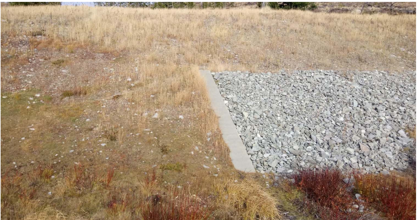
Photo II-B-13 Spillway channel transition point from till to riprap lining. Concrete sill shows no signs of damage or cracking, and the slope shows no signs of erosion (BTH-2017-16)
