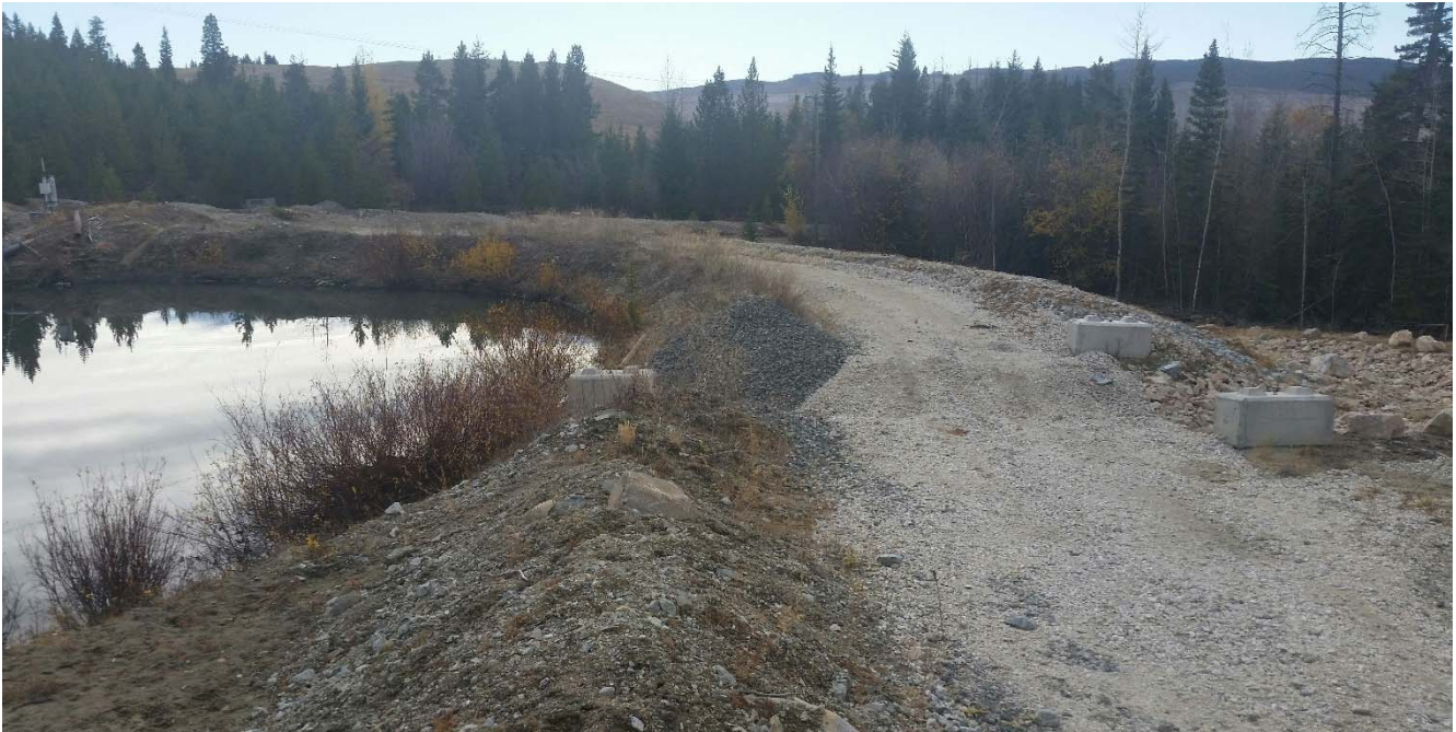
Photo II-C-4 Dam crest view towards left abutment and spillway swale, Uneven ground where spillway cuts through dam crest (BTH-2017-23)
