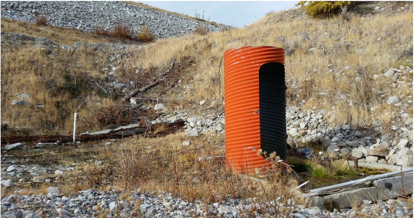
Photo II-B-9 Old gauge-house and decommissioned pump-well. Piezometer 1 standpipe visible on the left, directly behind gauge-house (BTH-2017-13)
