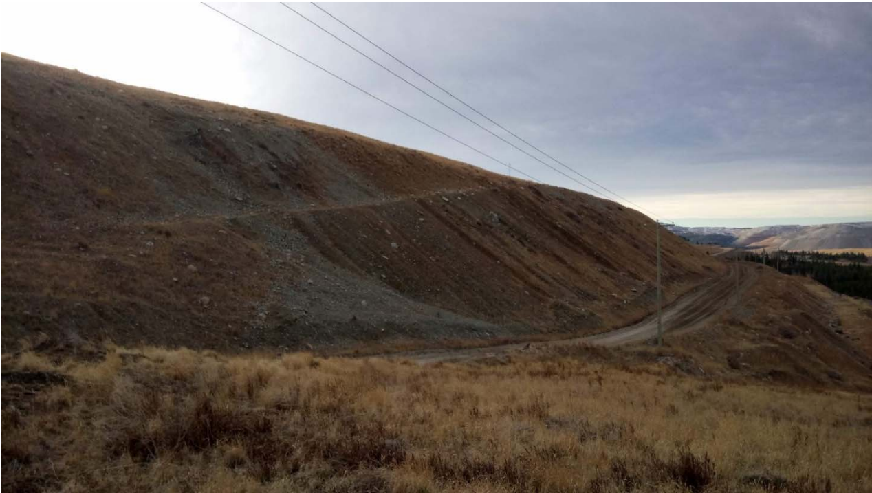
Photo II-A-6 Downstream slope of dam, view looking south (BTH-2017-05)
