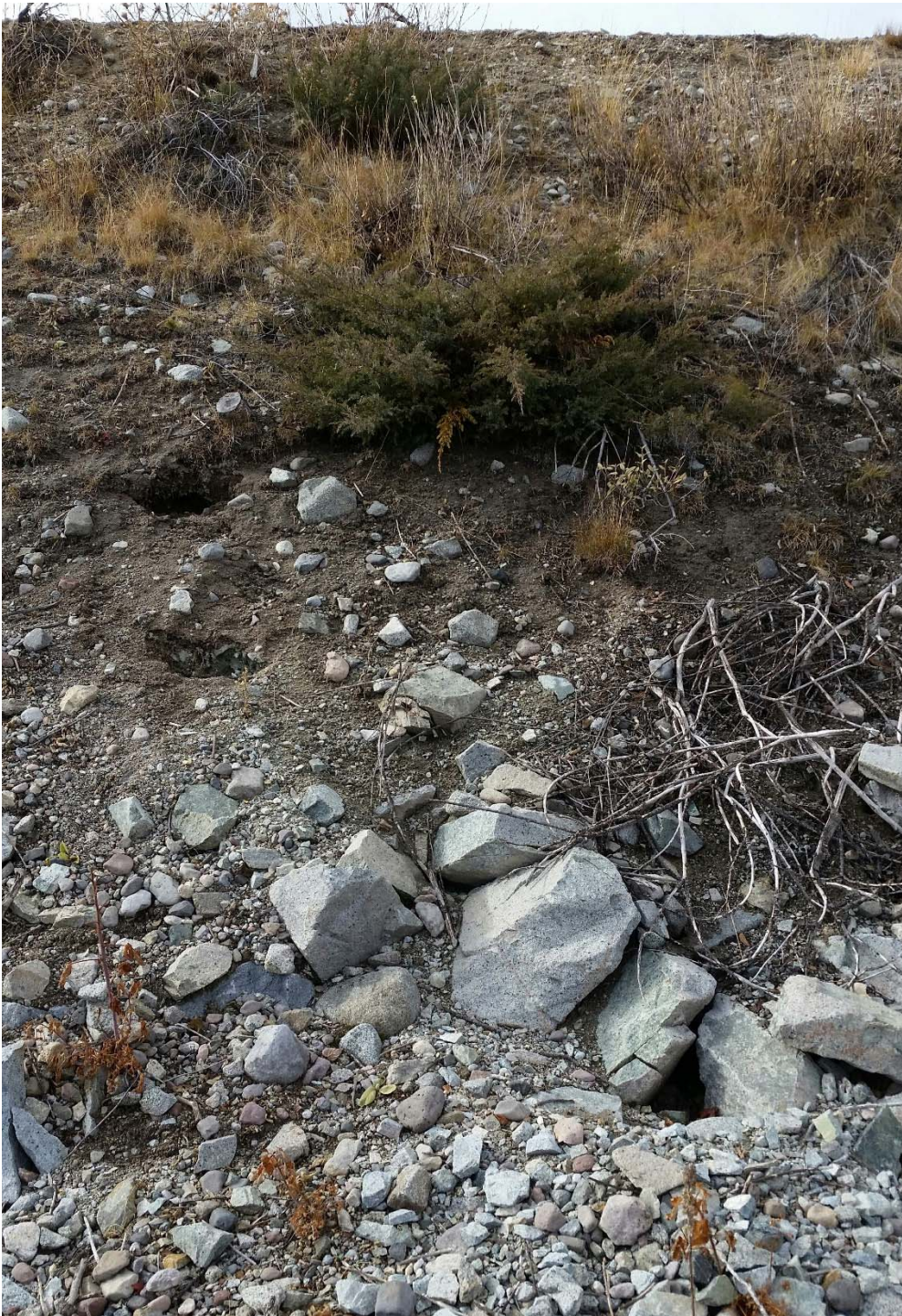
Photo II-B-22 Possible animal burrow site near dam left abutment (BTH-2017-14)
