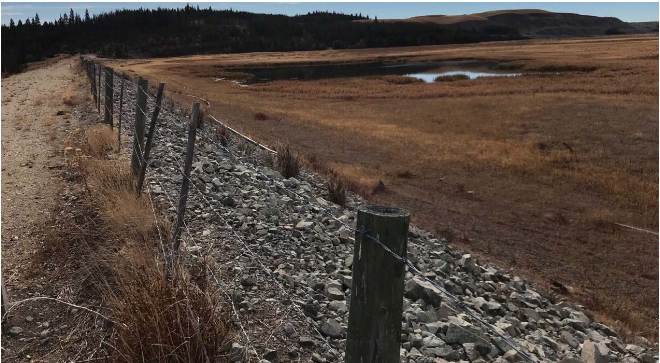
Photo II-B-19 View of upstream slope and tailings pond, no signs of erosion observed (BTH-2017-20)
