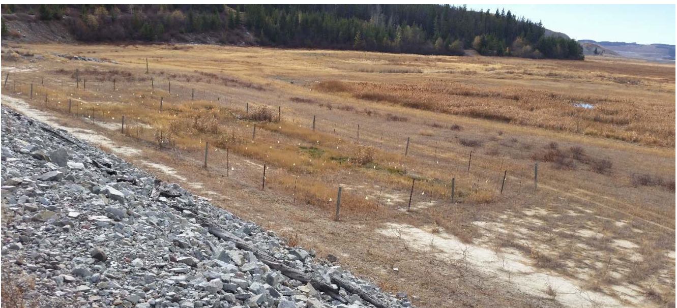
Photo II-B-21 View of fenced off reclamation area from crest of dam (BTH-2017-22)
