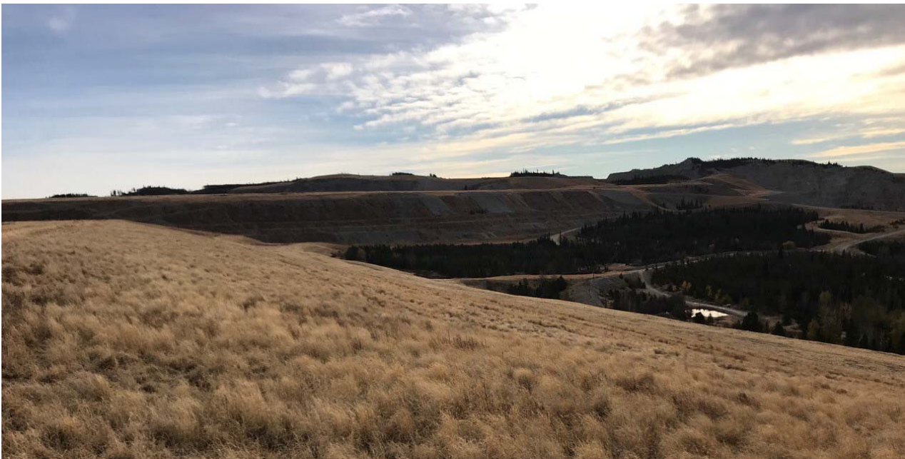
Photo II-A-7 Downstream slope of dam, view looking east from Trojan Dam crest (BTH-2017-06)
