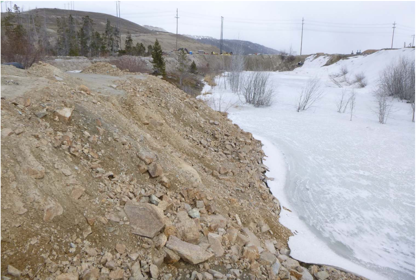
Photo II-7 Ponding in southern treed area looking west (SDP-2017-05)
