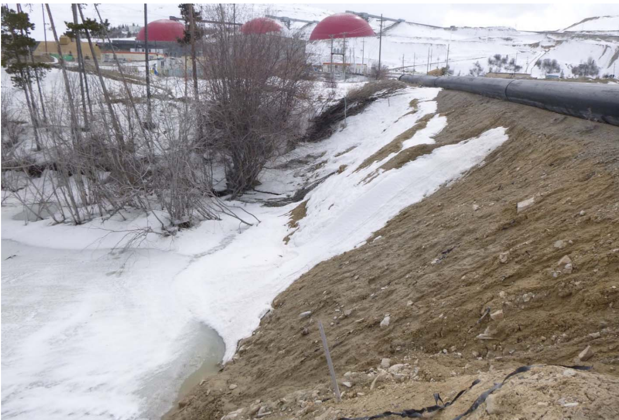
Photo II-6 Downstream slope of east embankment looking at southern treed area with ponding at toe (SDP-2017-05)
