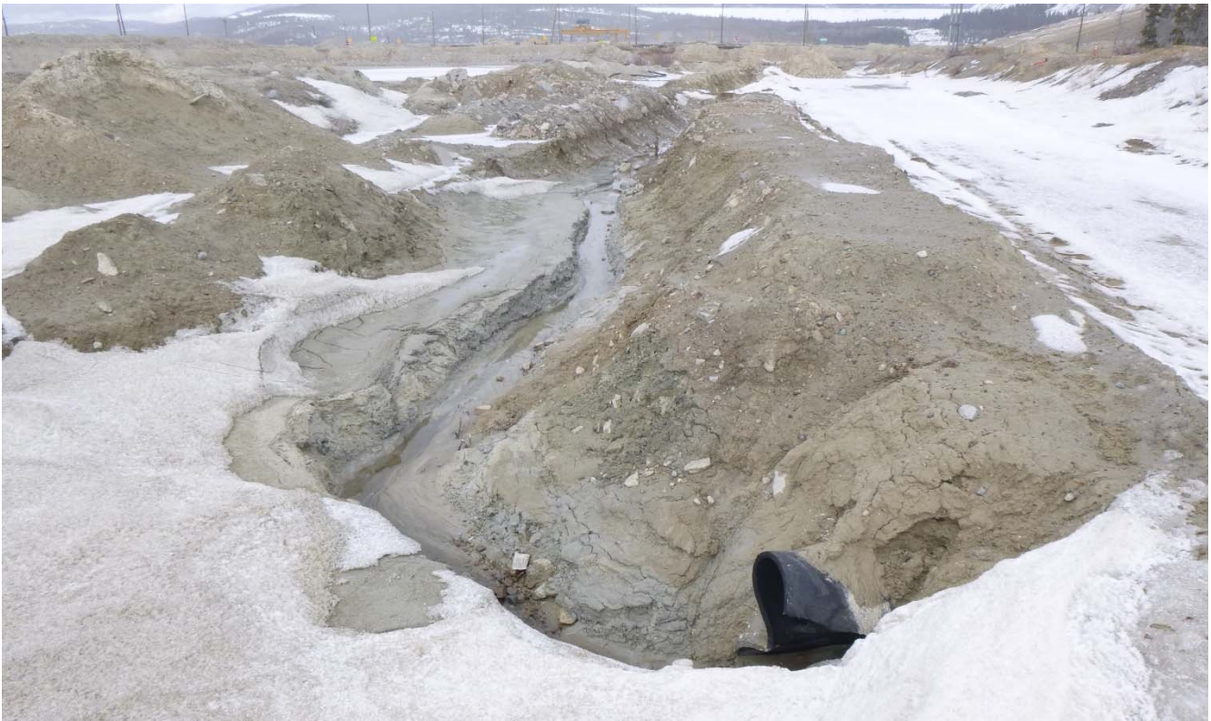
Photo II-10 Disconnected segment of pipe, partially buried along eastern embankment. Photo taken looking northwest (SDP-2017-04)
