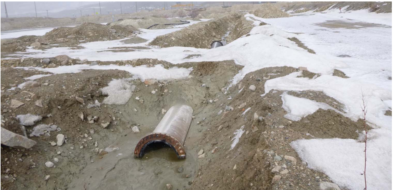
Photo II-10 Disconnected segment of pipe, partially buried along eastern embankment. Photo taken looking northwest (SDP-2017-04)
