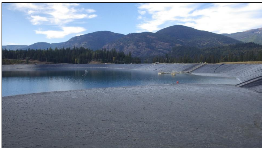
PHOTO 9 – North side of tailings basin from the east.
