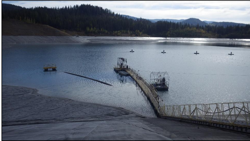
PHOTO 4 – Reclaim barge, access gangway and floating evaporators.
