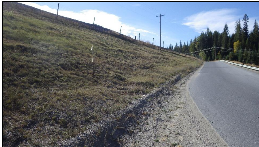
PHOTO 26 – Downstream slope of Northwest Dam.
