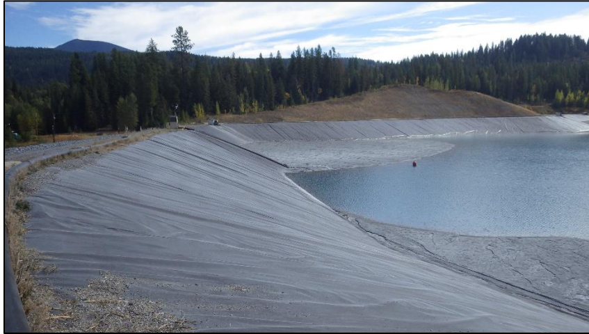
PHOTO 7 – Northeast geomembrane lined slope.
