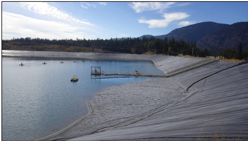
PHOTO 5 – Reclaim barge and evaporators from the east.
