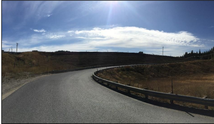
PHOTO 25 – Mine access road and downstream slope of Northwest Dam.
