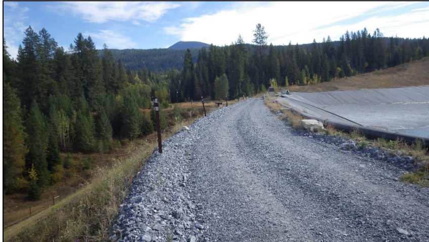
PHOTO 19 – Northeast perimeter road and dam crest.
