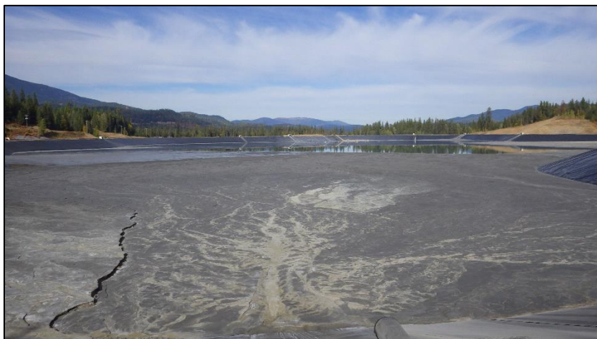
PHOTO 12 – E4 discharge location looking north.
