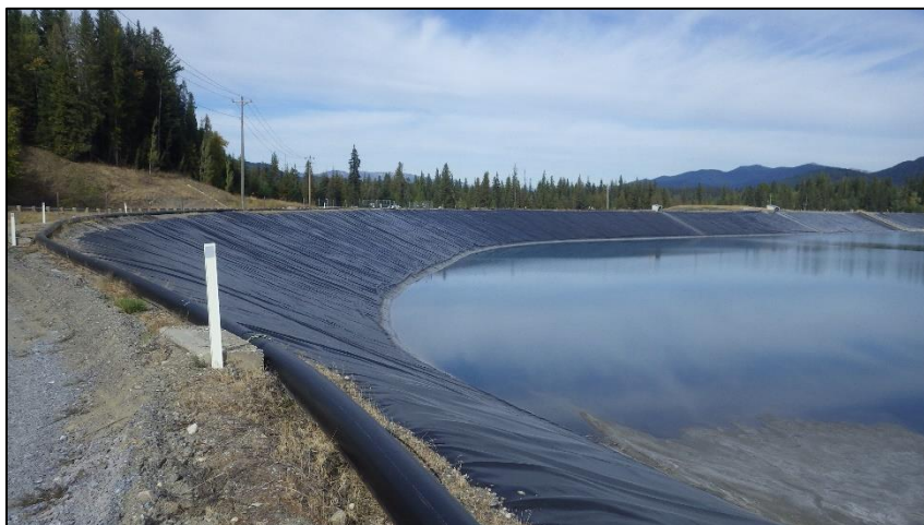
PHOTO 15 – View of northwest tailings basin from the west.
