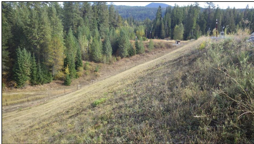
PHOTO 23 – Downstream face of Northeast Dam.
