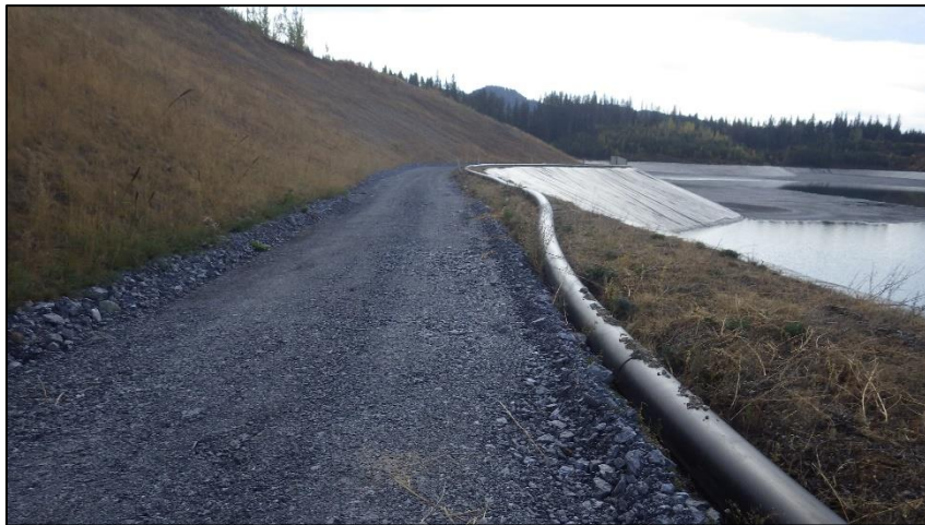
PHOTO 20 – Eastern perimeter road around tailings basin.
