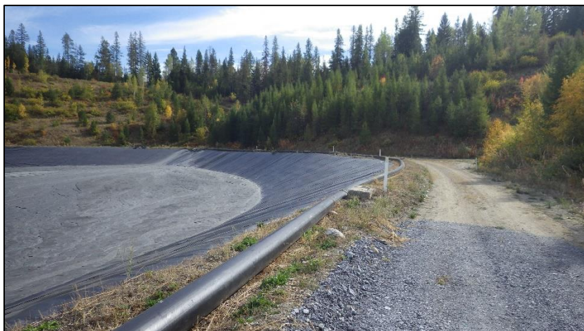
PHOTO 21 – Southern perimeter road around tailings basin.
