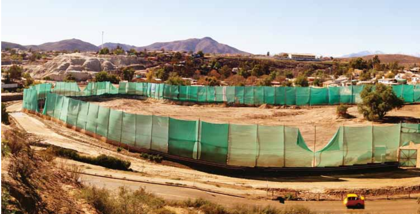
Cleanup underway of legacy tailings, unrelated to Teck operations, at Andacollo
