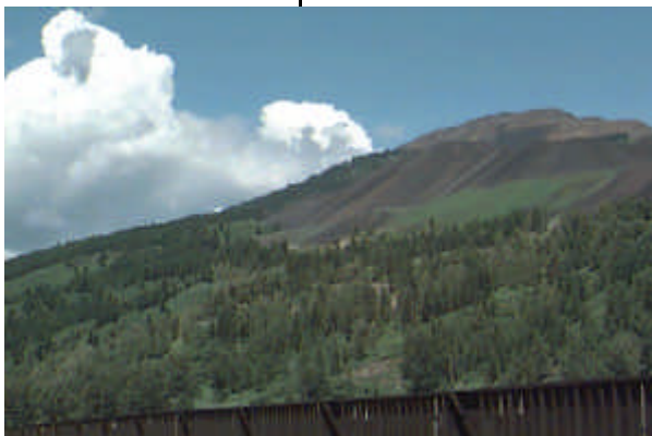
Early stages of reclamation of the Bodie Dump
