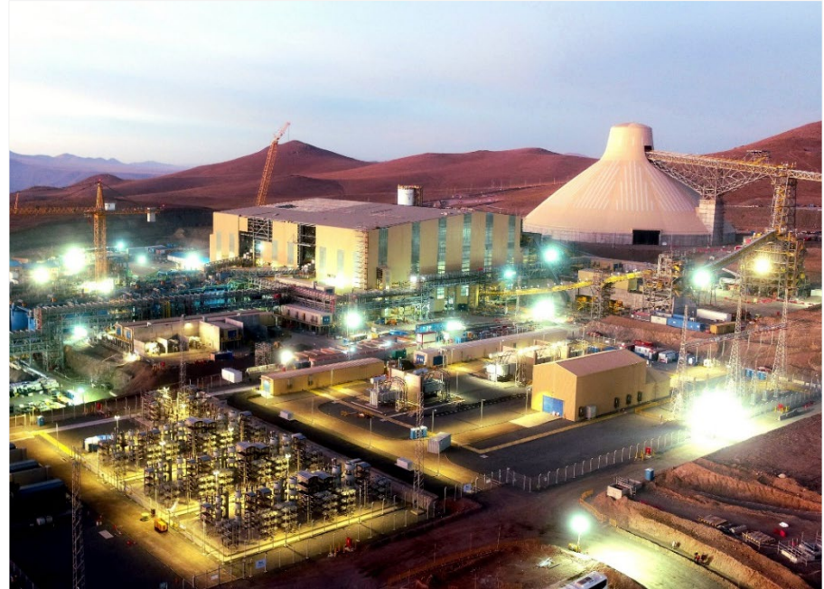
Concentrator substation, flotation area, grinding building, and ore stockpile dome
