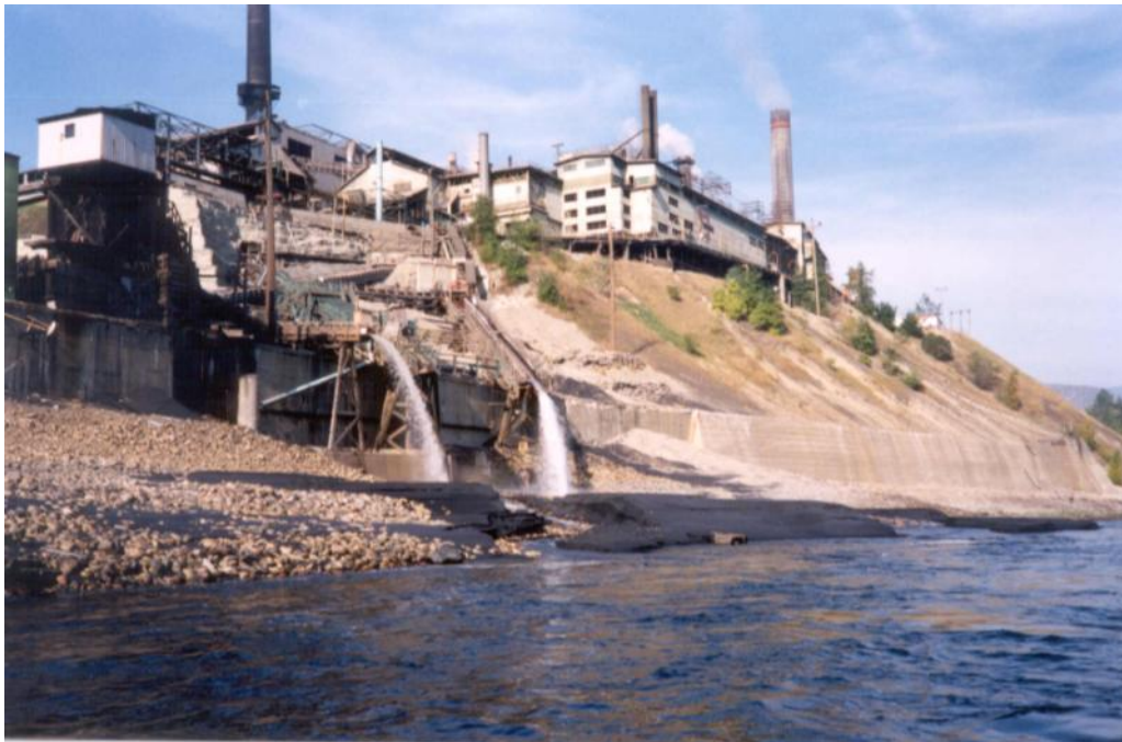
Figure 4.5 Historic Discharge of Slag to the Columbia River (Pre-1995 and Installation of Kivcet Smelter)
