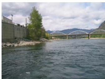
Near the New Bridge site
