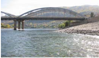
The New Bridge site
