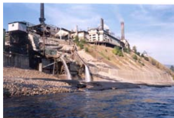
Historic discharge of slag to the Columbia River (pre-1995 and installation of Kivcet Smelter)
